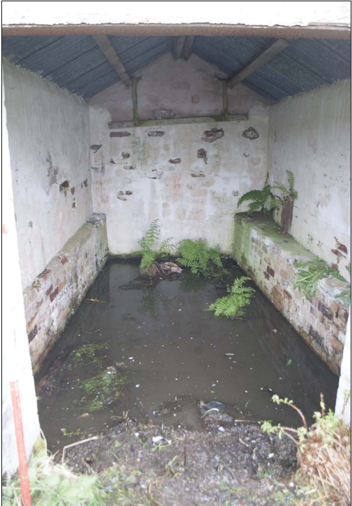
Plate 19: View of the interior of the boat house showing the ledge and tie-post for the boat; scale: 1x1m (archive reference: G2580_051).
