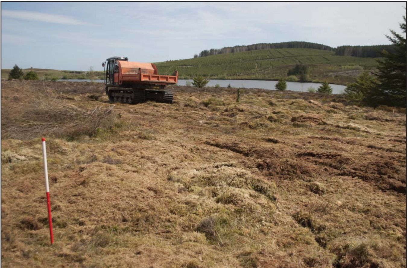
Plate 8: General view of compound area levelling with a tracked dumper; scale 1x1m; view from NW (archive reference: G2580_071).
