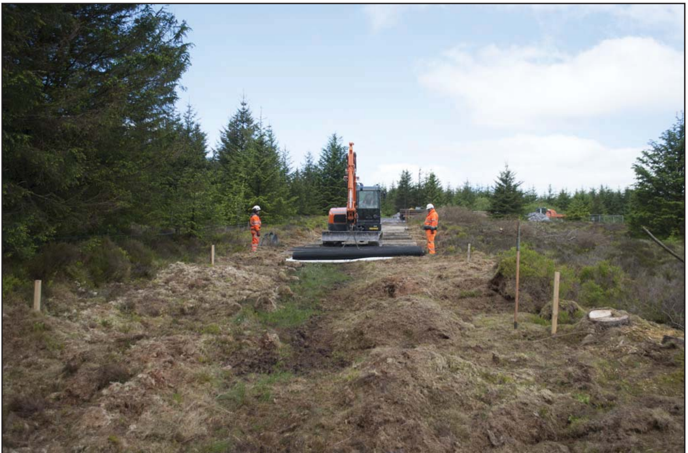
Plate 14: General view showing the laying of log matting; scale not used; view from E (archive reference: G2580_080).
