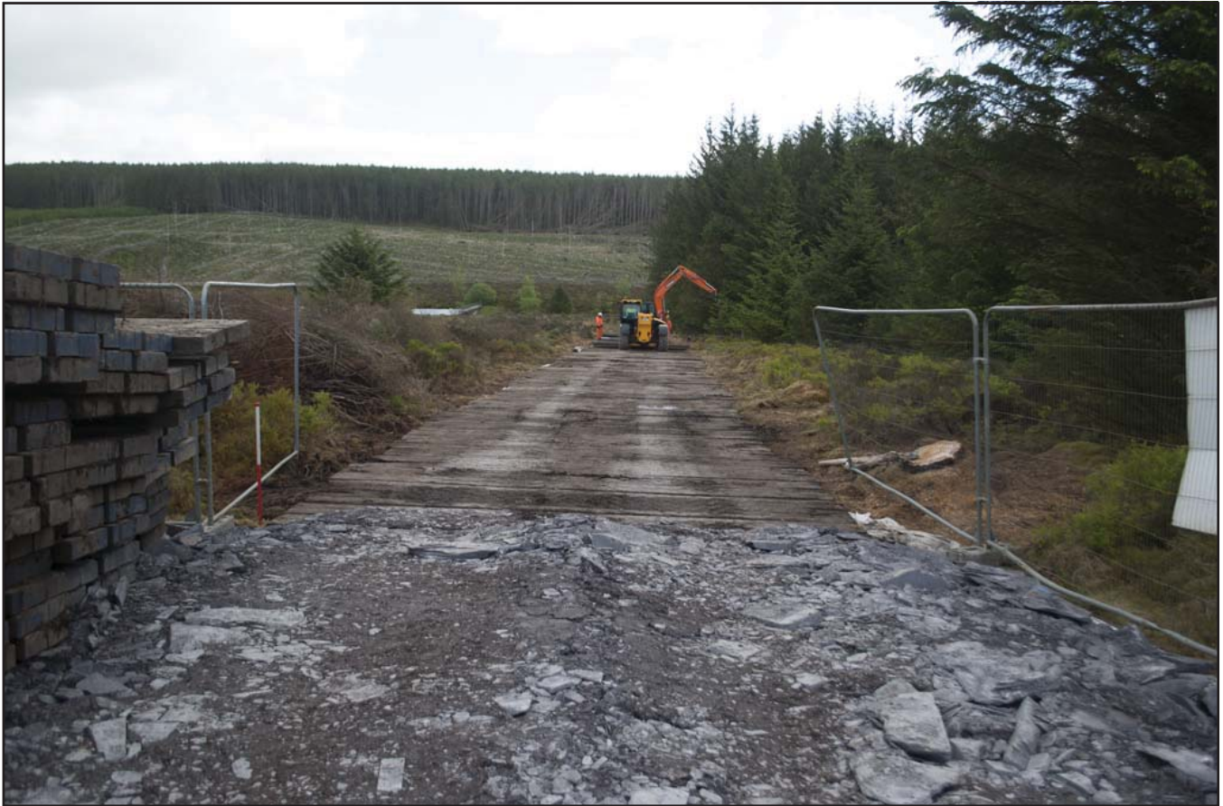
Plate 13: View of bog matting in place at west end of the track; scale not used; view from W (archive reference: G2580_079).
