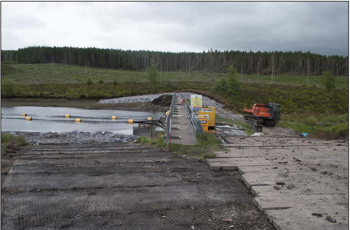
Plate 34: General view of the dam showing areas of chippings and log mats; scale 1x1m; view from W (archive reference: G2580_113).
