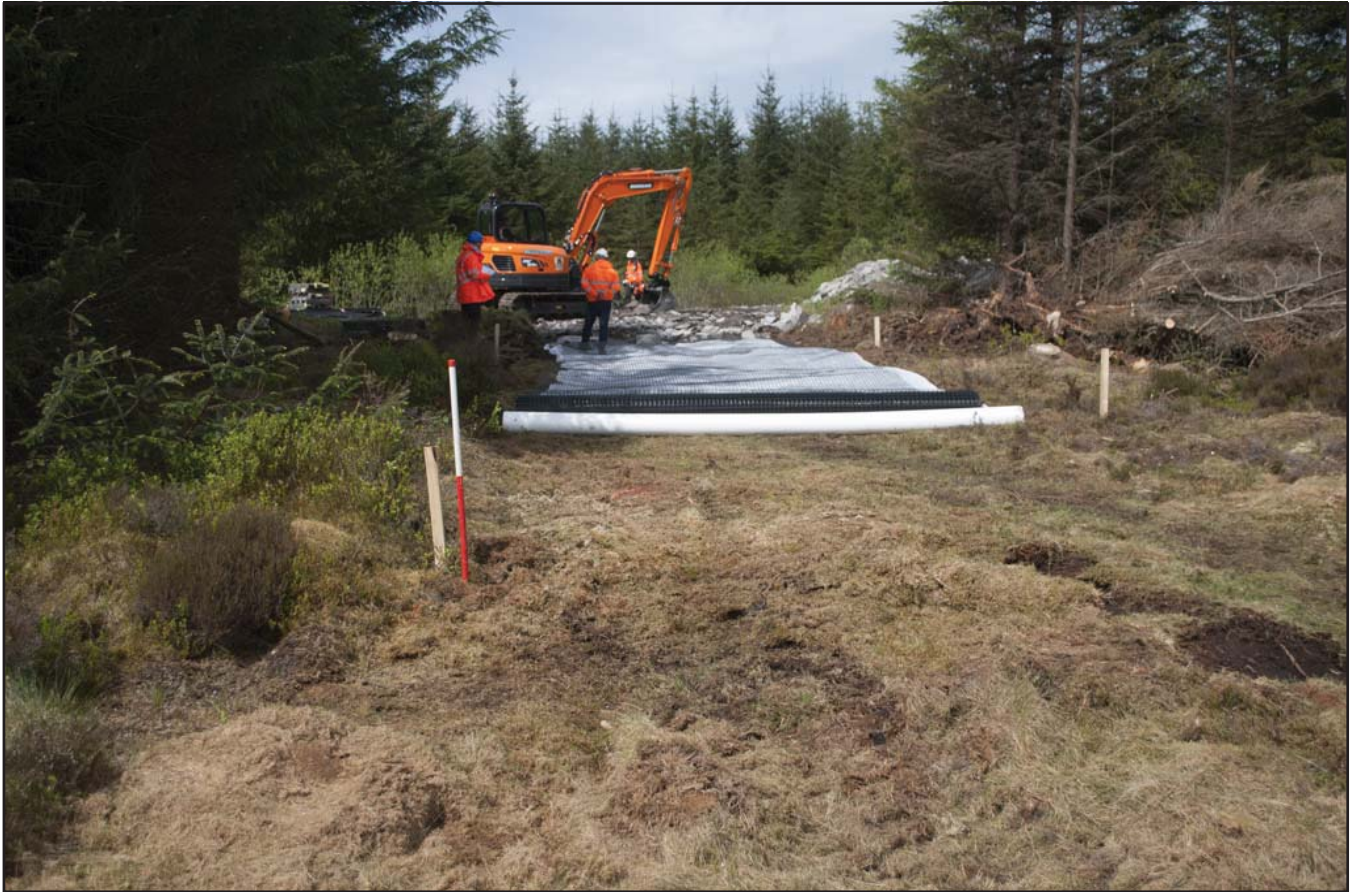
Plate 9: General view of trackway stoning up over log mats; scale 1x1m; view from E (archive reference: G2580_072).
