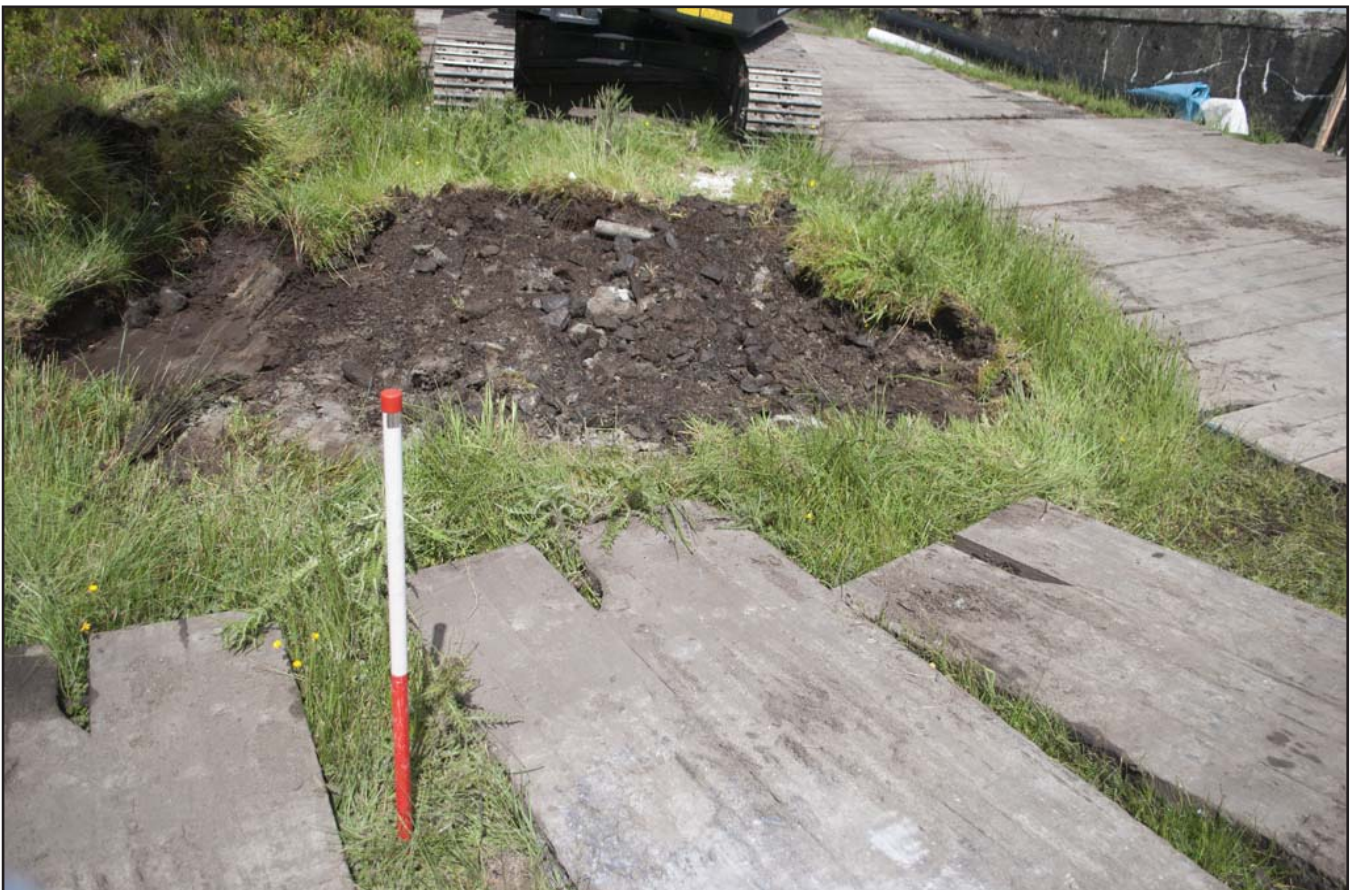
Plate 20: Action shot showing the removal of the grassy mound; scale 1x1m; view from SE (archive reference: G2580_087).
