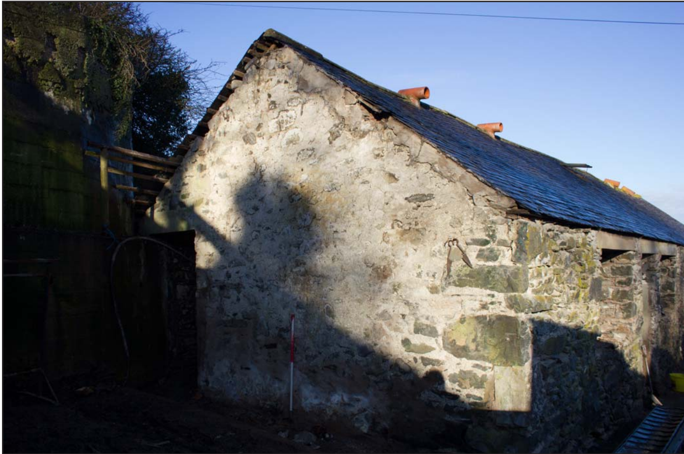
Plate 01: South facing external elevation, from the southeast. Scale 1.0m.
