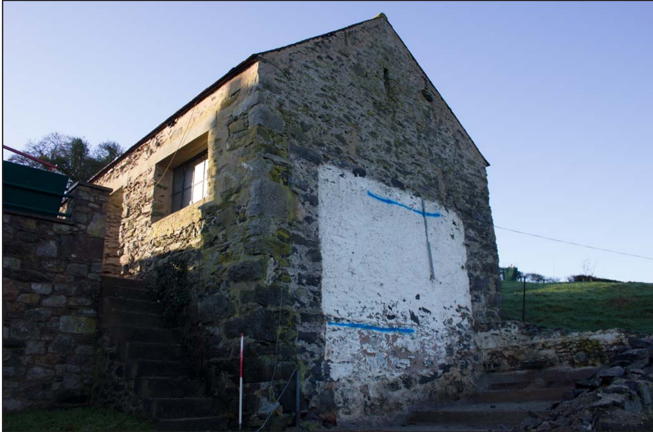
Plate 05: East and north facing external elevations, from the northeast. Scale 1.0m.
