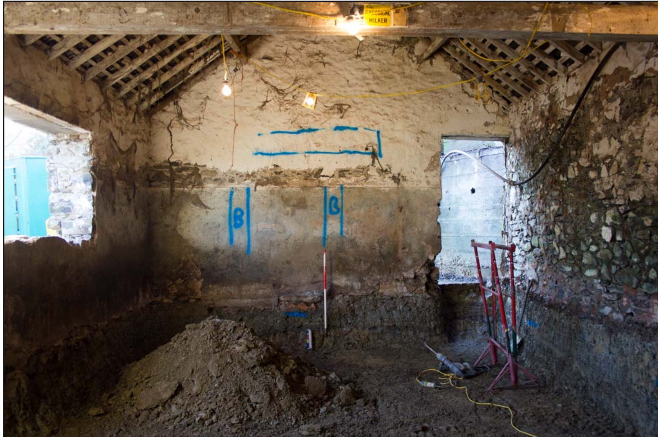
Plate 17: Room 3, from the north. Scale 1.0m.
