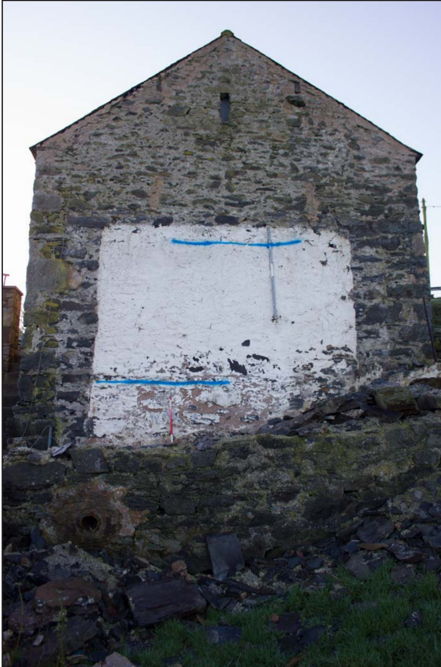
Plate 06: North facing external elevation, from the north. Scale 1.0m.
