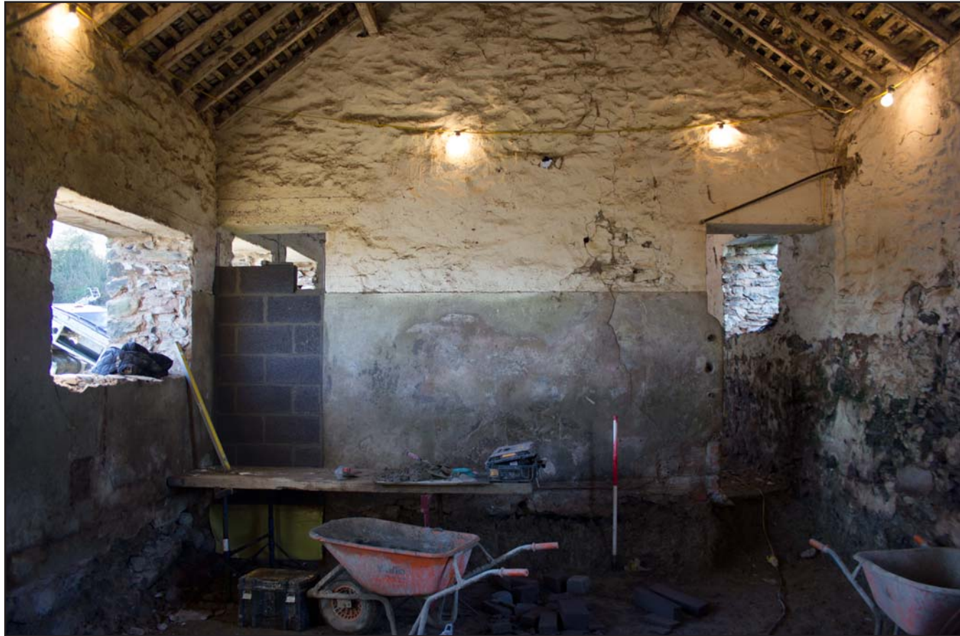
Plate 12: Room 1, from the north. Scale 1.0m.
