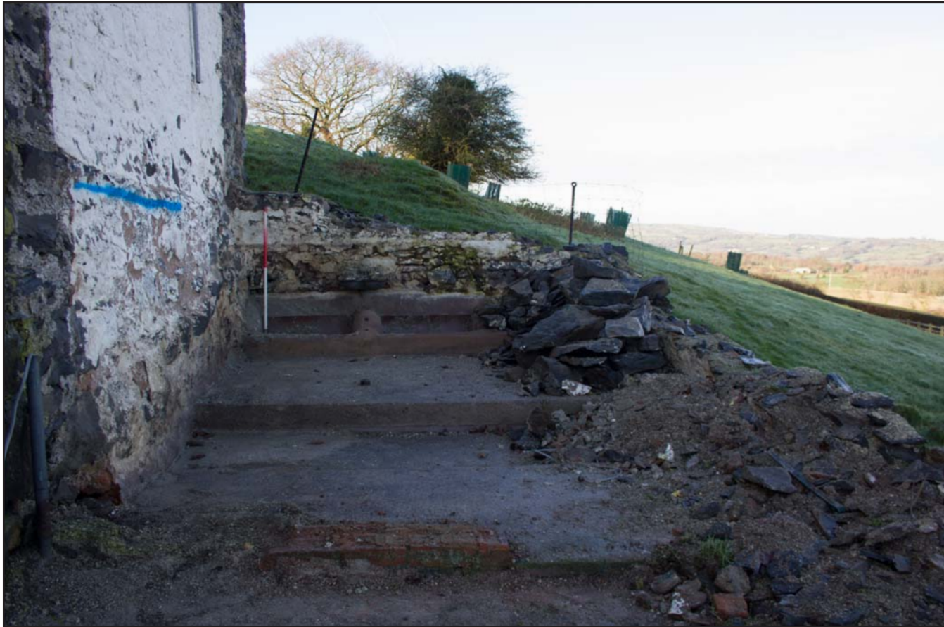
Plate 10: Demolished lean-to store, from the east. Scale 1.0m.
