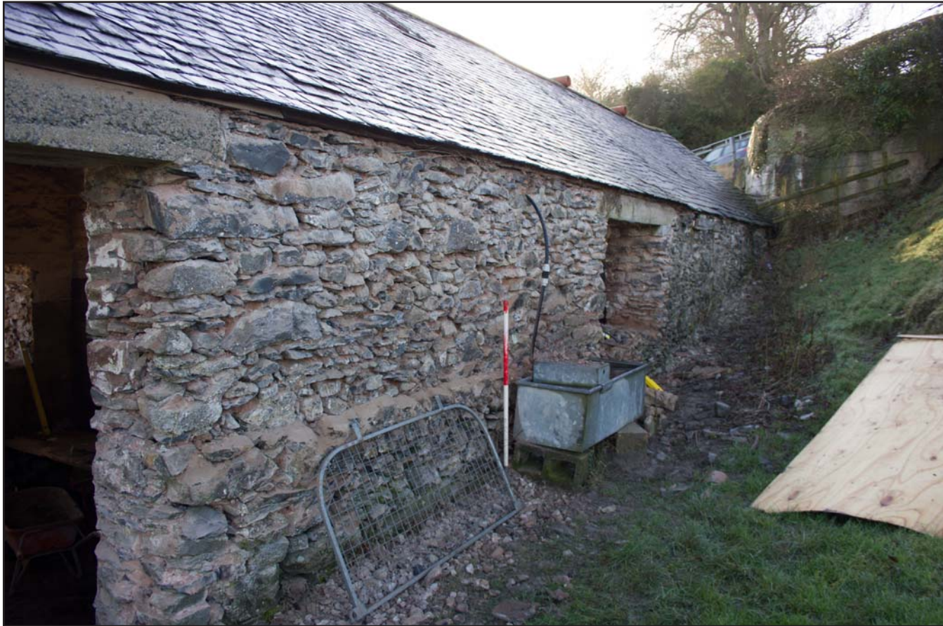
Plate 09: West facing external elevation (south), from the northwest. Scale 1.0m.
