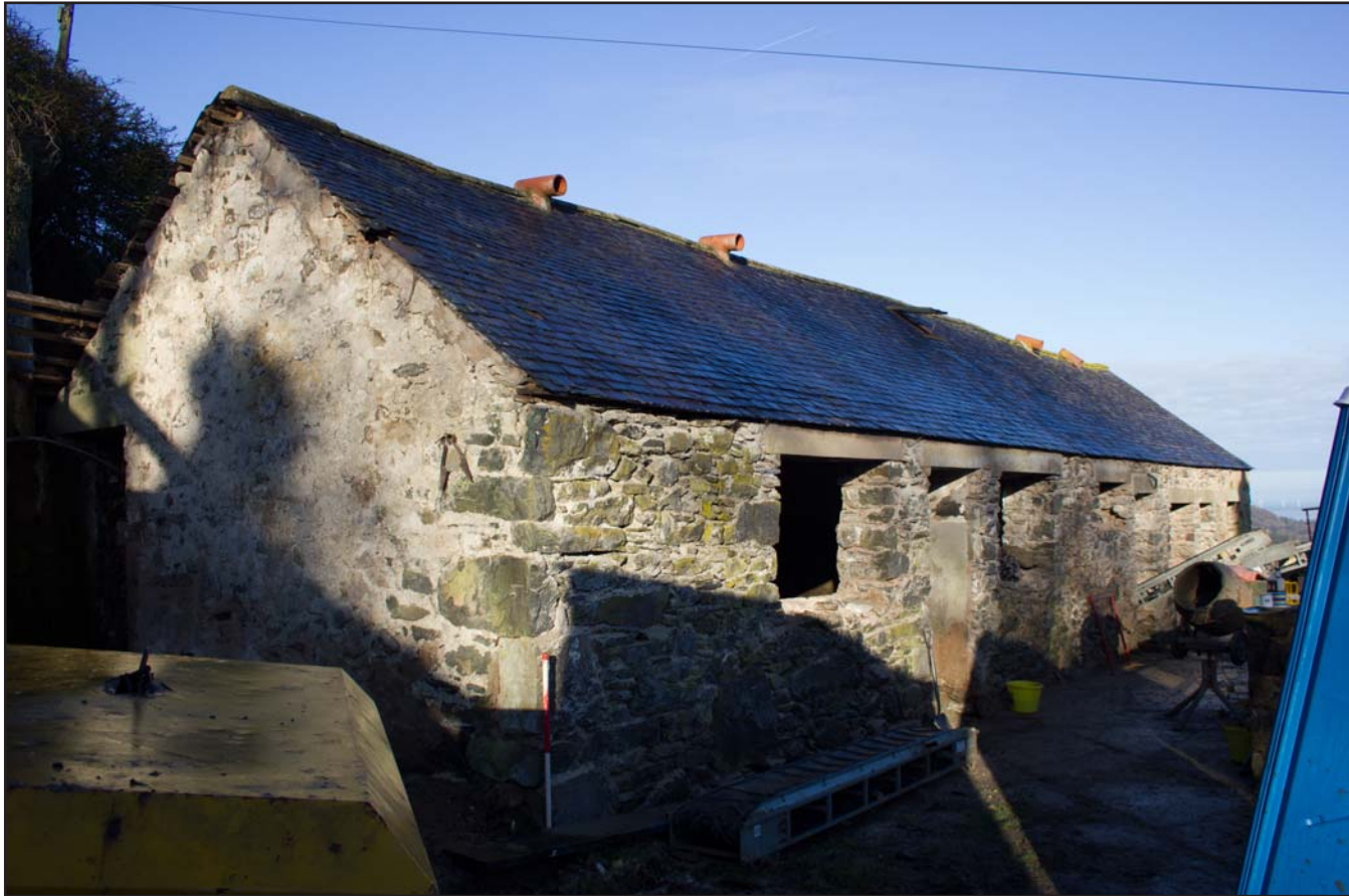
Plate 02: South and east facing external elevations, from the southeast. Scale 1.0m.
