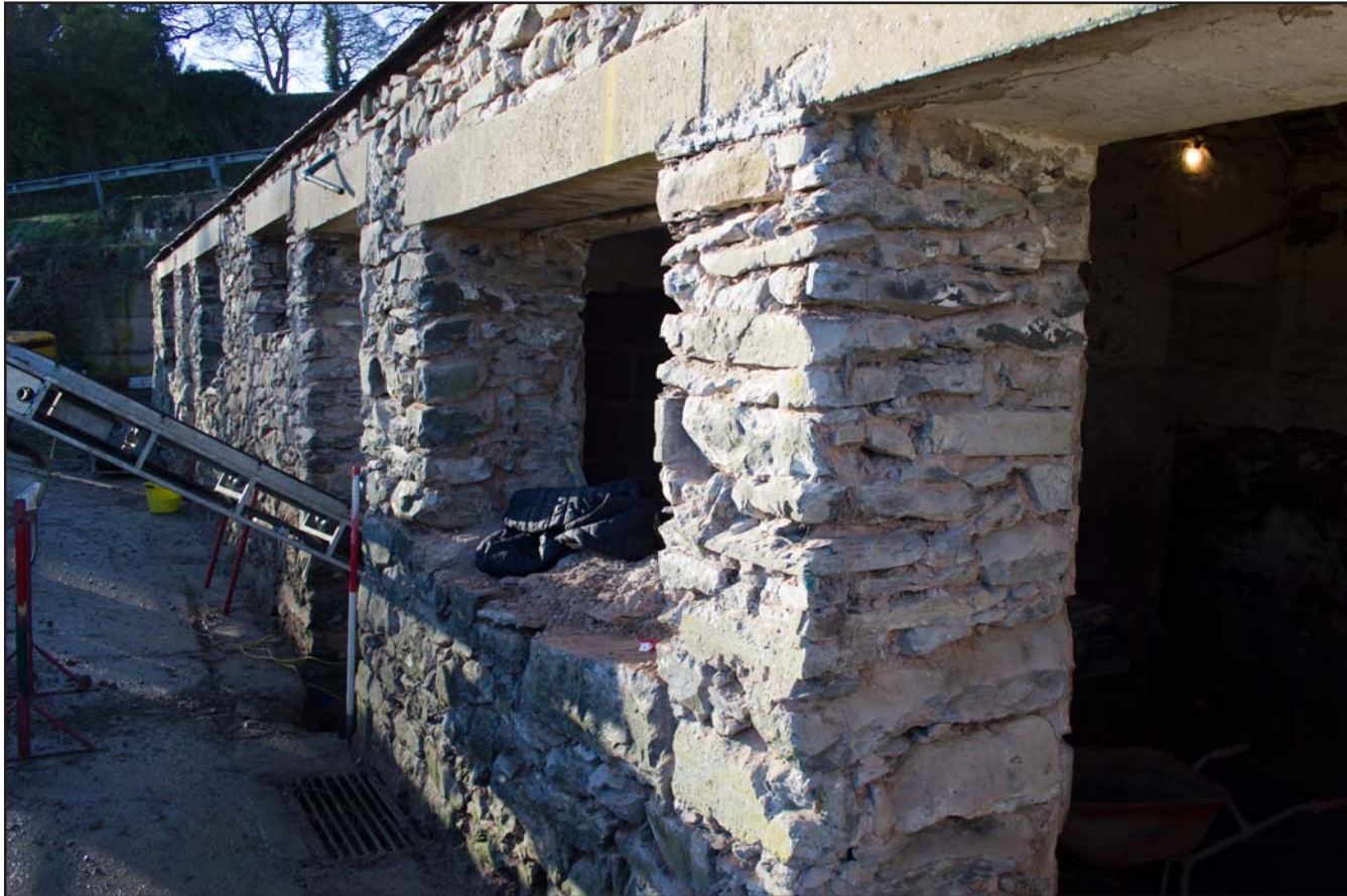
Plate 04: East facing external elevation, from the northeast. Scale 1.0m.
