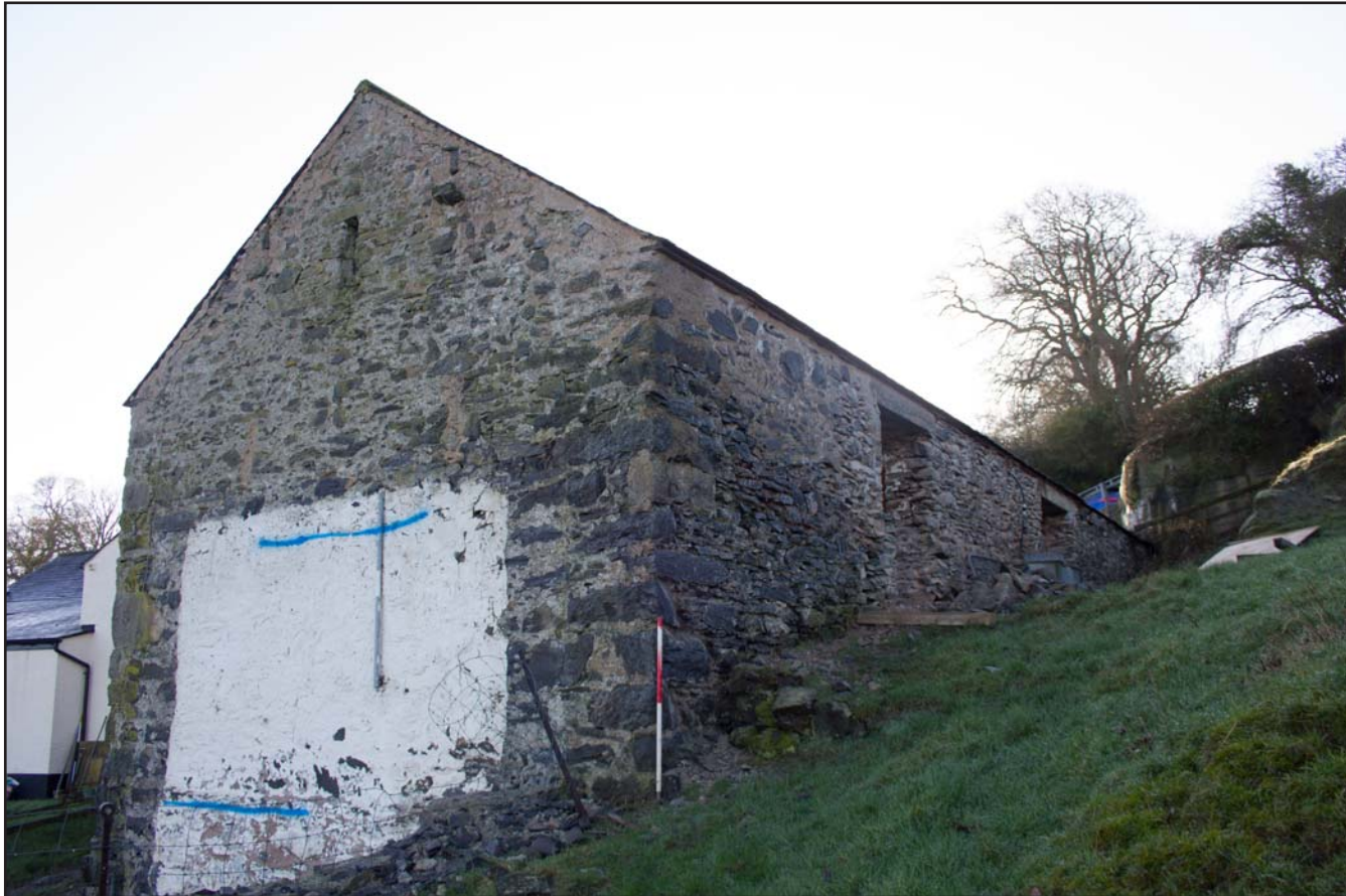
Plate 07: North and west facing external elevations, from the northwest. Scale 1.0m.
