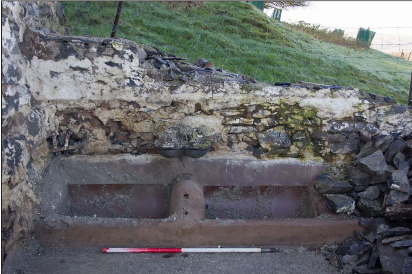
Plate 11: Demolished lean-to store showing troughs, from the east. Scale 1.0m.
