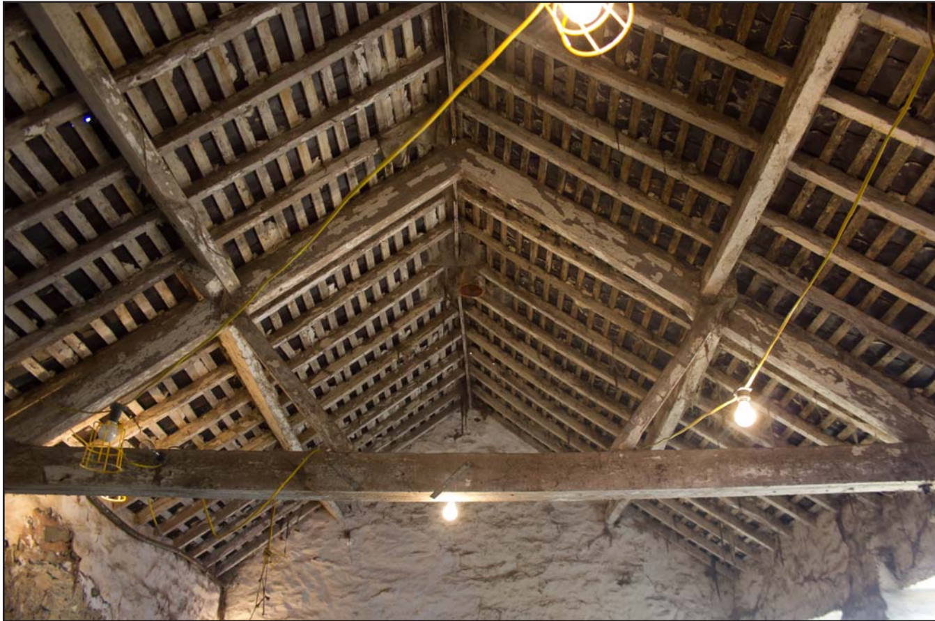
Plate 19: Room 3 showing truss, from the south.
