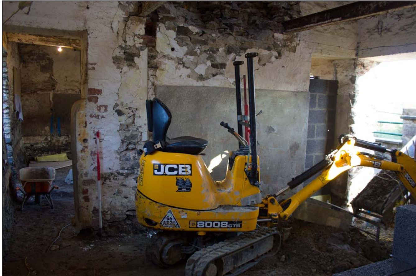
Plate 16: Room 2, from the southeast. Scale 1.0m.
