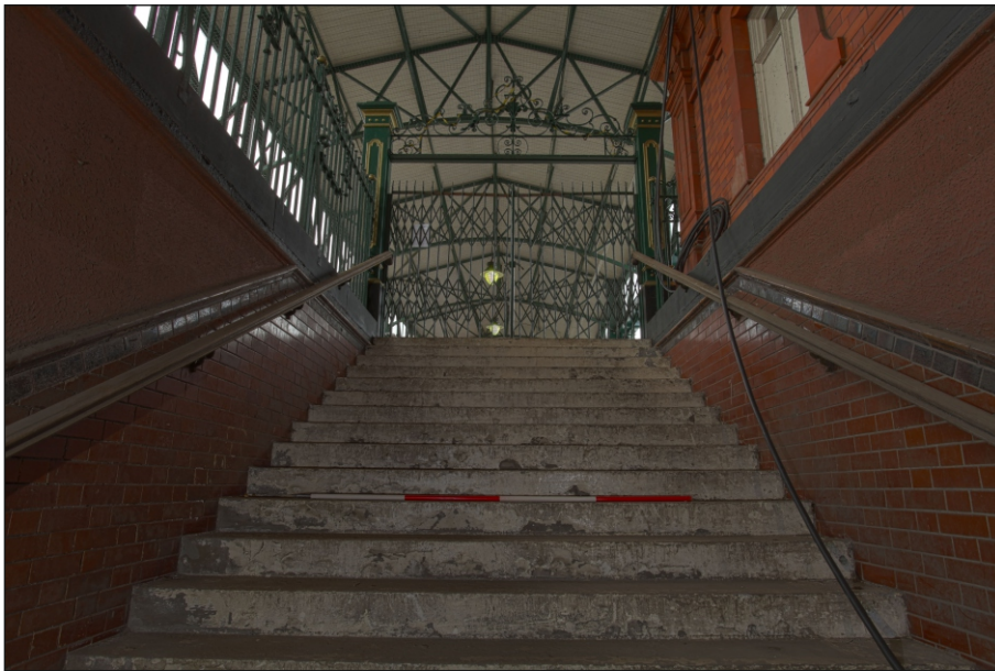
Plate 8: View of the staircase and gate to platform, looking northwest
