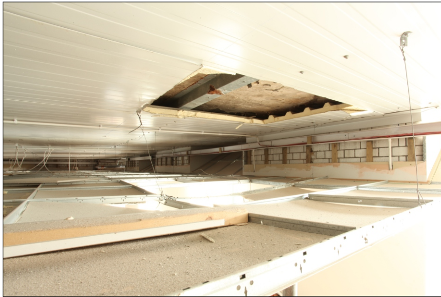
Plate 11: View above the suspended ceiling in room serving bays 5-9
