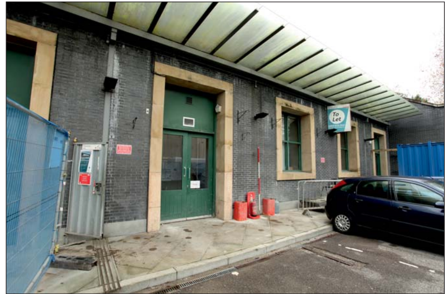
Plate 6: Oblique view of a typical door and windows, looking west
