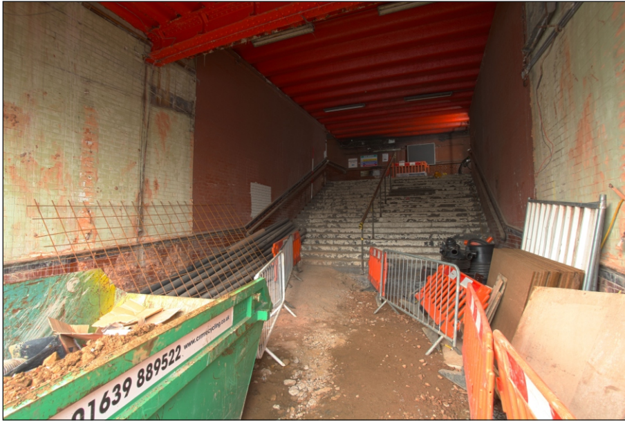
Plate 7: Detail of the original staircase leading to the platforms
