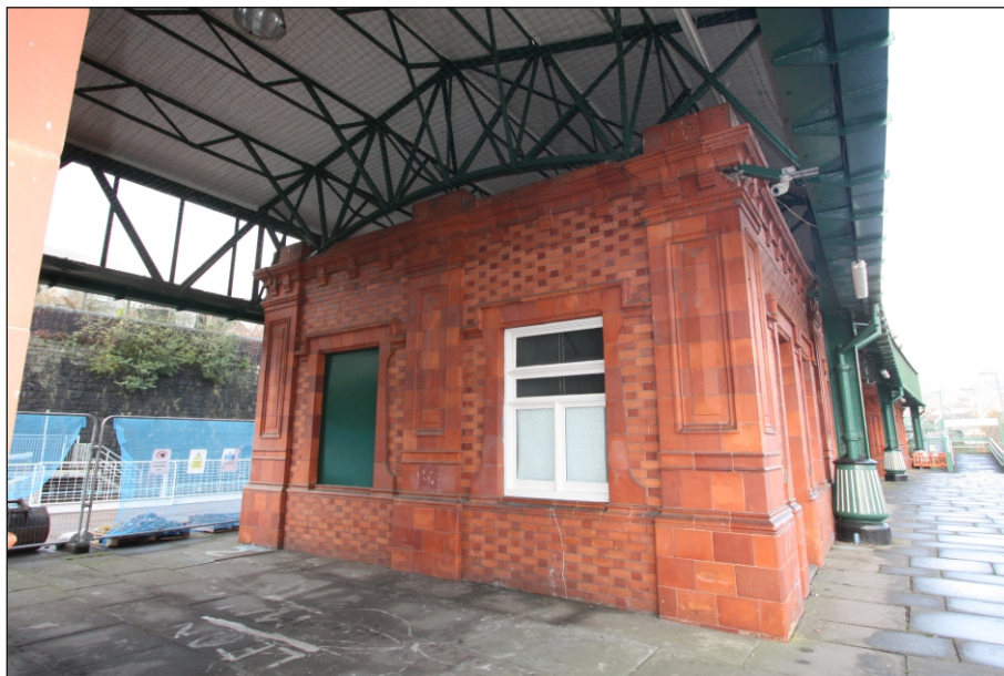
Figure 7: View of current station buildings on platform island, showing historic form
