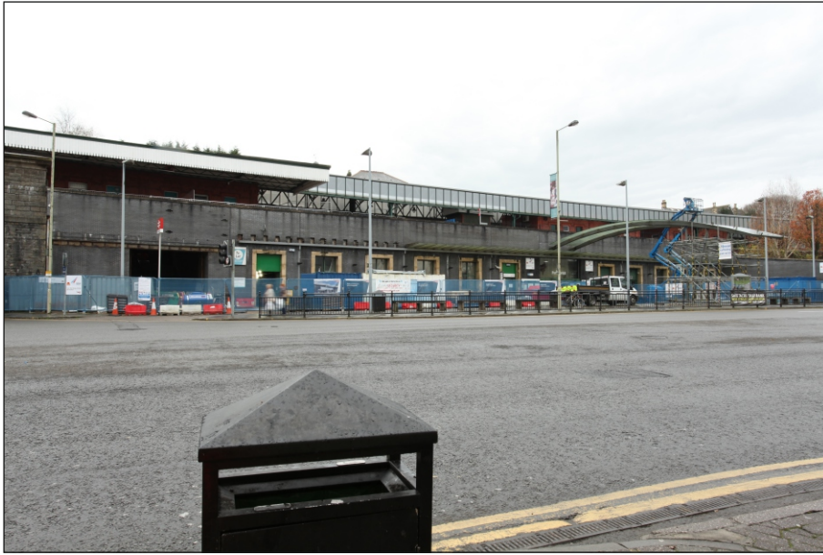
Plate 1: Oblique view of the principal (northeast) façade, looking west
