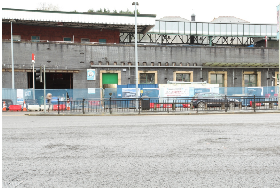
Plate 12: View of inserted openings within the principal facade, looking southwest
