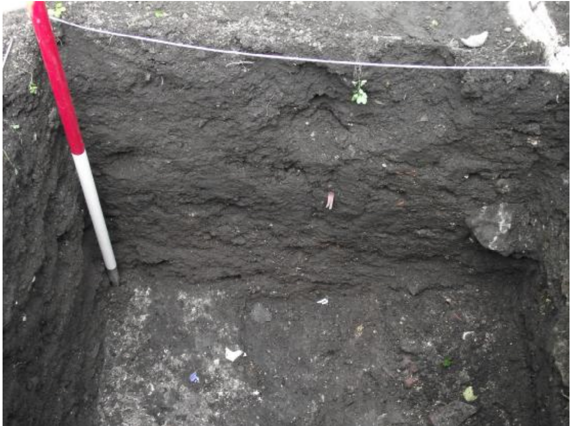
Plate 6. Limit of excavation and south-west facing section. The mortar patch (007) may be seen to the left of the image. The pan tile and mortar feature (006) is to the right of the image. Red plastic binding strip may be seen projecting from the section. Two leaves appear in this image (to the right of the base of the pit).
