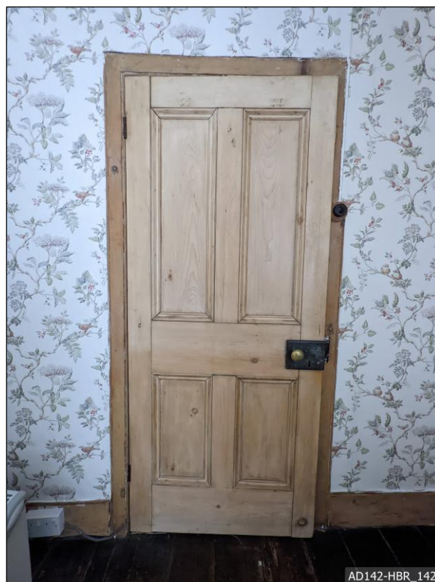
Plate 142 – View east, showing doorway to rear landing.
