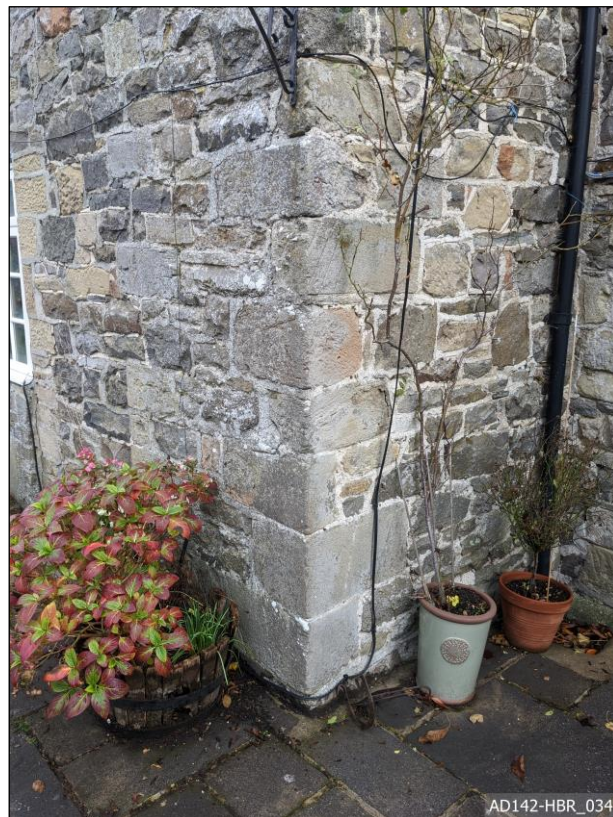
Plate 34 – View north-east, showing reused masonry as quoins.
