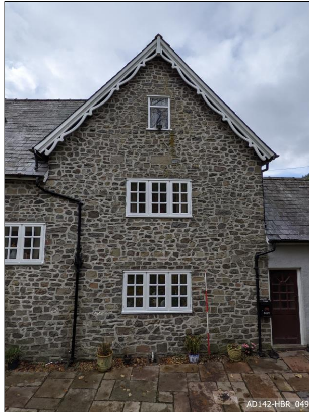
Plate 49 – View west, showing east elevation of wing.
