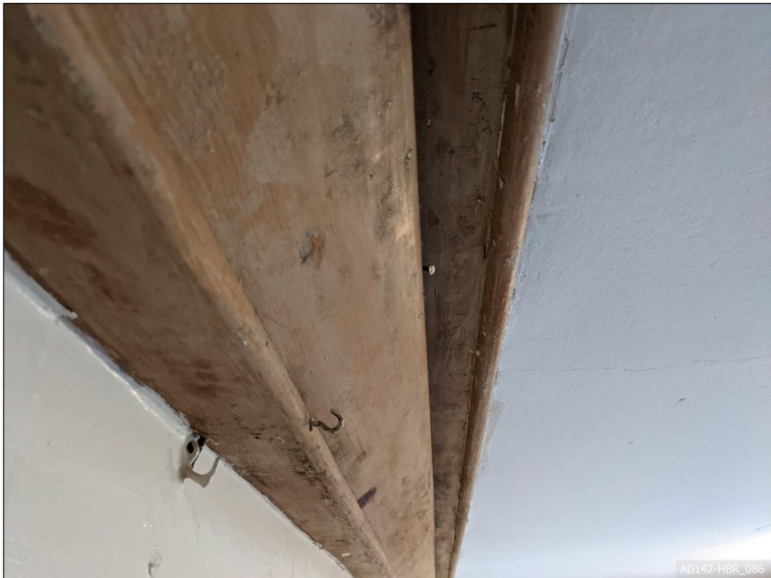
Plate 86 – View east, showing cornice in parlour.
