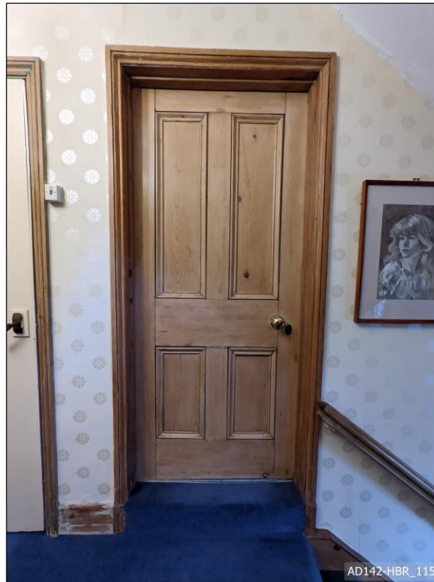
Plate 115 – View north, showing doorway to rear wing bedroom.
