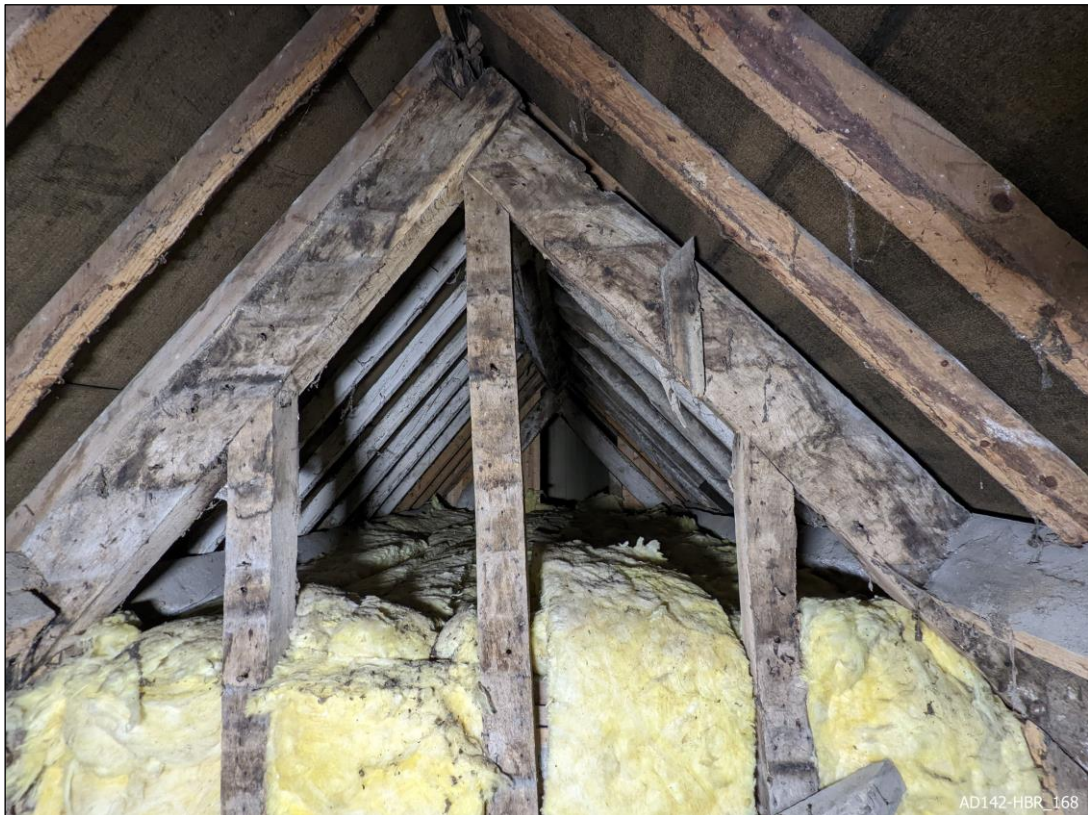
Plate 168 – View south, showing upper half of Truss 4.
