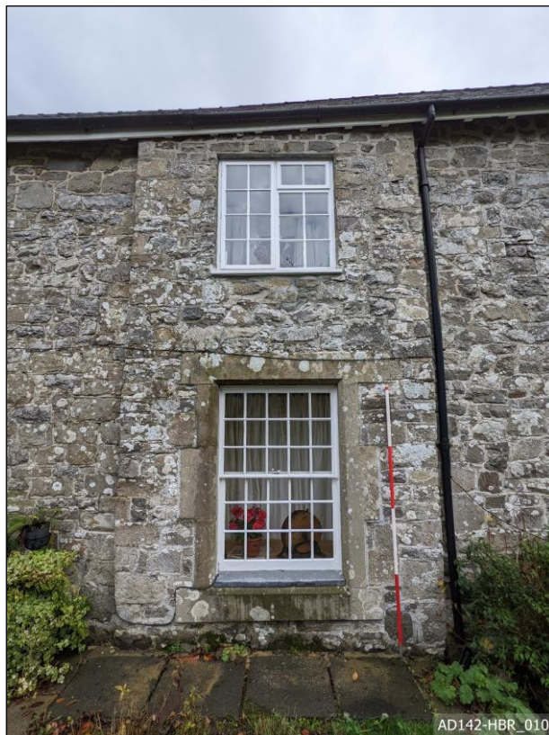
Plate 10 – View east, showing projected window panel.
