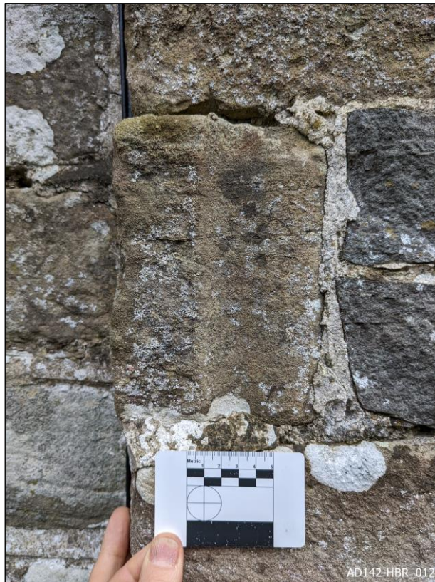
Plate 12 – View east, showing reused moulded masonry from abbey ruins.
