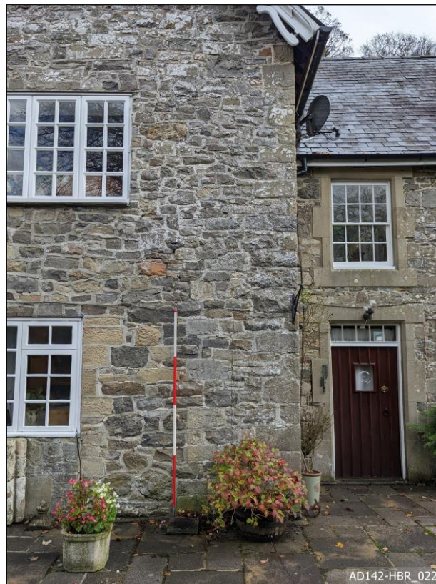
Plate 22 – View east, showing keying in of masonry.
