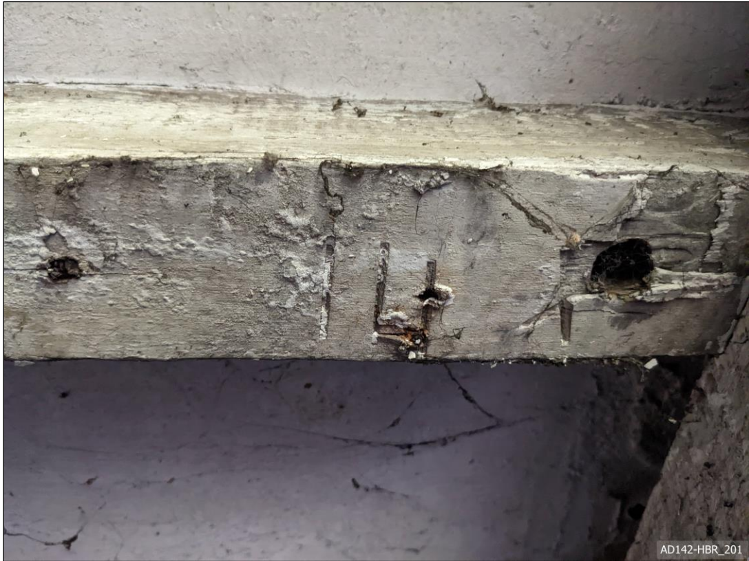
Plate 201 – View north, showing chisel cut assembly marks in Cell D.
