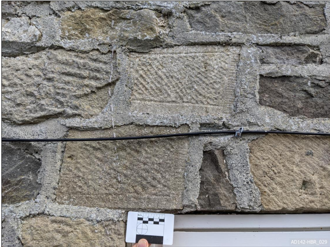
Plate 29 – View east, showing reused sandstone voussoir.
