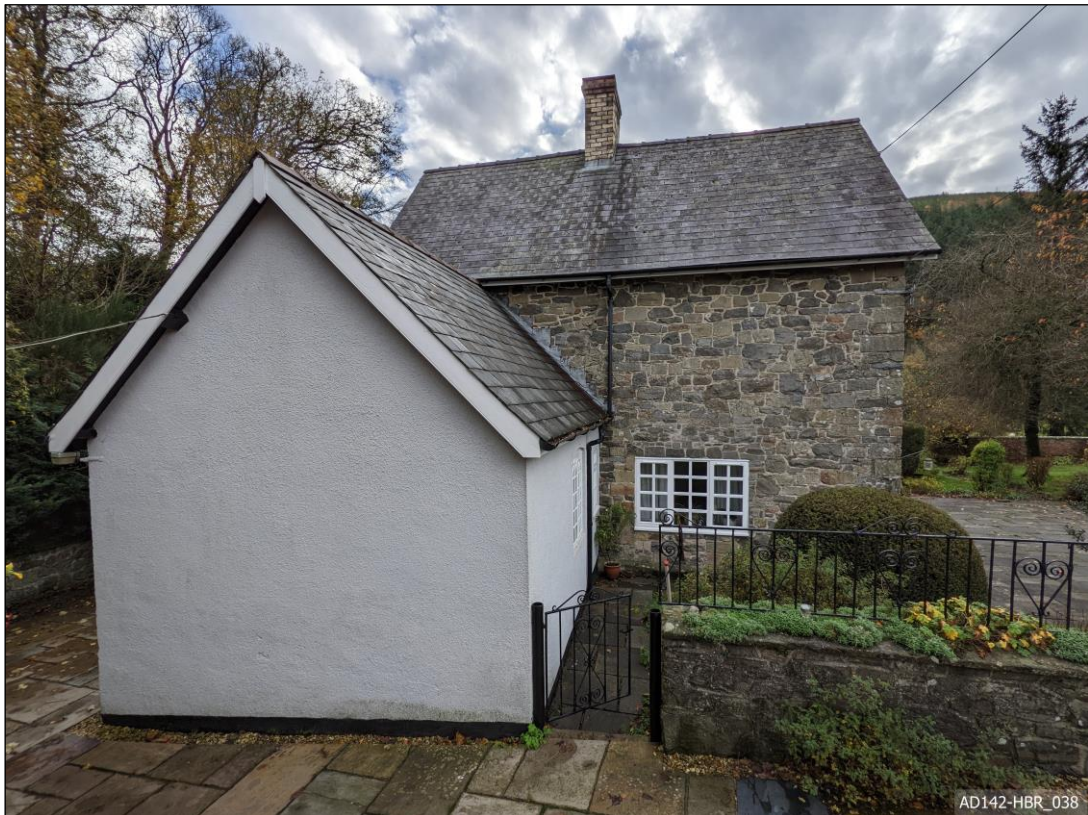
Plate 38 – View south, showing north elevation.
