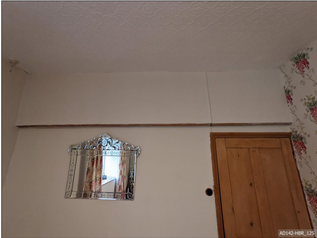
Plate 125 – View south, showing boxing to south of rear wing bedroom.
