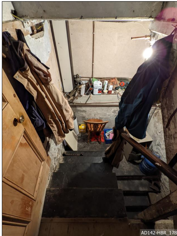
Plate 178 – View east, showing stairs to cellar.
