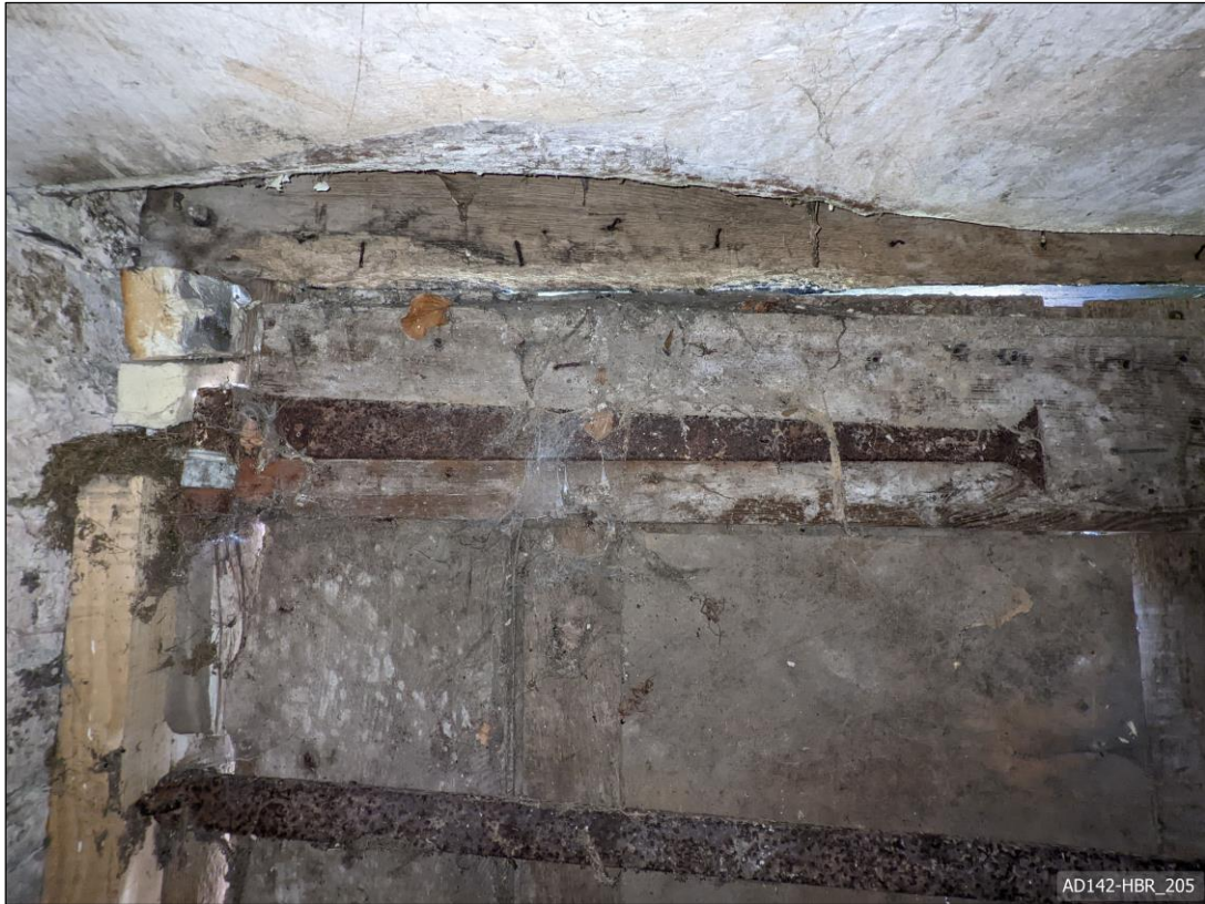
Plate 205 – View south, showing door hinge.
