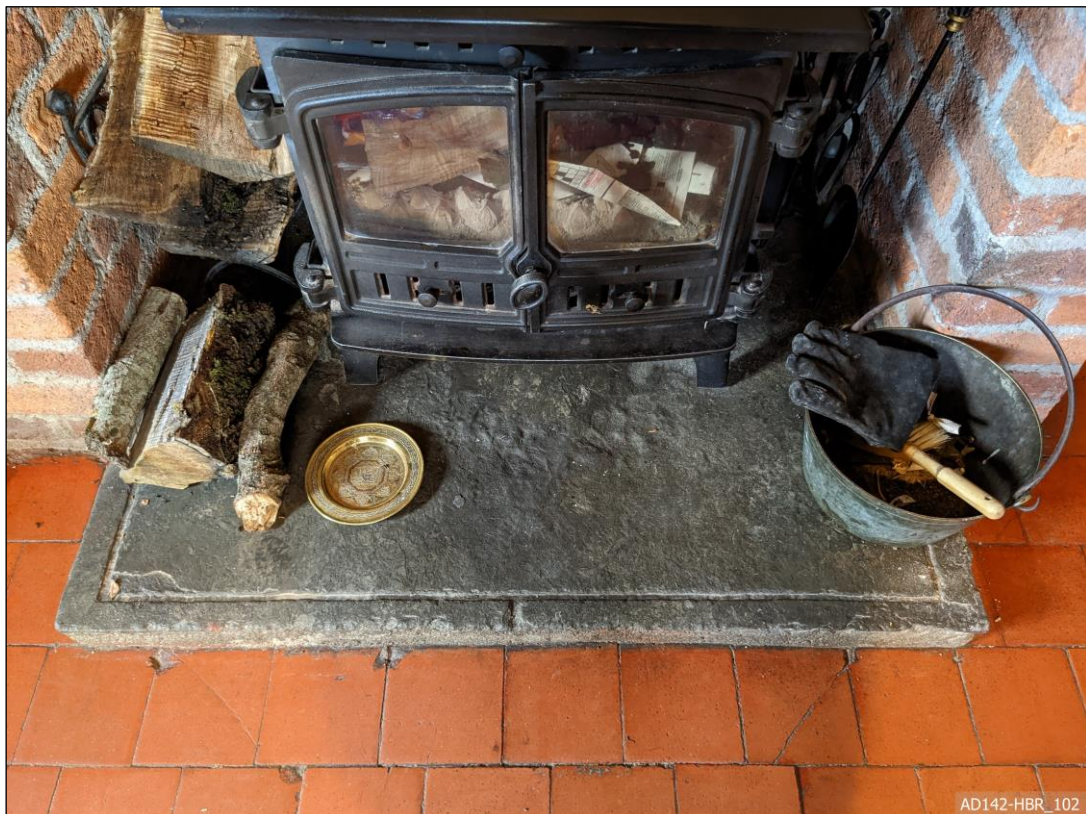
Plate 102 – View east, showing salting stone (imported) reused as hearth stone.
