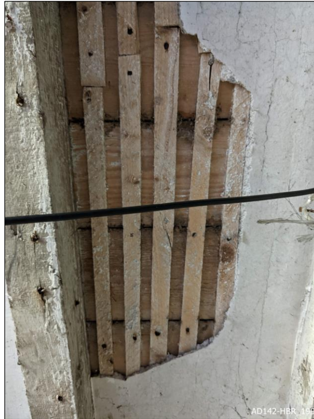
Plate 199 – View west, showing lathe-and-plaster ceiling of Cell D.
