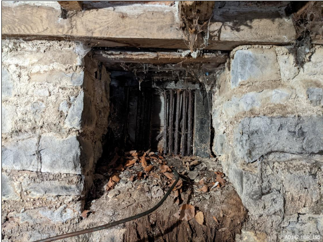
Plate 195 – View east, showing blocked ventilation window.
