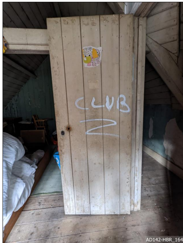
Plate 164 – View north, showing door to store room.
