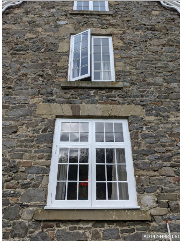
Plate 61 – View north, showing windows.
