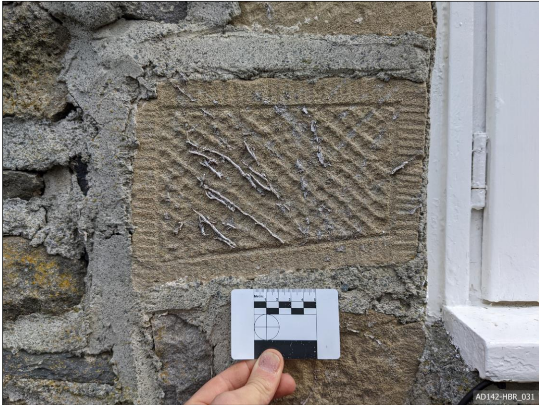
Plate 31 – View east, showing re-used sandstone voussoir.
