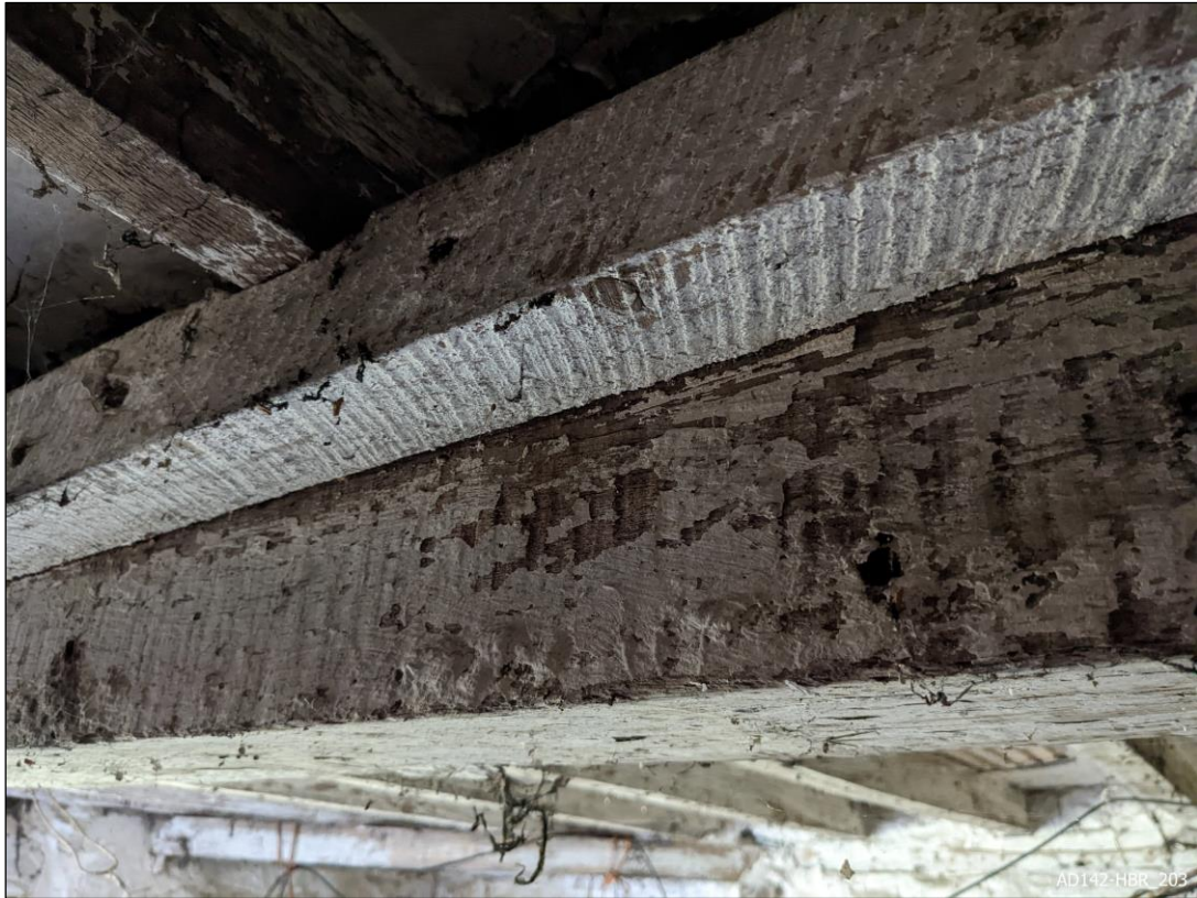
Plate 203 – View west, showing pit and circular sawn timbers in Cell D.
