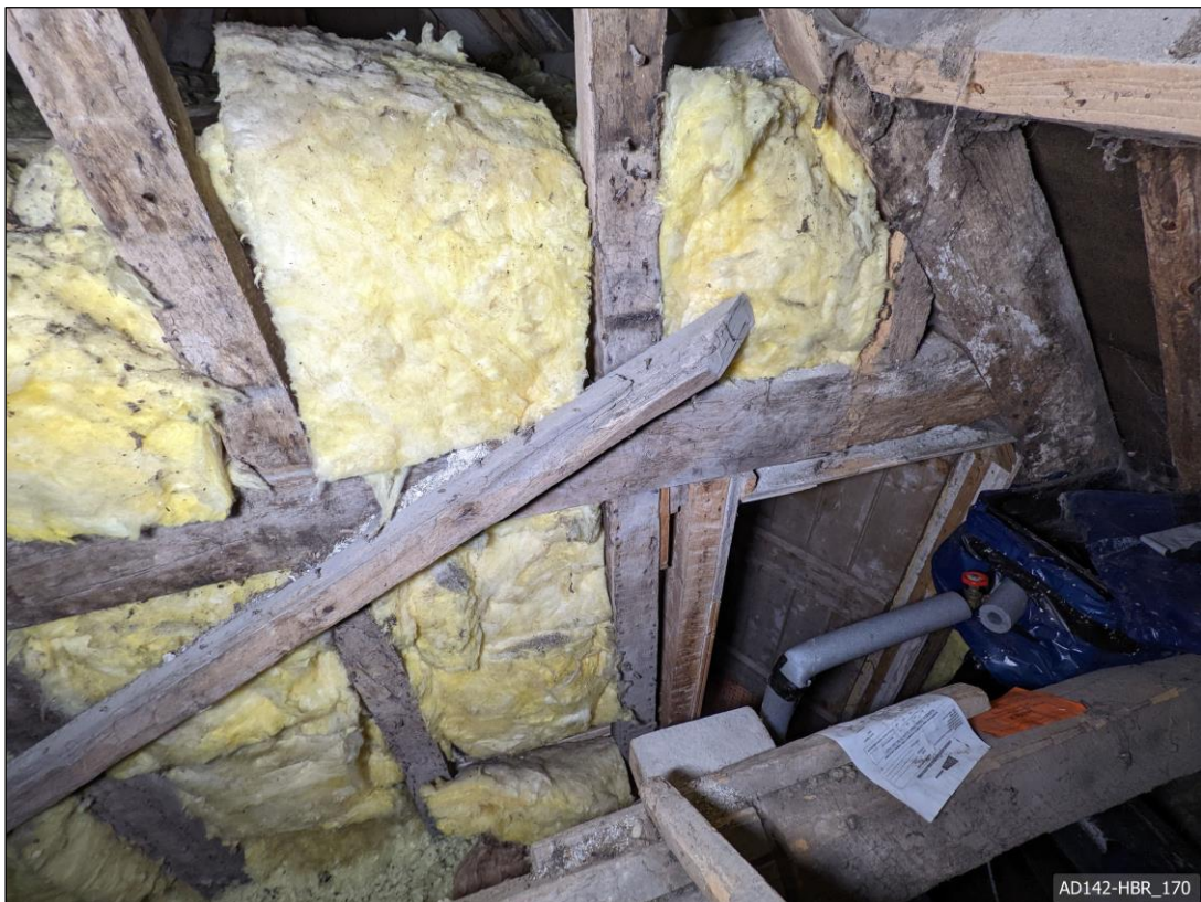
Plate 170 – View west, showing lower half of Truss 4.
