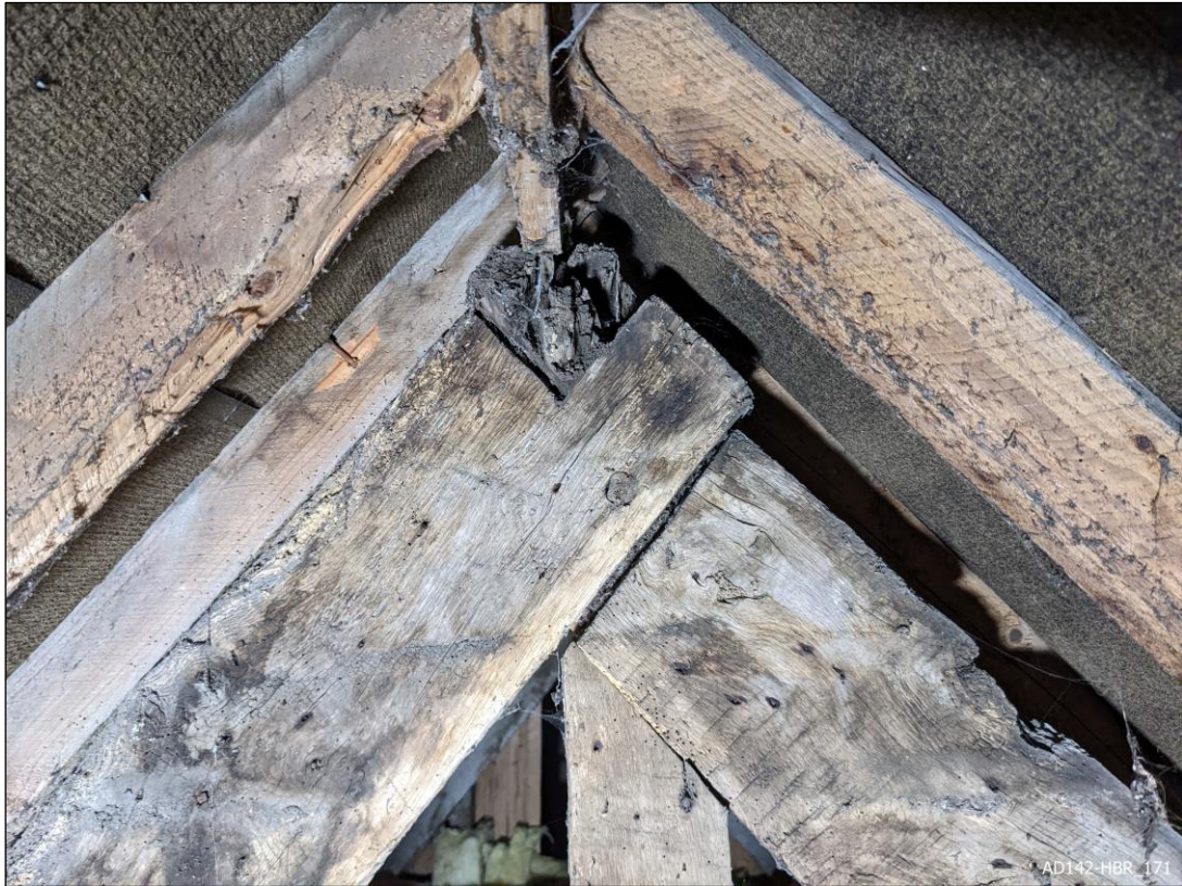
Plate 171 – View south, showing apex of Truss 4.
