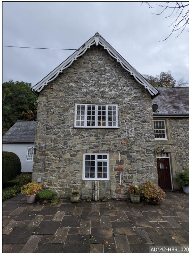
Plate 20 – View east, showing west elevation of wing.
