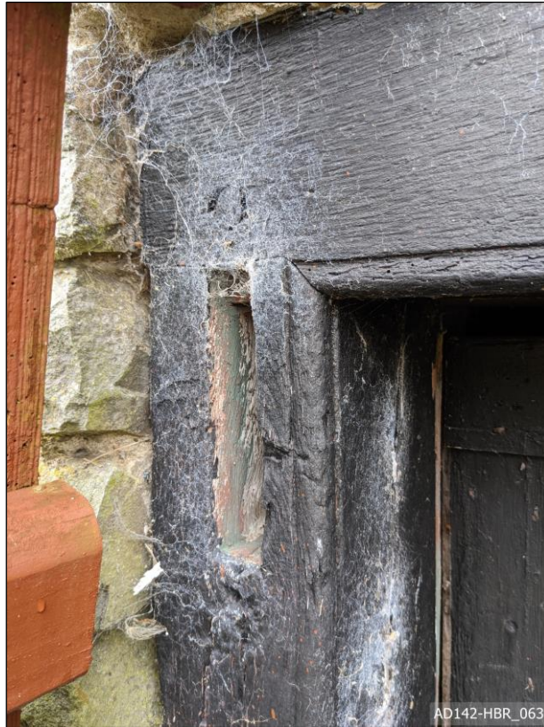
Plate 63 – View north, showing mortise to door frame.
