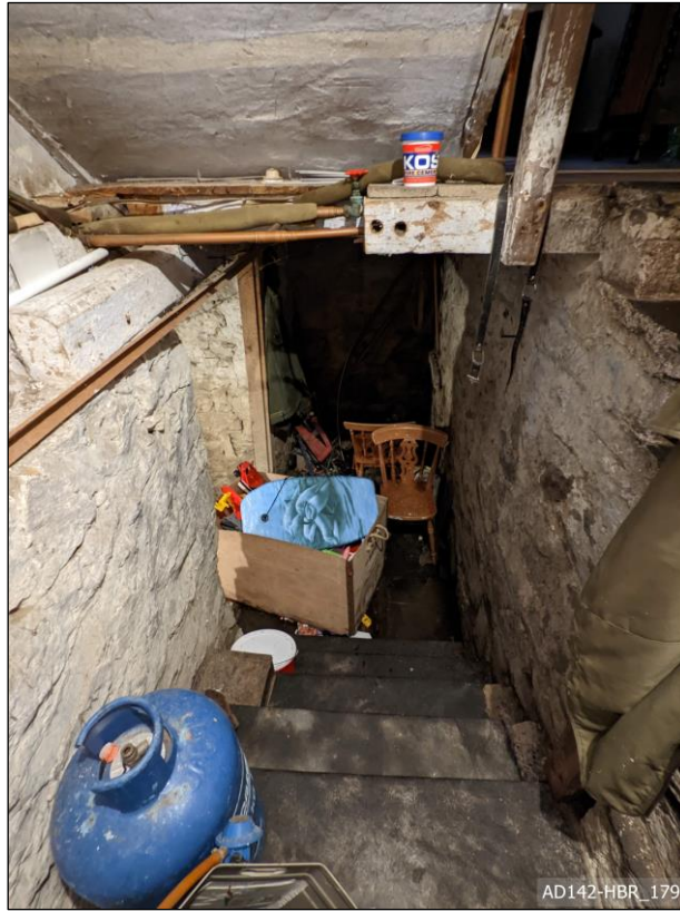
Plate 179 – View west, showing stairs to cellar.
