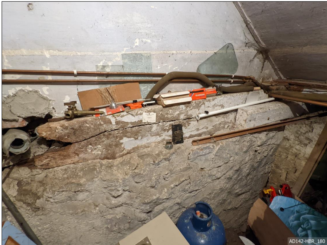
Plate 180 – View south, showing remains of Phase I transverse beam.
