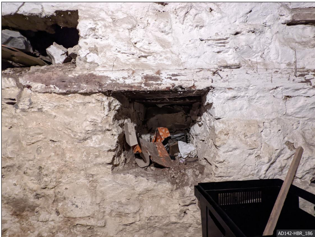
Plate 186 – View south, showing ventilation window to Cell B.
