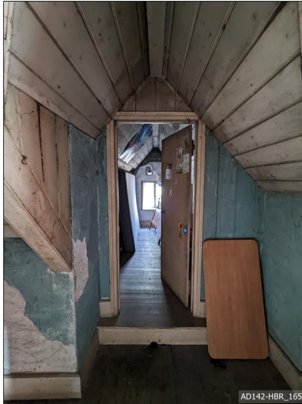
Plate 165 – View east, showing doorway to rear store room.
