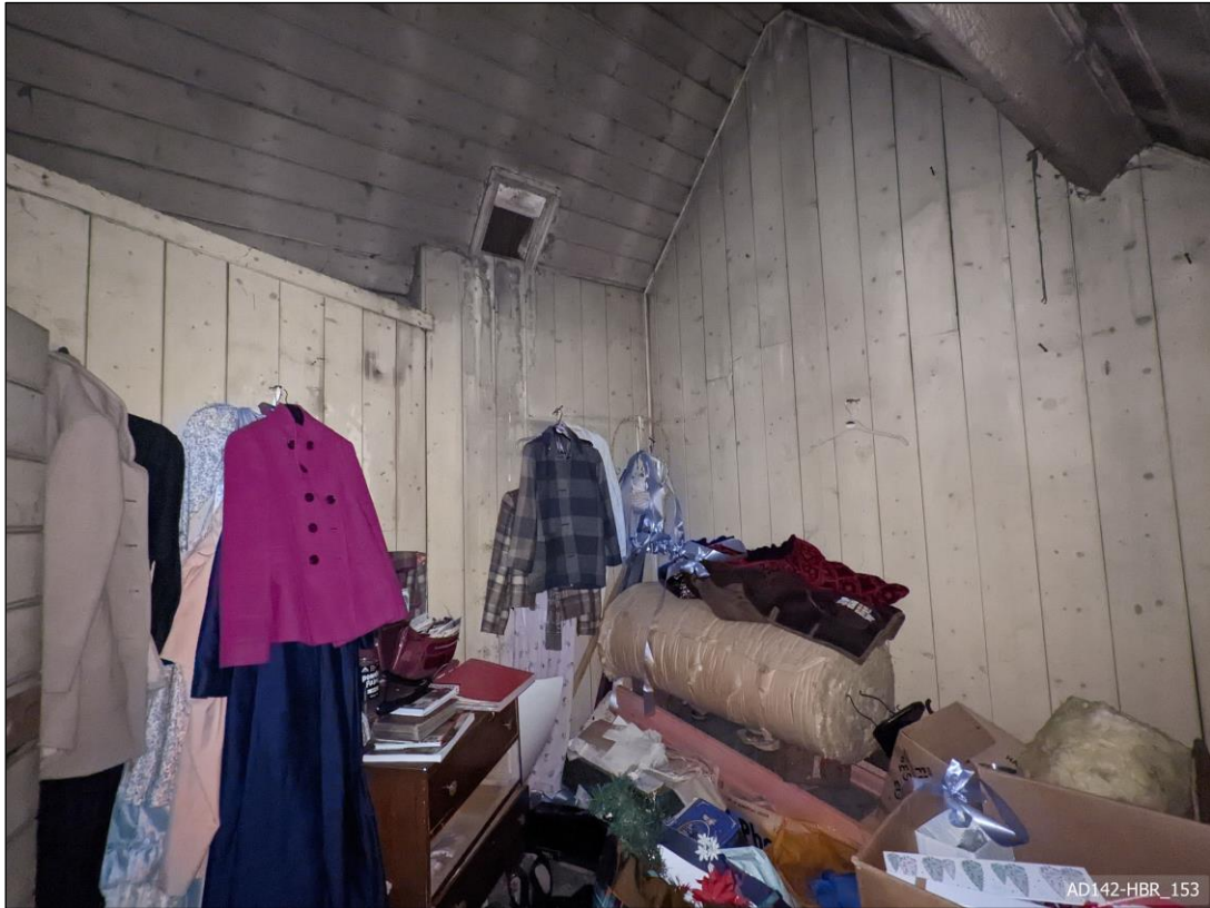
Plate 153 – View south-west, shoring store room.
