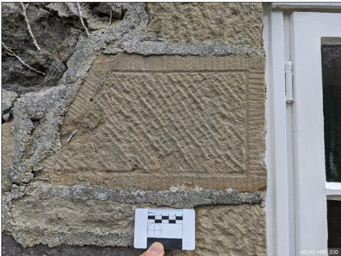
Plate 30 – View east, showing reused sandstone voussoir.
