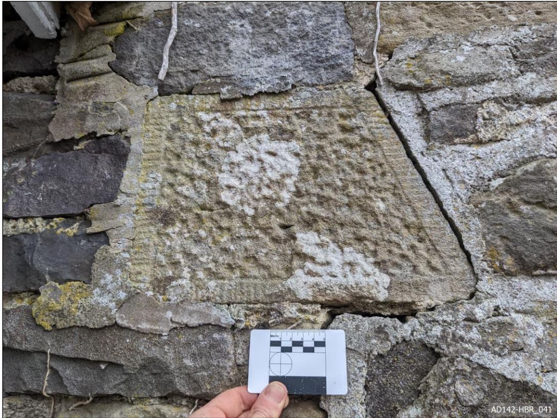
Plate 41 – View south, showing reused voussoir.
