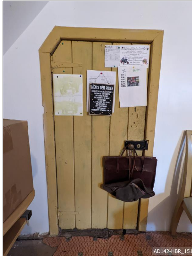
Plate 151 – View north, showing doorway to attic space.
