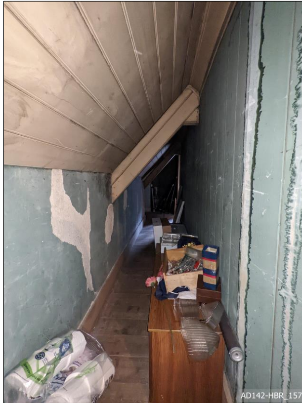
Plate 157 – View south, showing second floor corridor.
