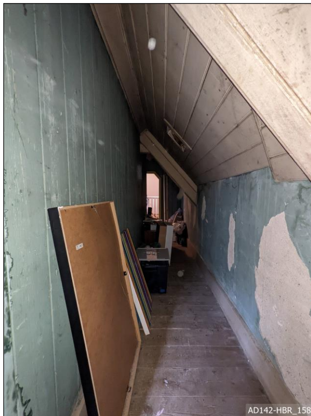
Plate 158 – View north, showing second floor corridor.
