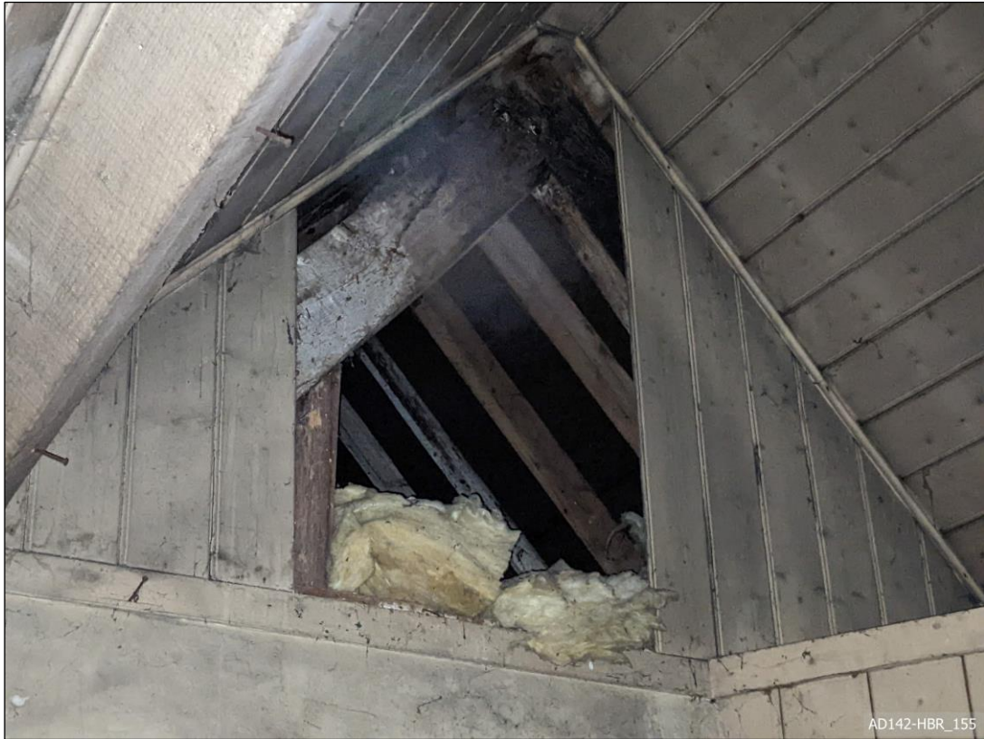
Plate 155 – View north-east, showing Truss 3.
