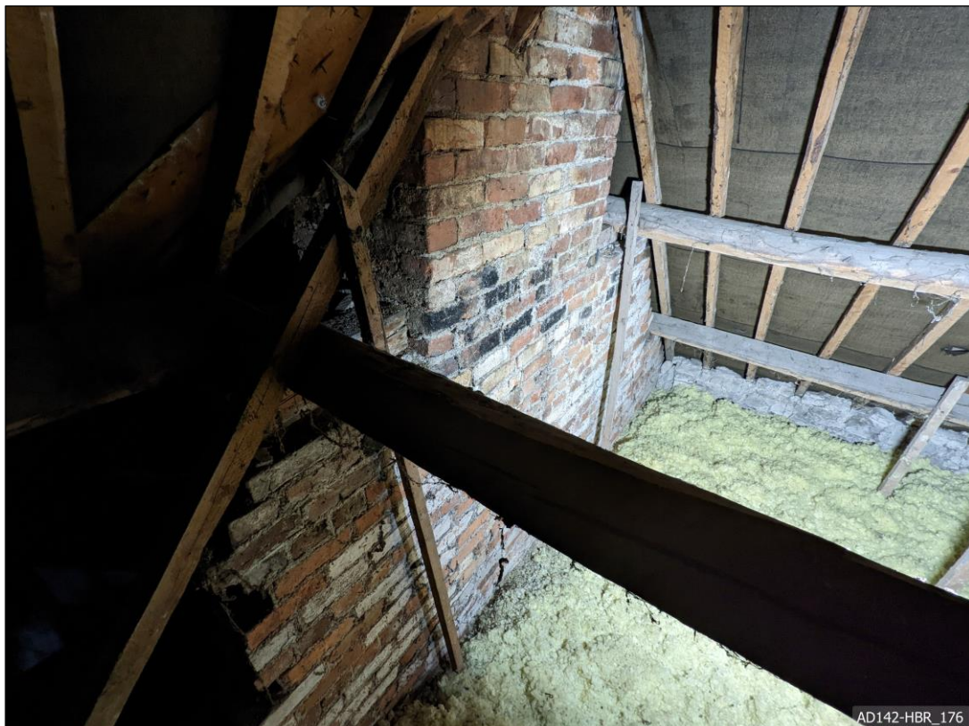
Plate 176 – View north-west, showing cross-wall and chimney of wing.
