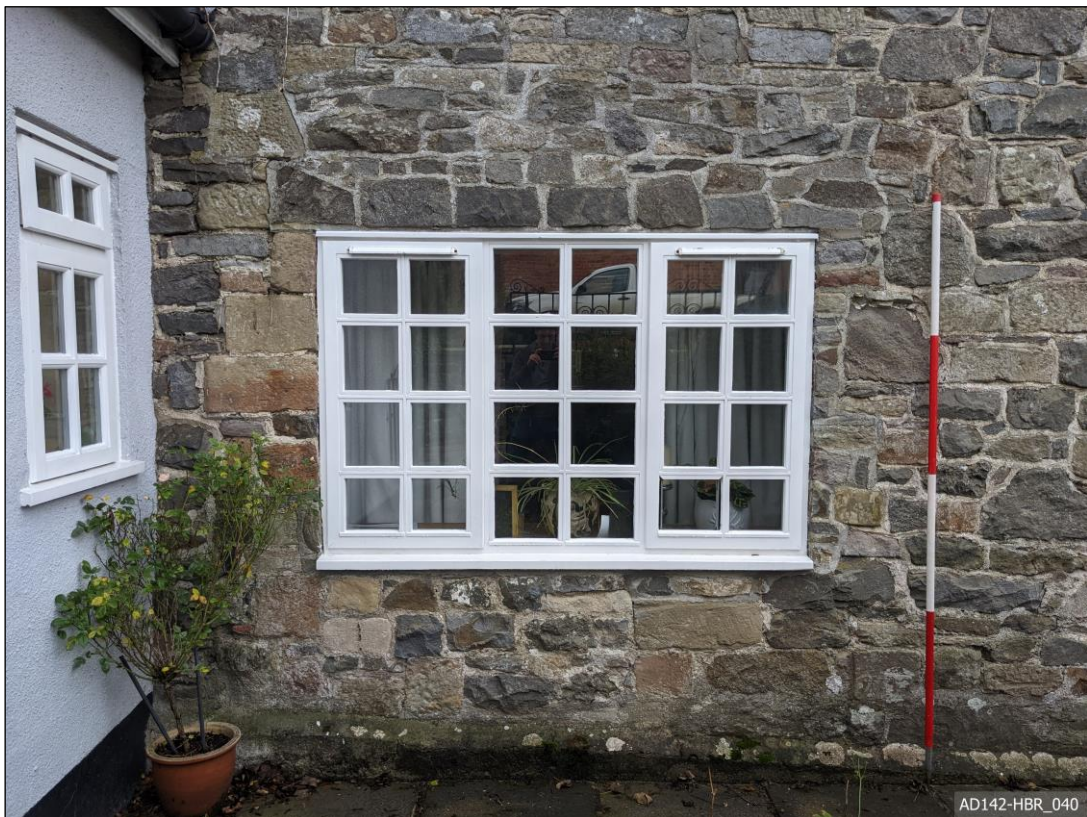
Plate 40 – View south, showing inserted window and earlier doorway jambs.
