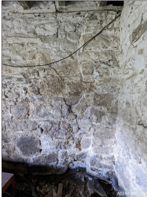
Plate 197 – View west, showing joint in masonry relating to south extension.
