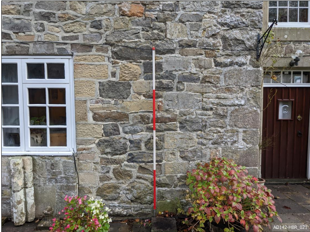
Plate 21 – View east, showing keying in of masonry.
