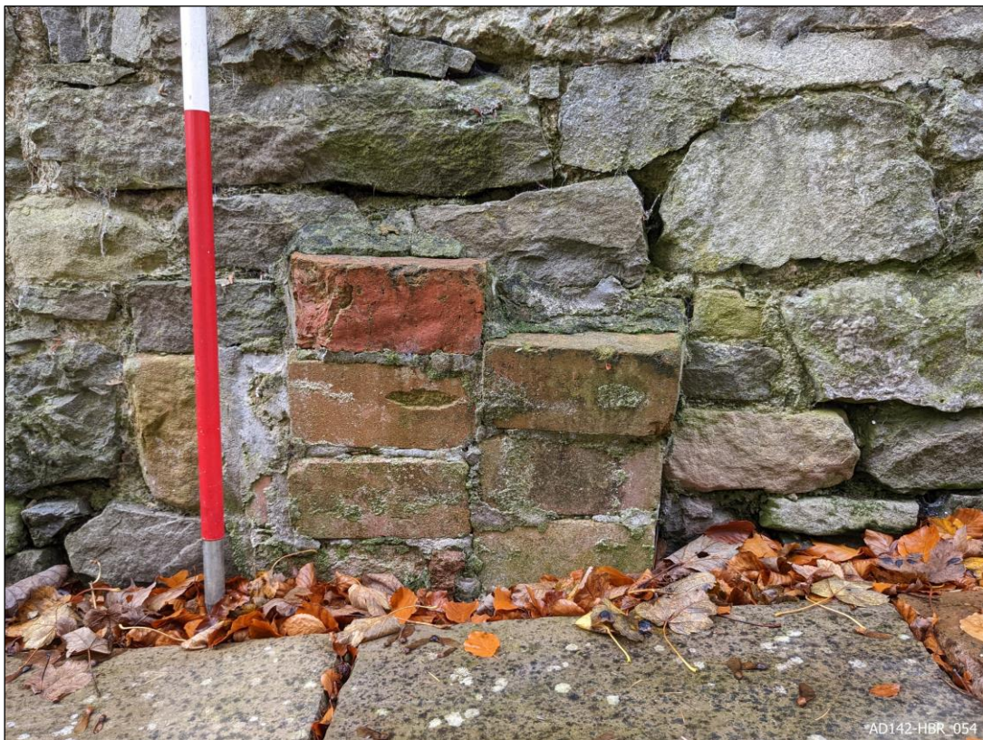
Plate 54 – View west, showing blocking of cellar ventilation window.
