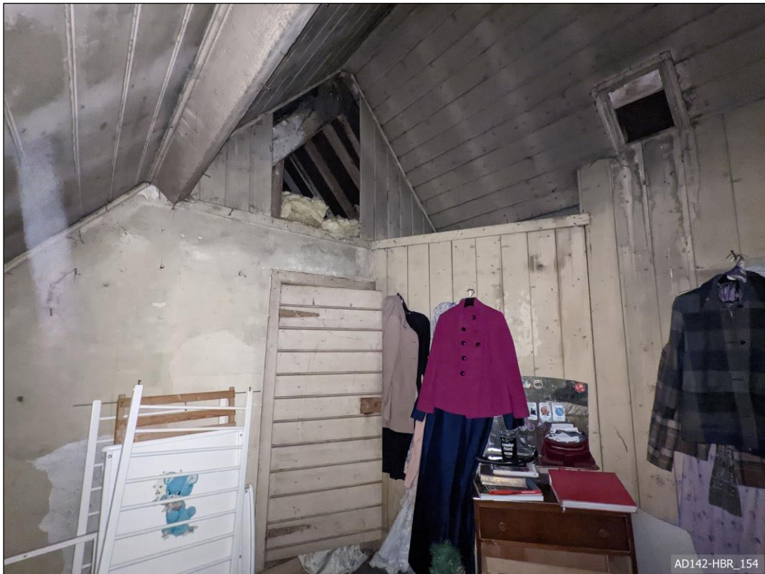
Plate 154 – View north-east, showing store room.
