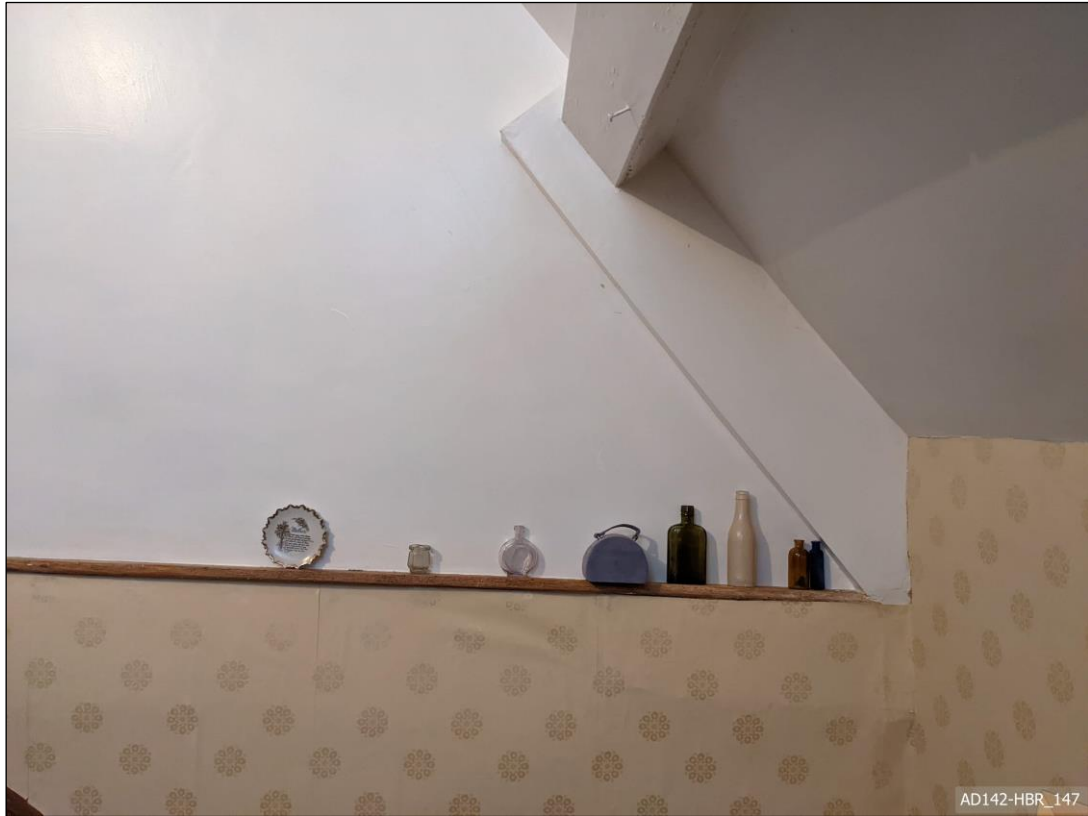
Plate 147 – View north, showing boxing of truss.
