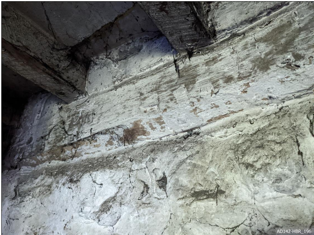
Plate 196 – View north, showing oak transverse beam between Cells B and C.
