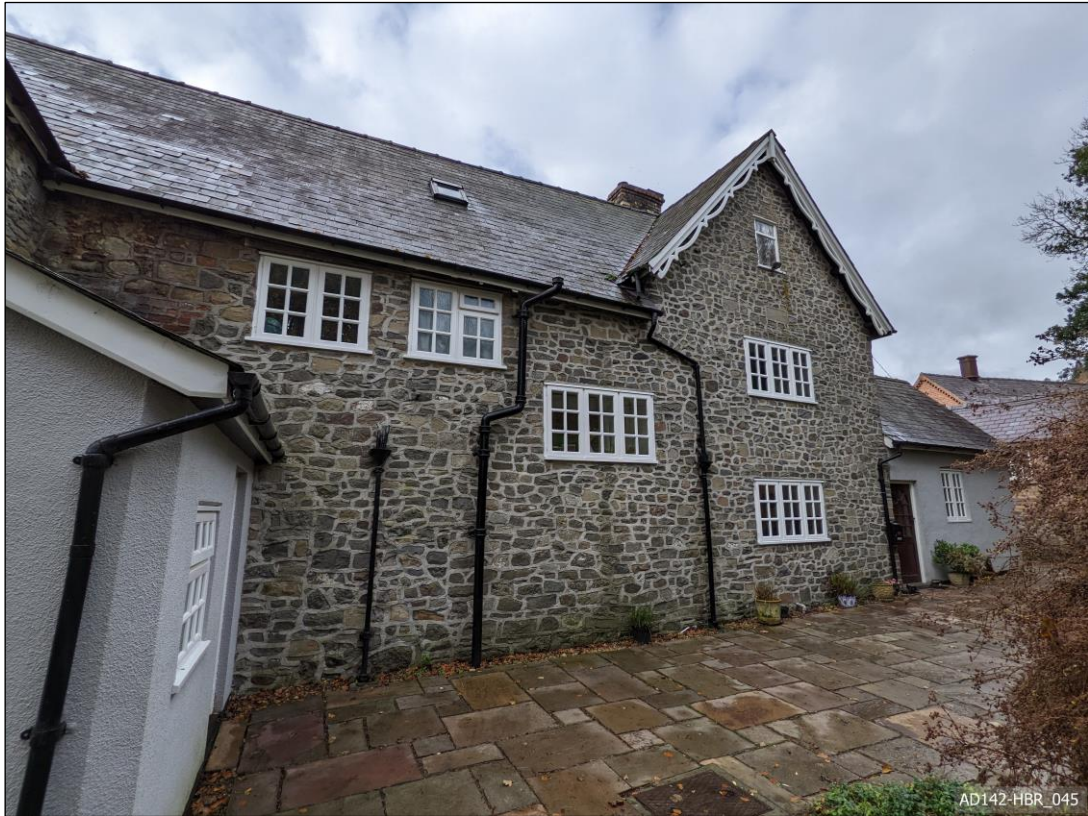
Plate 45 – View west, showing east elevation.
