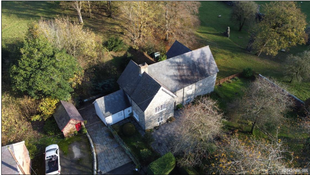
Plate 5 – View south-east, showing Home Farmhouse.
