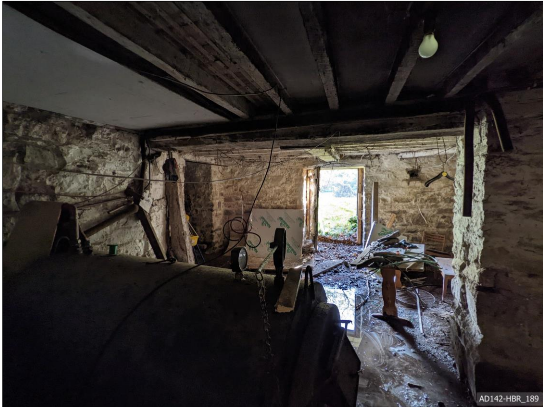
Plate 189 – View south-east, showing Cells C and D.
