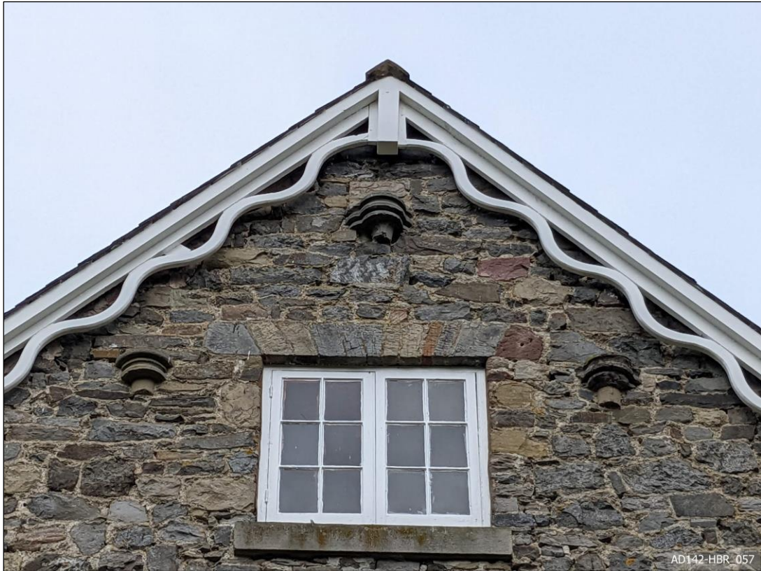
Plate 57 – View north, showing reused colonnette capitals.
