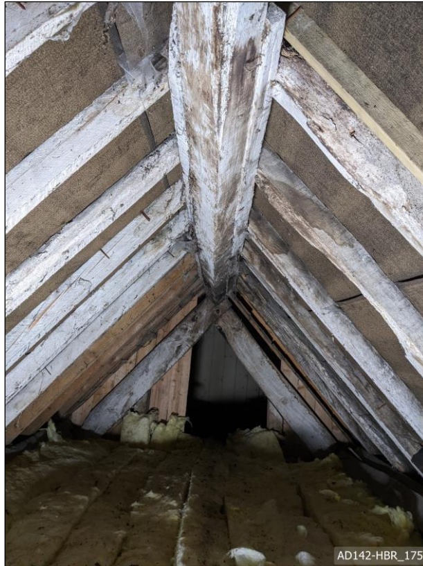
Plate 175 – View south, showing ridge and common rafters of Bay 4.
