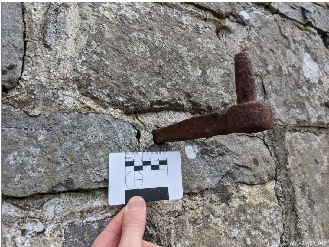
Plate 42 – View south, showing pintle for gate.
