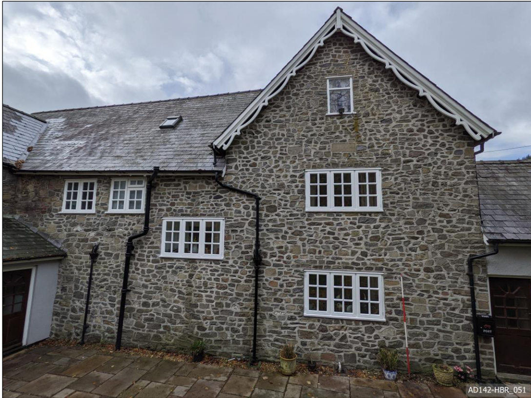
Plate 51 – View west, showing east elevation.
