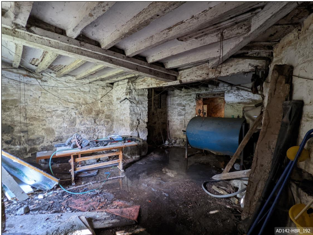
Plate 192 – View north-west, showing Cells C and D.
