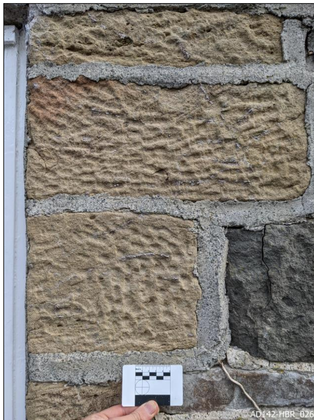
Plate 26 – View east, showing reused pecked sandstone blocks.
