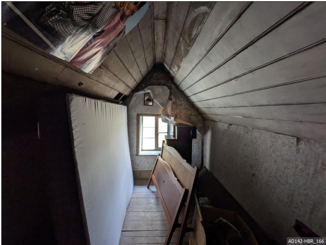
Plate 166 – View east, showing rear store room.
