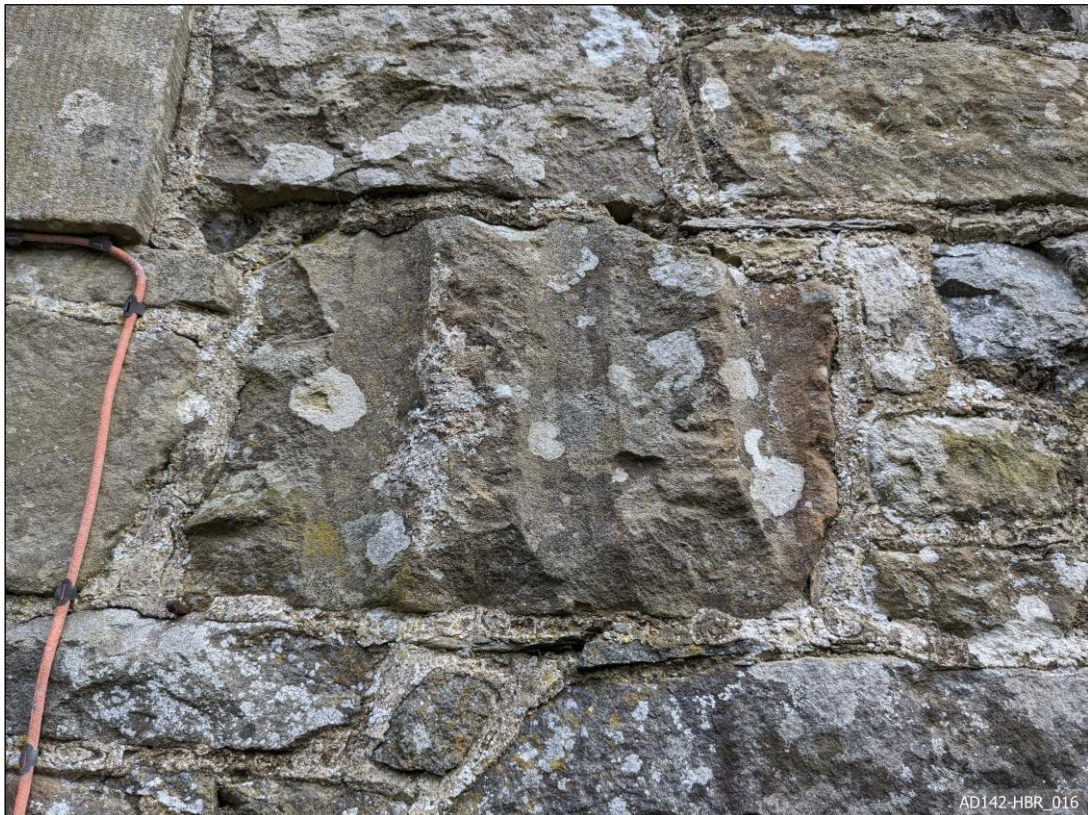
Plate 16 – View east, showing reused moulded masonry from abbey ruins.
