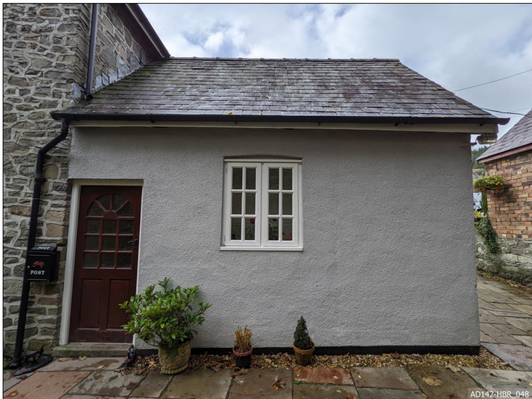
Plate 48 – View west, showing east elevation of north extension.
