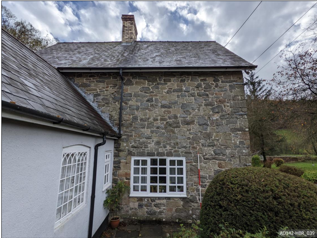
Plate 39 – View south, showing north elevation of wing.
