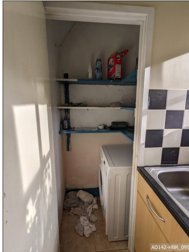
Plate 95 – View east, showing cupboard in utility room.
