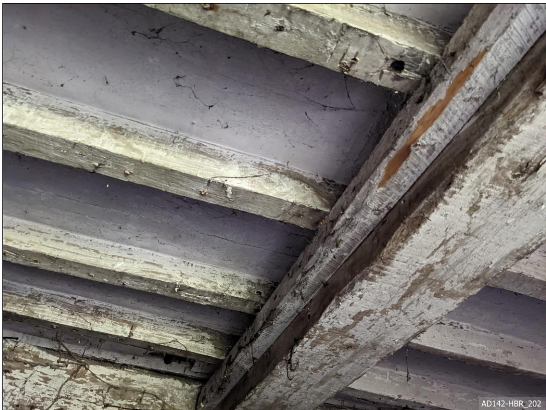
Plate 202 – View north, showing pit and circular sawn timbers in Cell D.
