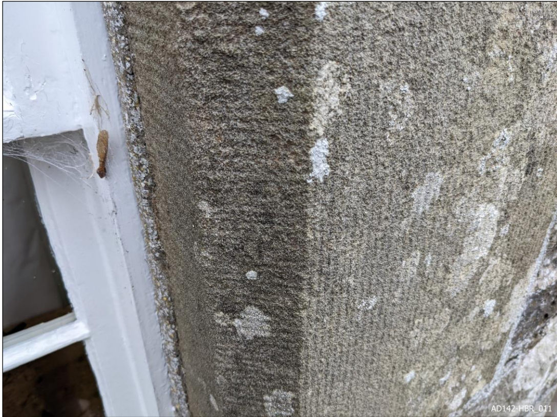
Plate 11 – View east, showing tooling of masonry window jamb.
