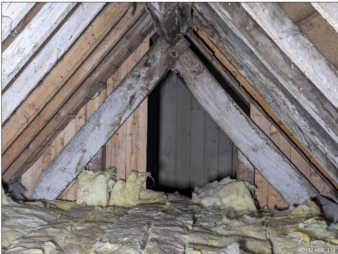
Plate 174 – View south, showing top of Truss 3.
