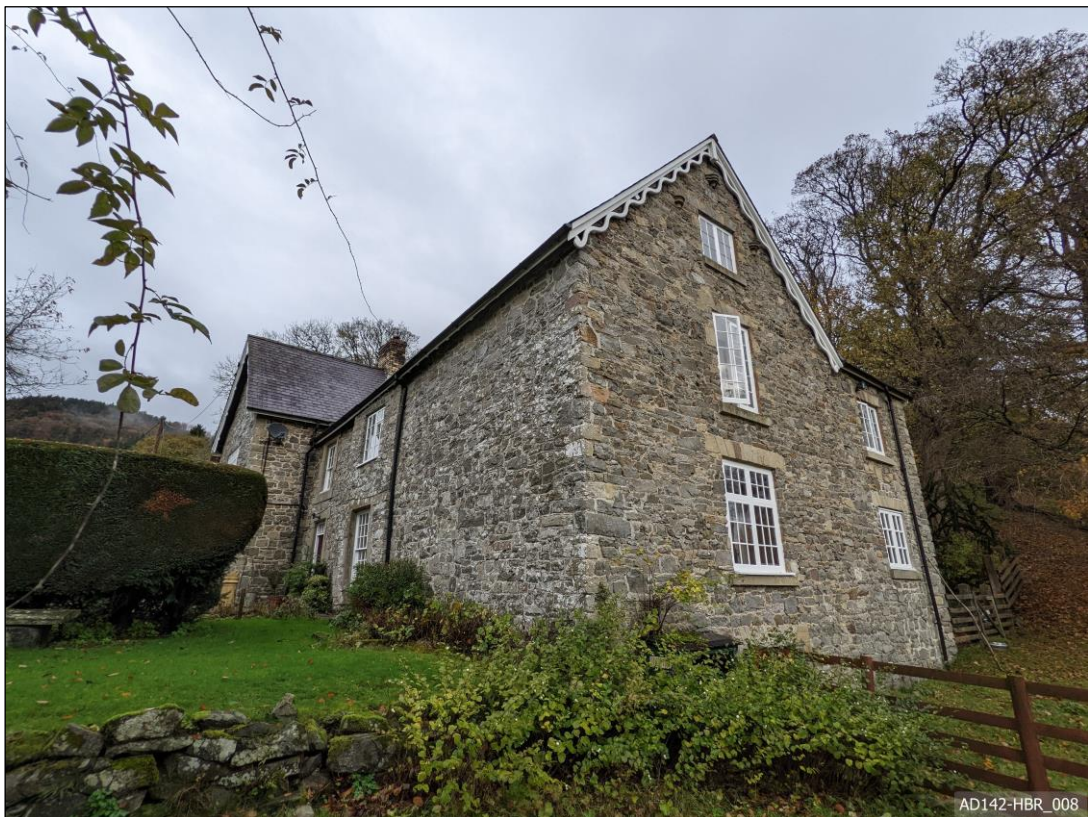
Plate 8 View north-east, showing \frac{3}{4} view of south and west elevations.
