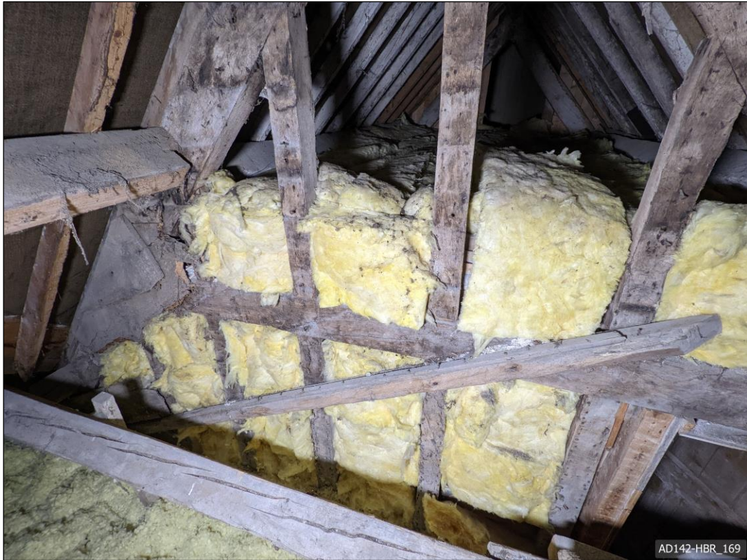
Plate 169 – View south-east, showing lower half of Truss 4.
