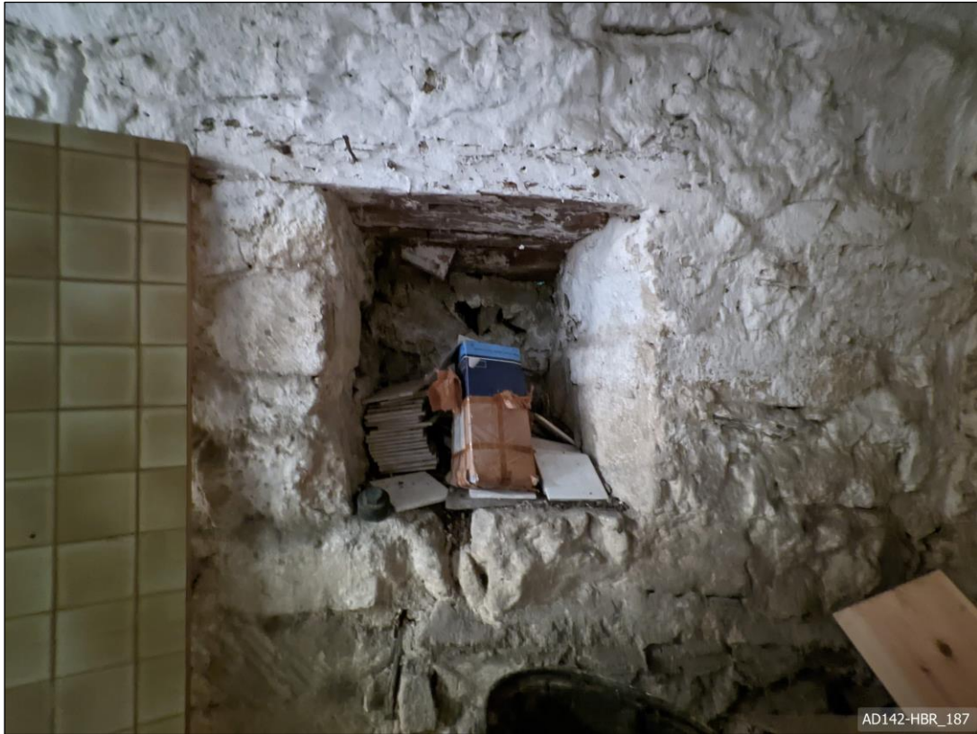
Plate 187 – View south, showing ventilation window to Cell B.
