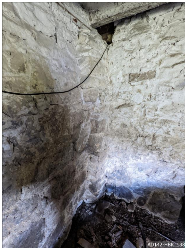
Plate 198 – View north, showing joint in masonry relating to south extension.
