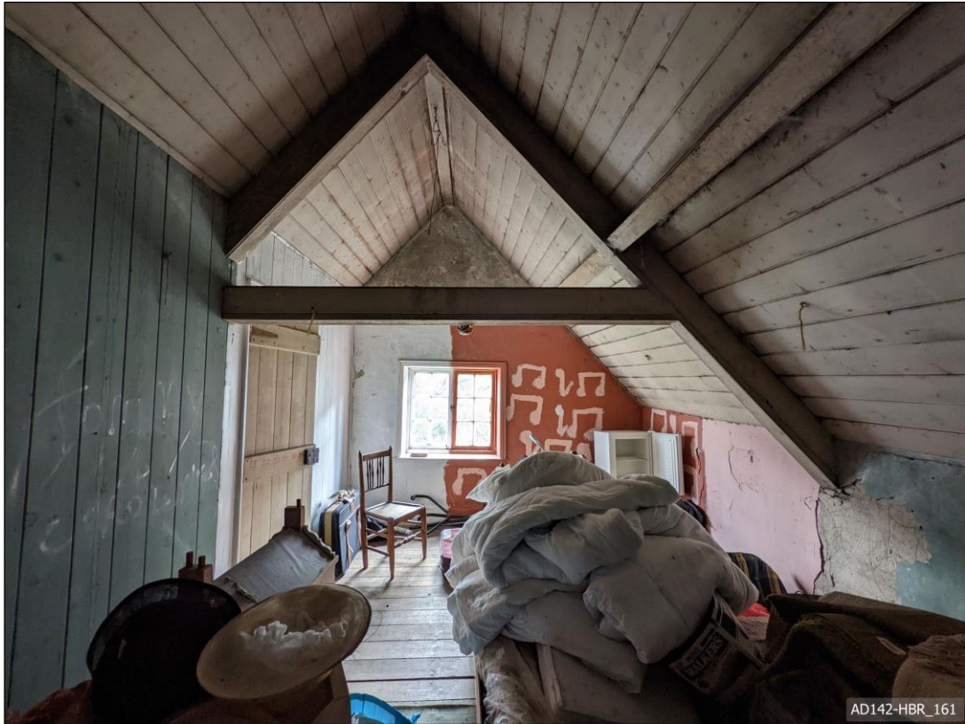
Plate 161 – View south, showing store room.
