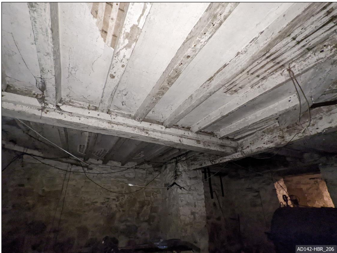
Plate 206 – View north-east, showing ceiling of Cell D.
