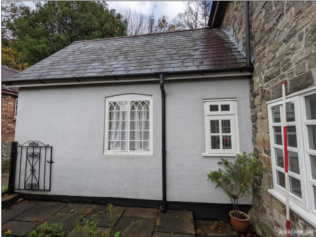
Plate 43 – View east, showing north elevation of north extension.
