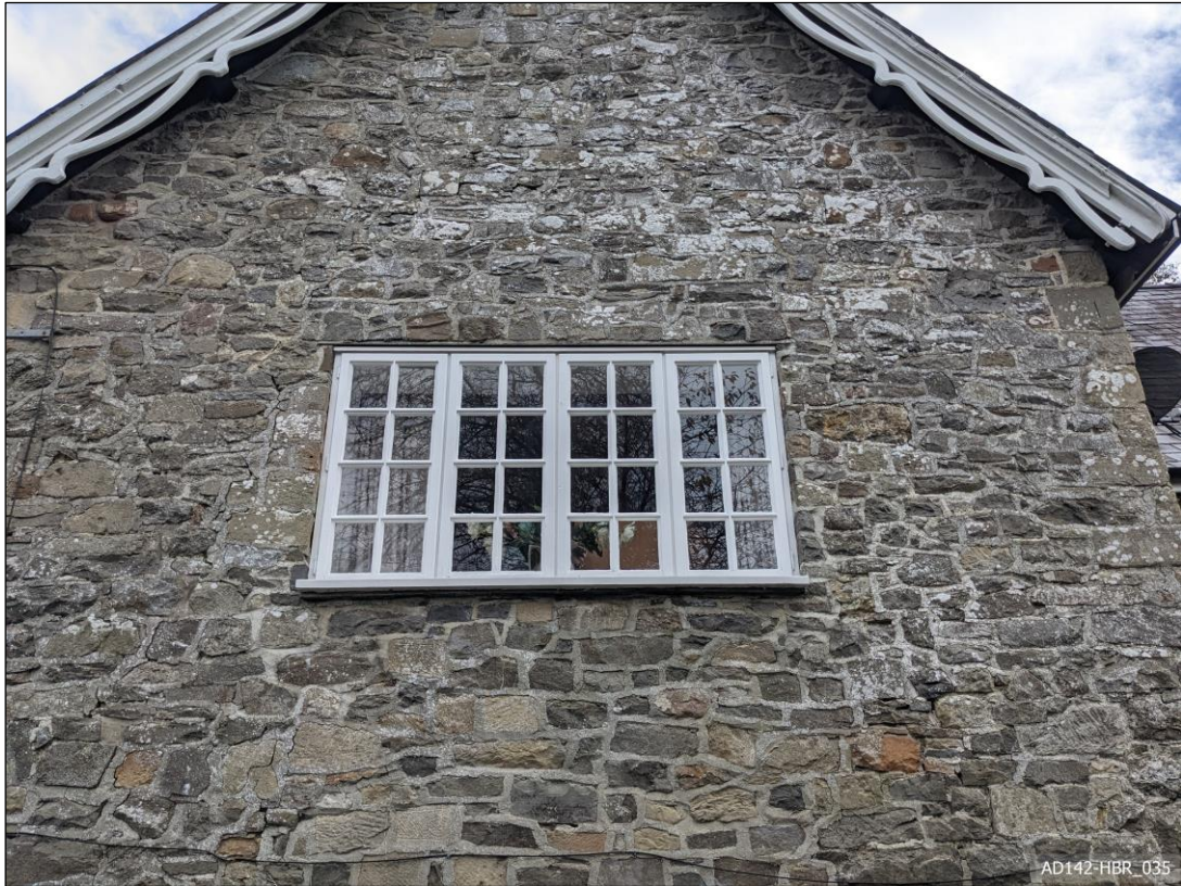
Plate 35 – View east, showing first floor window.
