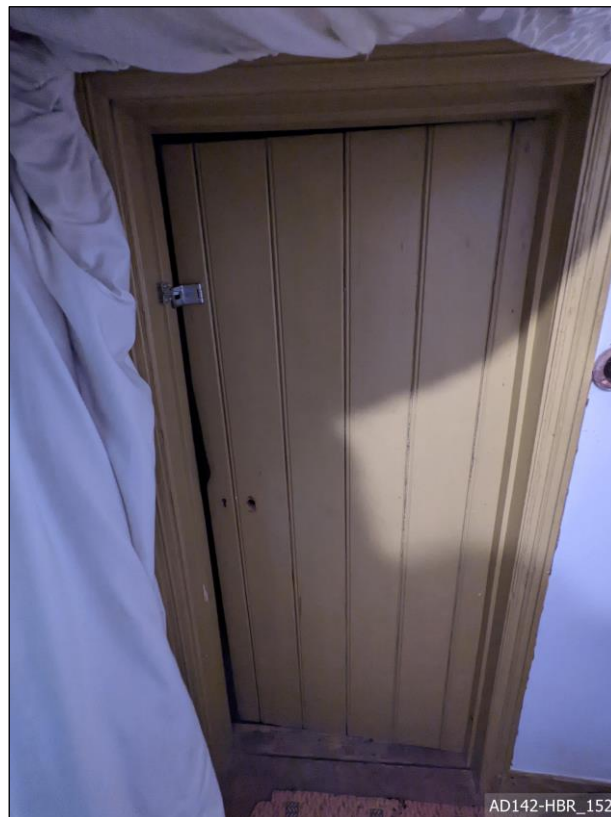
Plate 152 – View south, showing doorway to store room.
