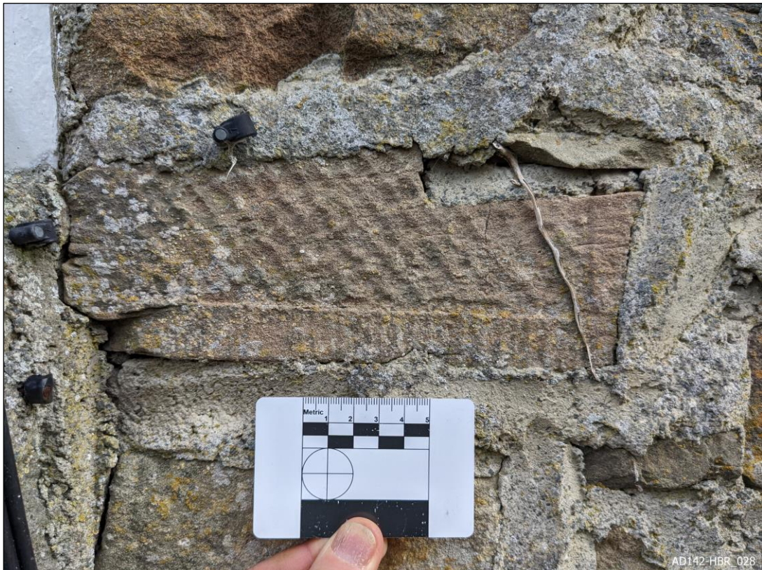
Plate 28 – View east, showing reused sandstone voussoir.
