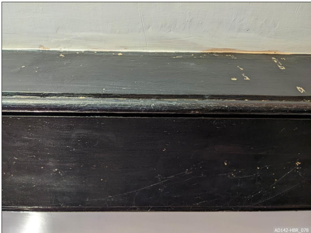
Plate 78 – View north, showing beaded boxing of transverse beam in dining room.
