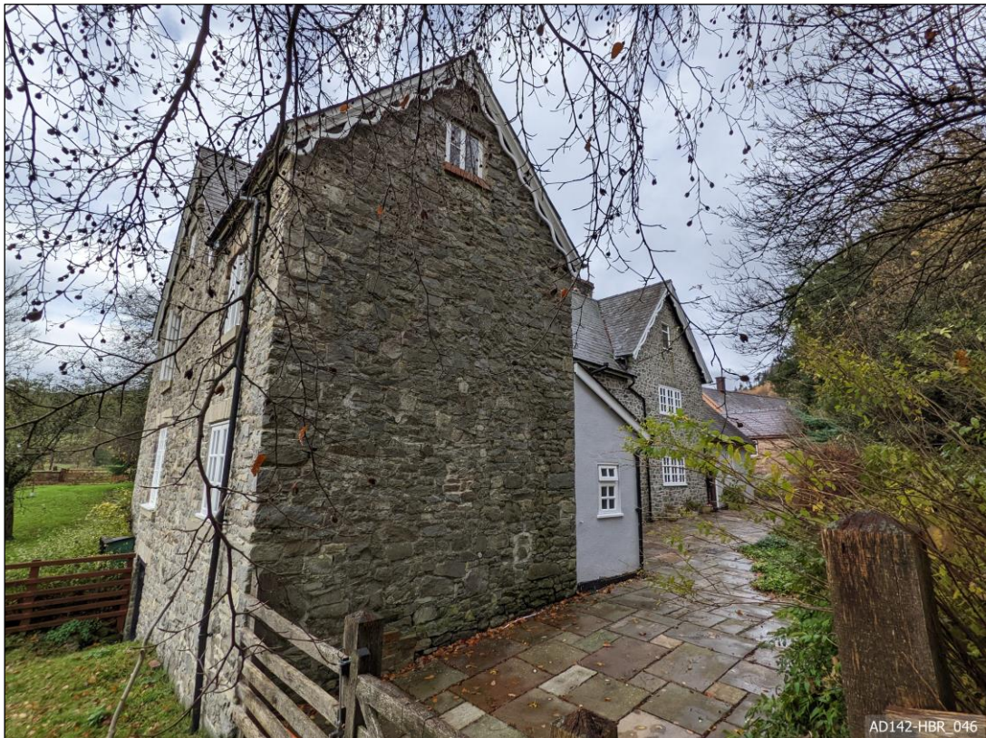
Plate 46 – View west, showing east elevation.
