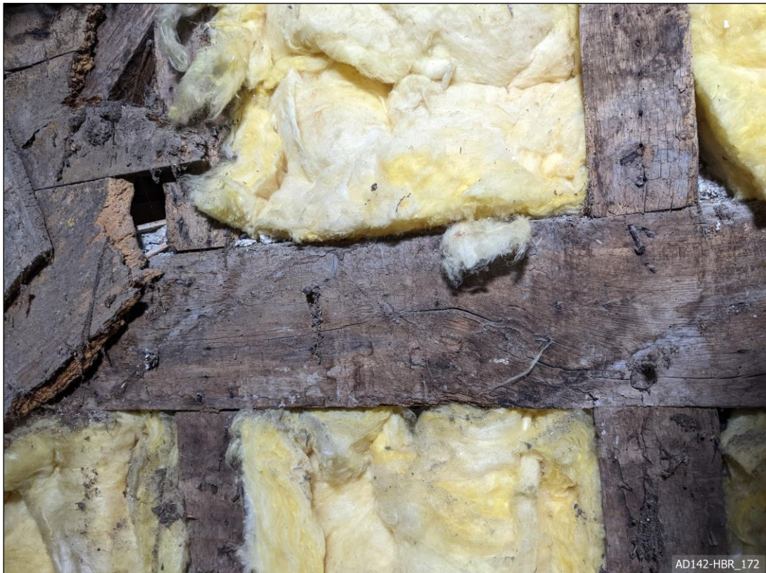
Plate 172 – View south, showing pegged and nailed studs of Truss 4.
