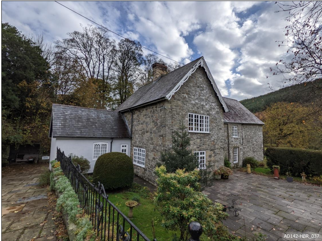
Plate 37 – View south-east, showing north and west elevations.
