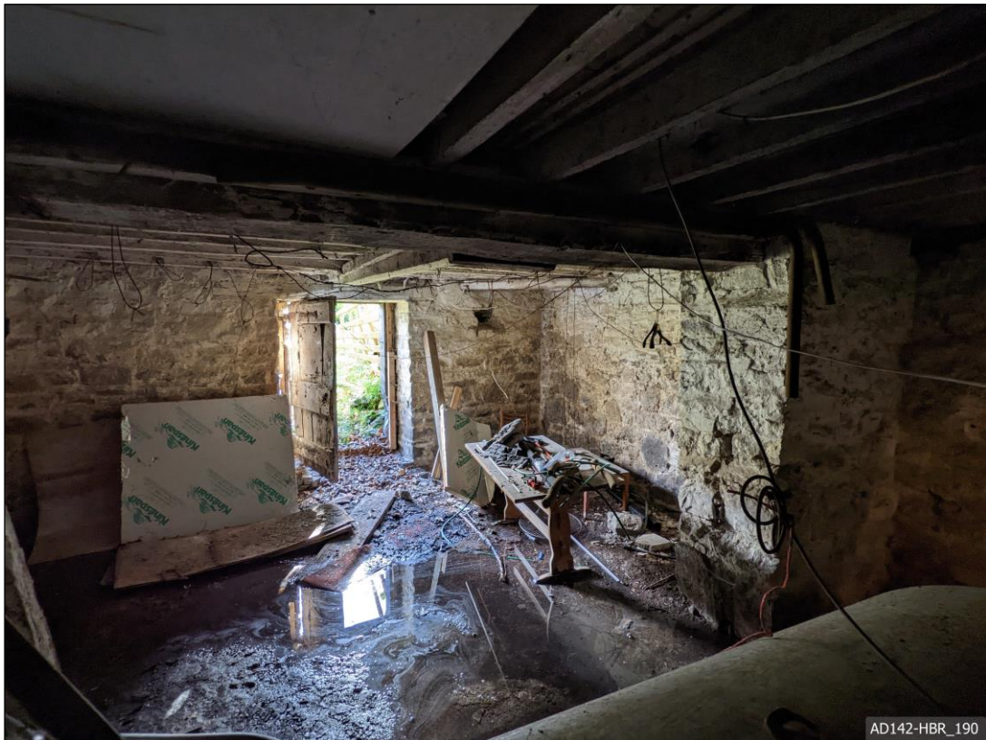
Plate 190 – View south-east, showing Cells C and D.
