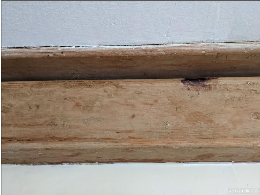
Plate 85 – View north, showing cornice in parlour.
