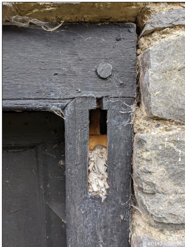
Plate 62 – View north, showing mortice to door frame.
