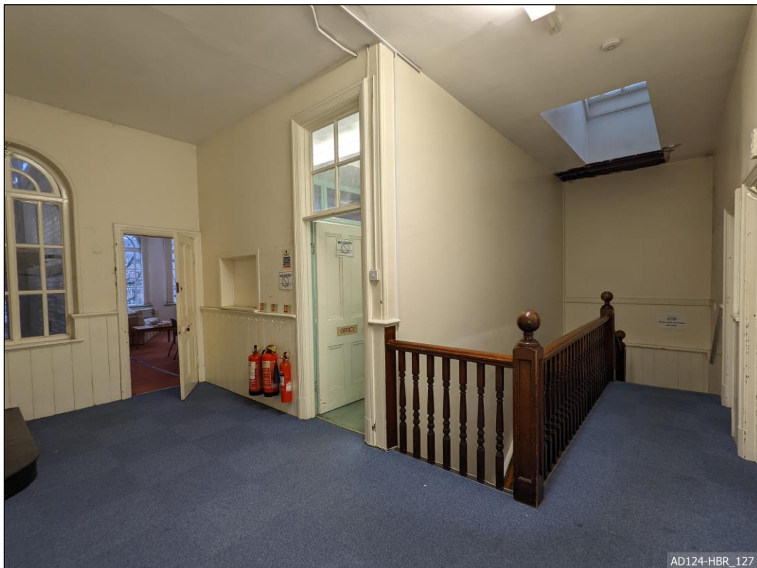
Plate 127 – View south-west, showing vestry stair and landing.
