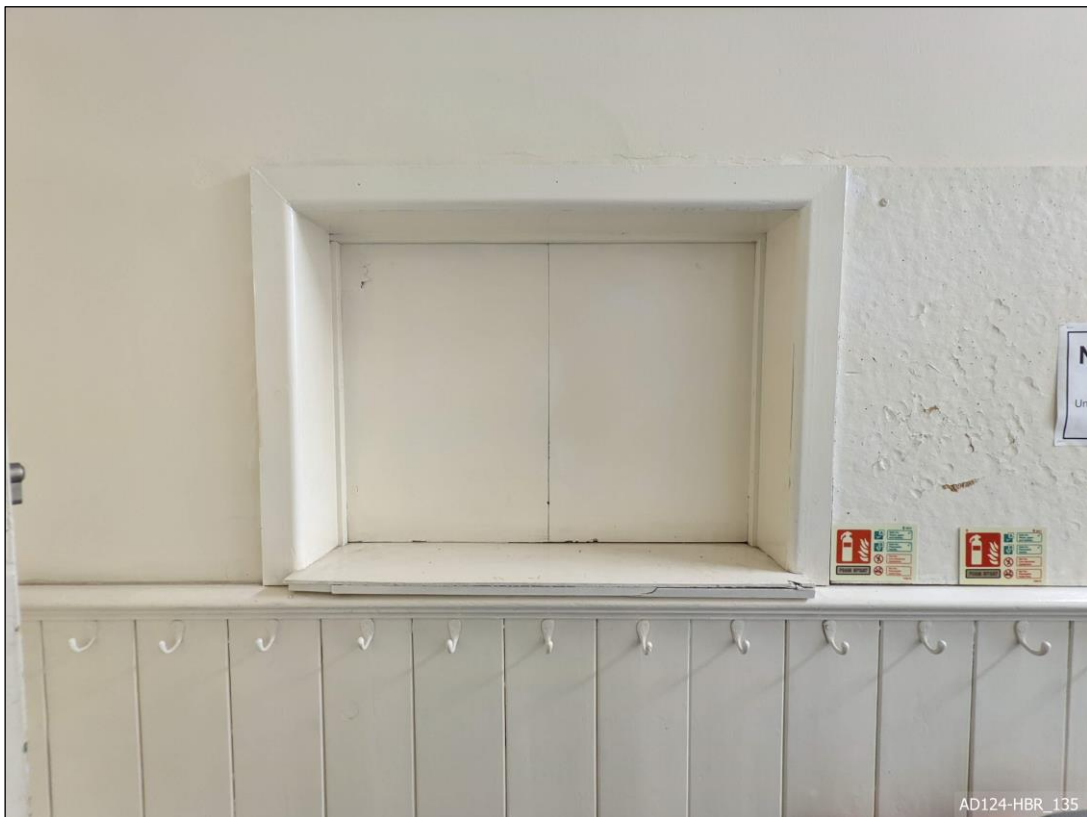
Plate 135 – View west, showing hatch to office from vestry office.
