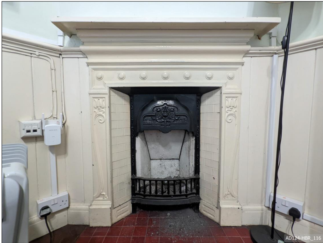
Plate 116 – View north-east, showing fireplace in vestry day room.
