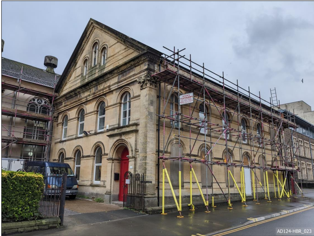
Plate 23 – View north-west, showing \frac{3}{4} view of lecture hall.
