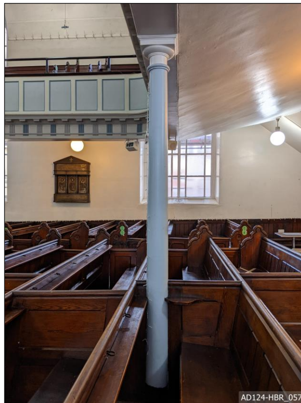
Plate 57 – View east, showing iron gallery column.
