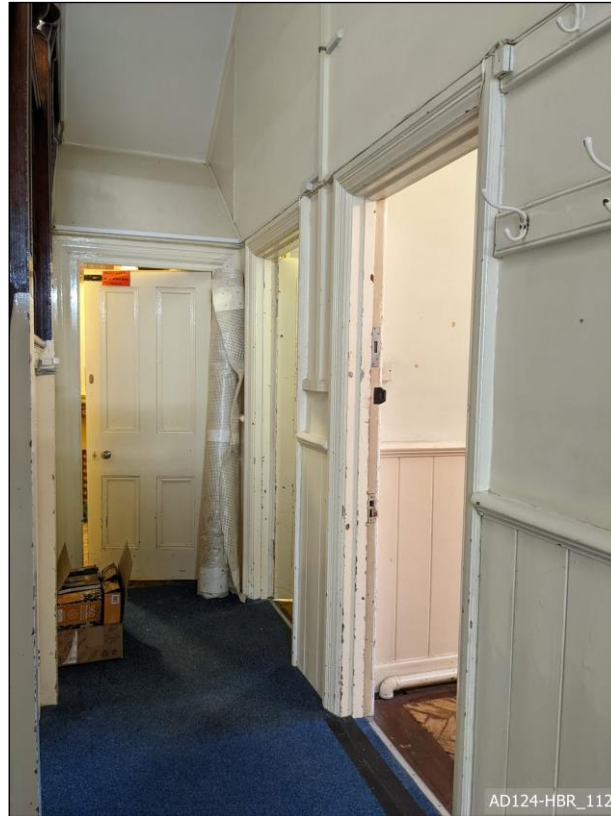
Plate 112 – View west, showing entrance to vestry and store rooms.
