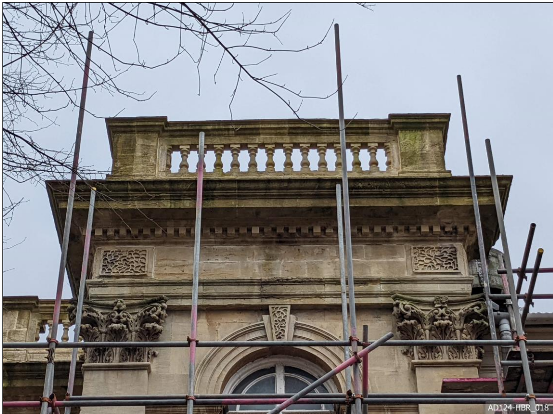
Plate 18 – View east, showing balcony to main chapel, with vermiculいた panels, and Corinthian pilaster capitals.
