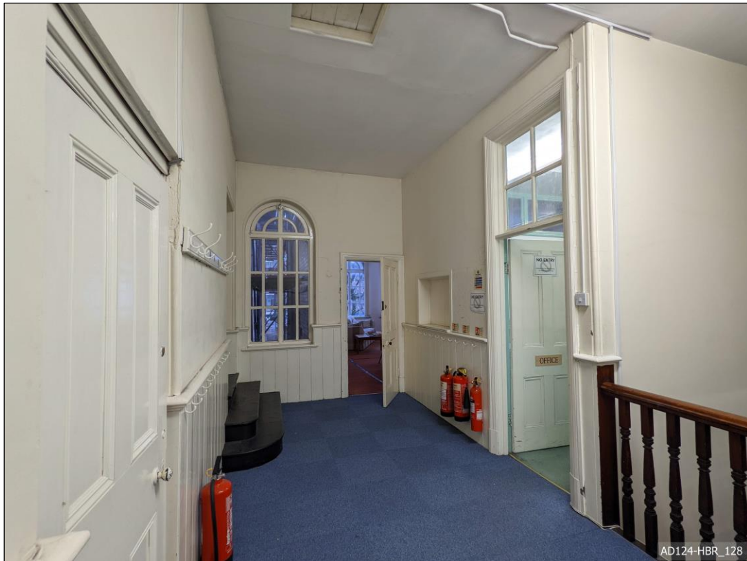
Plate 128 – View south, showing vestry landing and doorways to vestry office and first floor school room.
