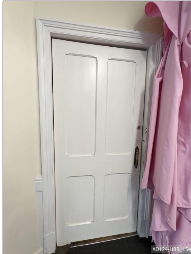
Plate 154 – View north, showing doorway to cupboard (former entrance lobby) of lecture hall.
