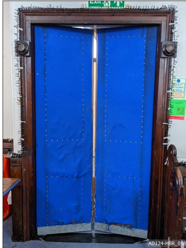
Plate 58 – View south, showing double doors to east lobby.
