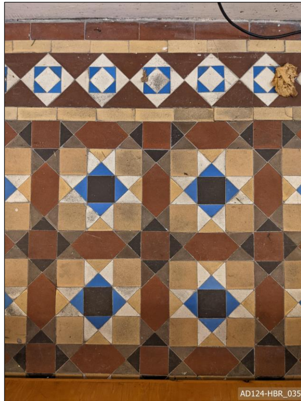
Plate 35 – Polychromatic tiling to entrance hall of chapel.
