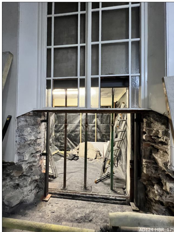
Plate 175 – View east, showing opened wall.
