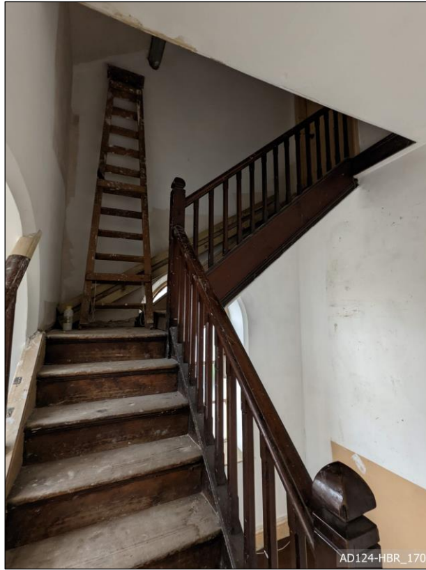
Plate 170 – View south, showing stair from south lobby of lecture hall.
