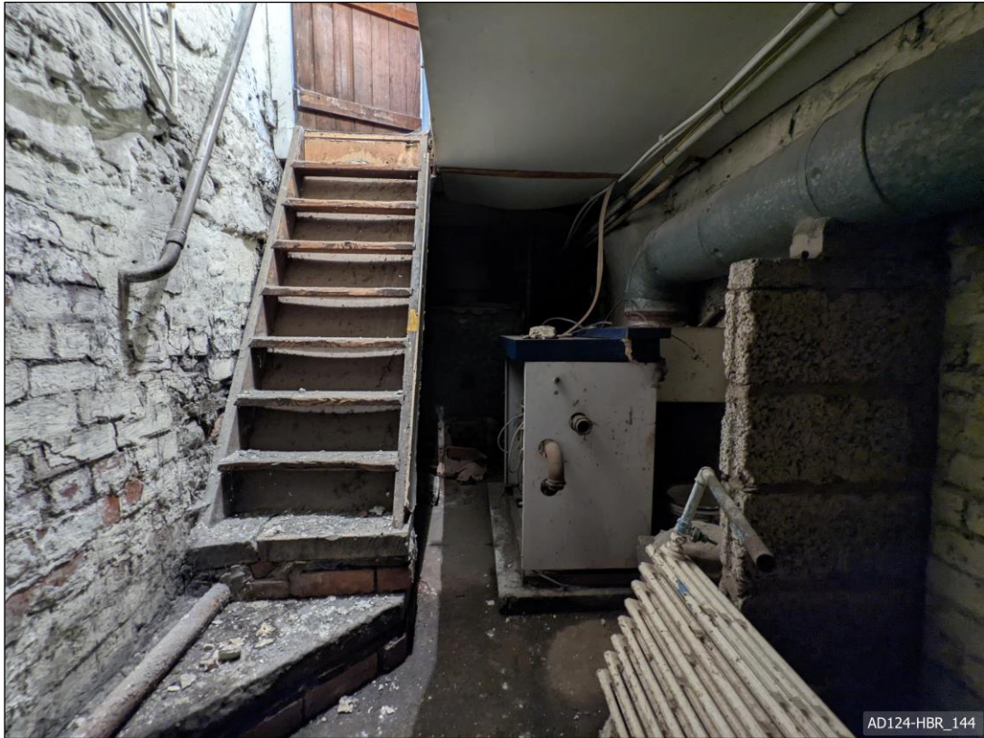
Plate 144 – View south, showing basement.
