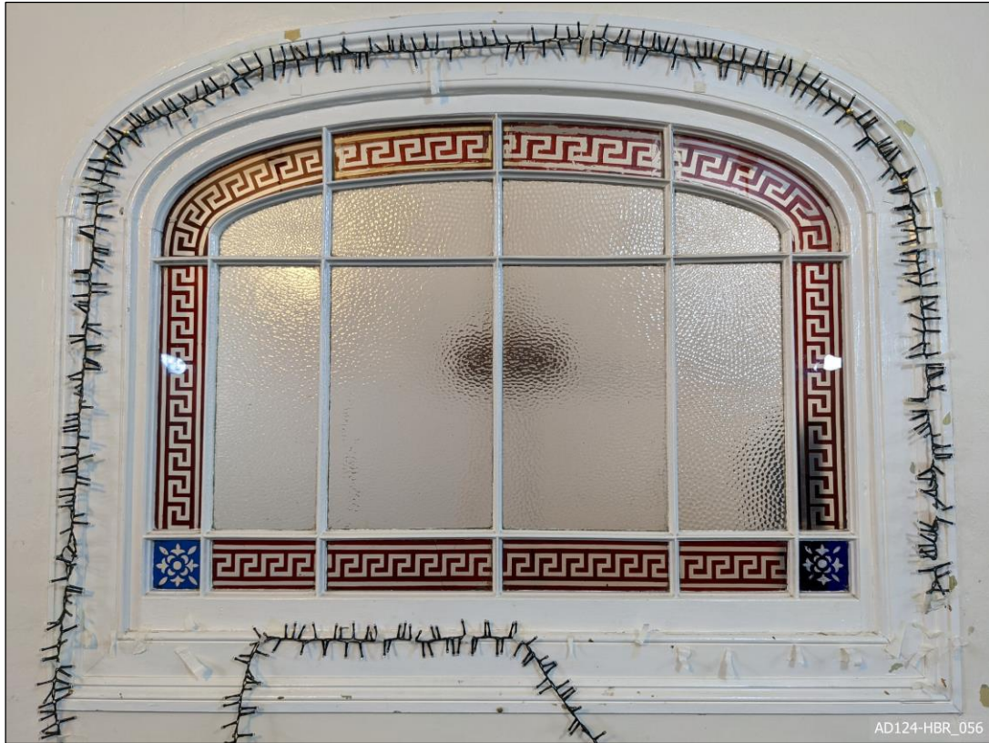
Plate 56 – View south, showing window between entrance hall and chapel hall.
