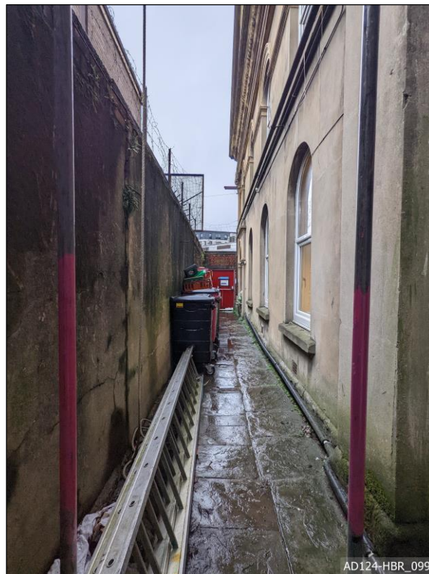
Plate 99 – View east, showing passageway to north of lecture hall.
