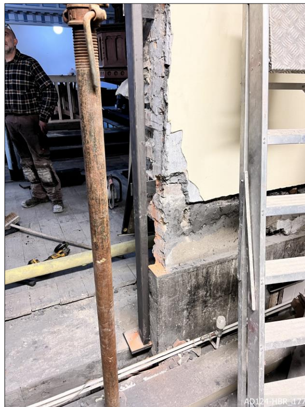
Plate 177 – View west, showing surviving plinth to chapel wall.
