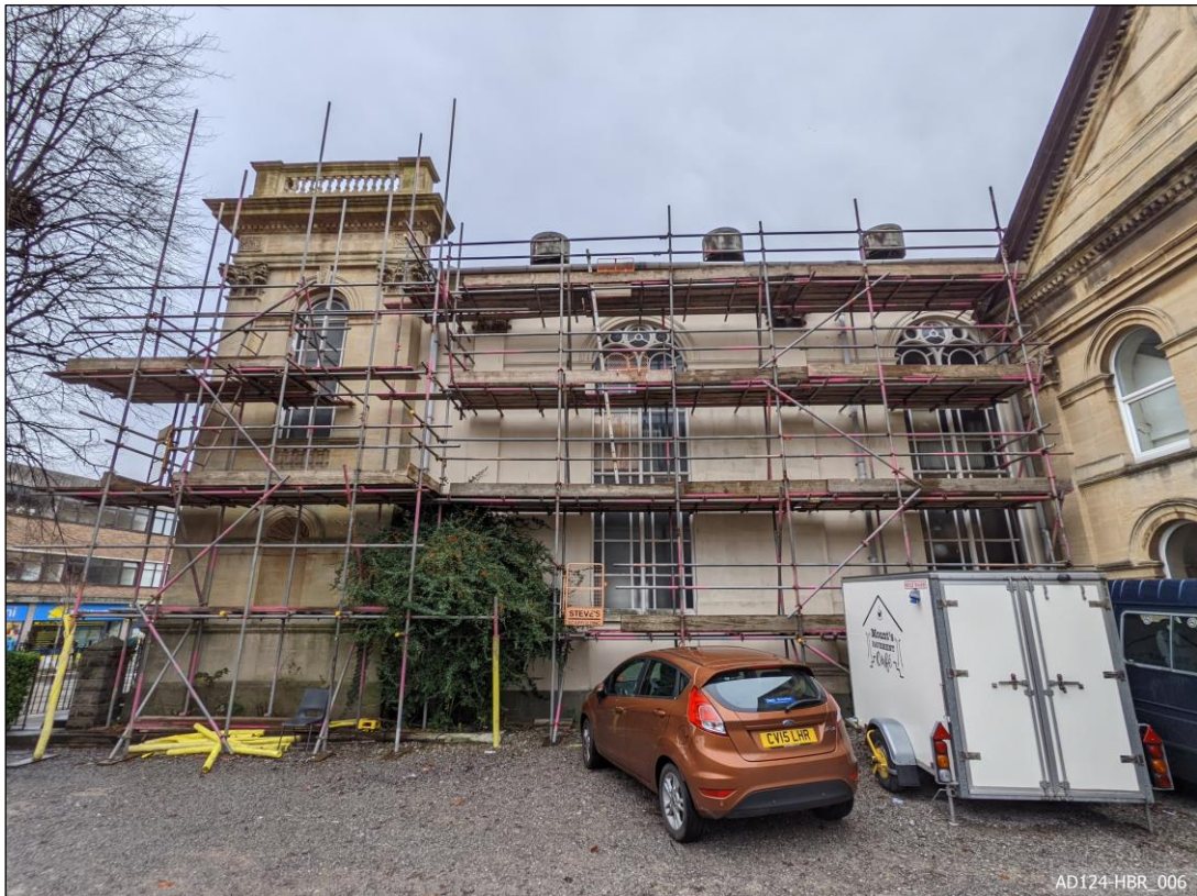
Plate 6 – View west, showing east elevation of main chapel.
