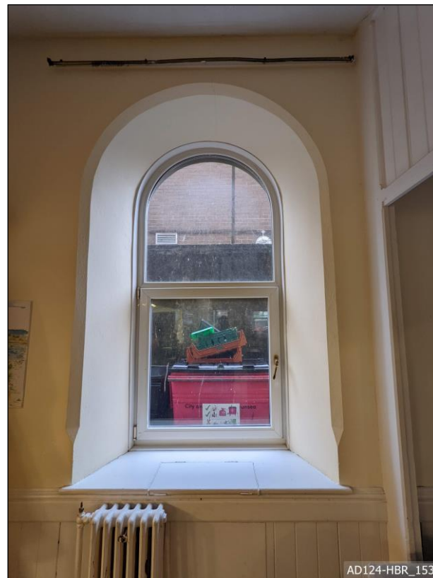
Plate 153 – View north, showing ground floor window of lecture hall.
