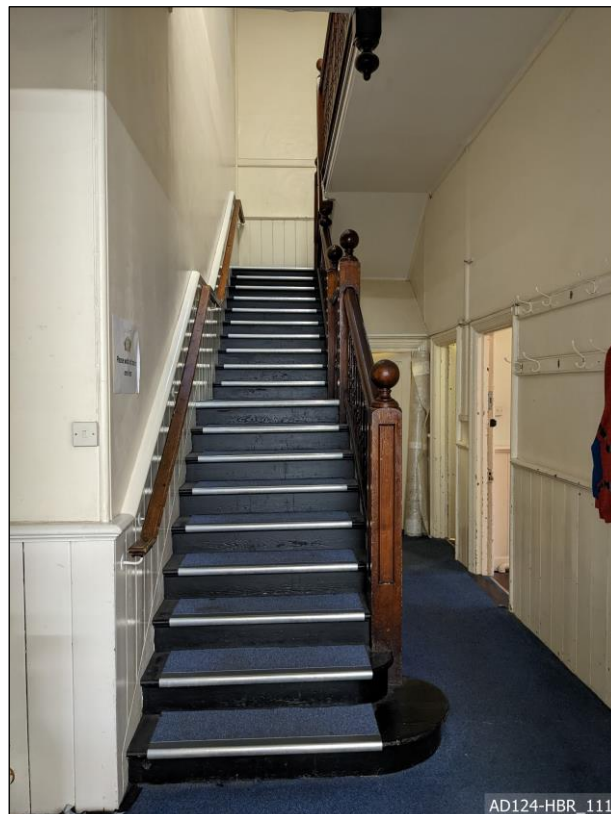
Plate 111 – View west, showing stair to first floor of vestry and school rooms.
