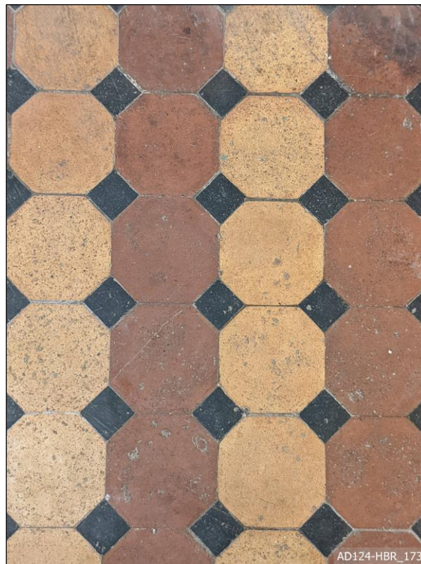
Plate 173 – View showing tiles in south lobby of lecture hall.
