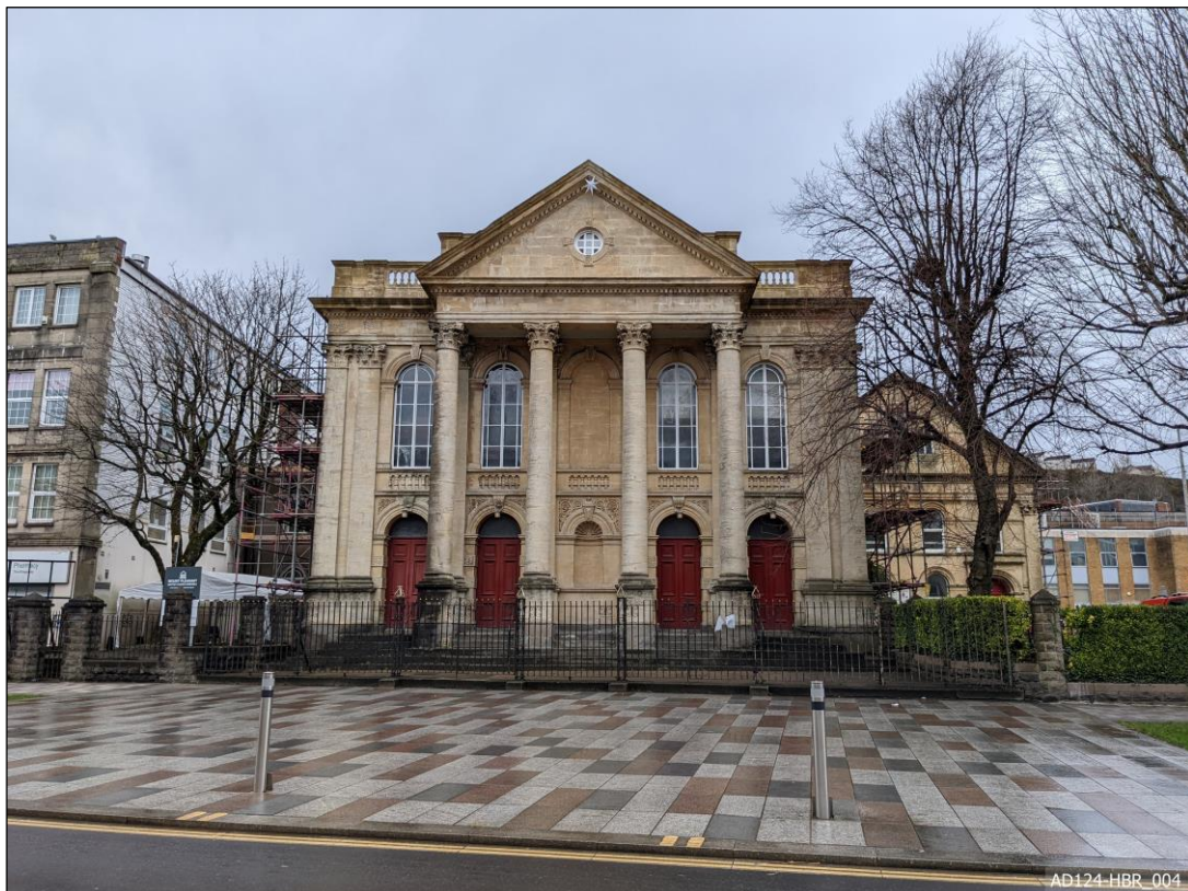
Plate 4 – View north, showing principal elevation, with lecture hall to east.
