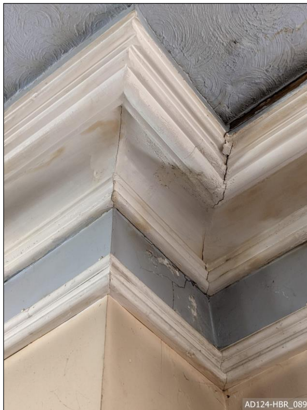
Plate 89 – View showing cornice detail of chapel hall.
