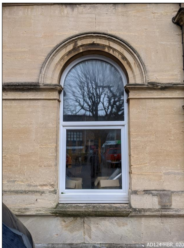
Plate 20 – View north, showing window of south elevation of lecture hall.
