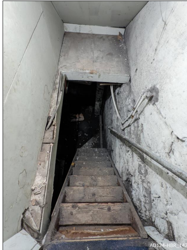
Plate 142 – View north, showing stairs to basement.
