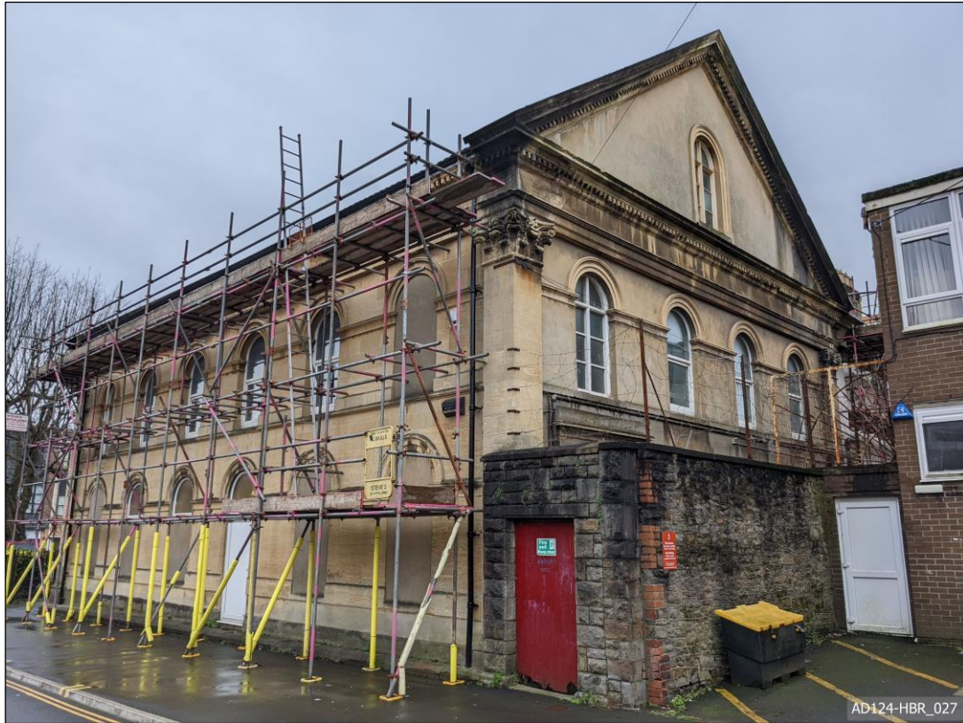
Plate 27 – View south-west, showing \frac{3}{4} view of lecture hall.
