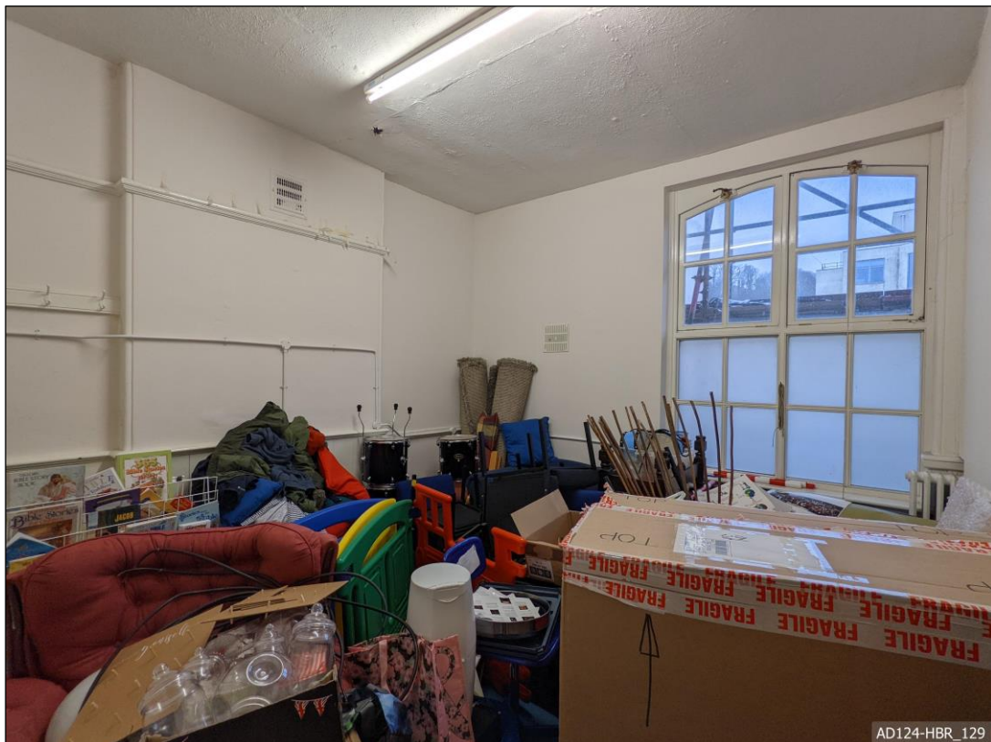
Plate 129 – View north-west, showing first floor vestry store room.
