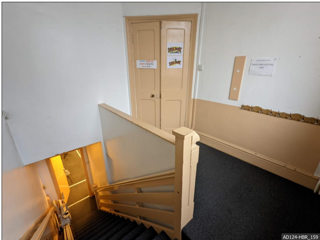
Plate 159 – View south-west, showing stair from ground floor of lecture hall.
