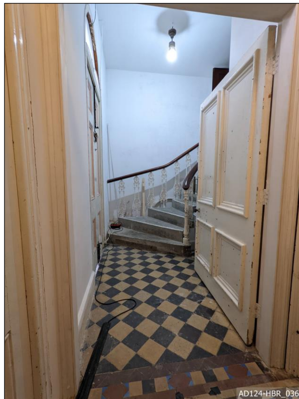
Plate 36 – View west, showing west stair to gallery.
