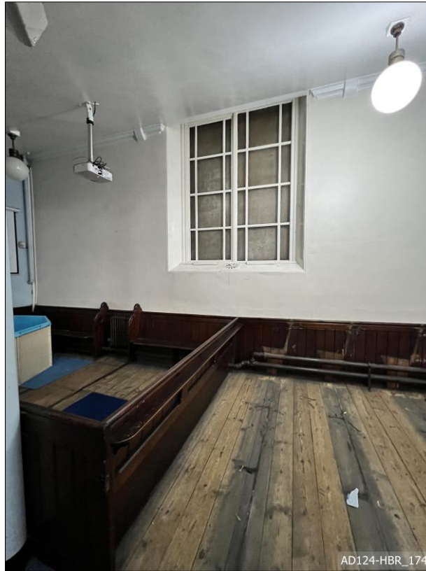
Plate 174 – View east, showing window to be opened into doorway.
