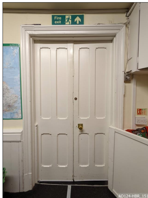
Plate 151 – View west, showing access to corridor.
