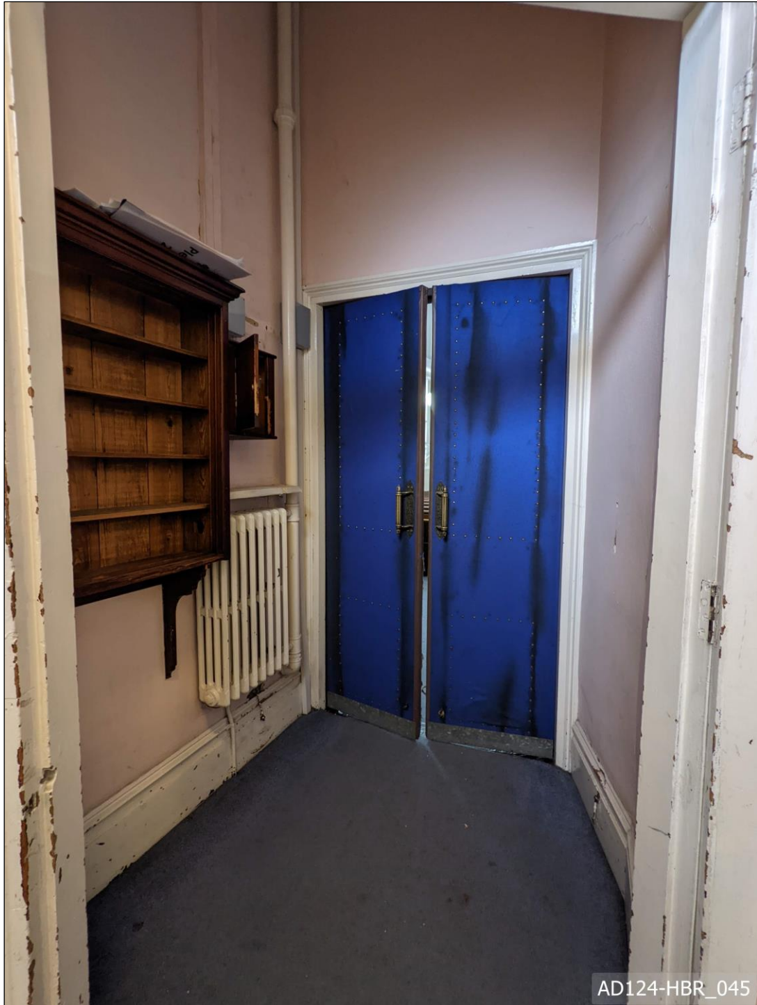
Plate 45 – View north, showing west lobby from entrance hall to chapel hall.
