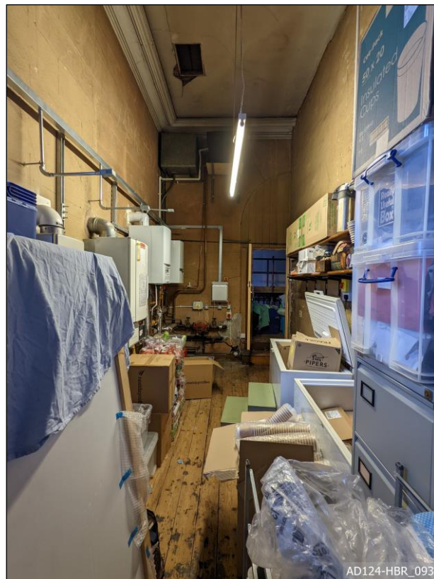
Plate 93 – View east, showing first floor store room.
