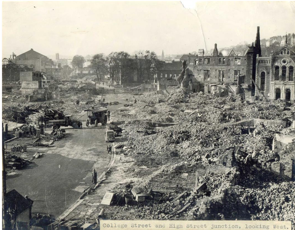
Fig. 8 – Bomb damage surrounding Mount Pleasant, WWII, 1941.
