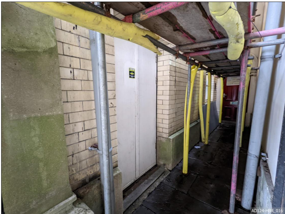
Plate 16 – View north-west, showing brick lateral wall to school rooms.
