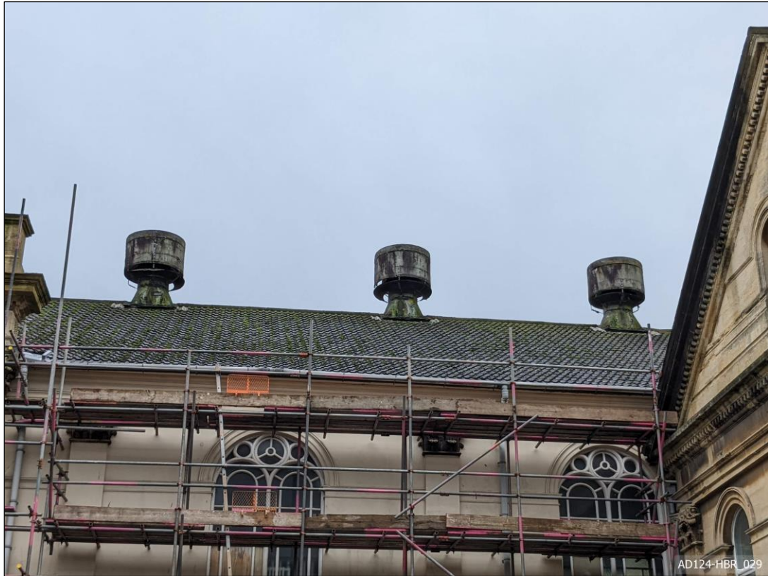
Plate 29 – View west, showing ventilation cowls to roof of main chapel.
