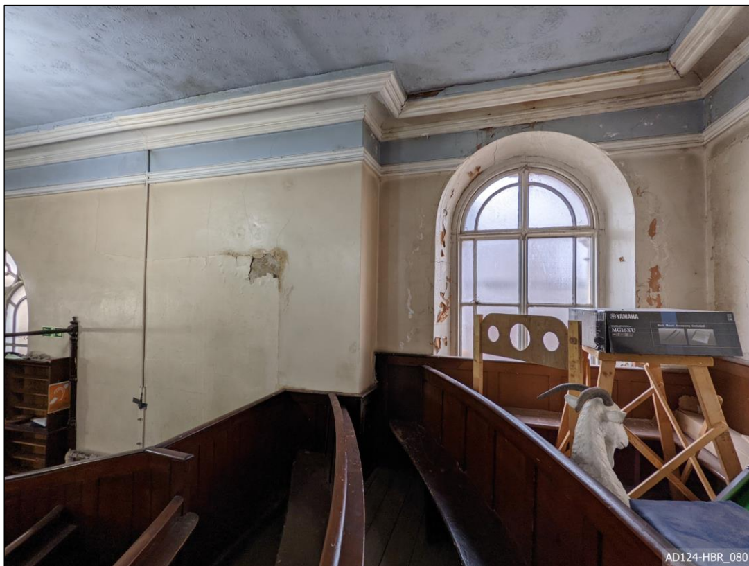
Plate 80 – View east, showing return between original chapel of 1825 and 1875 alterations.
