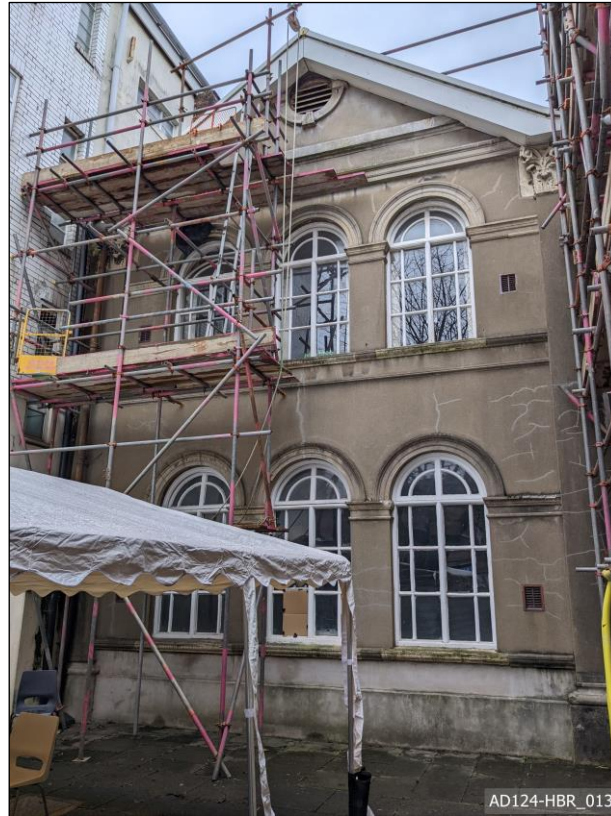
Plate 13 – view north, showing south elevation of school rooms.
