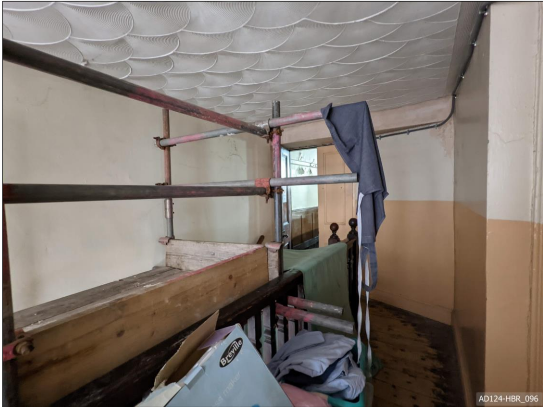
Plate 96 – View south, showing landing and doorway to chapel hall gallery.
