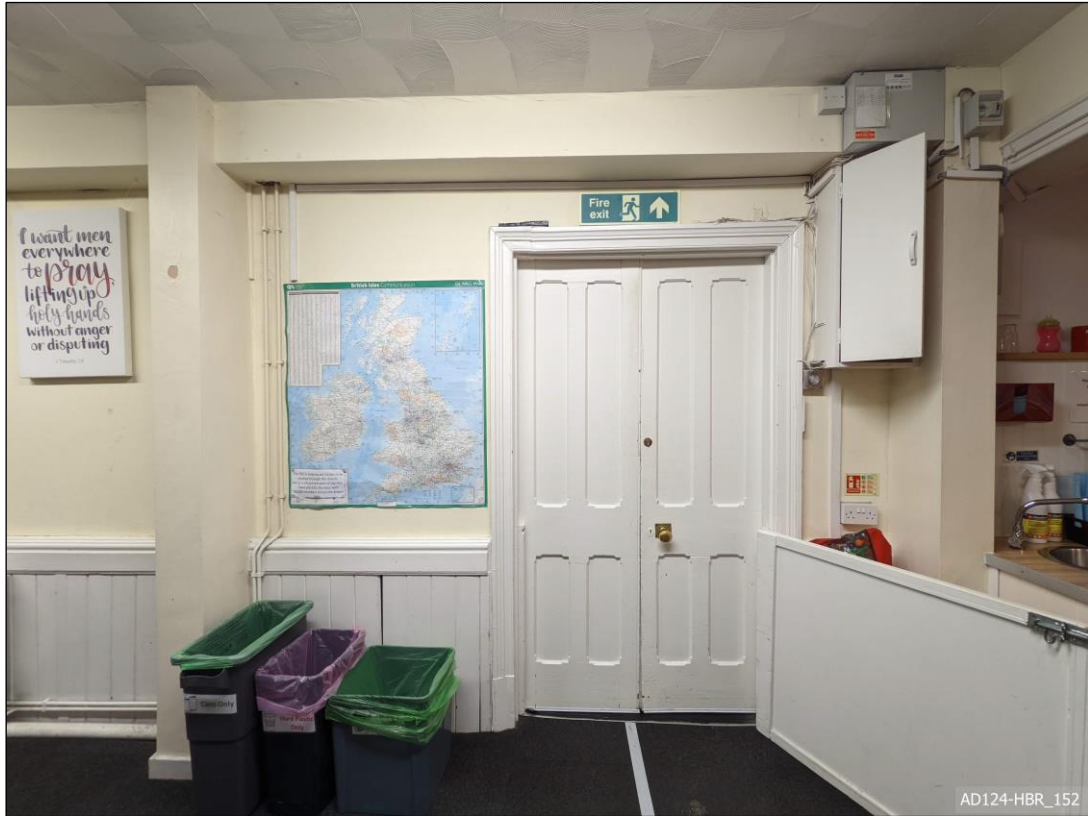
Plate 152 – View west, showing access to corridor.
