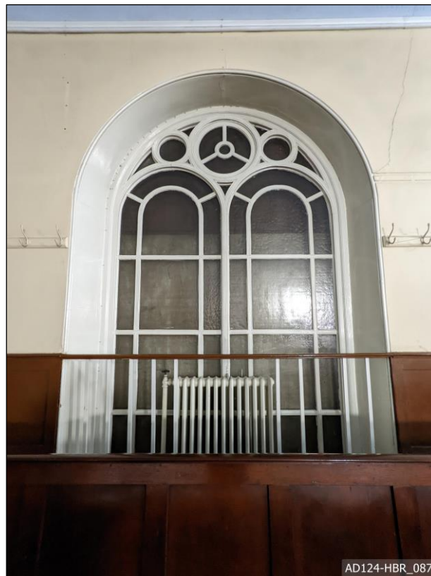
Plate 87 – View east, showing window blocked by 1885 addition of lecture hall.
