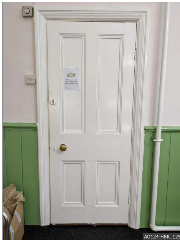
Plate 125 – View east, showing doorway to ground floor school room.
