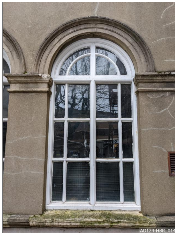
Plate 14 – View north, showing window of school rooms.
