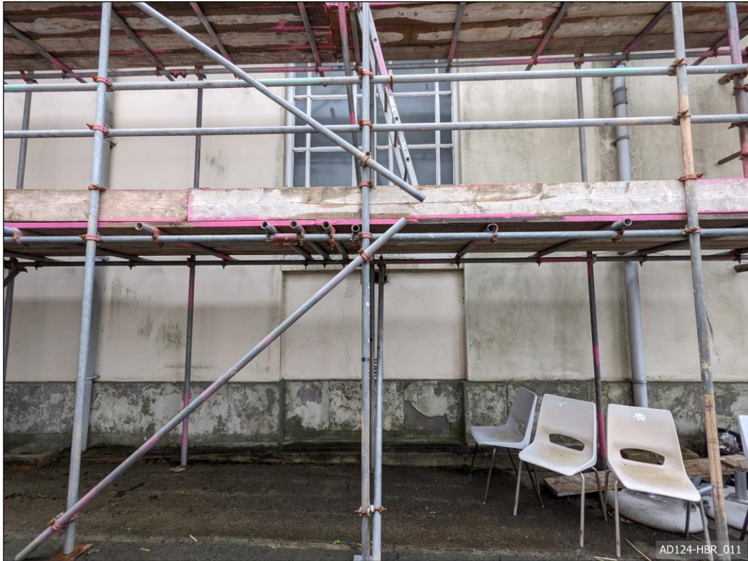
Plate 11 – View east, showing location of new disabled access (through window).
