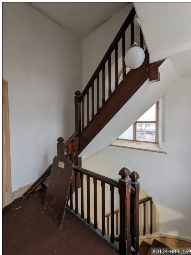
Plate 169 – View north-east, showing stair from south lobby of lecture hall.
