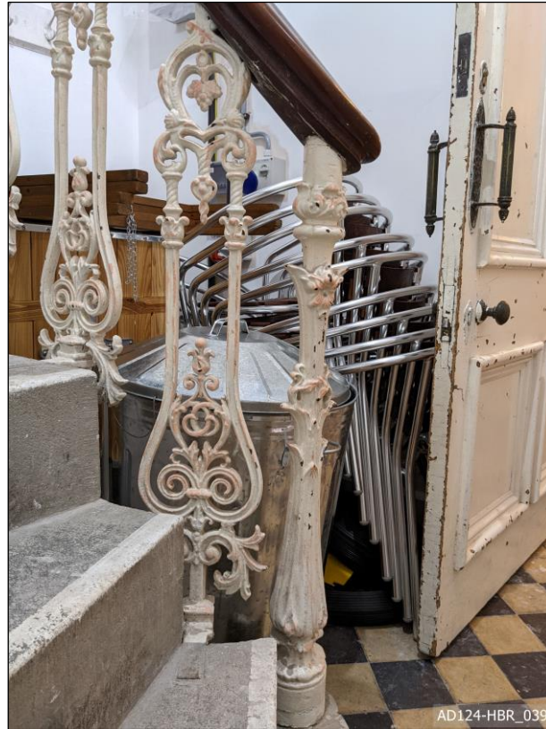
Plate 39 – View east, showing iron newel and baluster of west stair.
