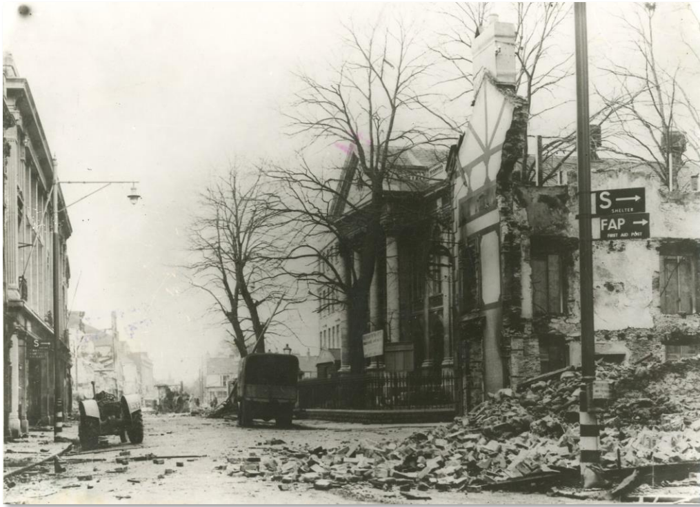
Fig. 9 – Bomb damage around Mount Pleasant, WWII, 1941. N.B. Ventilation cowls to roof.
