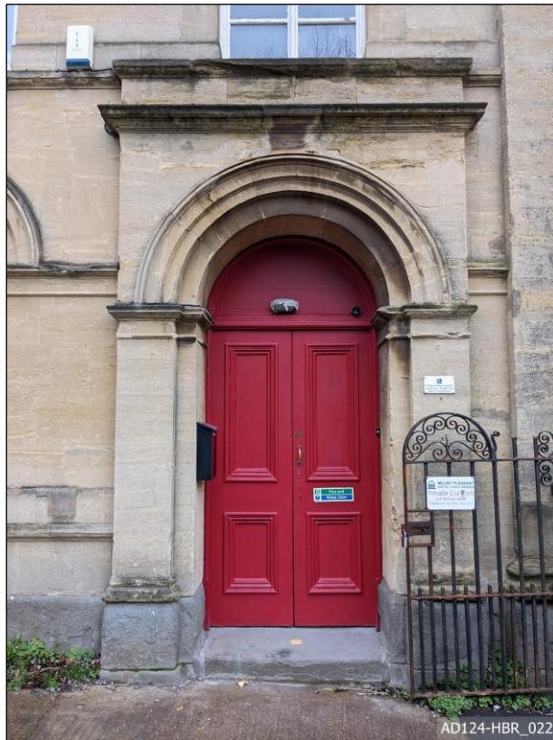
Plate 22 – View north, showing entrance to lecture hall from south.
