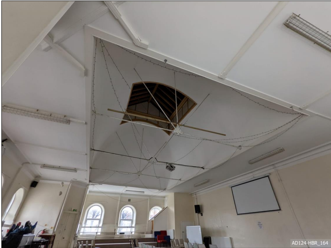
Plate 164 – View south-west, showing lantern over lecture hall.
