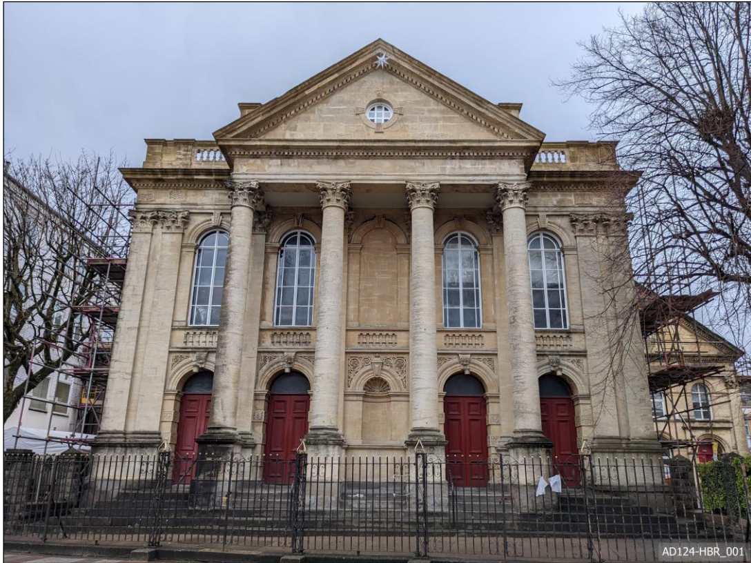
Plate 1 – View north, showing principal elevation.
