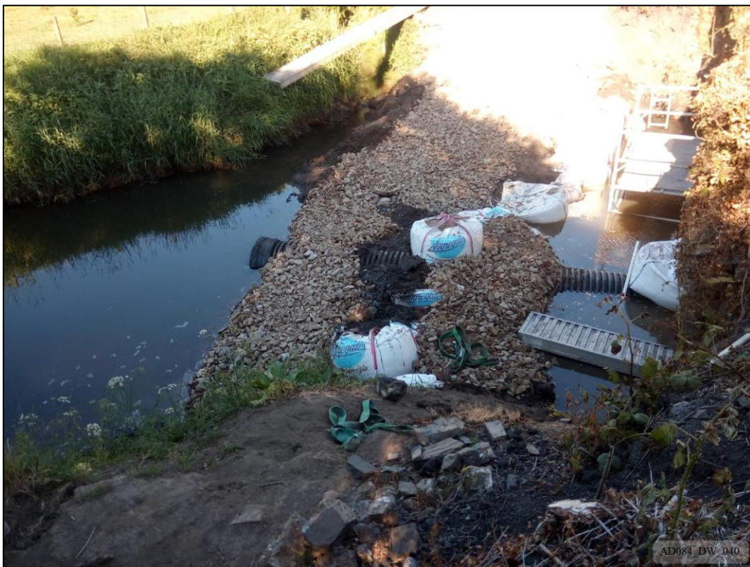
Plate 40 – During works – View east, showing damming of river.
