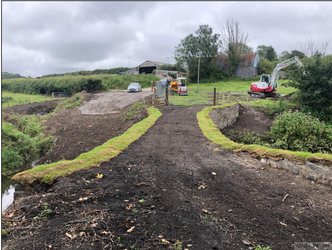
Plate 99 – Post-works – View east, showing completed roadway with turf wall capping.
