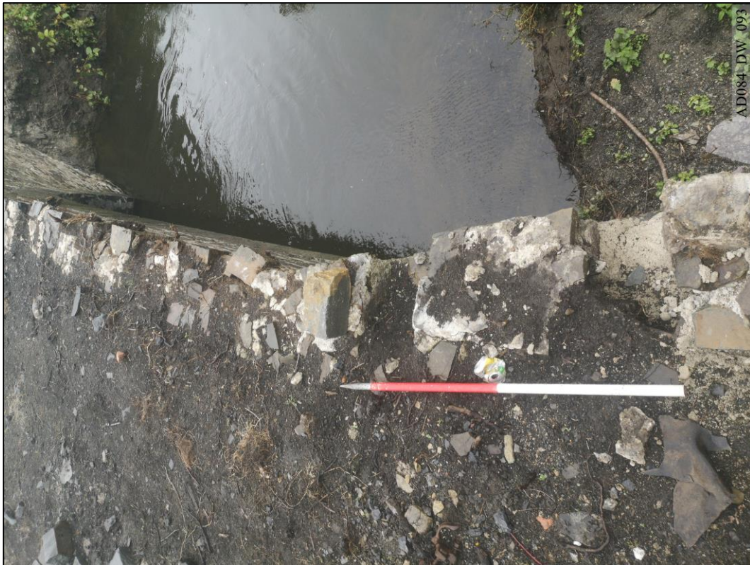
Plate 93 – During works – Wall top to south elevation, showing opening in masonry.
