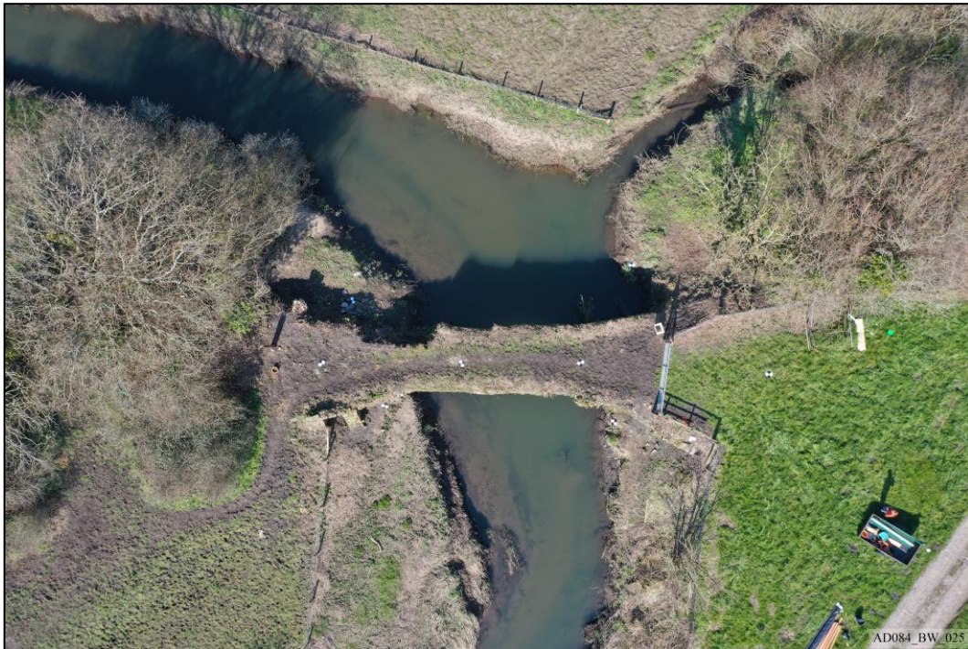
Plate 25 – Pre-works – Nadir view, after clearance works.
