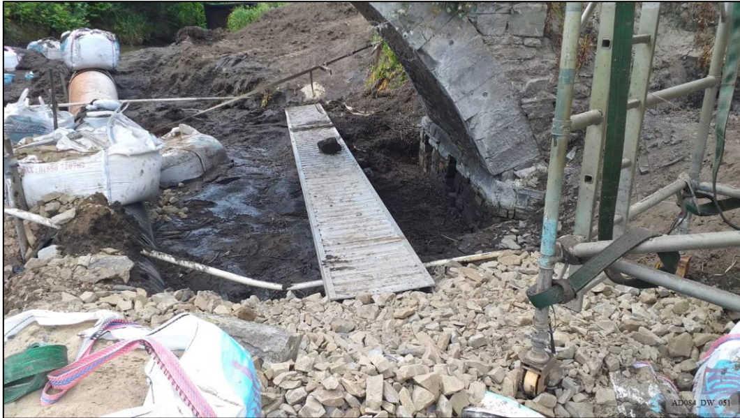
Plate 51 – During works – View south, showing lower west abutment.
