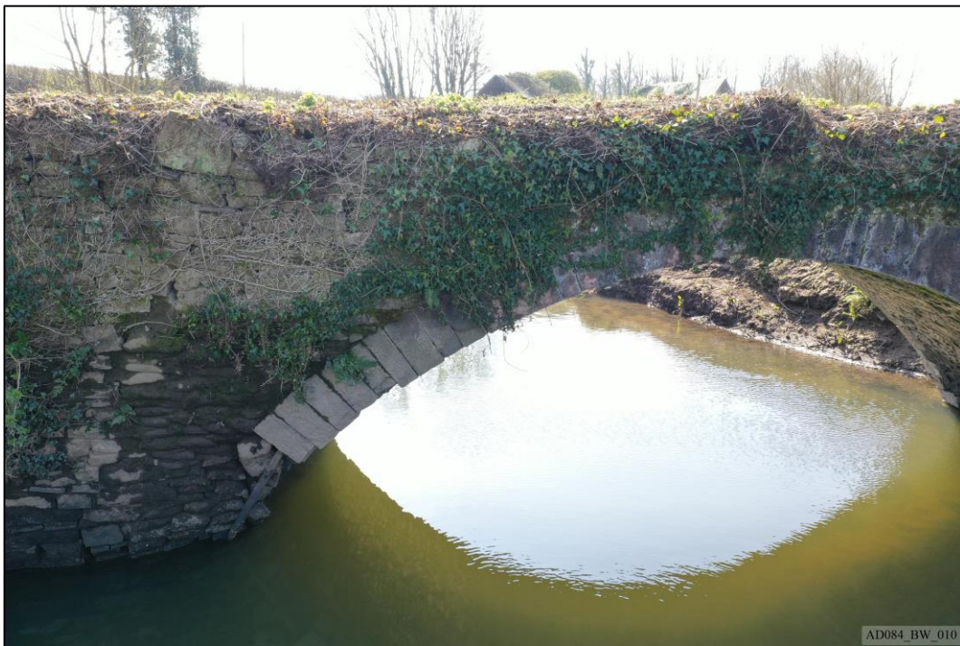
Plate 10 – Pre-works – North elevation, showing abutment and arch.
