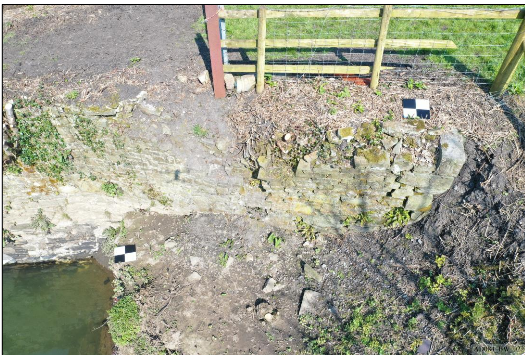
Plate 22 – Pre-works – South elevation, showing east wing wall.
