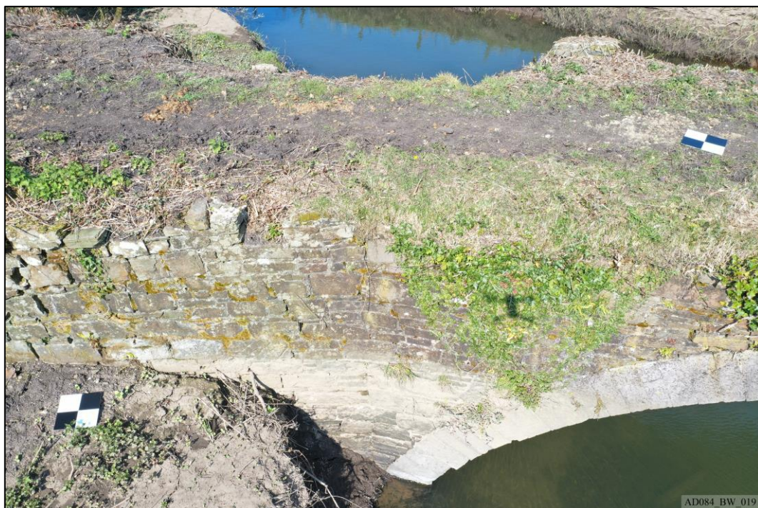
Plate 19 – Pre-works – South elevation, showing arch and west abutment.
