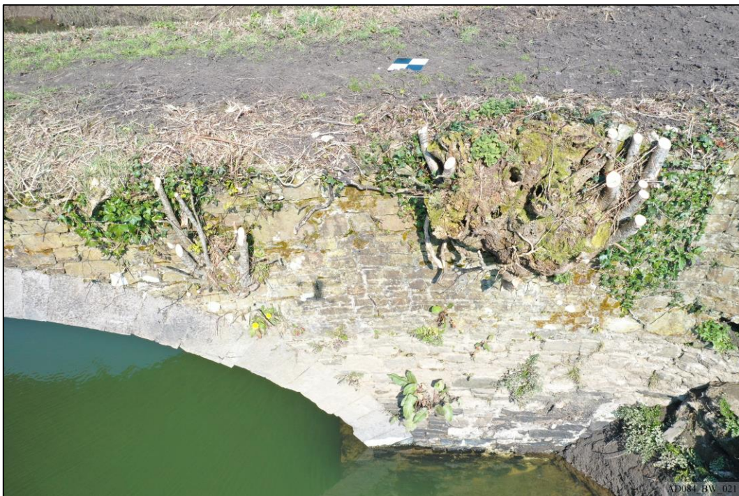
Plate 21 – Pre-works – South elevation, showing arch and east abutment.
