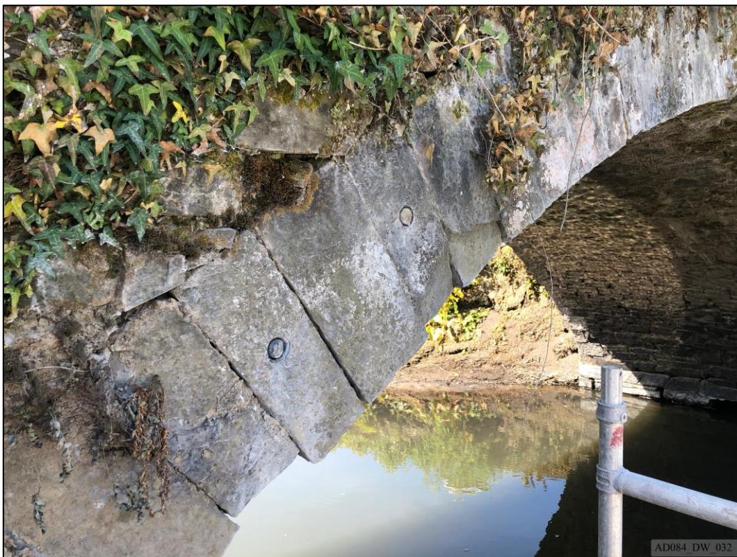
Plate 32 – During works – North elevation, showing Cintec anchors to voussoirs.
