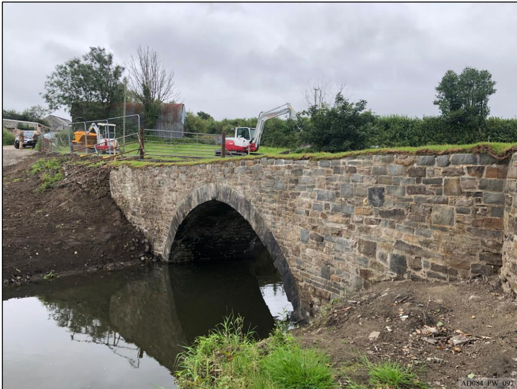
Plate 97 – Post-works – Completed north elevation.
