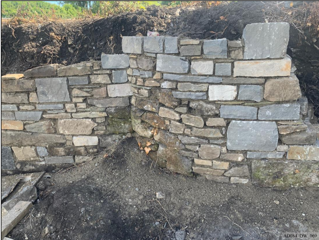
Plate 69 – During works – North elevation, rebuilding of west wing and retaining wall.
