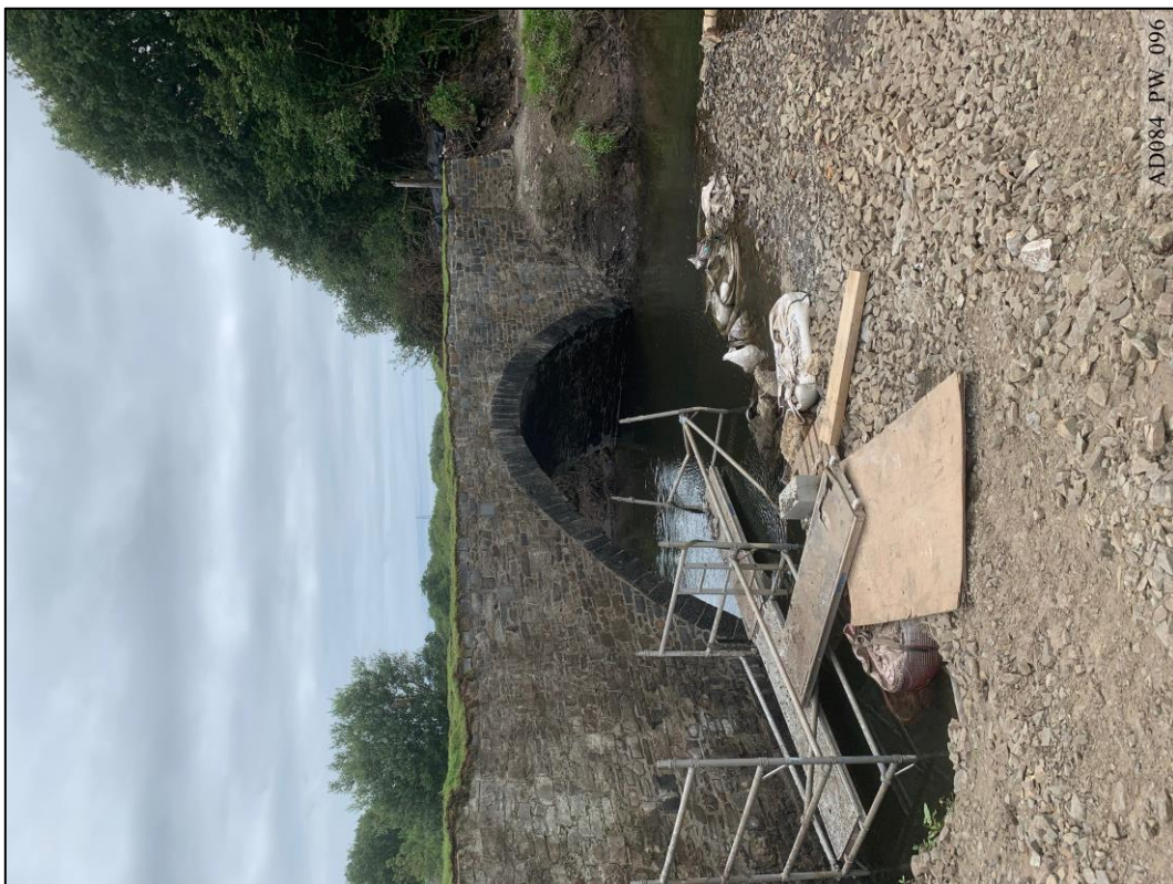
Plate 96 – Post-works – Completed north elevation.
