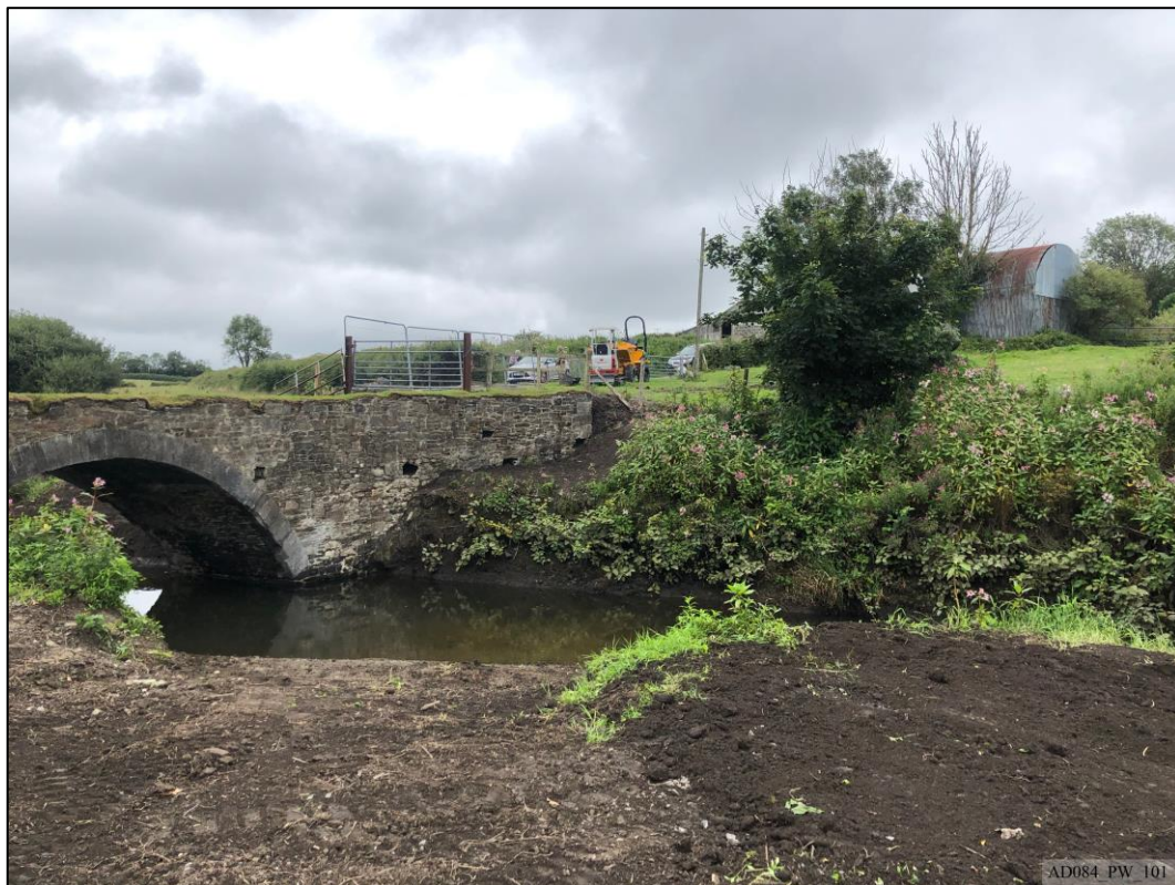
Plate 101 – Post-works – View north-east, showing cleared banks and bridge.
