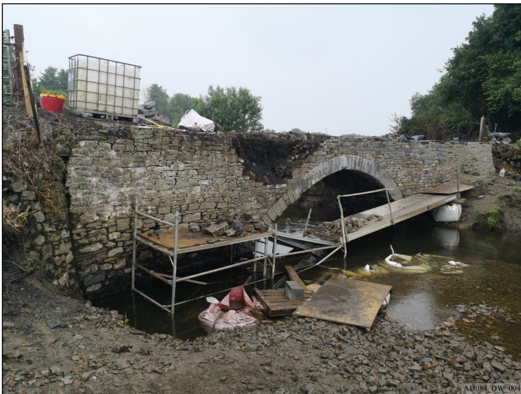
Plate 94 – During works – North elevation, showing collapse of east spandrel.
