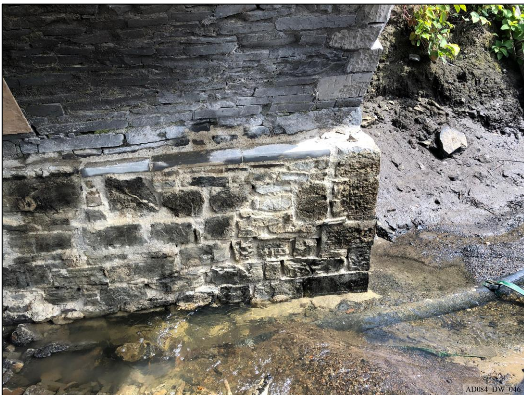
Plate 46 – During works – View east, showing repair to east abutment.
