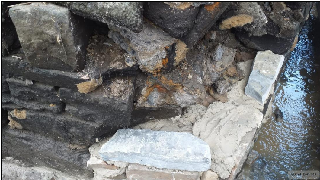
Plate 45 – During works – North elevation, showing repair to east abutment.
