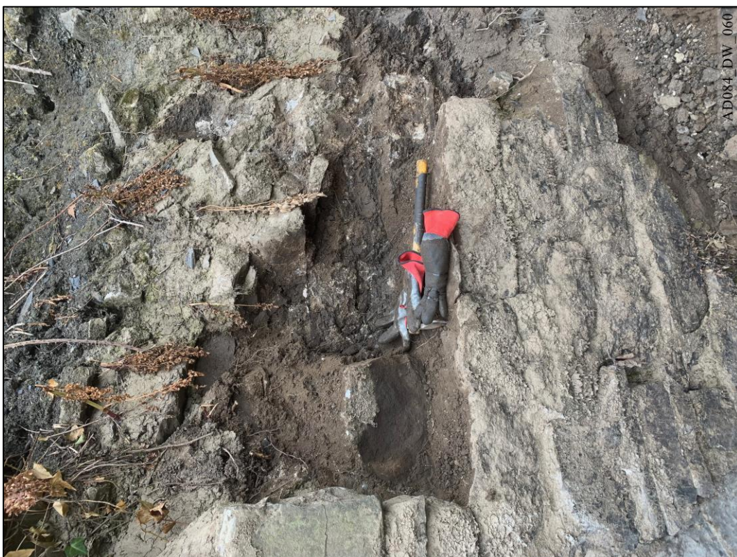
Plate 60 – During works – North elevation, cleaning of masonry to north wing wall.
