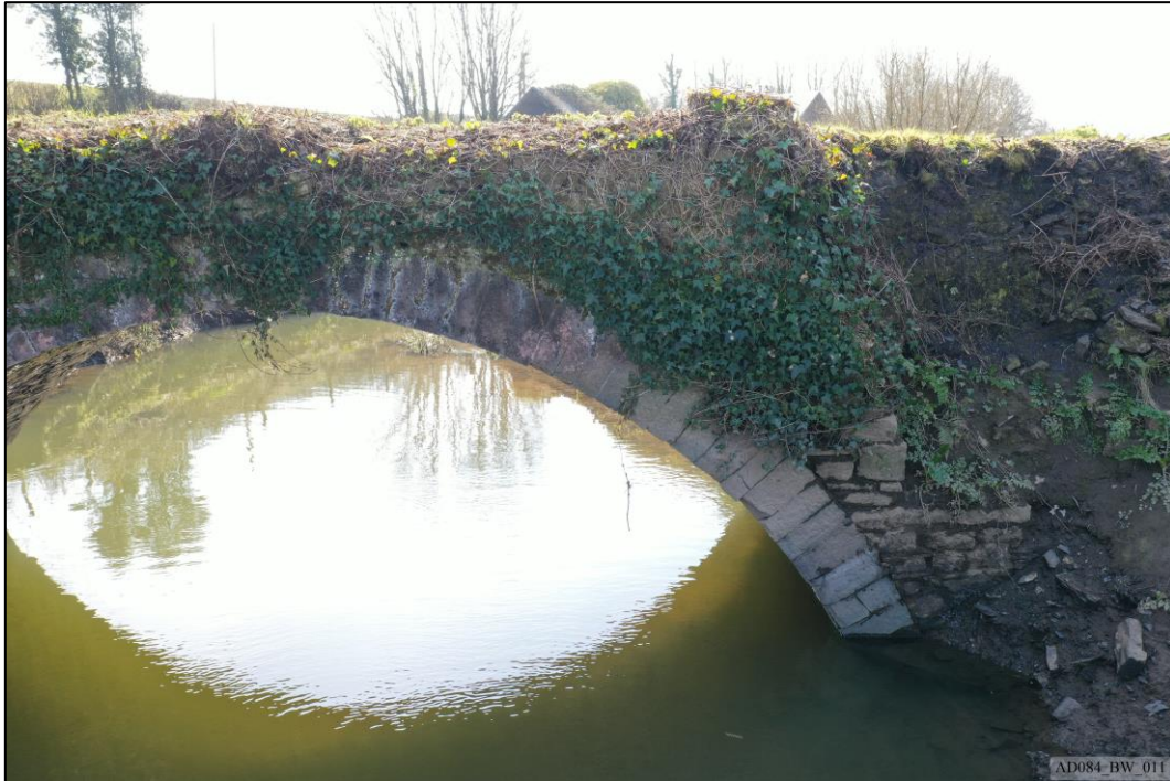
Plate 11 – Pre-works – North elevation, showing arch and west abutment.
