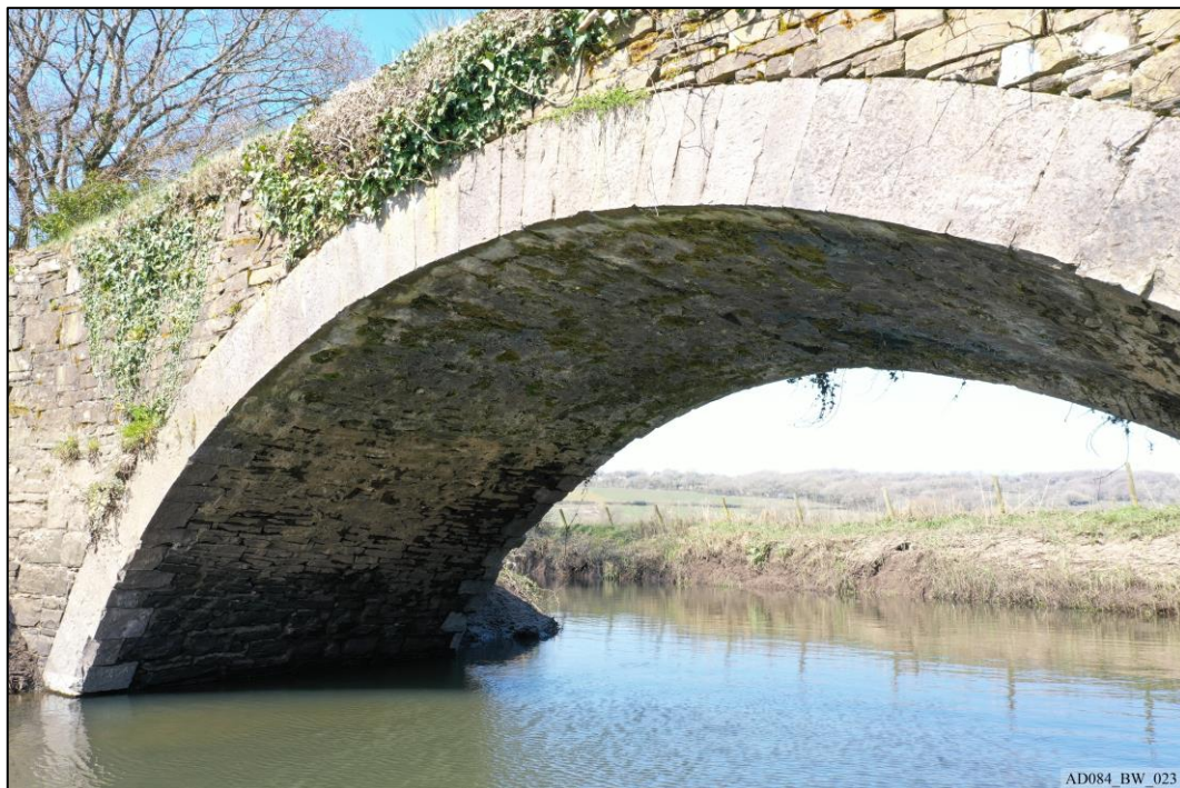
Plate 23 – Pre-works – Arch and barrel vault of west abutment, viewed from south.
