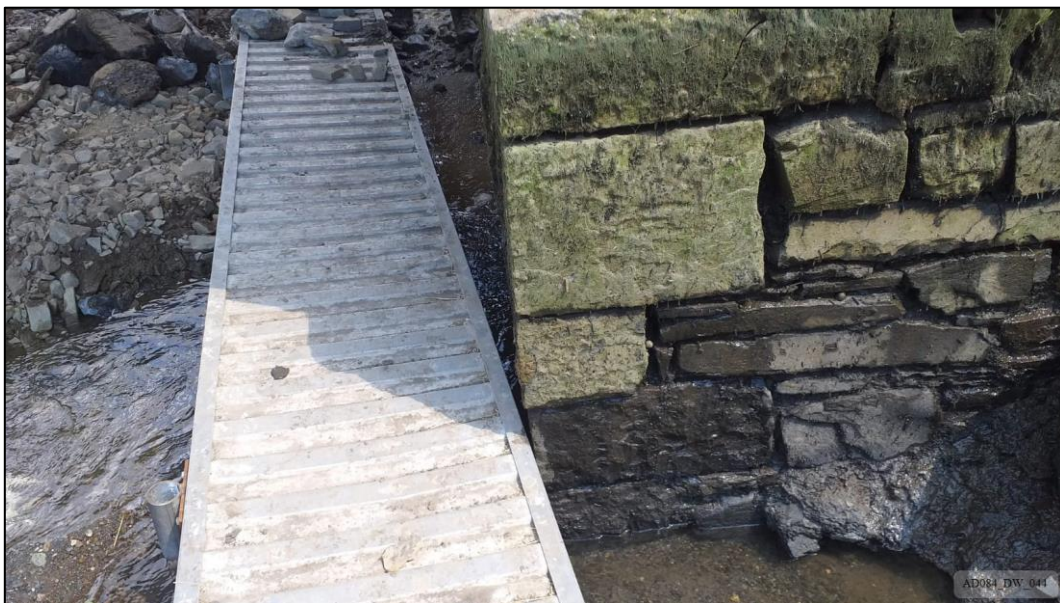
Plate 44 – During works – South elevation, showing quoins to earlier east abutment.
