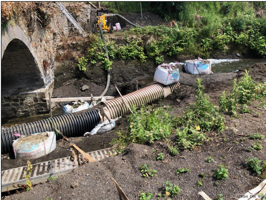
Plate 36 – During works – View east, showing damming of river.
