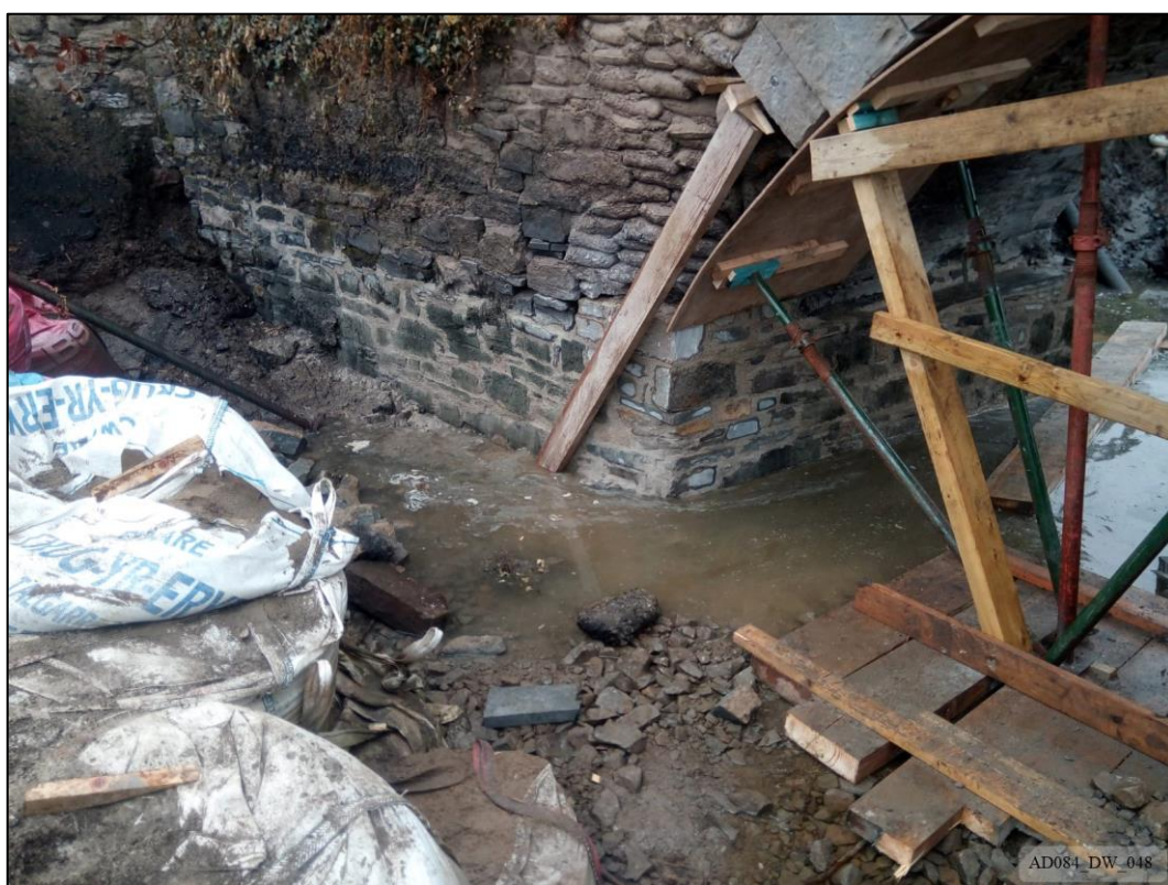
Plate 48 – During works – North elevation, showing repair to lower east abutment.
