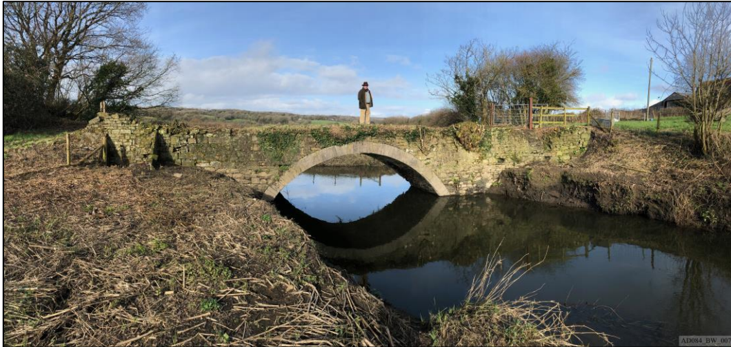
Plate 7 – Pre-works – South elevation, after clearance works.
