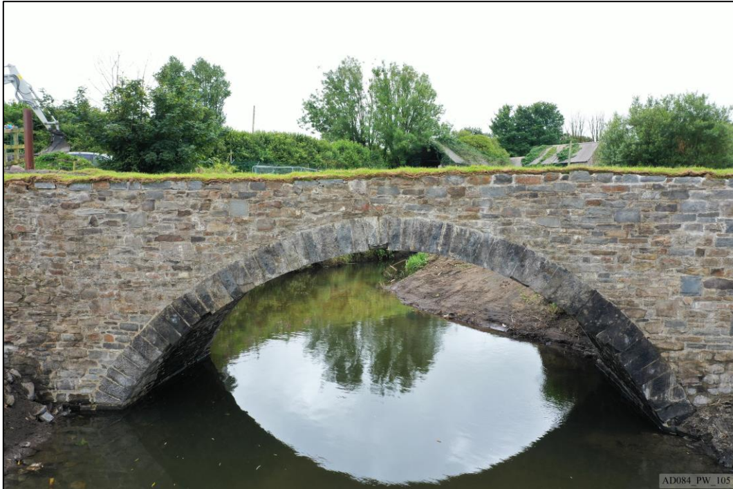
Plate 105 – Post-works – North elevation, showing arch and spandrels.
