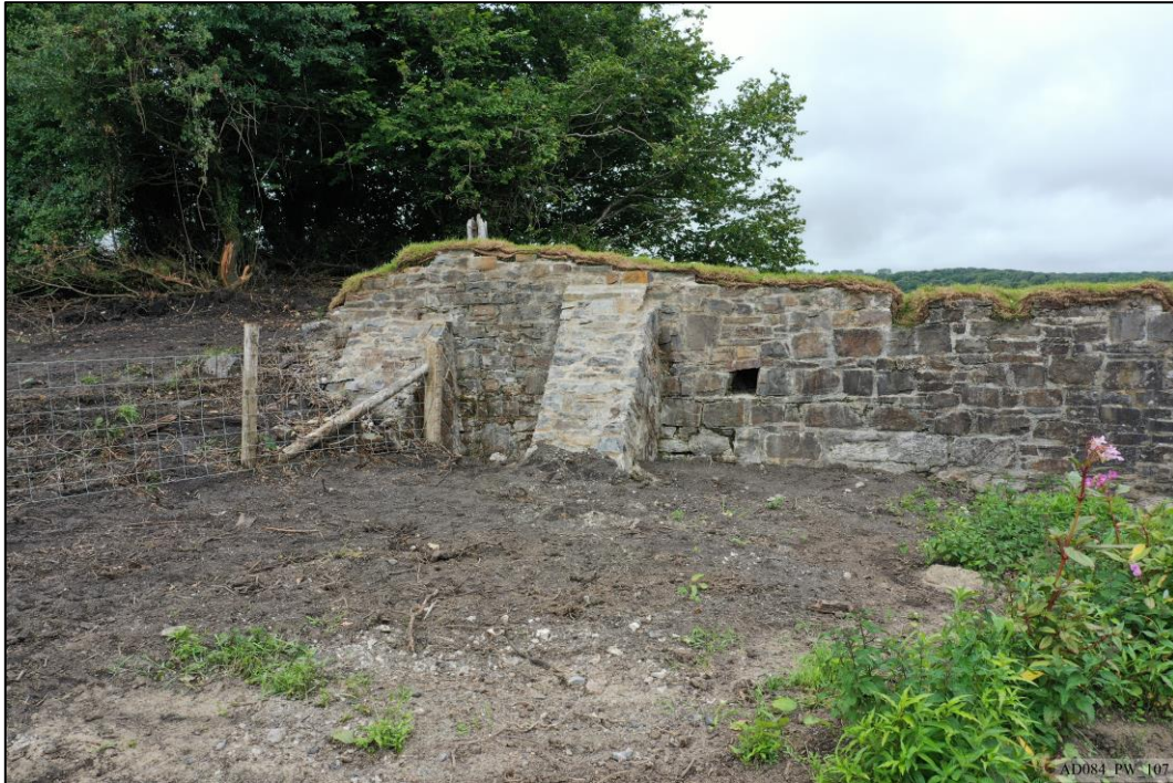
Plate 107 – Post-works – South elevation, west retaining and wing wall.
