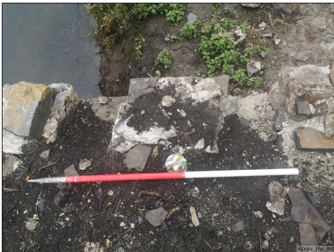
Plate 92 – During works – Wall top to south elevation, showing opening in masonry.
