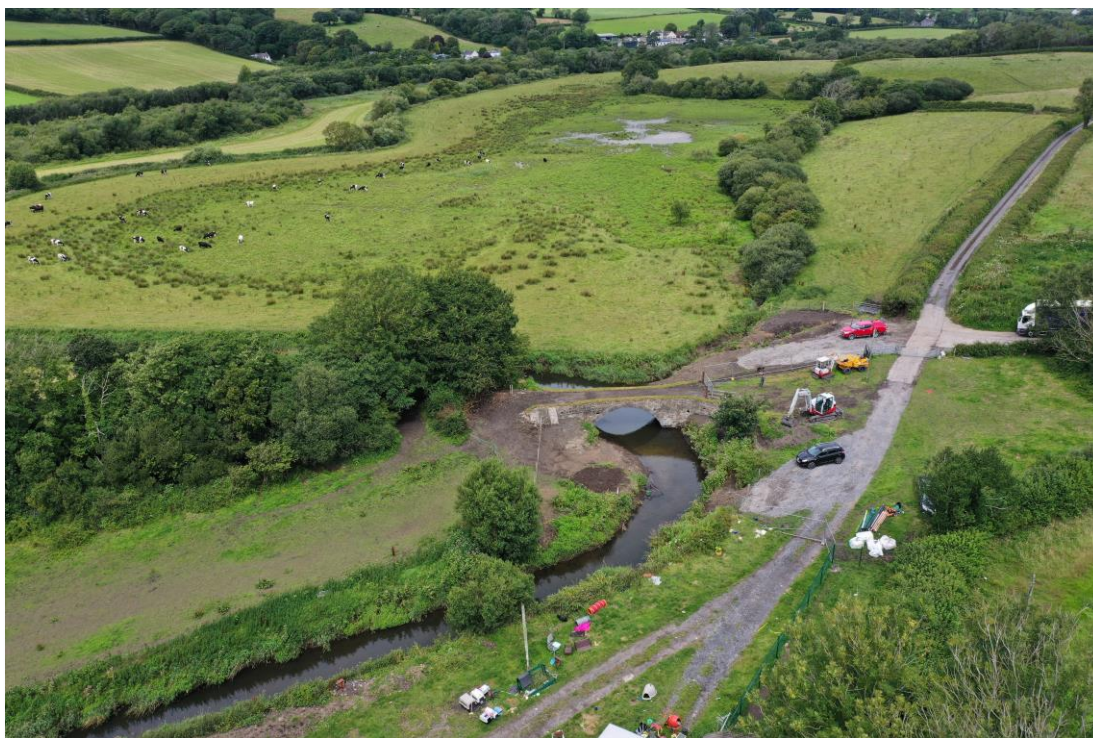
Fig. 1 – Post-work aerial photograph of Pwll-y-Llygod
