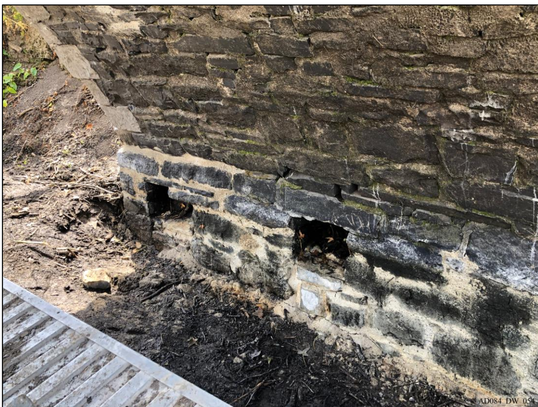
Plate 54 – During works – View west, showing repointing to north abutment.
