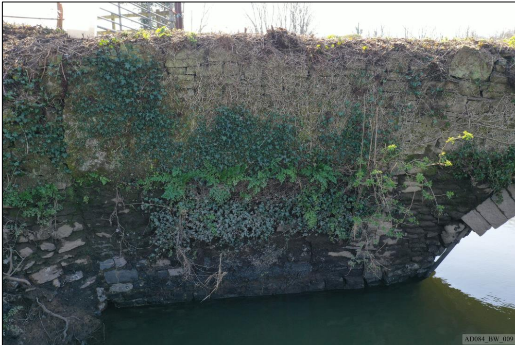
Plate 9 – Pre-works – North elevation, showing east wing wall and abutment..
