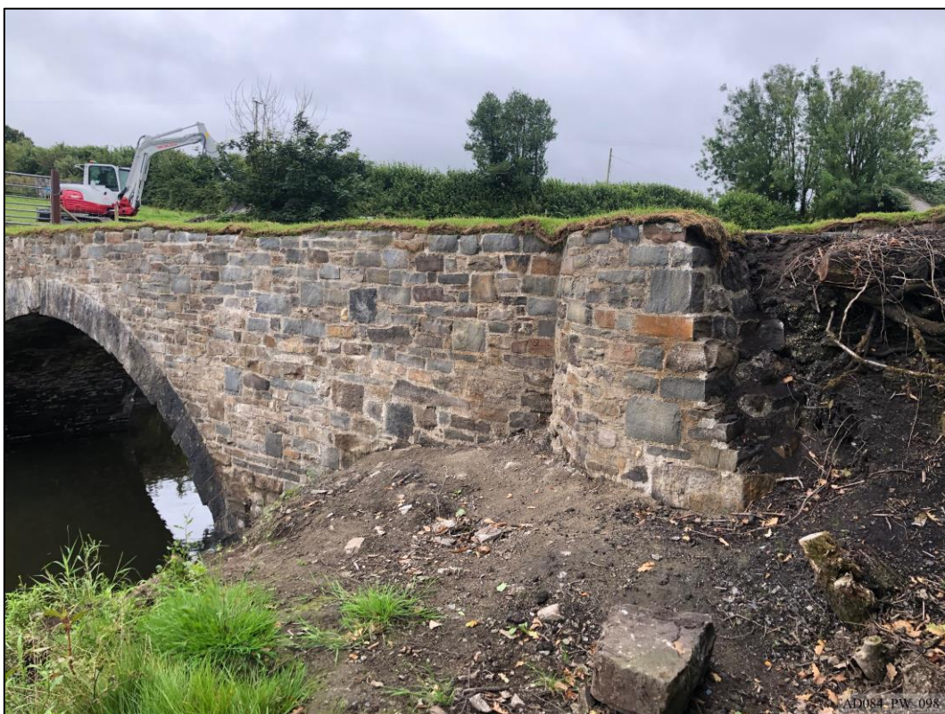
Plate 98 – Post-works – Completed north elevation.
