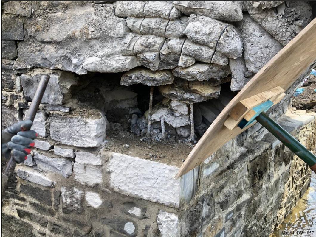
Plate 57 – During works – North elevation, showing removal of east spandrel repair.
