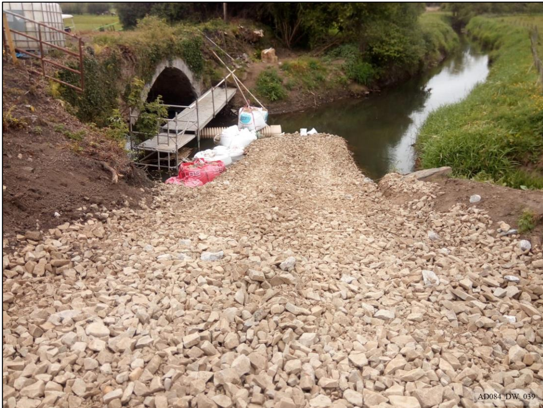
Plate 39 – During works – View west, showing extended trackway and damming of river.
