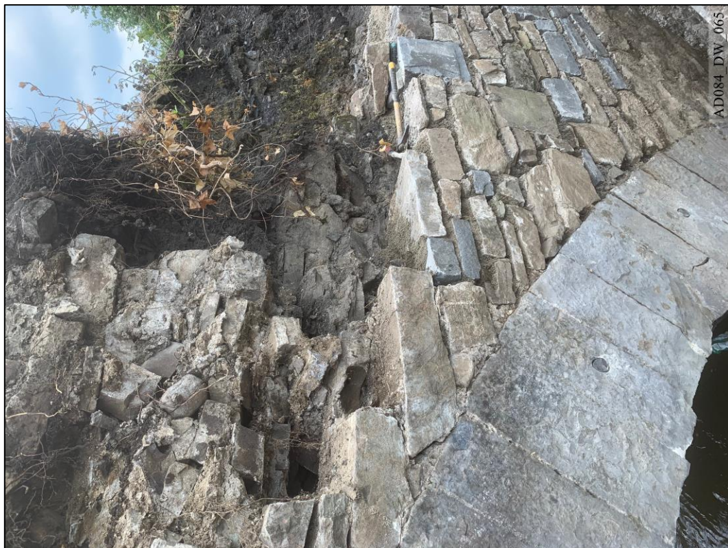
Plate 65 – During works – North elevation, rebuilding of west spandrel and wing wall.
