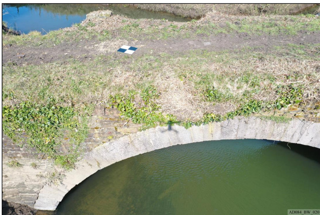
Plate 20 – Pre-works – South elevation, showing arch.
