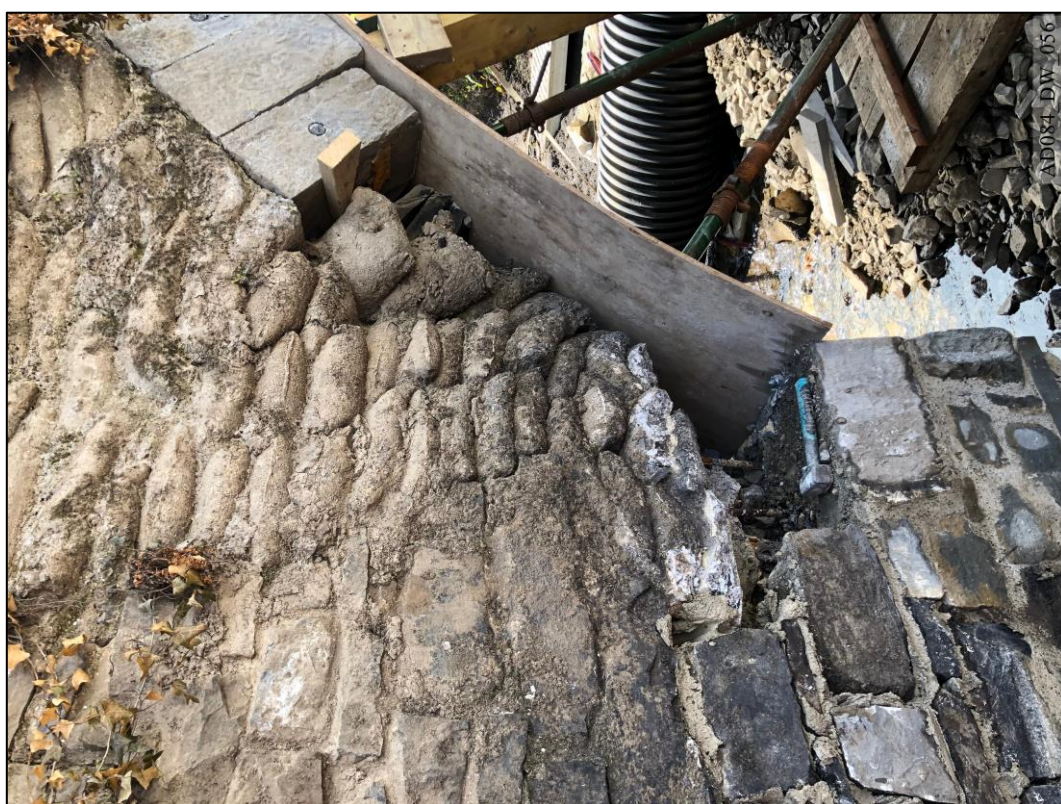
Plate 56 – During works – North elevation, showing east spandrel repair and arch former.
