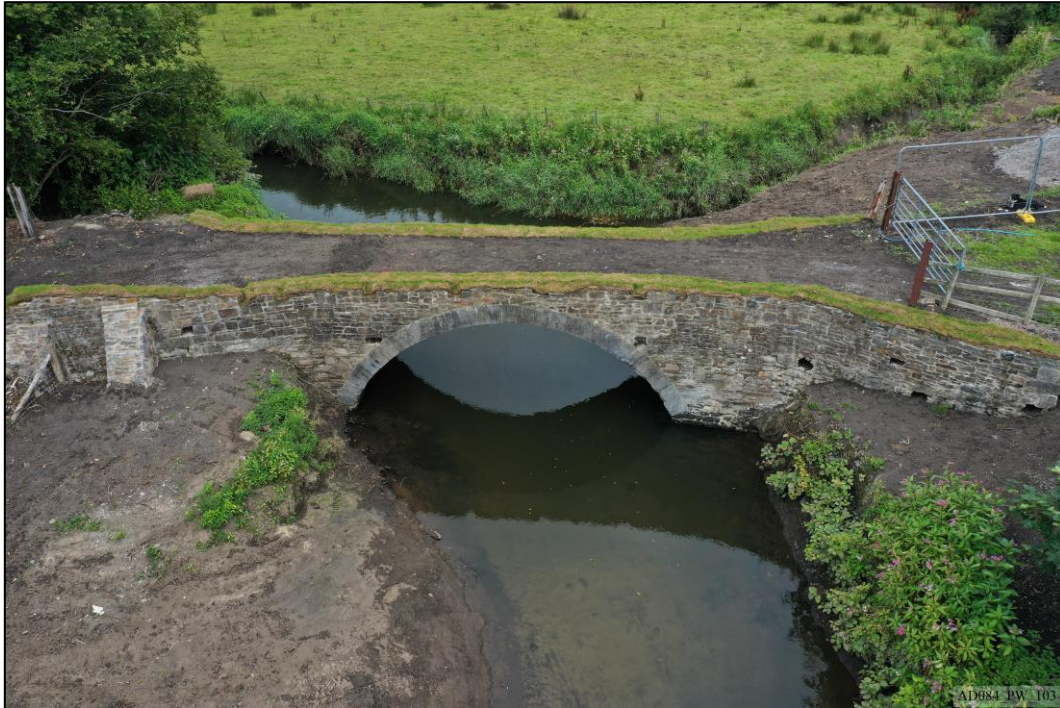
Plate 103 – Post-works – South elevation.
