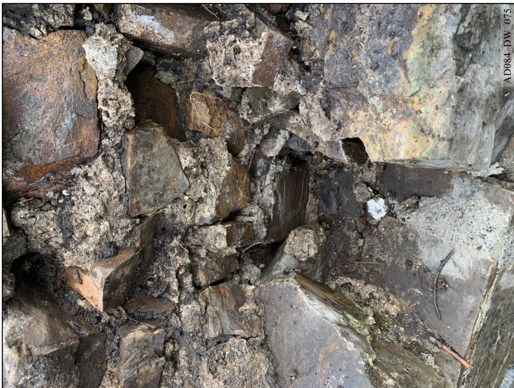
Plate 75 – During works – South elevation, showing core masonry to west wing wall.
