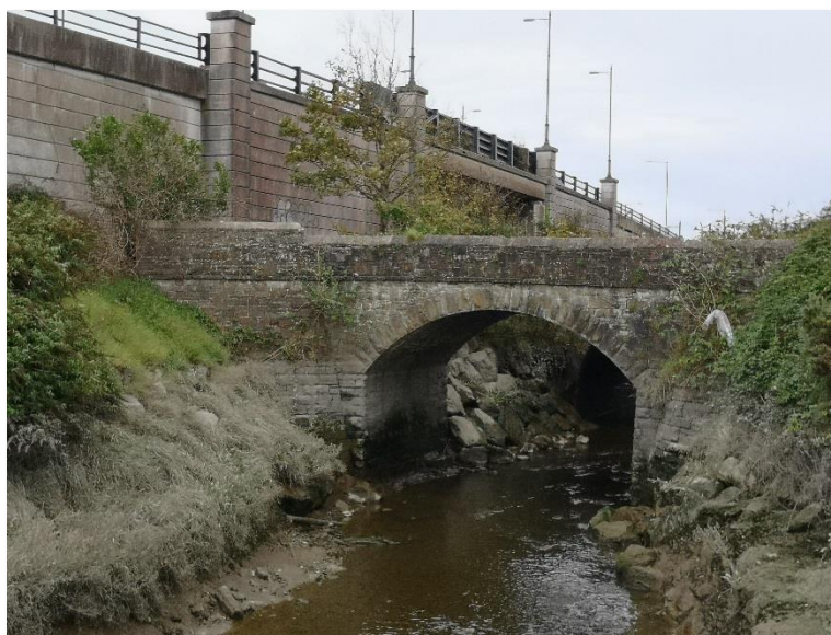
Fig. 7 – New Cut Canal Bridge, Llanelli.
