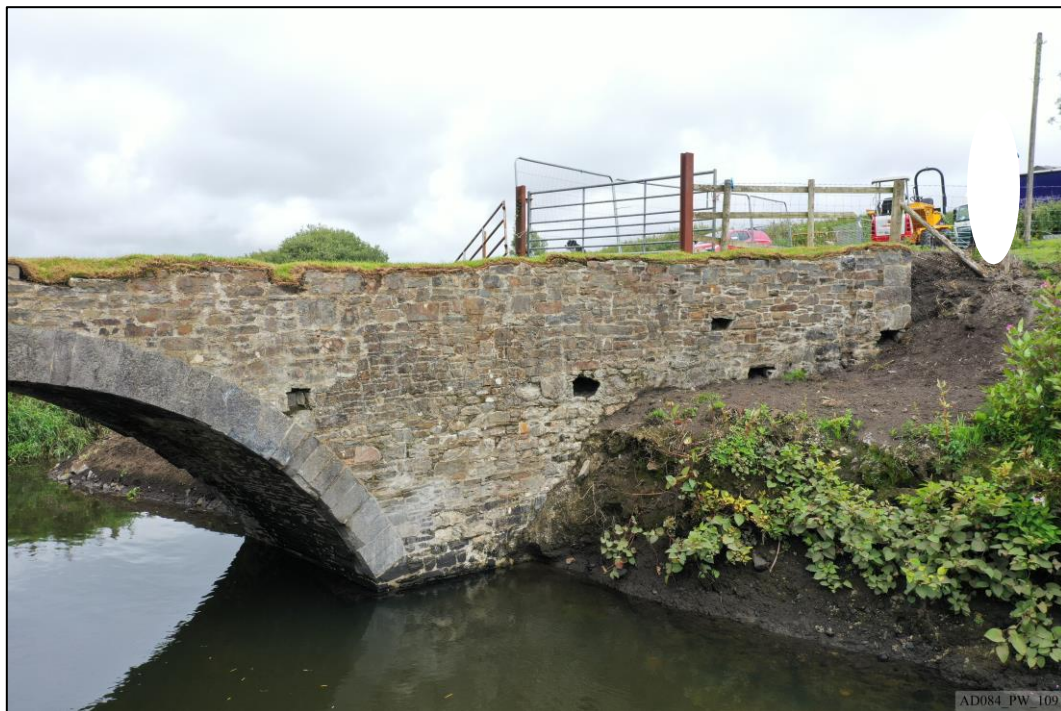
Plate 109 – Post-works – South elevation, arch and west spandrel and wing wall.
