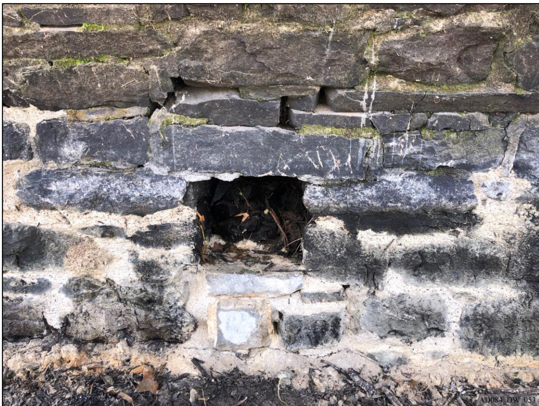
Plate 53 – During works – View west, showing north opening to lower west abutment.
