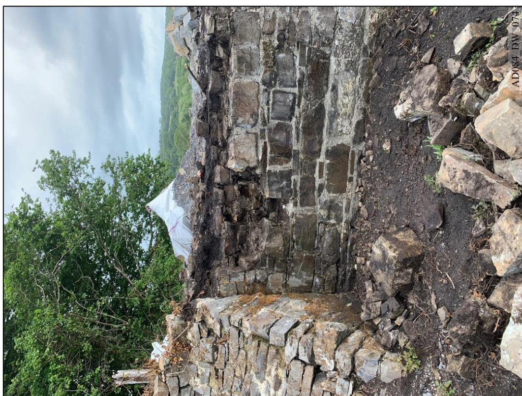
Plate 74 – During works – South elevation, showing dismantling of deteriorated masonry.
