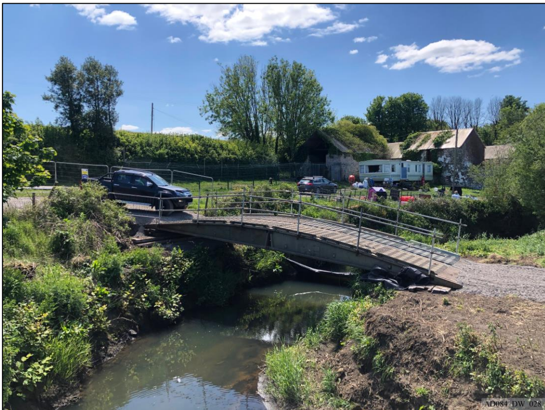
Plate 28 – During works – Installation of temporary bridge to south.
