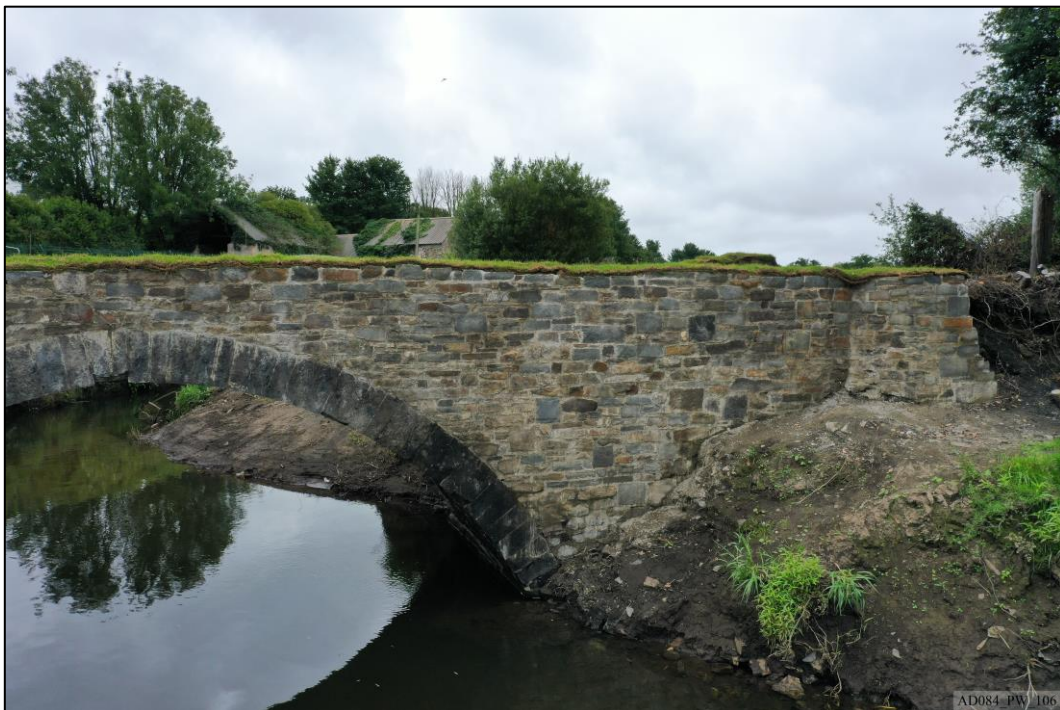
Plate 106 – Post-works – North elevation, showing west spandrel and wing wall.
