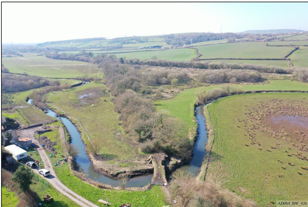
Plate 26 – Pre-works – View west, showing Carway Siding and Kymer's Canal, after clearance works.
