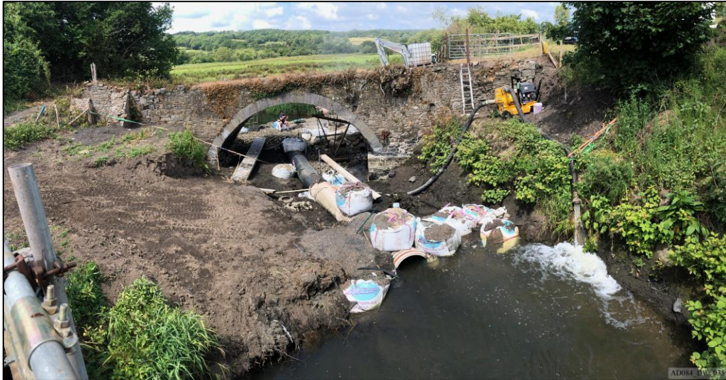
Plate 35 – During works – View towards north, showing damming of river.
