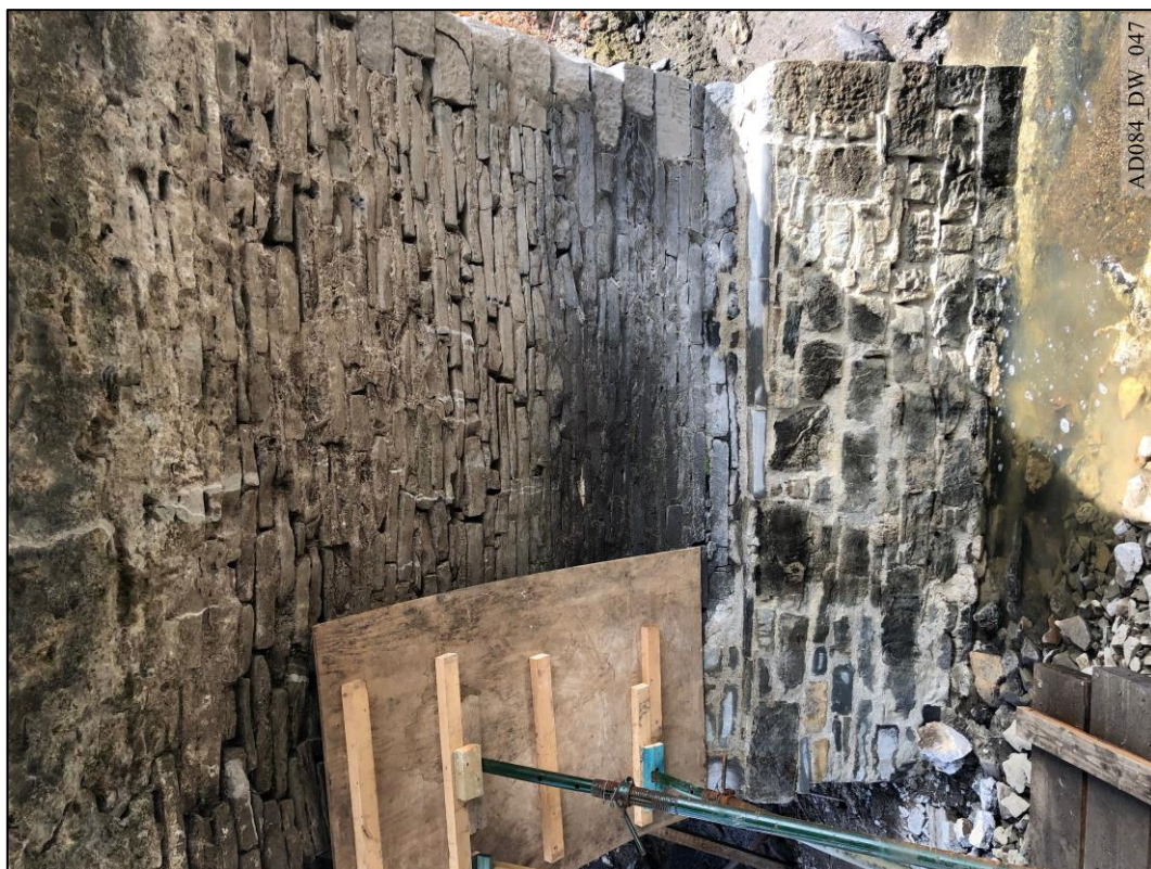
Plate 47 – During works – View east, showing repairs to east abutment.
