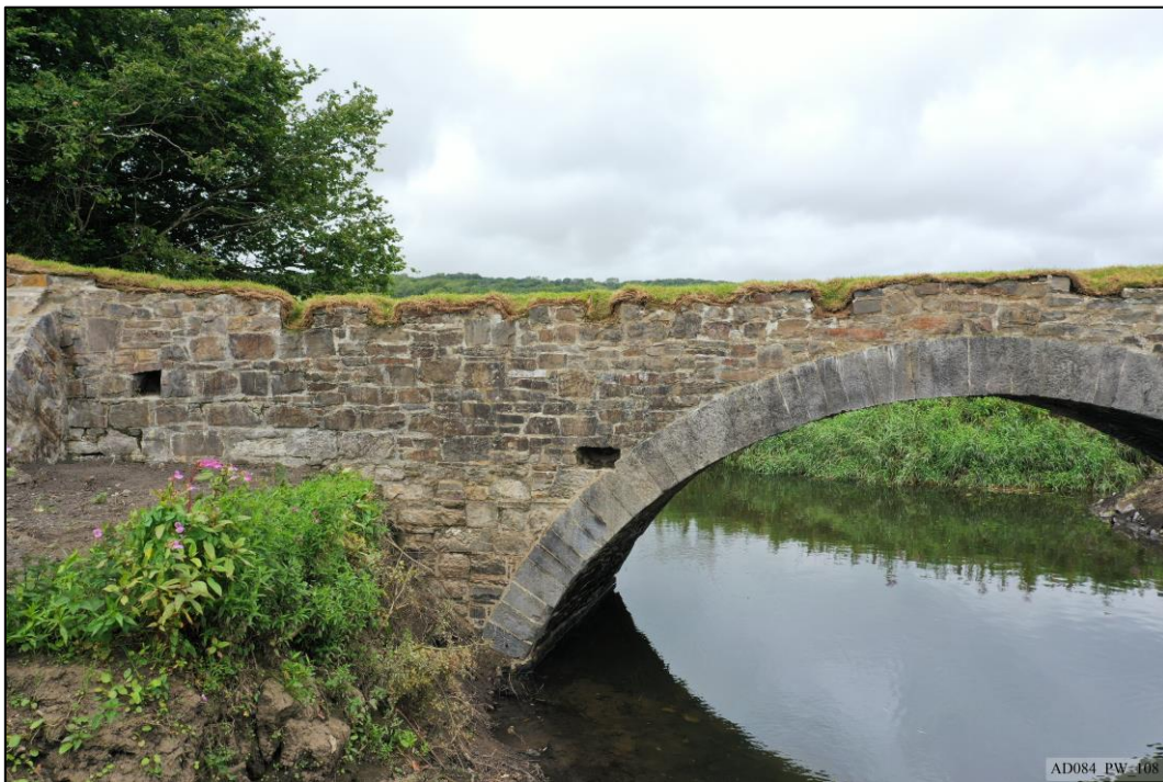
Plate 108 – Post-works – South elevation, west spandrel and arch.
