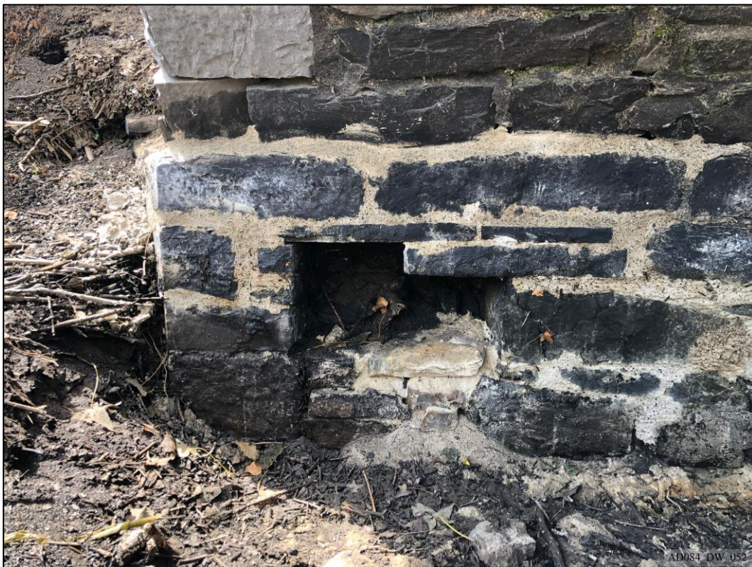
Plate 52 – During works – View west, showing south opening to lower west abutment.
