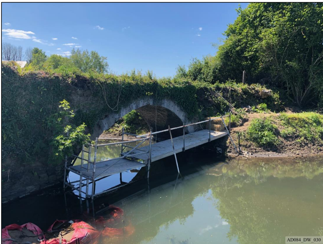
Plate 30 – During works – North elevation, with scaffold and partial damming.
