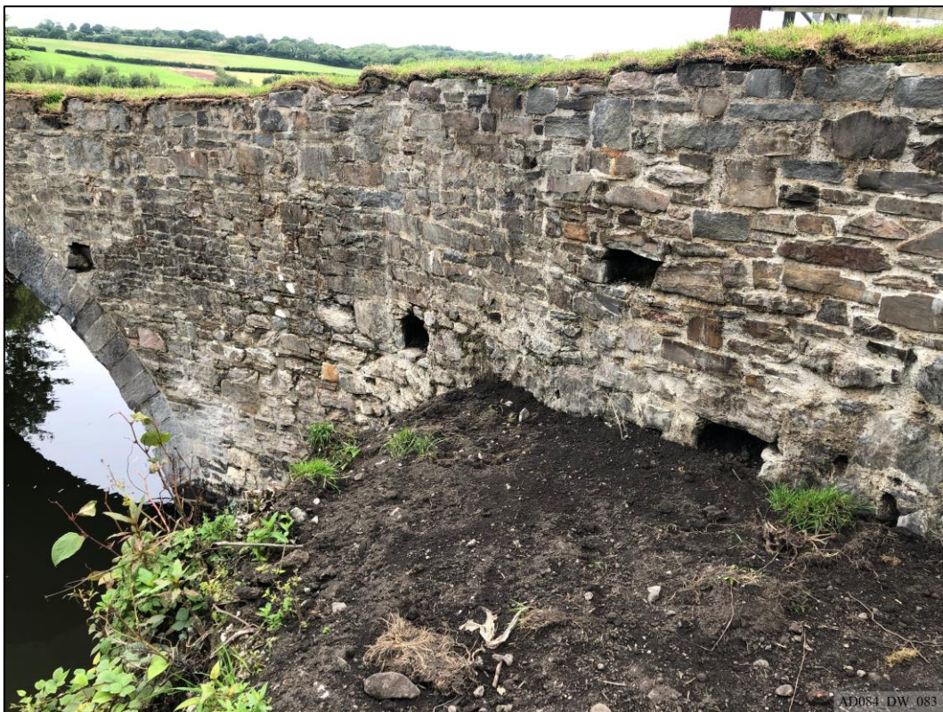
Plate 83 – During works – South elevation, showing completed rebuild of east wing wall.
