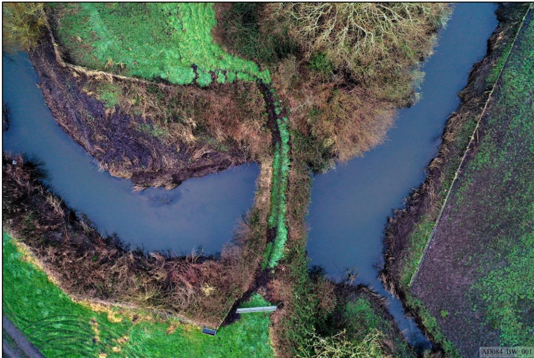
Plate 1 – Pre-works – Nadir view before clearance works.
