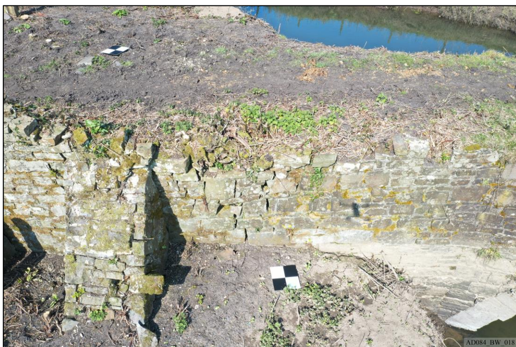
Plate 18 – Pre-works – South elevation, showing west wing wall and spandrel.
