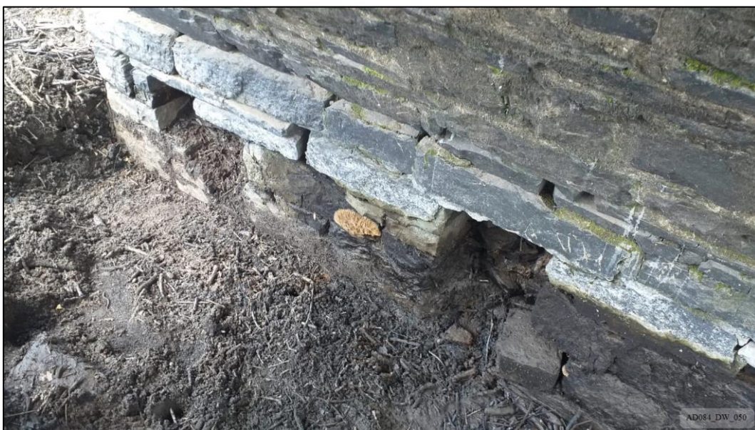
Plate 50 – During works – View east, showing lower abutment.
