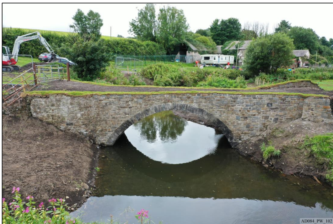
Plate 102 – Post-works – North elevation.
