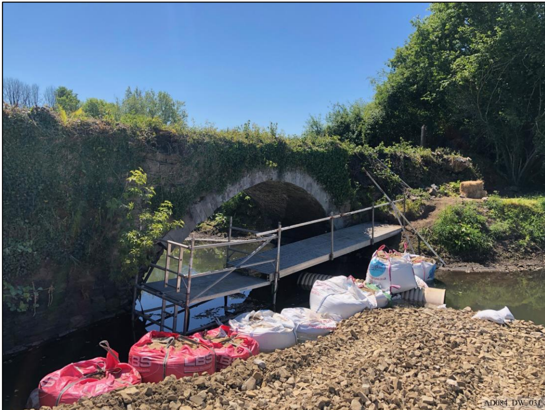
Plate 31 – During works – North elevation, showing scaffold and river damming.
