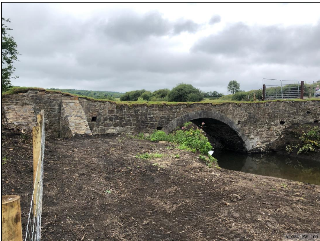
Plate 100 – Post-works – Completed south elevation.
