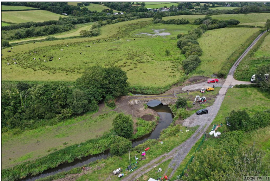
Plate 111 – Post-works – View toward north.
