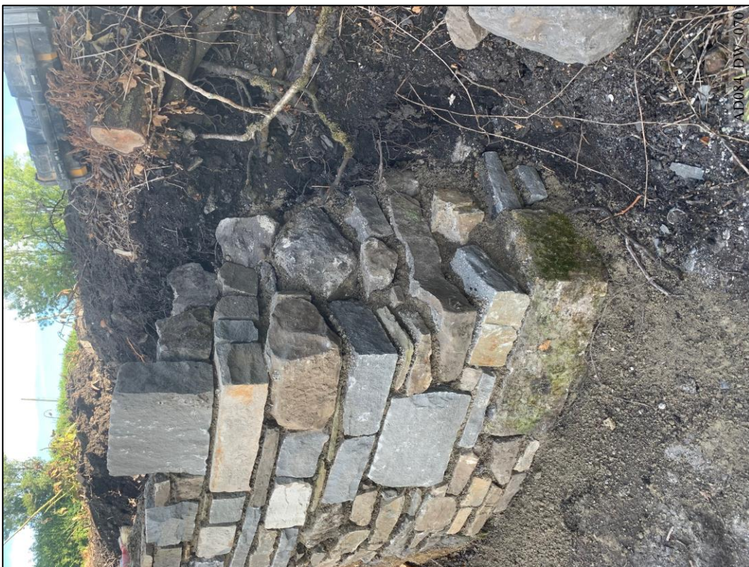
Plate 70 – During works – North elevation, showing end and core of retaining wall.
