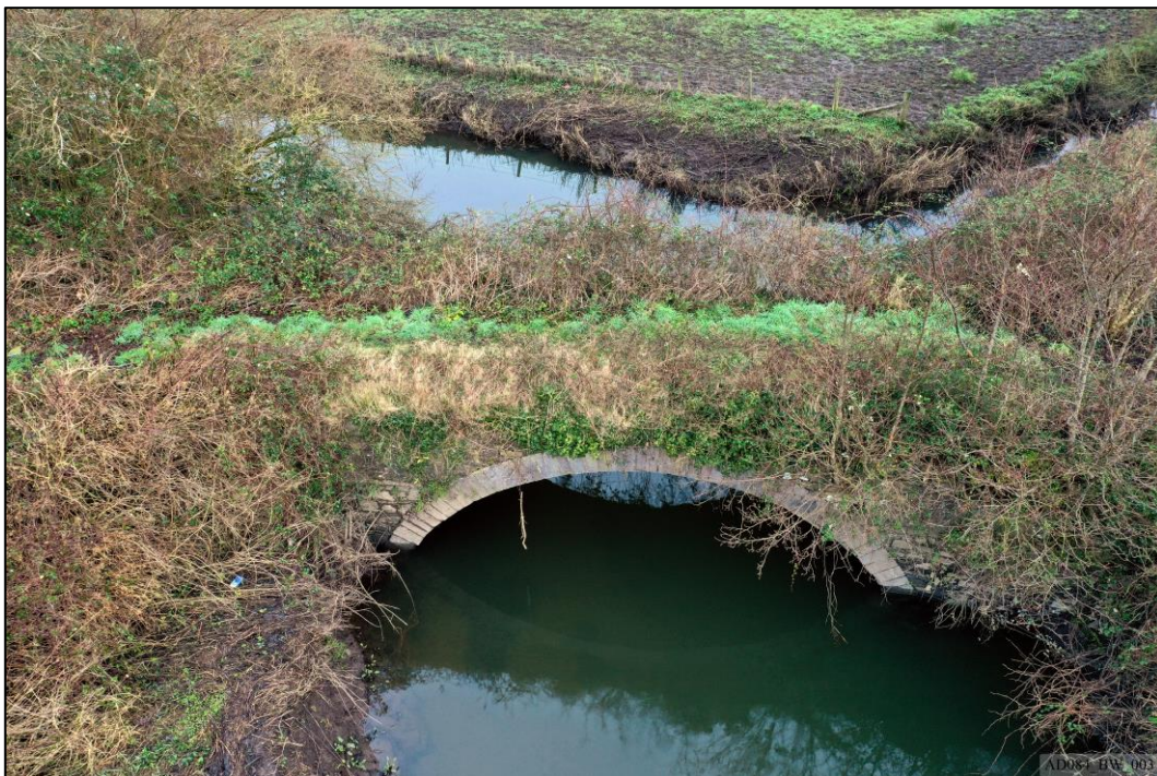
Plate 3 – Pre-works – South elevation, before clearance works.
