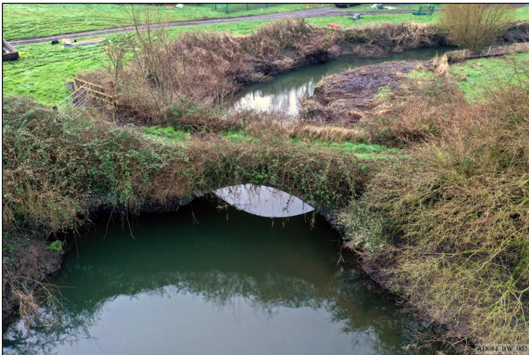
Plate 2 – Pre-works – North elevation, before clearance works.
