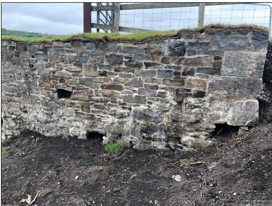
Plate 84 – During works – South elevation, showing completed rebuild of east wing wall.
