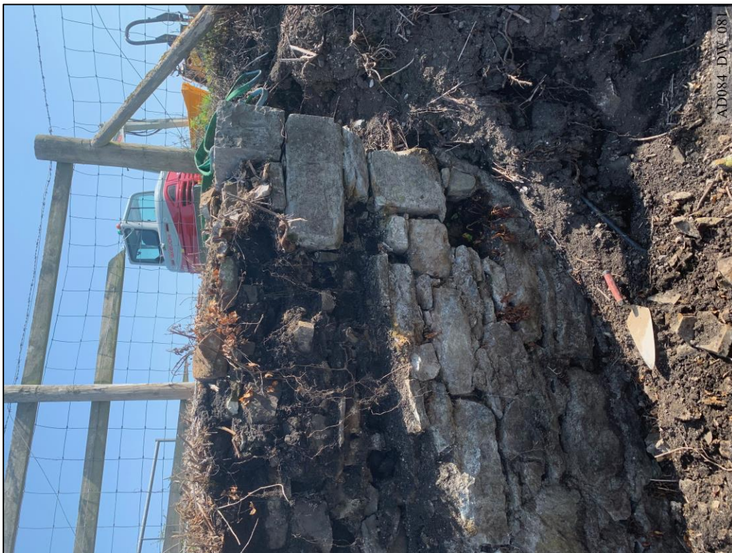
Plate 81 – During works – South elevation, showing damage to east wing wall.
