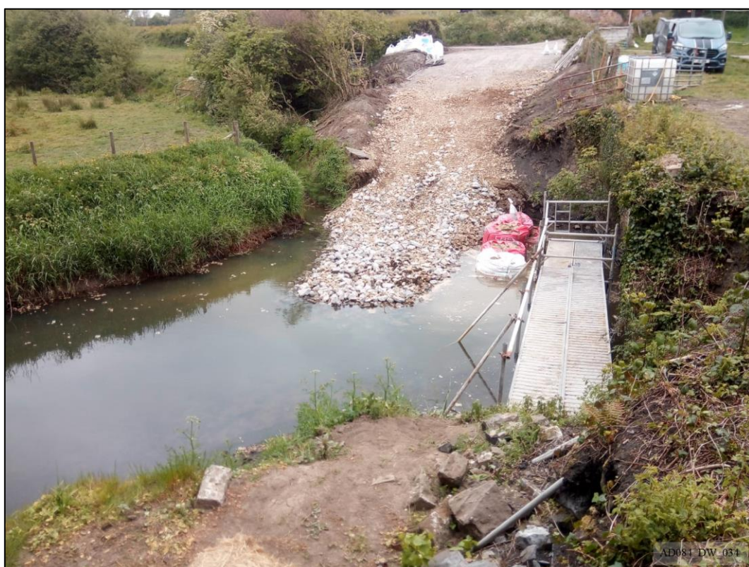
Plate 34 – During works – View east, showing trackway to river.
