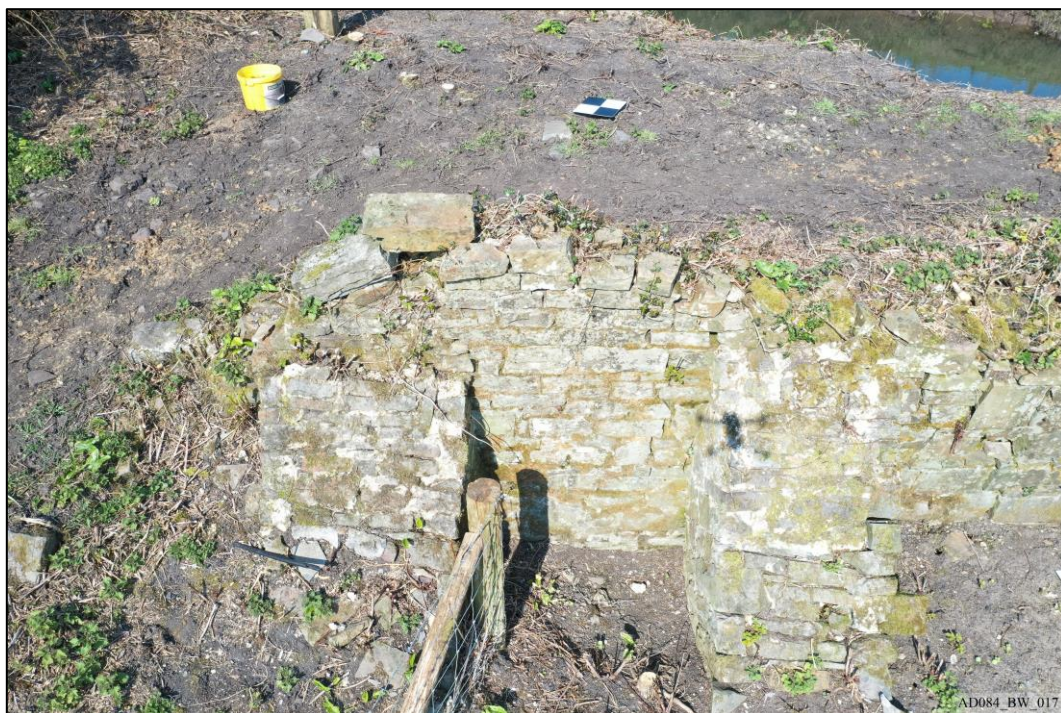
Plate 17 – Pre-works – South elevation, buttresses to west wing wall.
