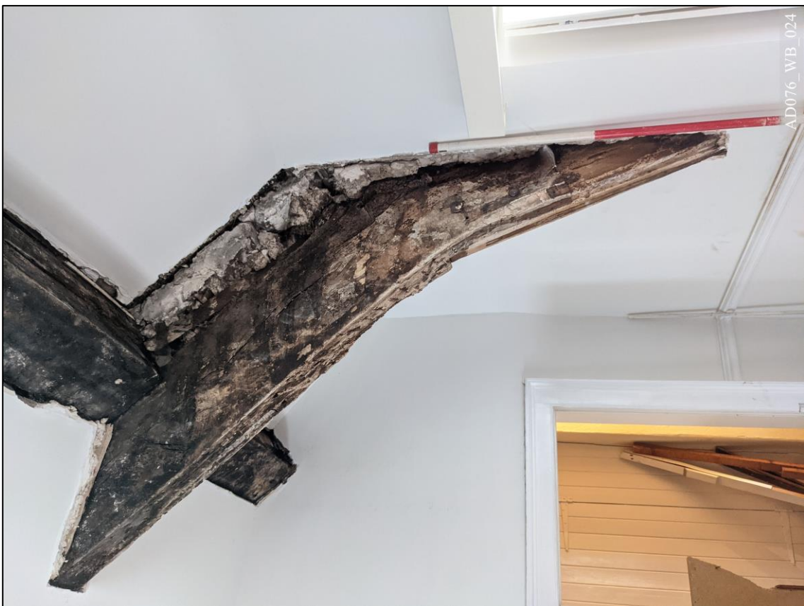
Plate 24 – View east, showing raised cruck blade (south) [FF.10].
