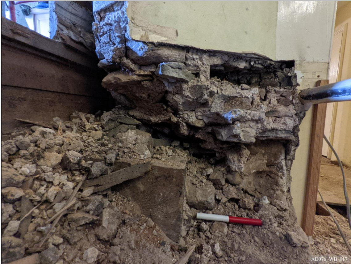
Plate 17 – View west, showing core of 17 th century wall.
