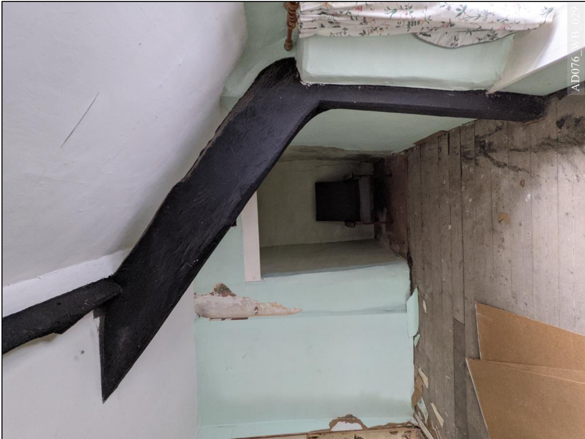
Plate 29 – Truss to western range [FF.15].
