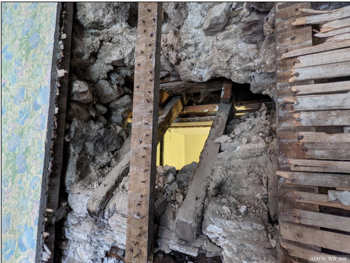
Plate 8 – View north, showing exposed common rafters [FF.01].
