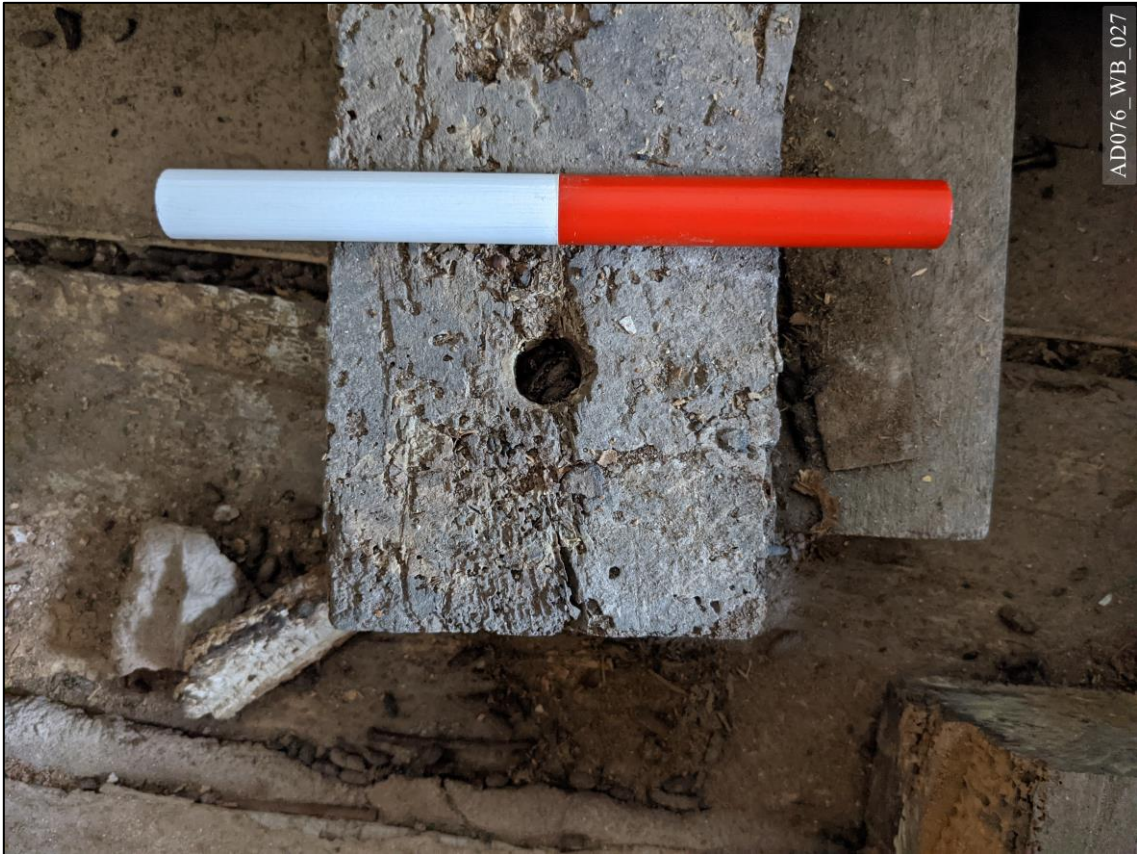
Plate 27 – Peg hold in lodged joist, first floor [FF.10].
