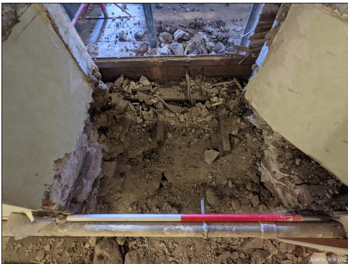
Plate 12 – View south, showing reduction of sill height [FF.03].
