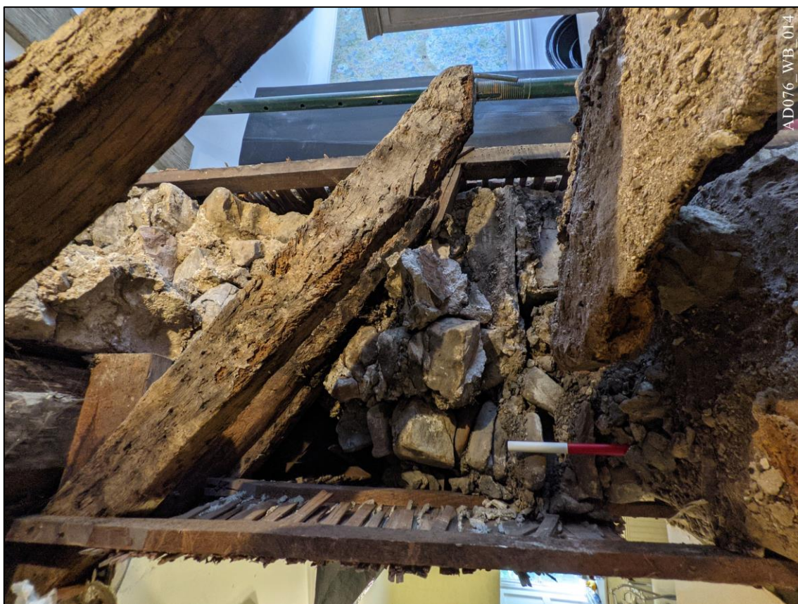
Plate 14 – View east, showing change in masonry and common rafters.
