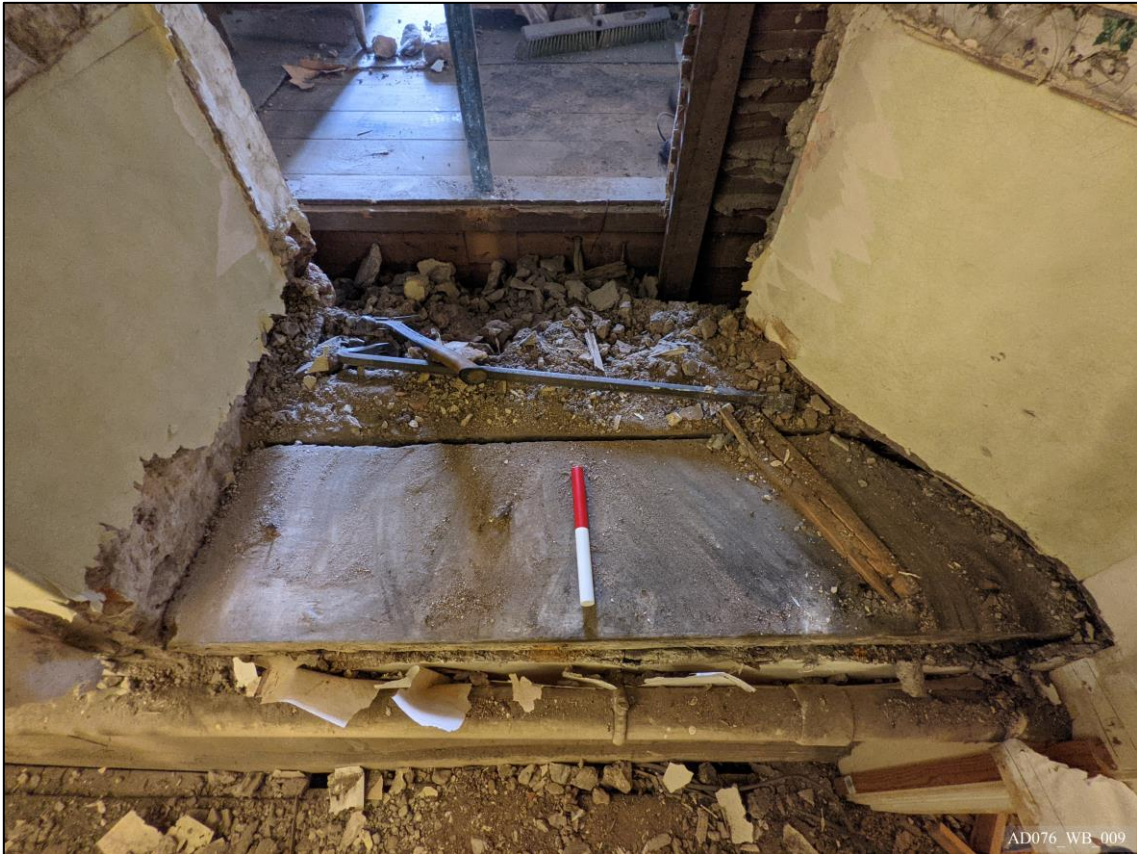
Plate 9 – View south, showing oak window sills [FF.03].
