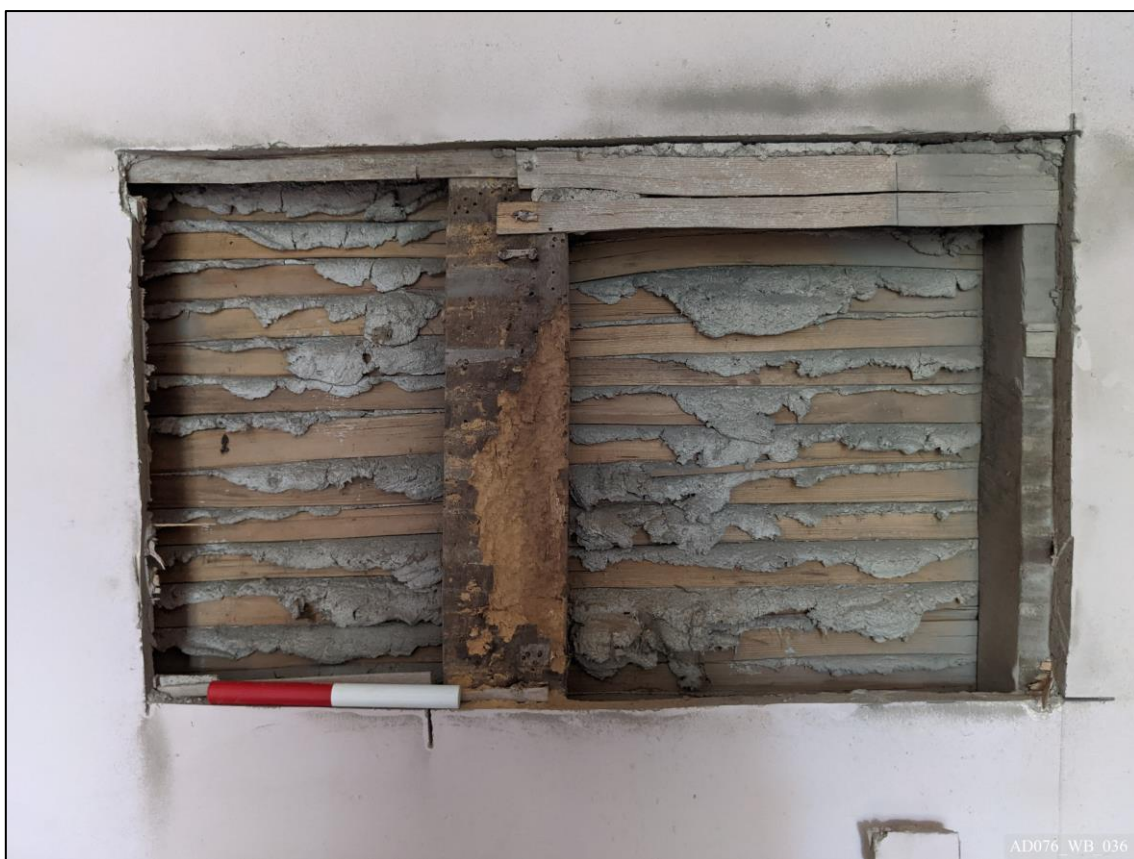
Plate 36 – View east, showing partition wall between [GF.15] and [GF.16].
