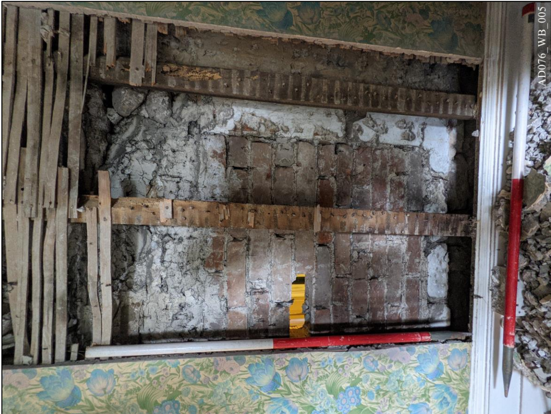
Plate 5 – View north, showing brick window blocking [FF.01].
