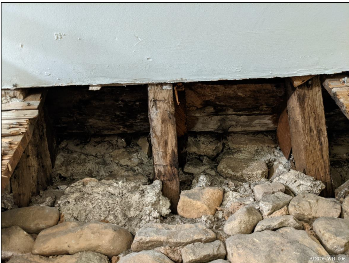
Plate 6 – View south, showing change in masonry, common rafters, and valley-board [FF.03].
