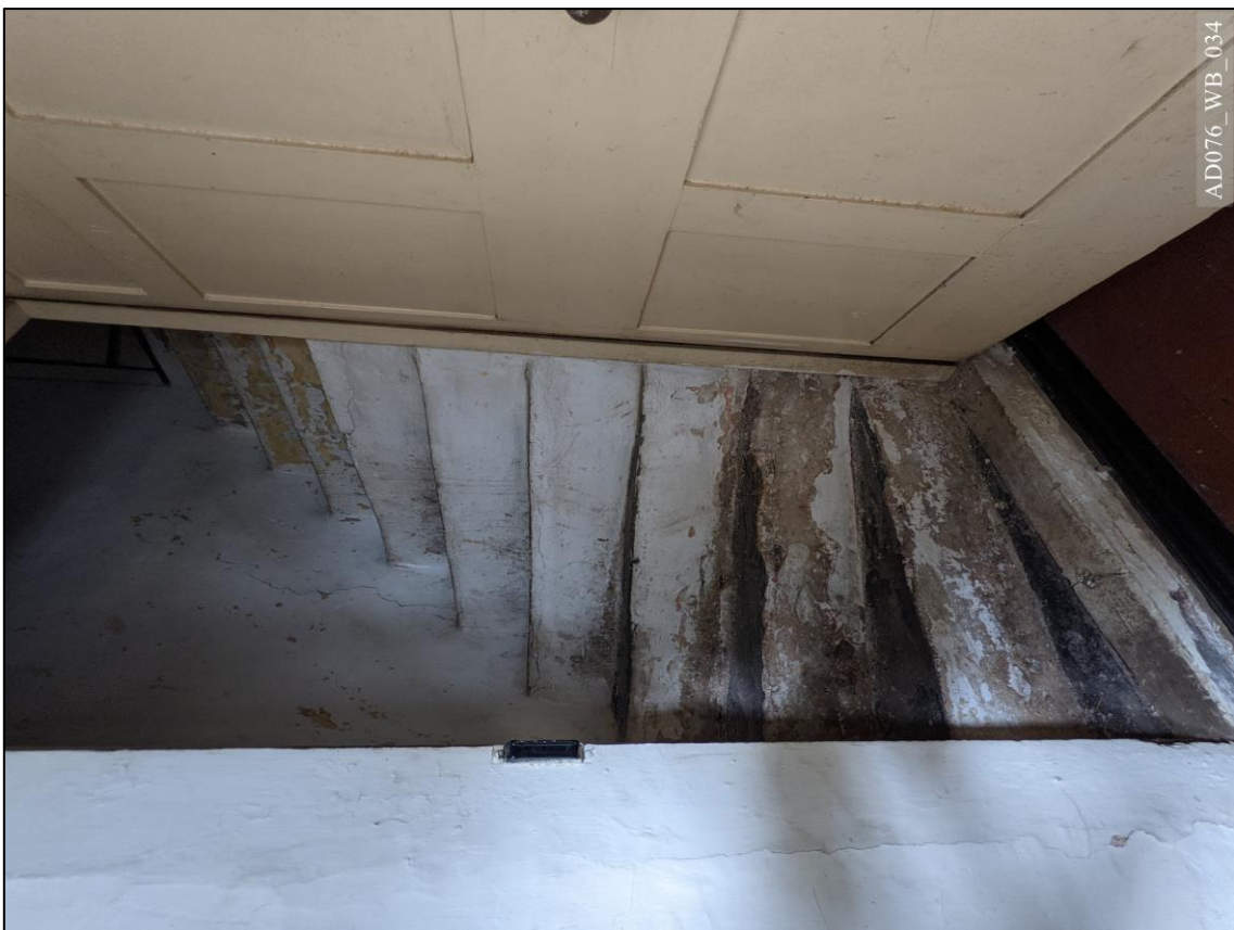
Plate 34 – View west, showing chimney stair from [GF.18] to [FF.16].
