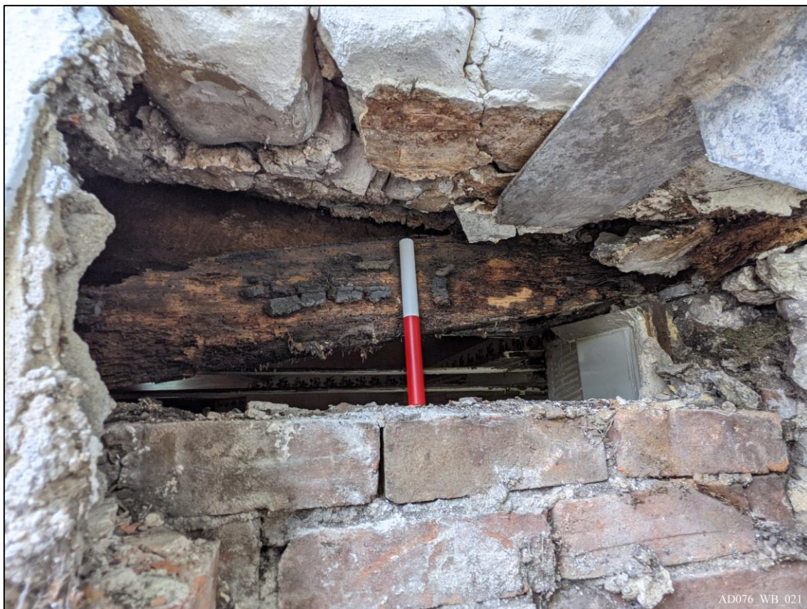
Plate 21 – View west, showing oak lintels to kitchen doorway [GF.19].
