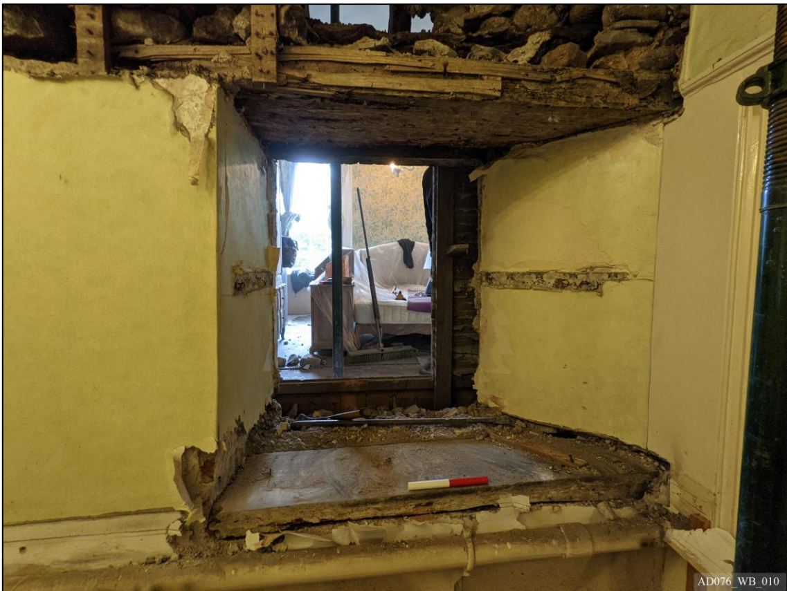
Plate 10 – View south, showing unblocked window [FF.03].
