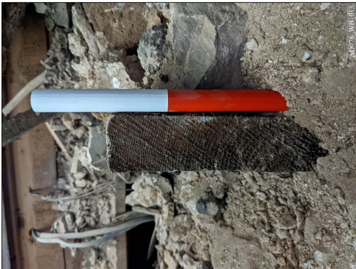
Plate 13 – View south, showing end of pine joist of the Georgian wing [FE.01].
