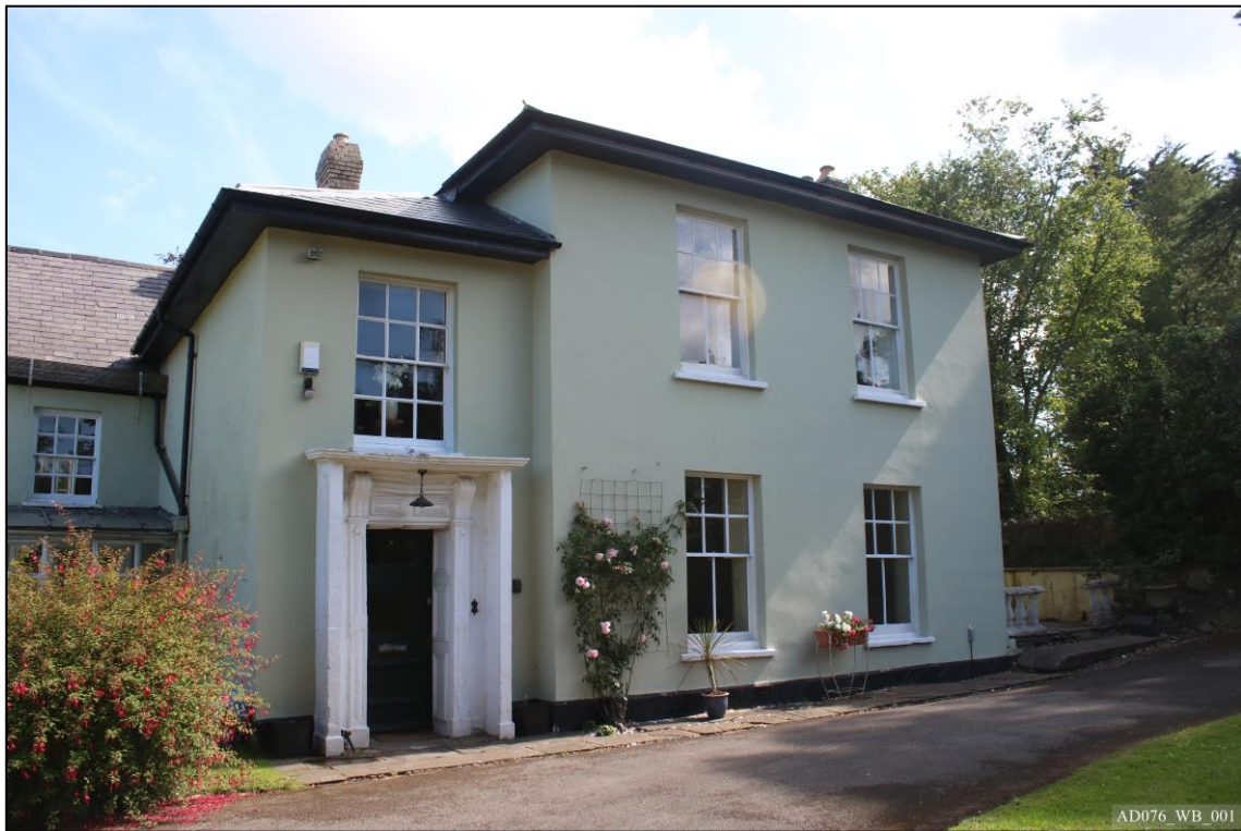
Plate 1 – Georgian wing – South Elevation
