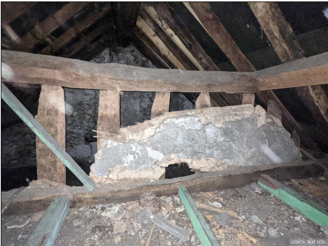
Plate 26 – View east, showing surviving 16 th century partition in left.
