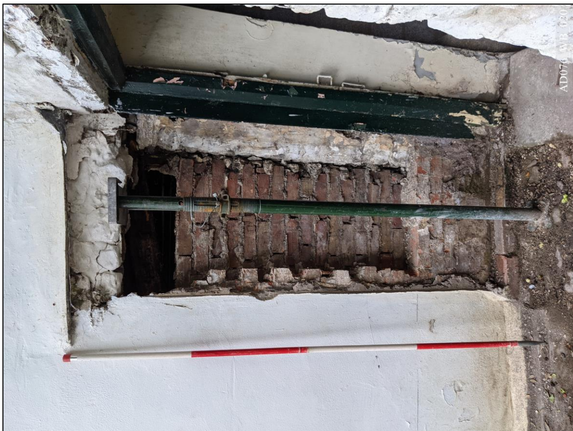
Plate 20 – View west, showing blocked kitchen doorway [GF.19].
