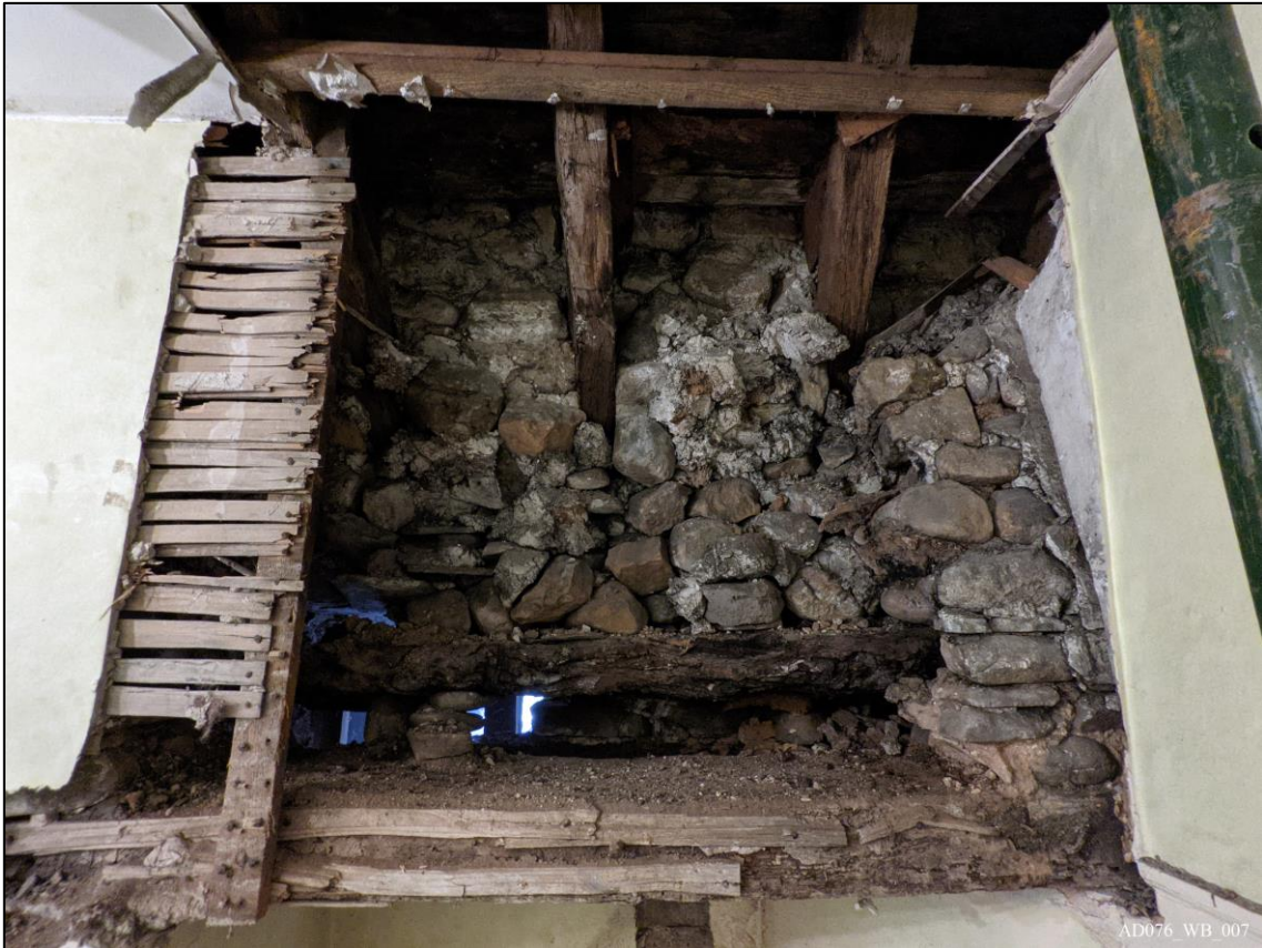
Plate 7 – View south, showing change in masonry, common rafters, and valley-board [FF.03].
