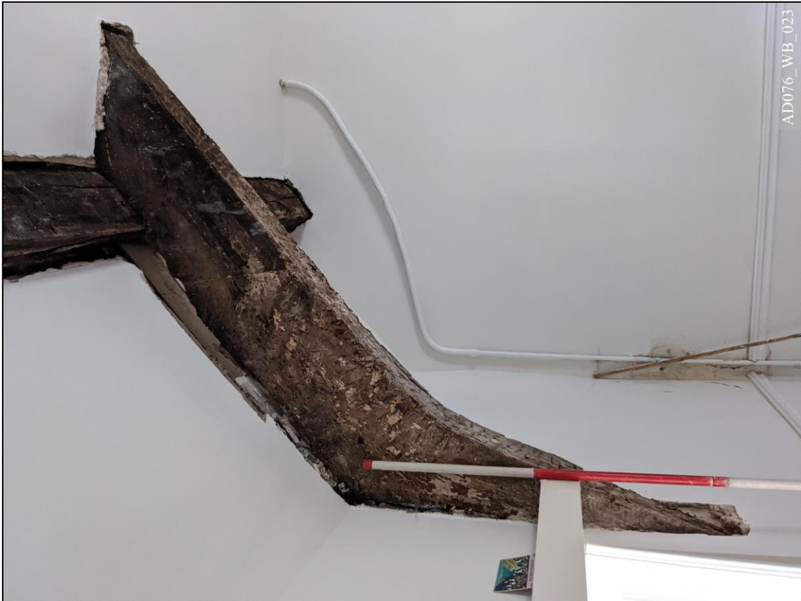
Plate 23 – View east, showing raised cruck blade (north) [FF.10].
