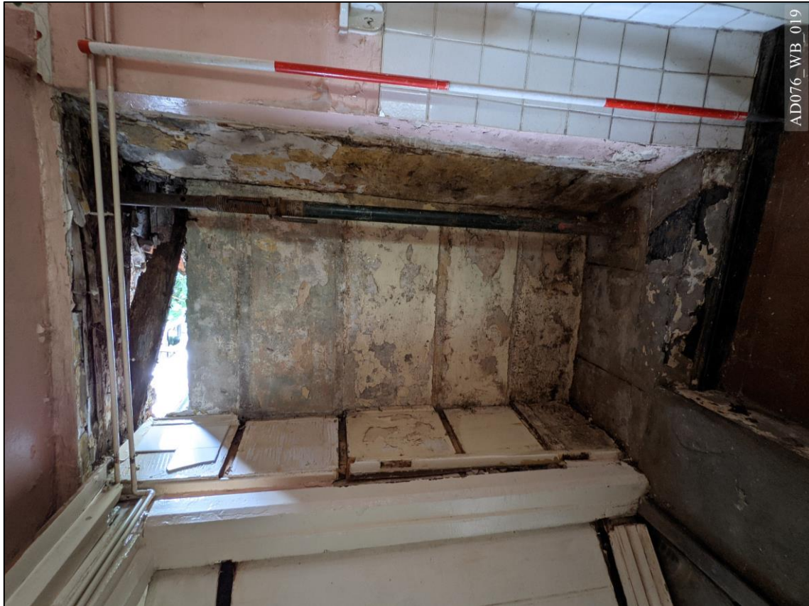
Plate 19 – View east, showing blocked kitchen doorway [GF.19].
