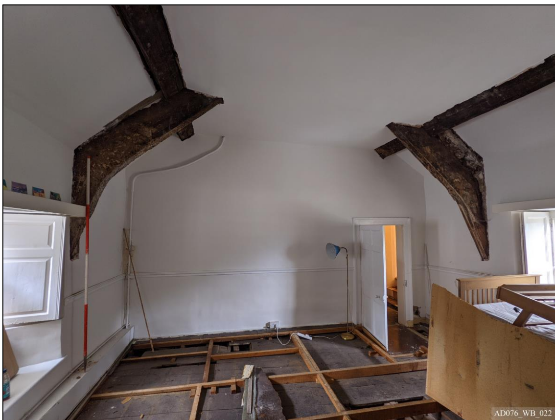
Plate 22 – View east, showing raised crucks at first floor [FF.10].
