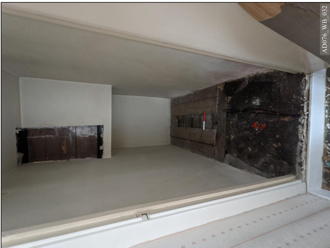
Plate 32 – First floor latrine, now cupboard to [FF.11].
