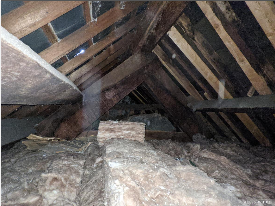
Plate 25 – View east, showing apex and collar of cruck in left.
