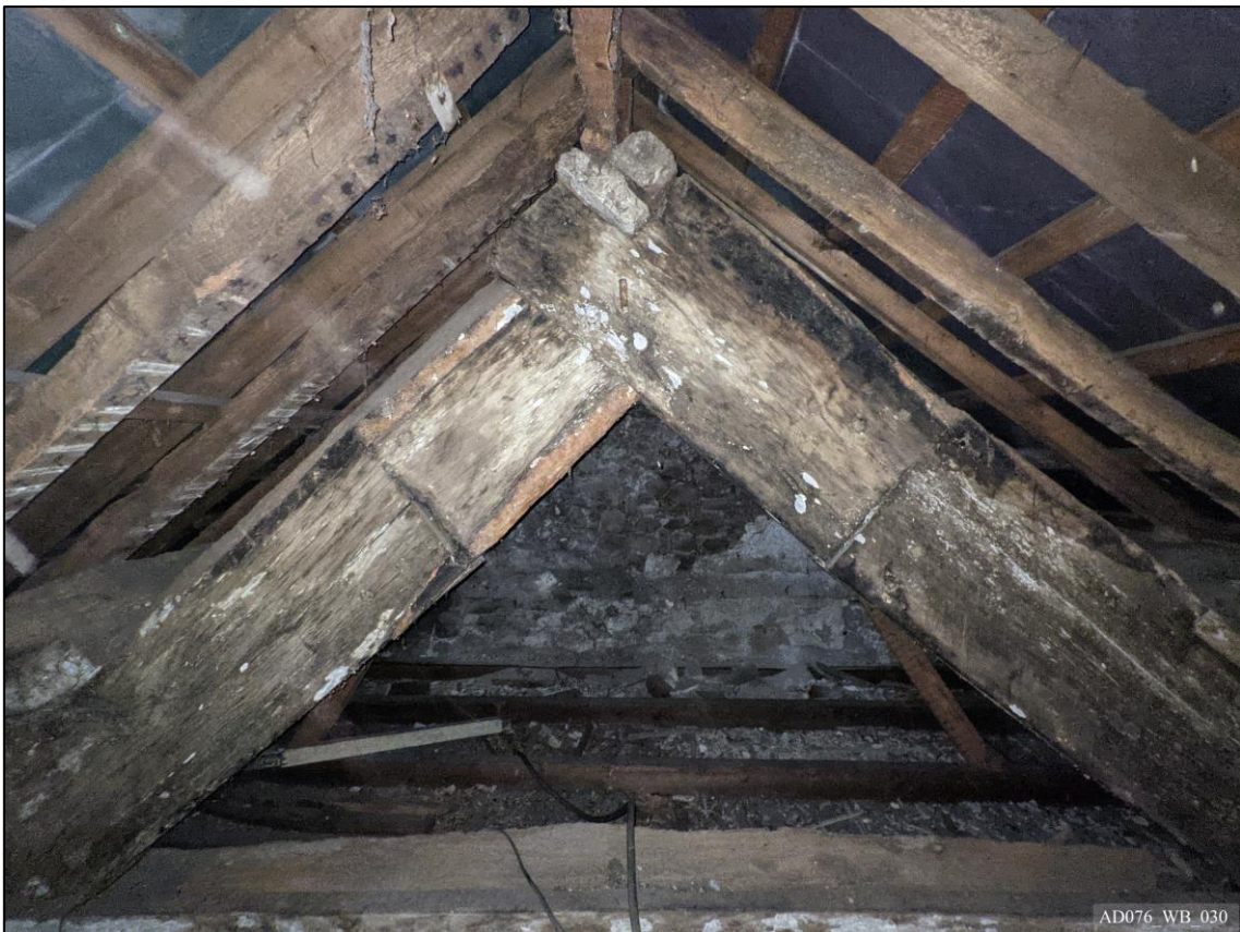
Plate 30 – Apex of truss.
