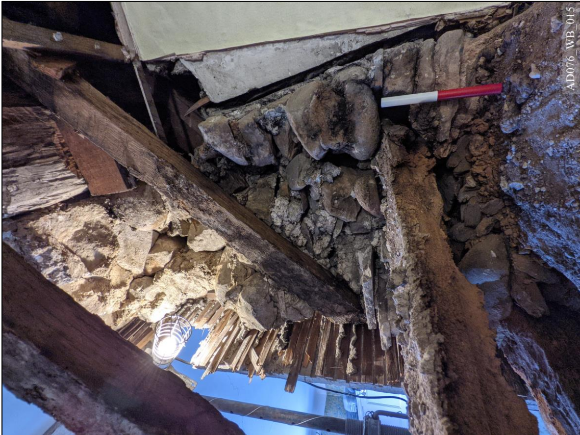
Plate 15 – View west, showing change in masonry and common rafters.
