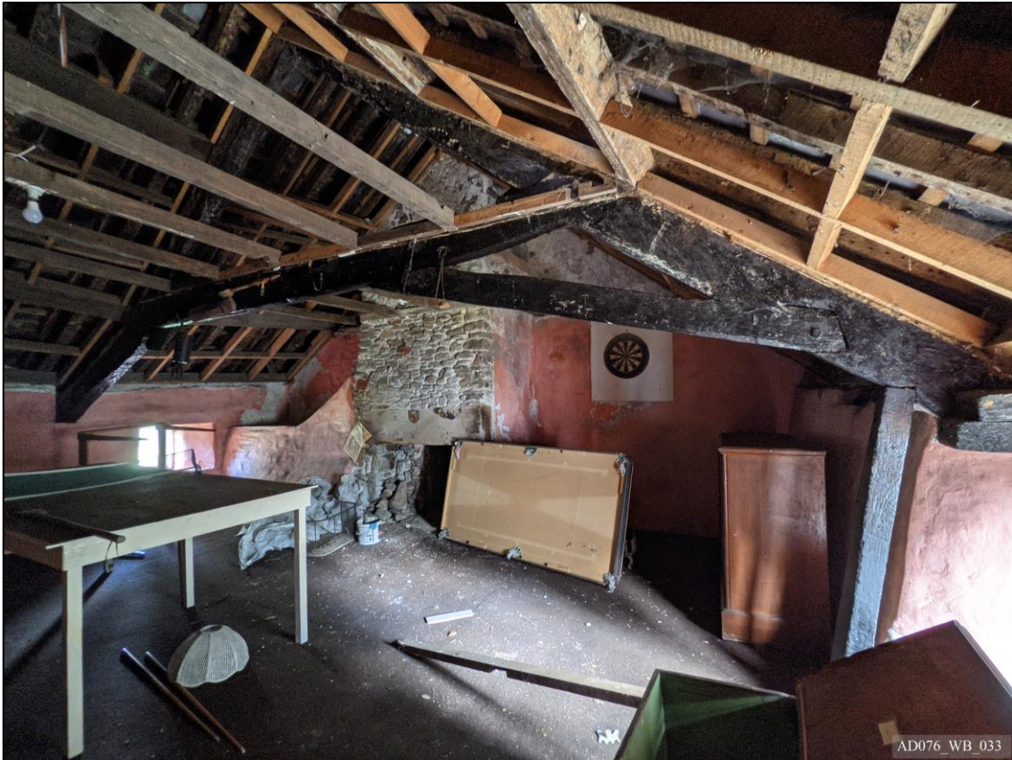
Plate 33 – View north, showing truss to [FF16].
