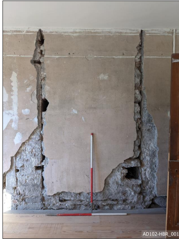
Plate 1 – Doorway A – View south-west, showing north-east elevation.
