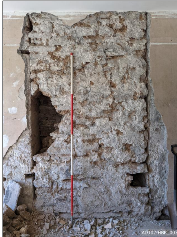
Plate 7 – View south-west, showing removal of plaster.
