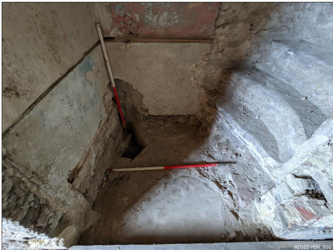
Plate 16 – Doorway B – View south-west, showing intermural steps and stair.
