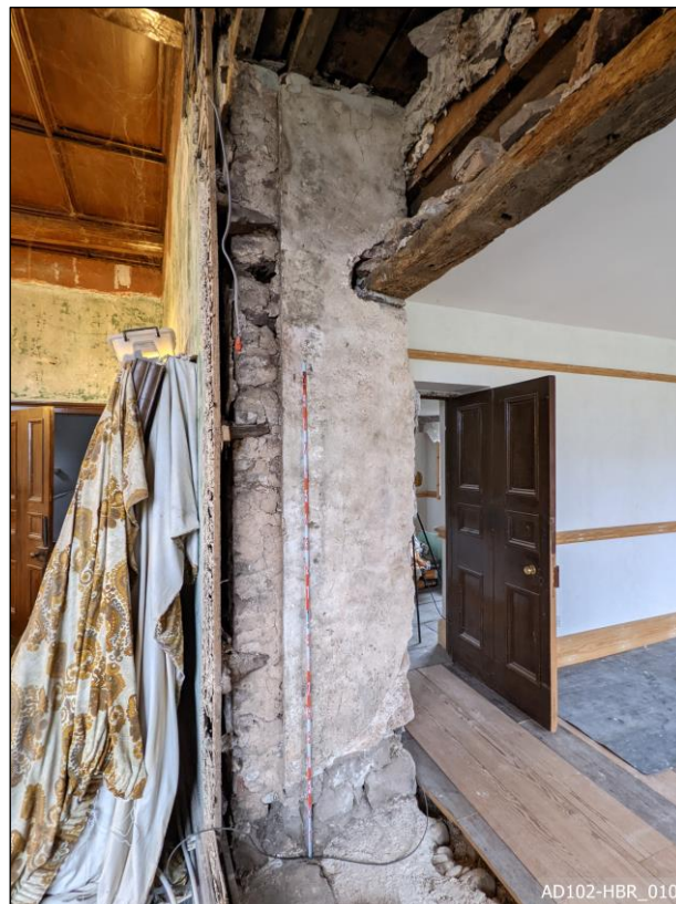
Plate 10 – Doorway A – View north, showing north reveal of doorway.
