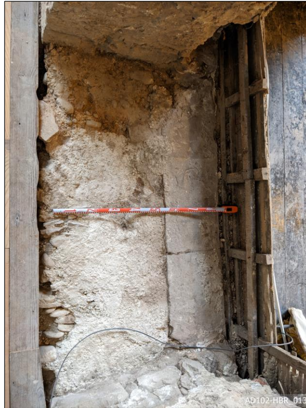
Plate 13 – Doorway A – Threshold of doorway.
