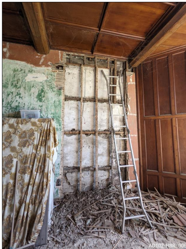
Plate 6 – Doorway A – View north-west, showing removal of lath-and-plaster.
