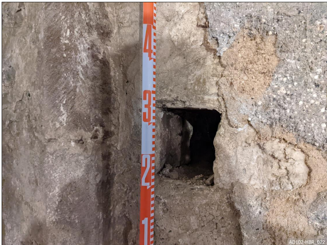
Plate 22 – Doorway B – View south, showing draw bar socket.
