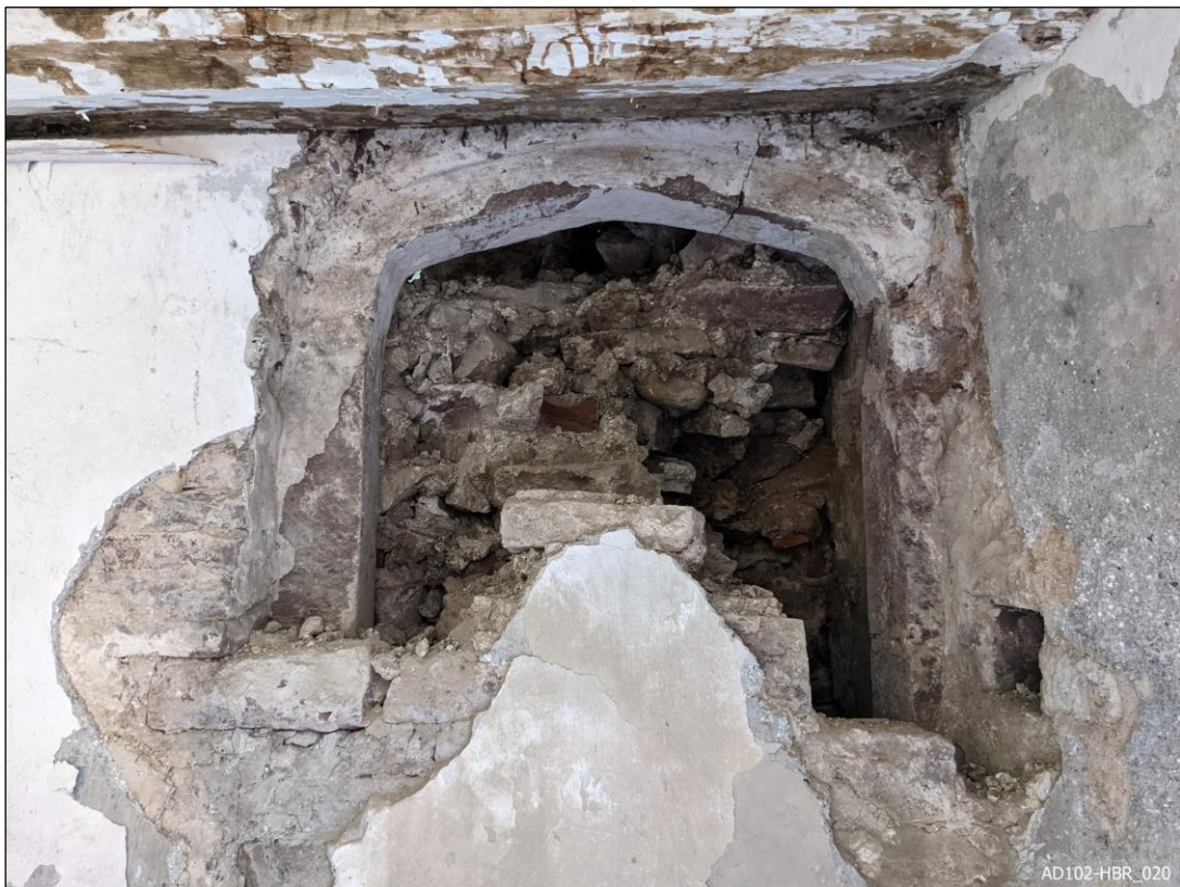
Plate 20 – Doorway B – View north-east, showing doorway unblocking.
