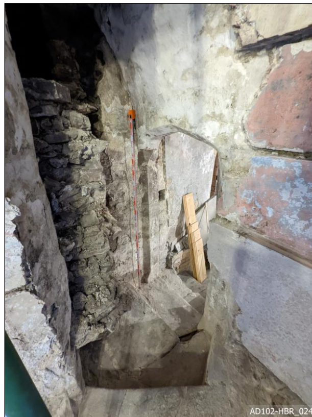
Plate 24 – Doorway B – View south, showing intermural stair passage.
