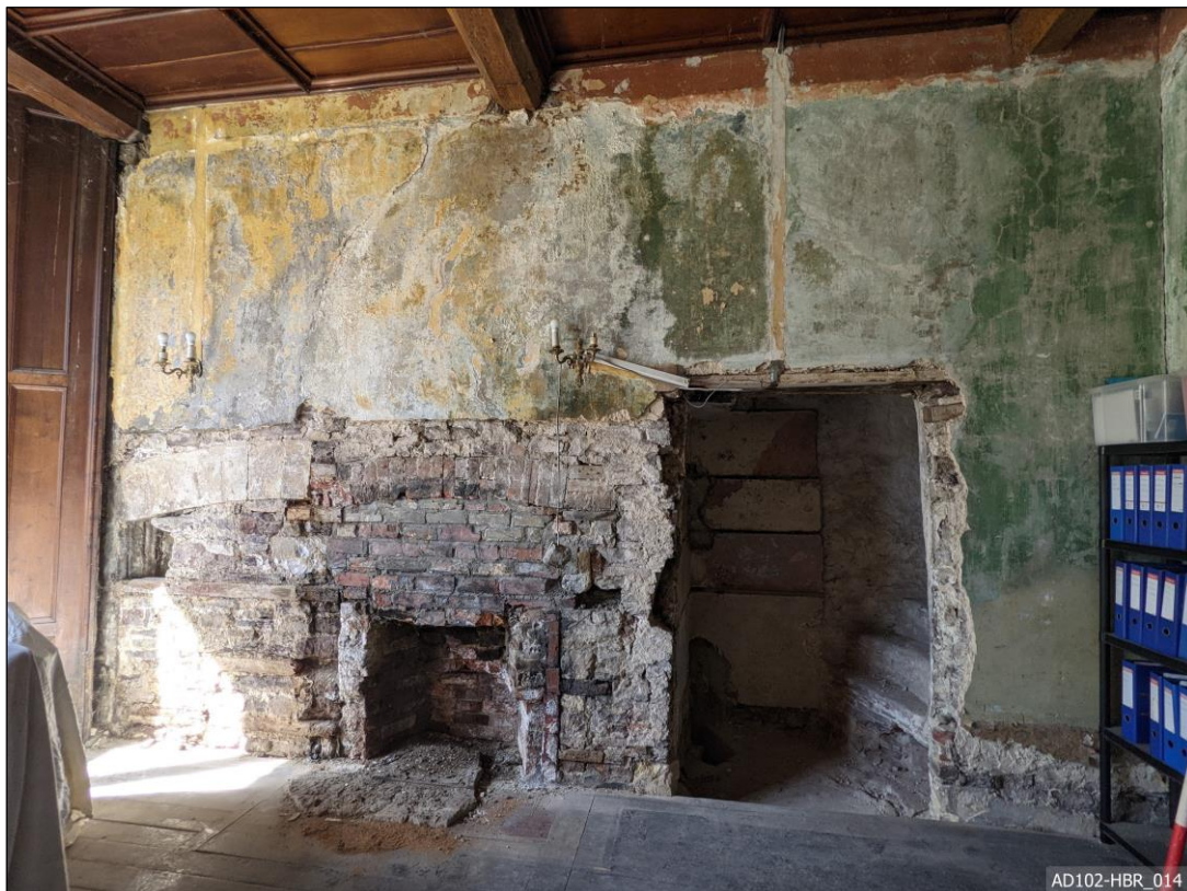
Plate 14 – Doorway B – View south-west, showing north-east elevation.
