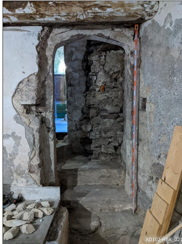
Plate 21 – Doorway B – View north-east, showing doorway reopened.
