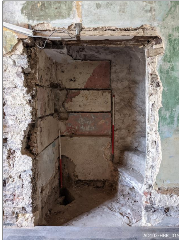
Plate 15 – Doorway B – View south-west, showing north-east elevation.
