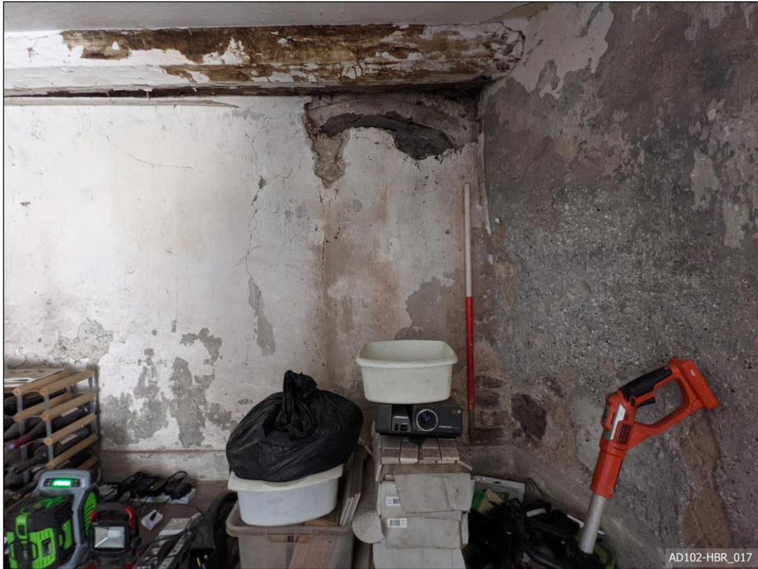
Plate 17 – Doorway B – View north-east, showing south-west elevation.
