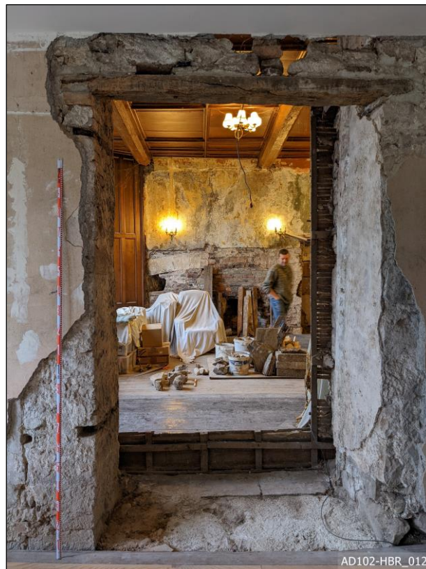
Plate 12 – Doorway A – View south-west, showing opened doorway with lower head.
