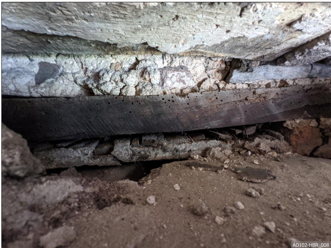
Plate 8 – Doorway A – View north-east, showing early-19 th century lath-and-plaster of door passage head.
