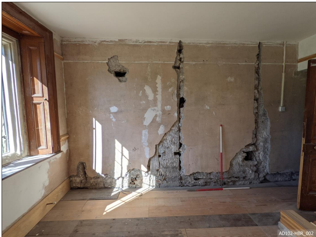
Plate 2 – Doorway A – View south-west, showing north-east elevation.
