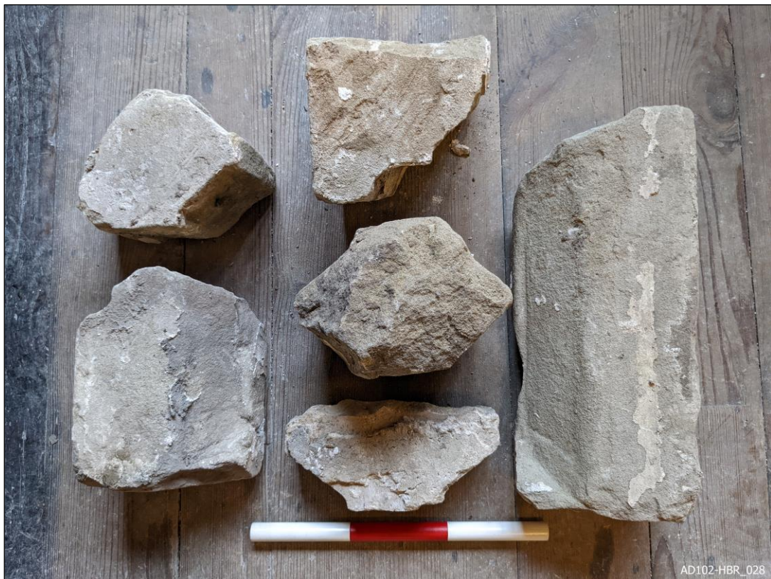
Plate 28 – Doorway A – Recovered window mullions and jambs.
