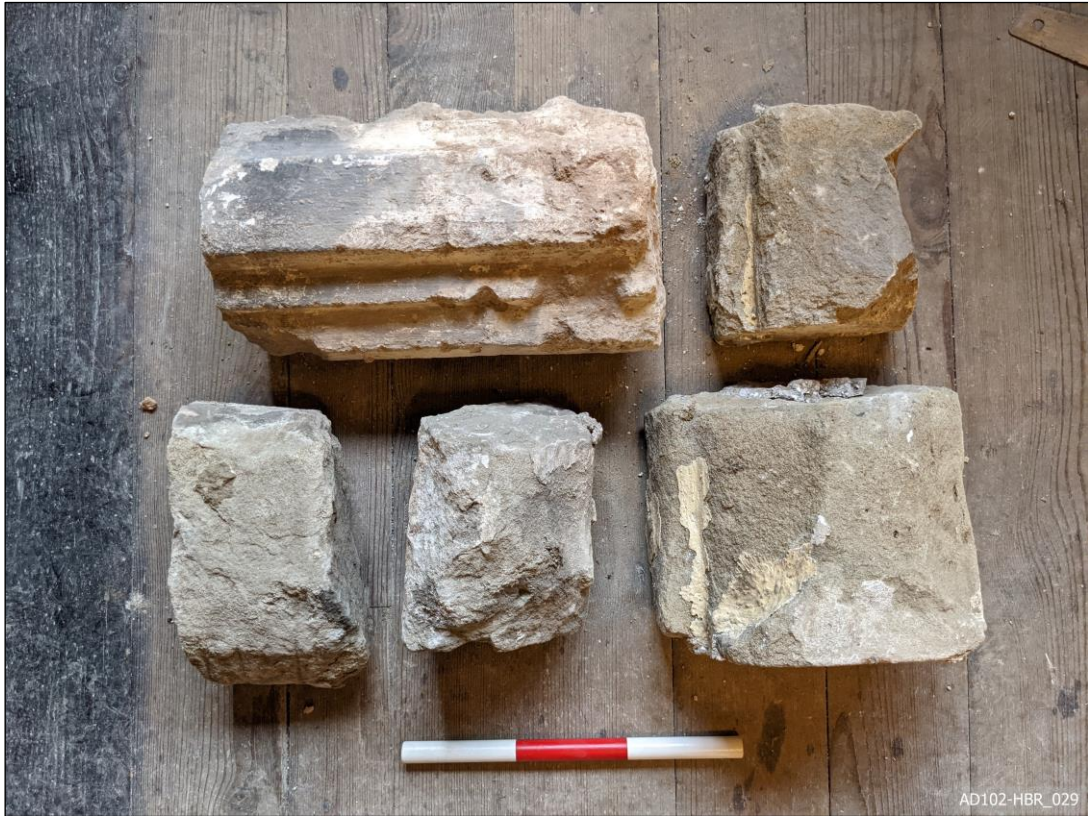
Plate 29 – Doorway A – Recovered window mullions and jambs.
