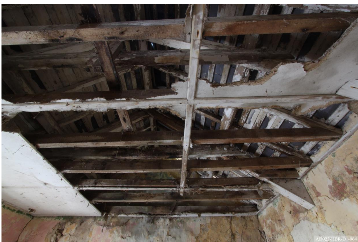
Plate 64 – View towards south of extension, showing roof truss 10.
