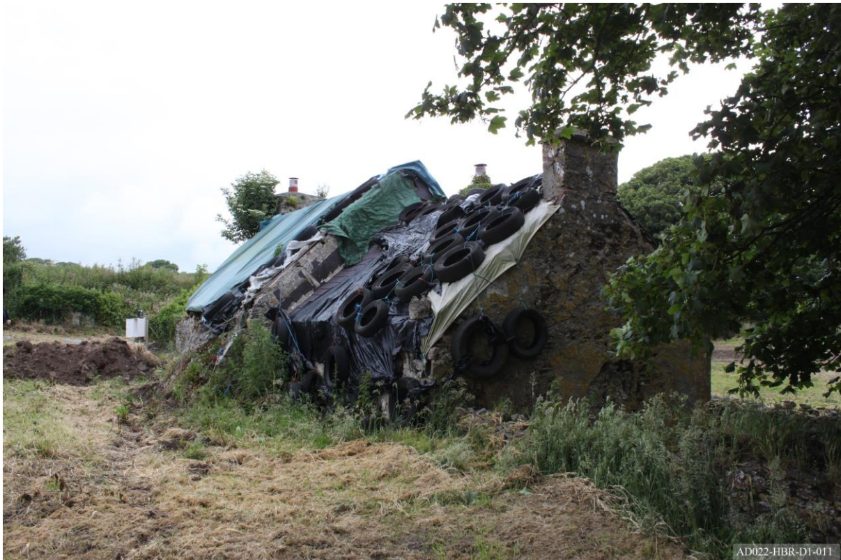
Plate 11 – View towards north, showing extension and cottage.
