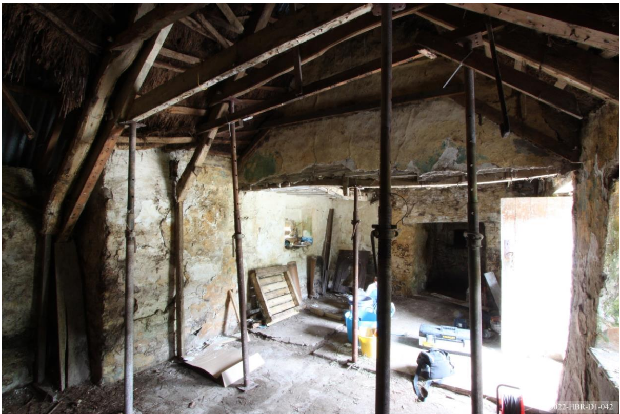
Plate 42 – View north-west of cottage.
