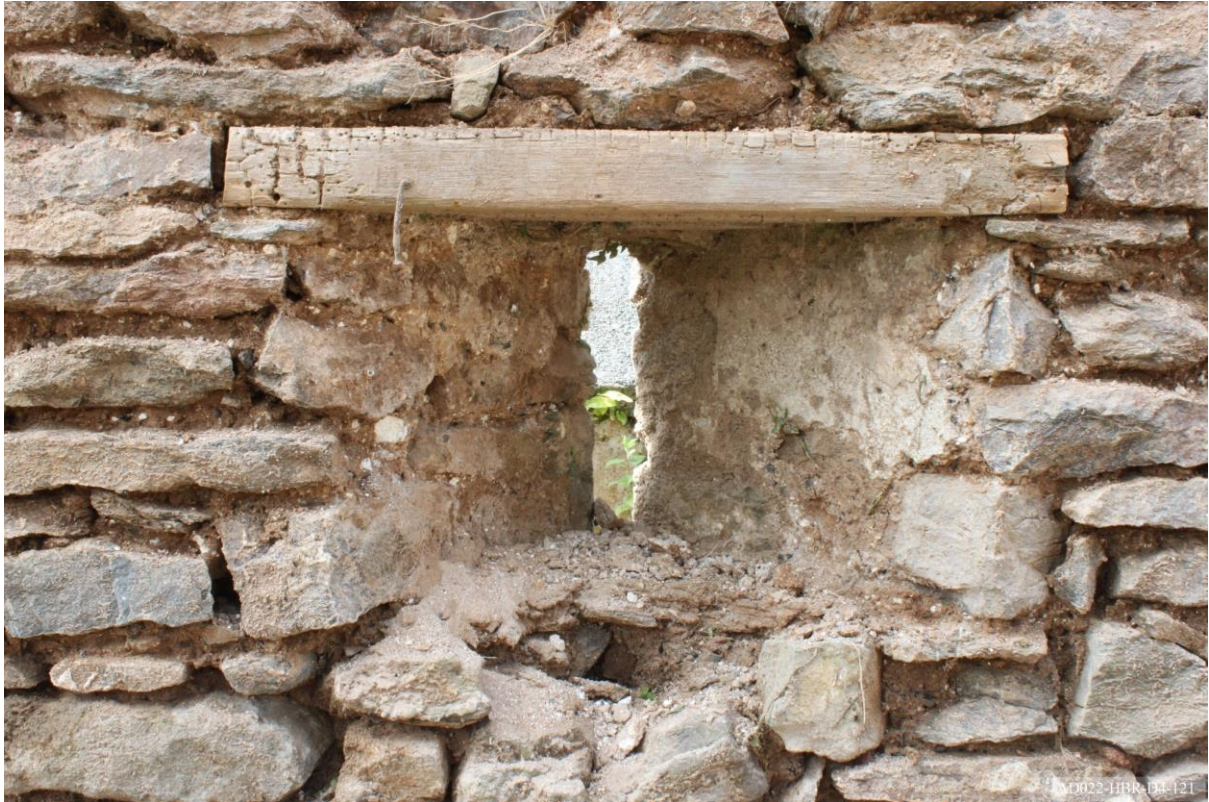
Plate 121 – View towards south of HB1, showing ventilation slit.
