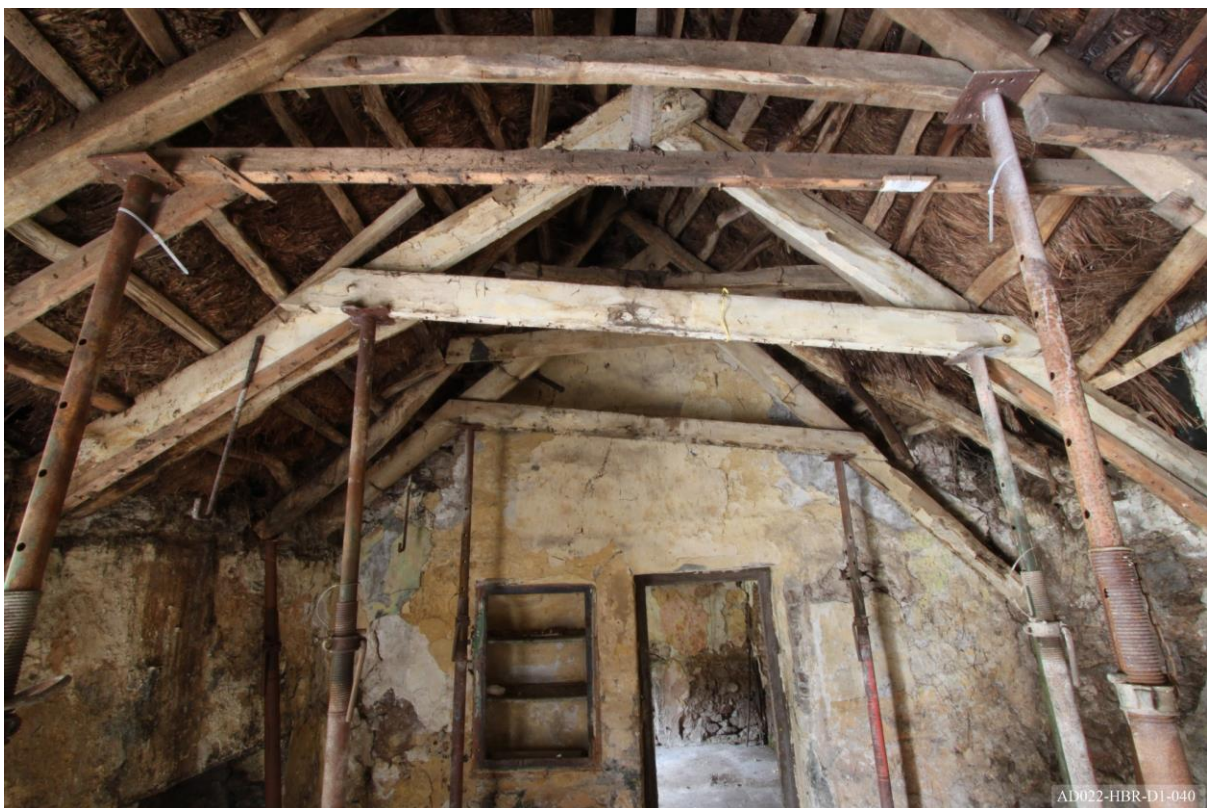
Plate 40 – View towards south of cottage, showing trusses 4-8.
