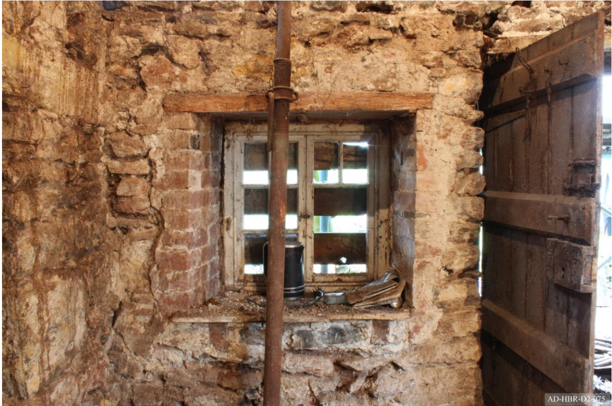
Plate 75 – View towards east of cottage, showing brick reveals to northern window.
