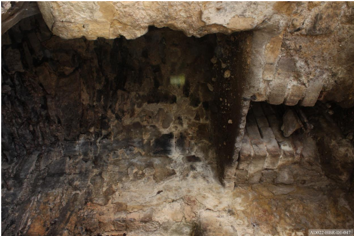
Plate 47 – View towards east of cottage, showing later hearth insertion.
