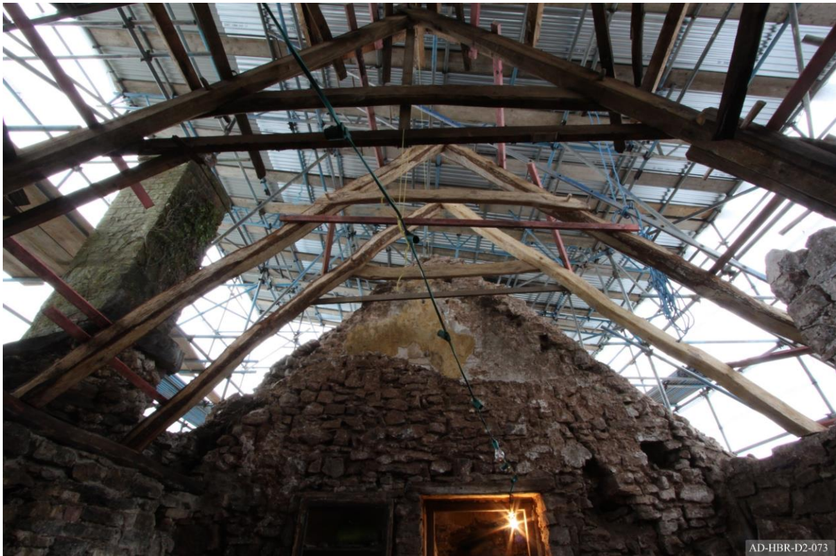
Plate 73 – View towards south of cottage, showing new trusses to south end.
