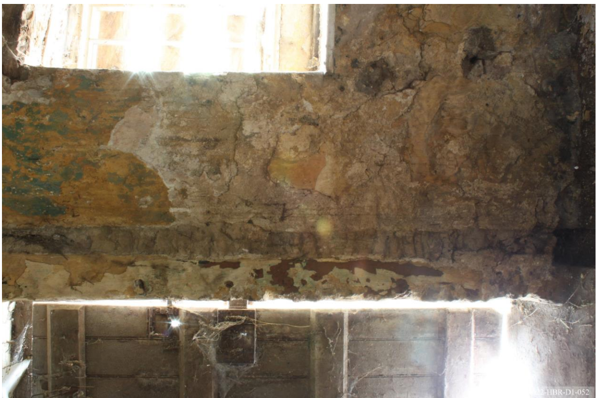
Plate 52 – View towards east of cottage, showing plaster scar of former partition.
