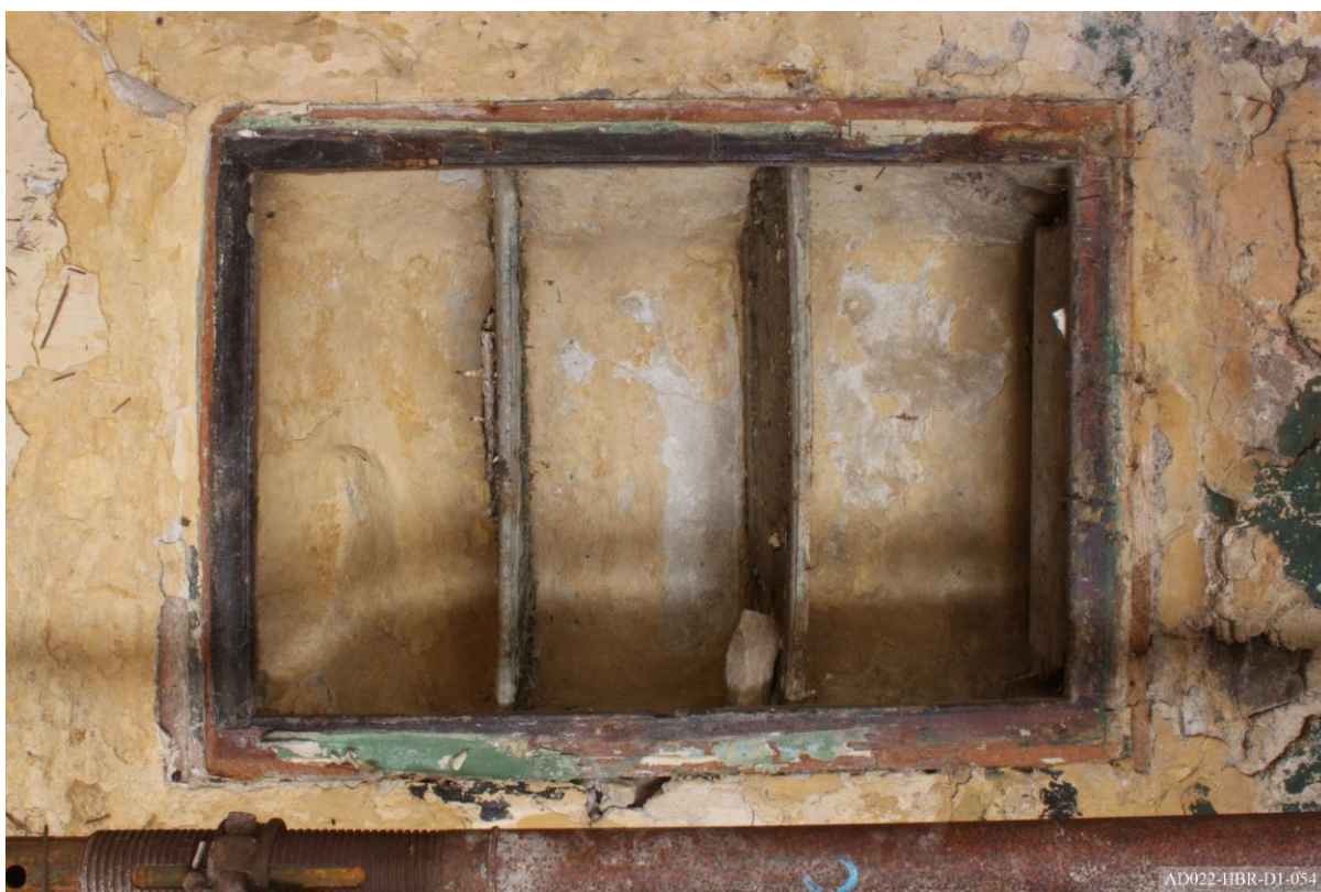
Plate 54 – View towards south of cottage, showing wall cupboard.
