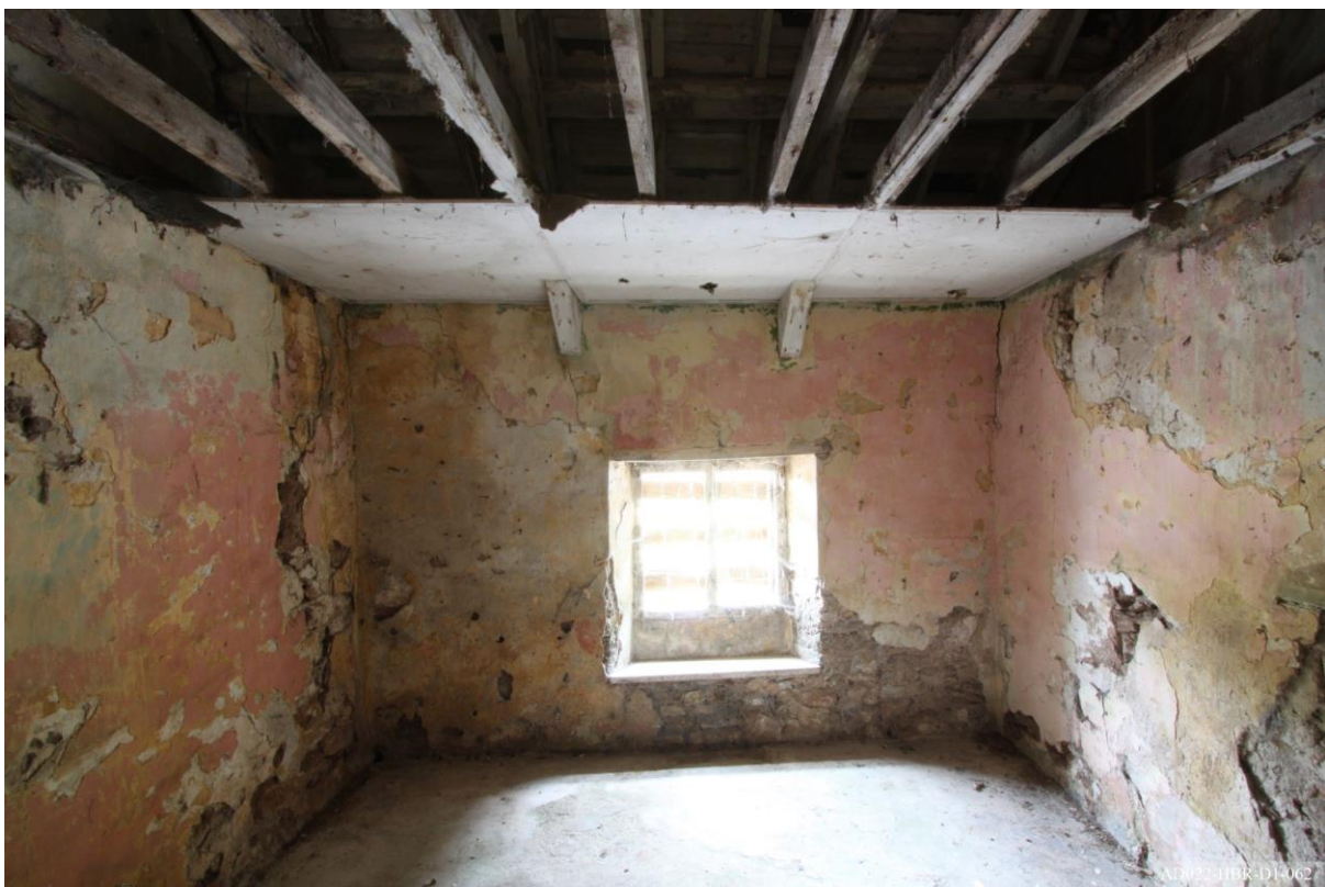
Plate 62 – View towards east of extension, showing window.
