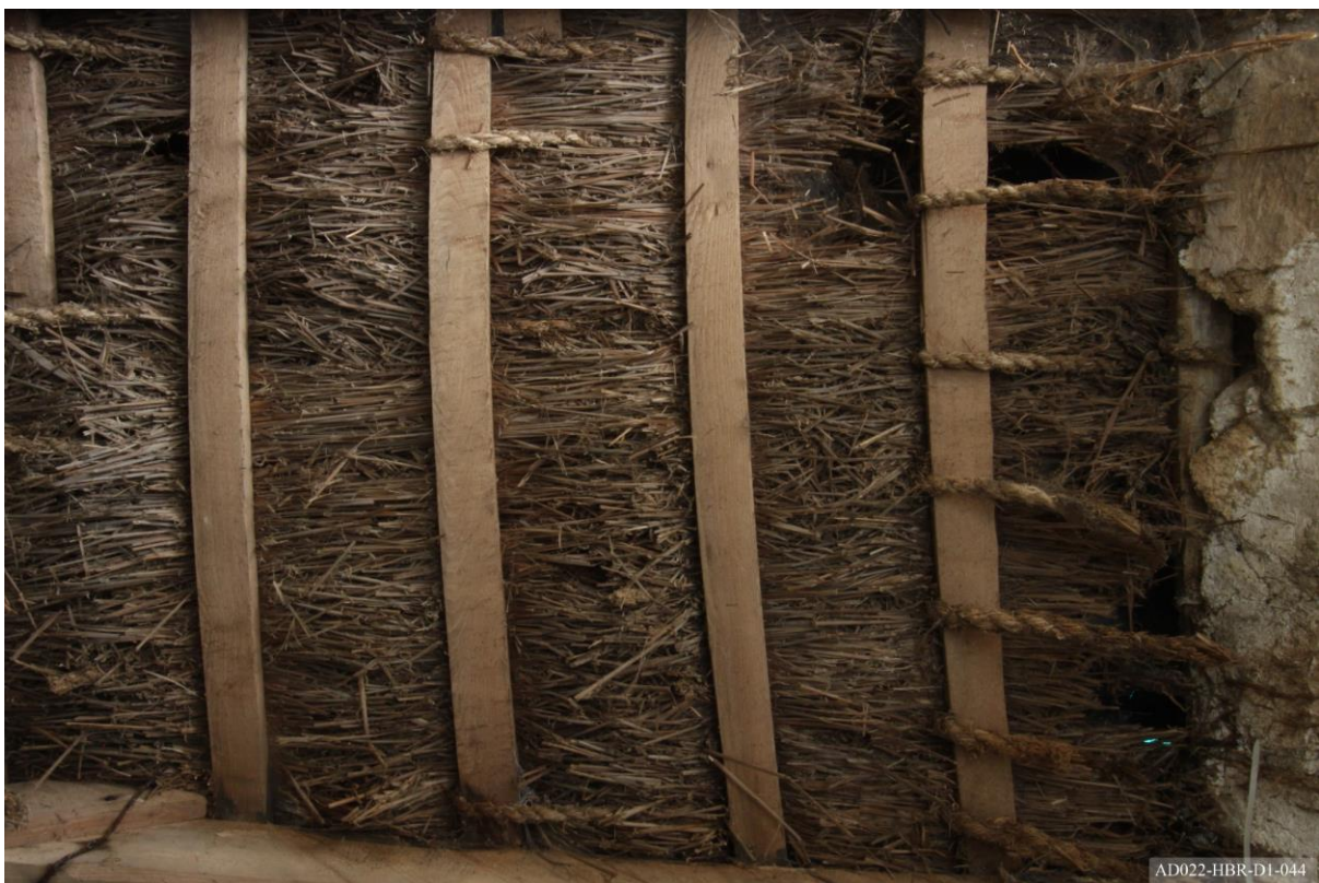
Plate 44 – View towards east of cottage, showing detail of underthatch.
