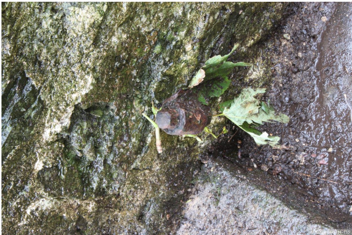
Plate 135 – Iron pintle to pigsty entrance.
