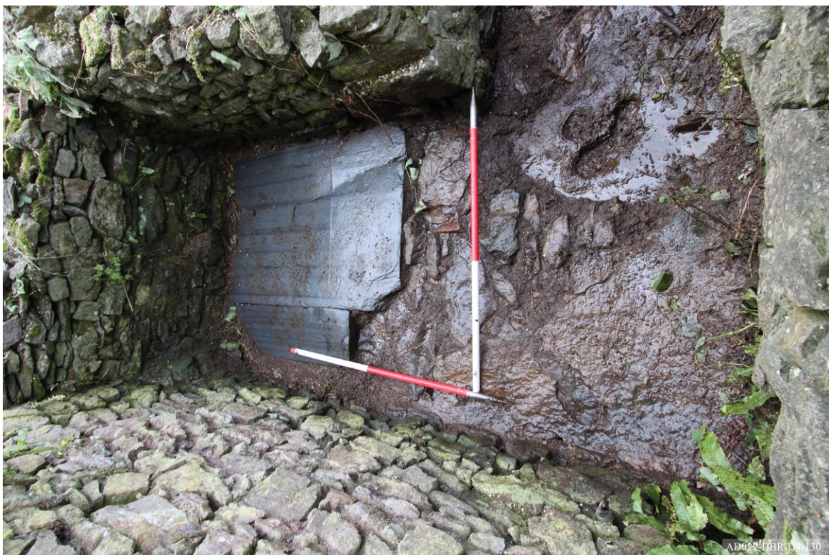
Plate 130 – View towards west of pigsty internal bay, showing conglomerate floor.
