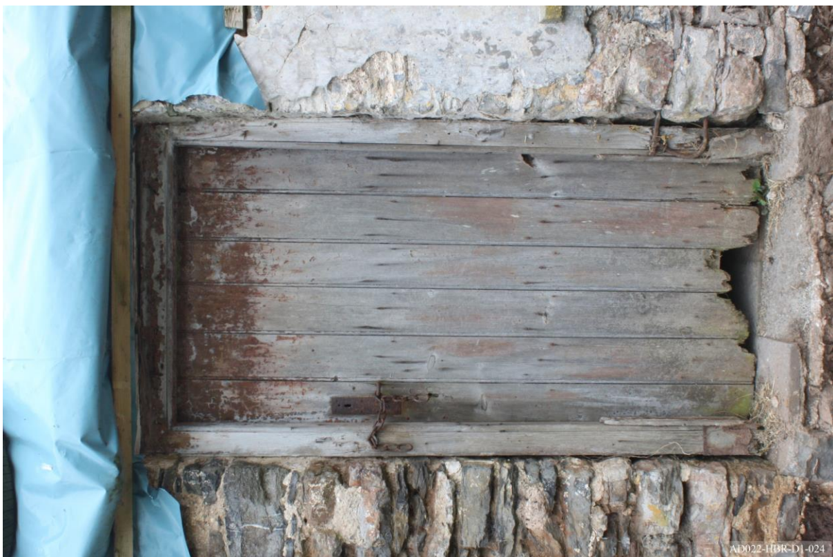
Plate 24 – View of east elevation, showing doorway to cottage.
