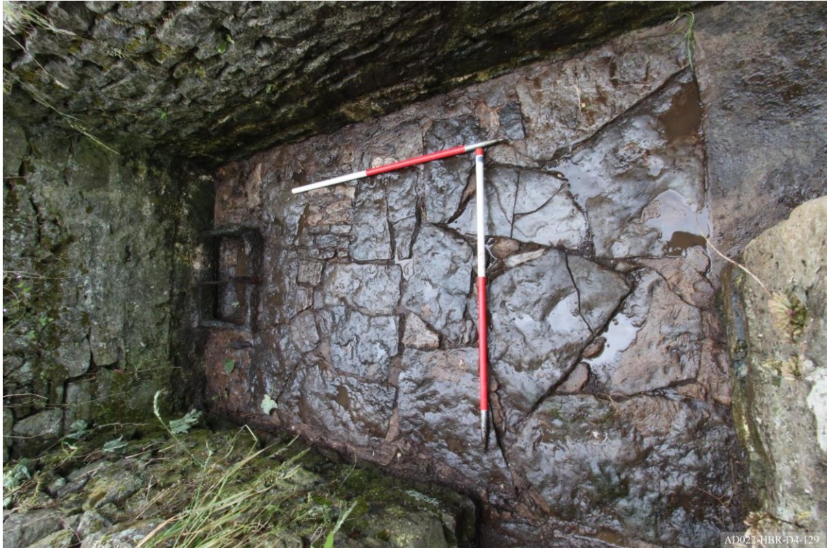
Plate 129 – View towards west of pigsty external bay, showing conglomerate floor and trough.
