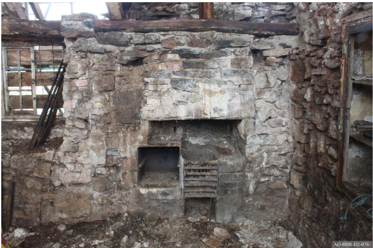
Plate 76 – View towards east of cottage, showing inserted masonry of the lateral chimney.
