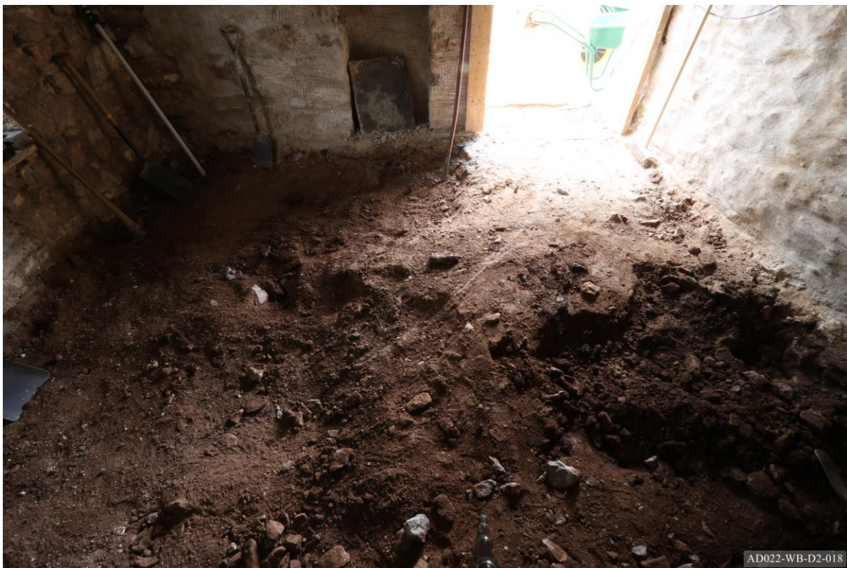
Plate 154 – Internal excavation, showing natural subsoil (205) and bedrock (206) in extension.
