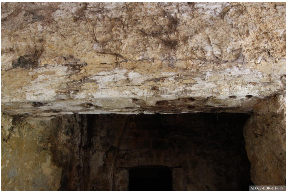
Plate 58 – View towards north of cottage, showing fireplace bresummer of reused oak.
