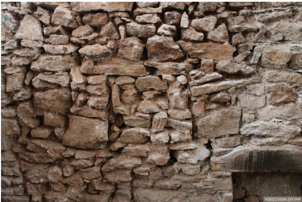
Plate 98 – View towards south of extension, showing blocked window to south gable wall prior to dismantling.
