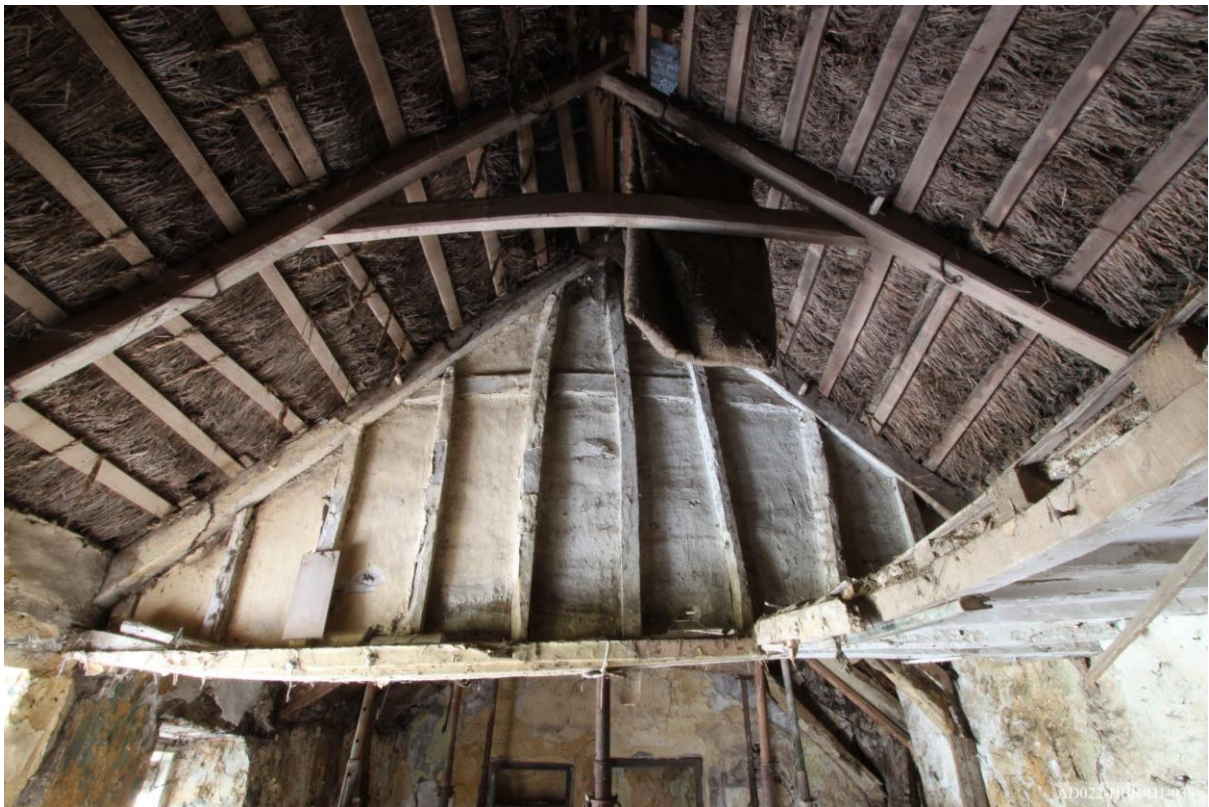
Plate 38 – View towards south of cottage, showing truss 2 and 3 (partition).
