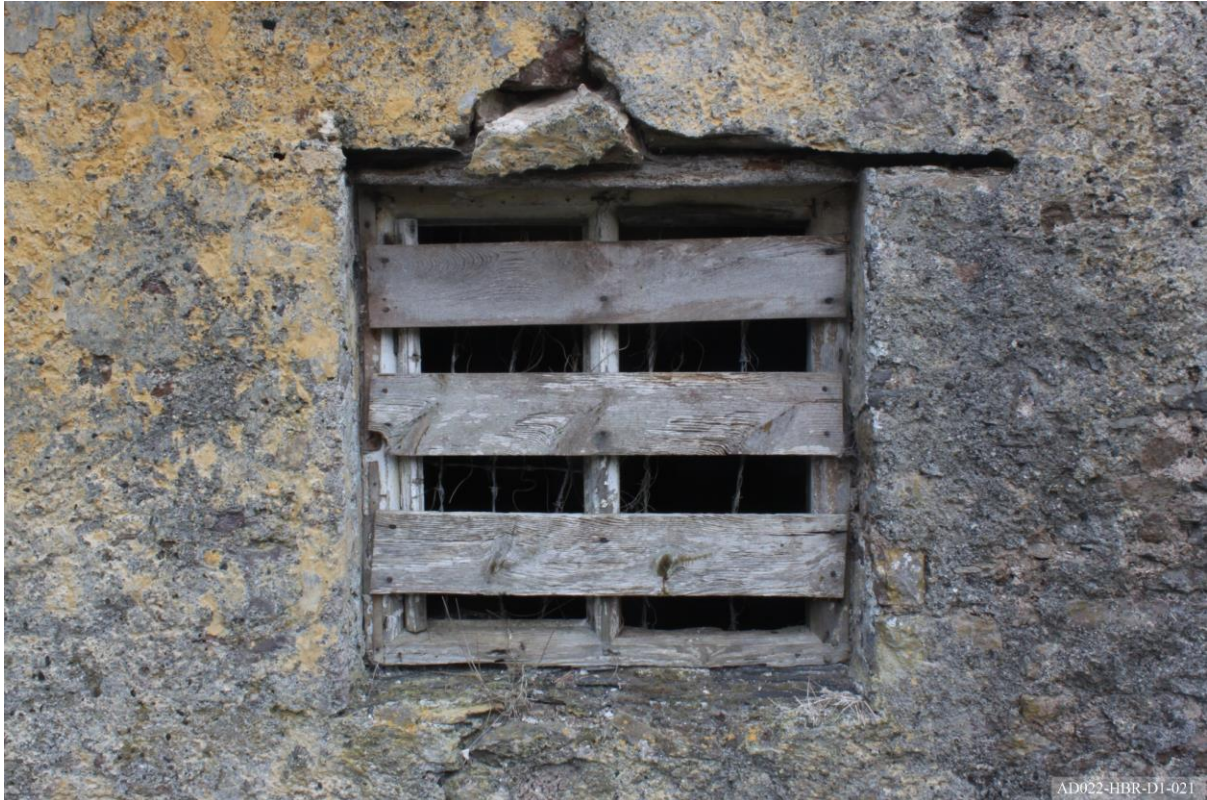
Plate 21 – View of east elevation, showing window to extension.
