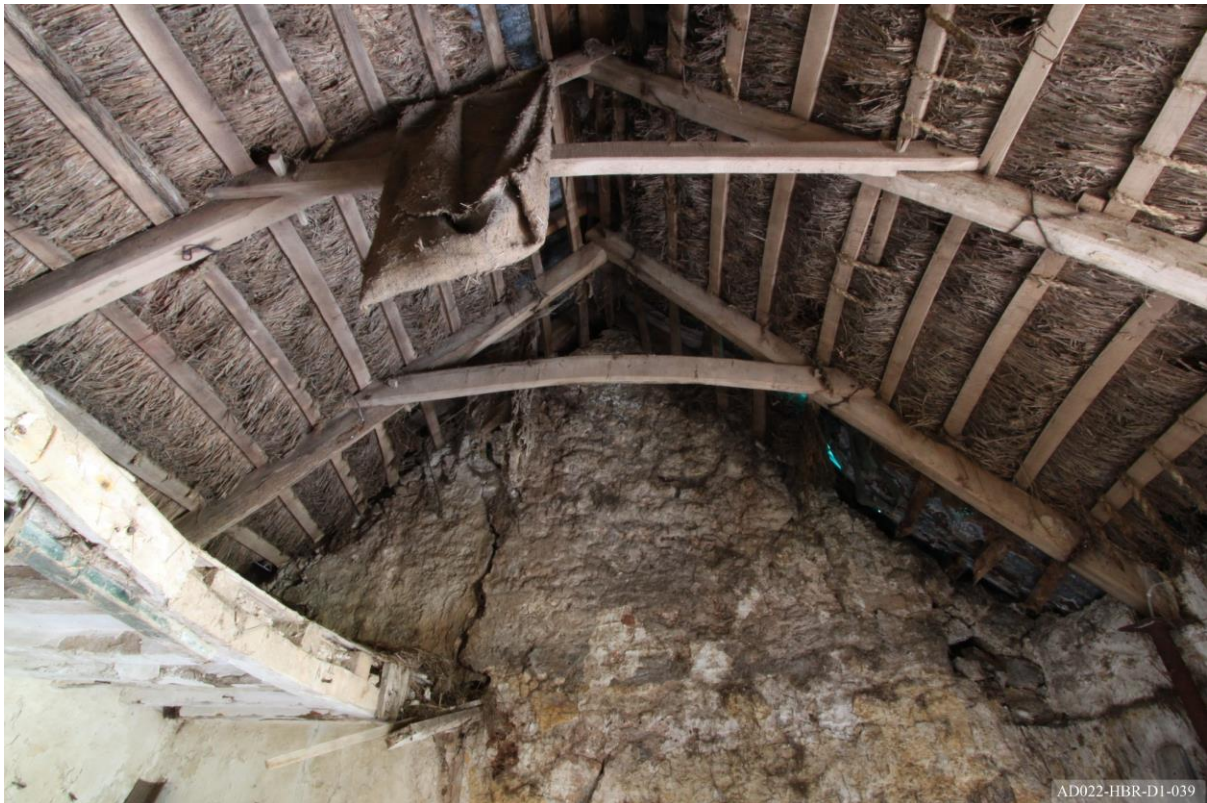
Plate 39 – View towards north of cottage, showing truss 1 and 2.
