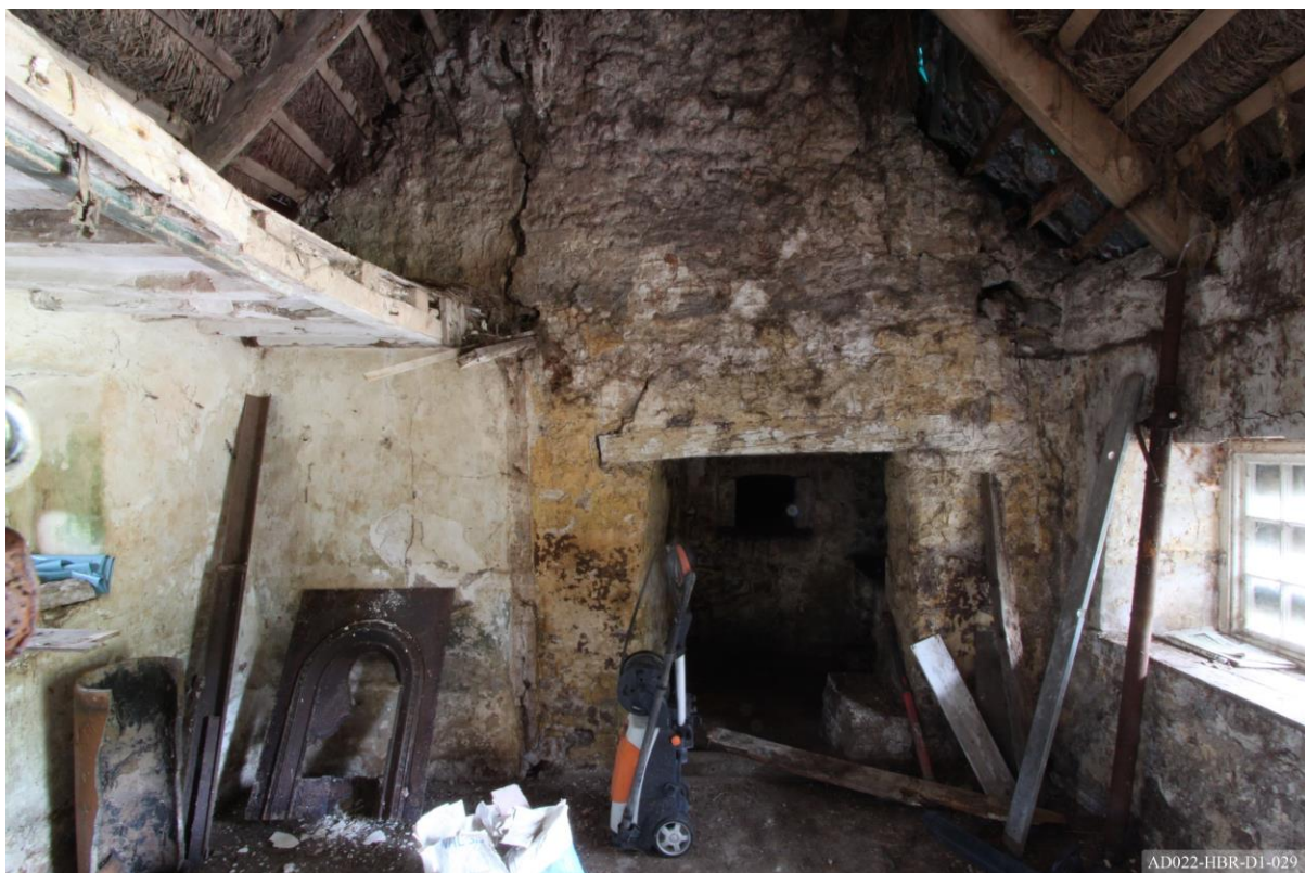
Plate 29 – View towards north of cottage, showing fireplace and pantry ceiling.
