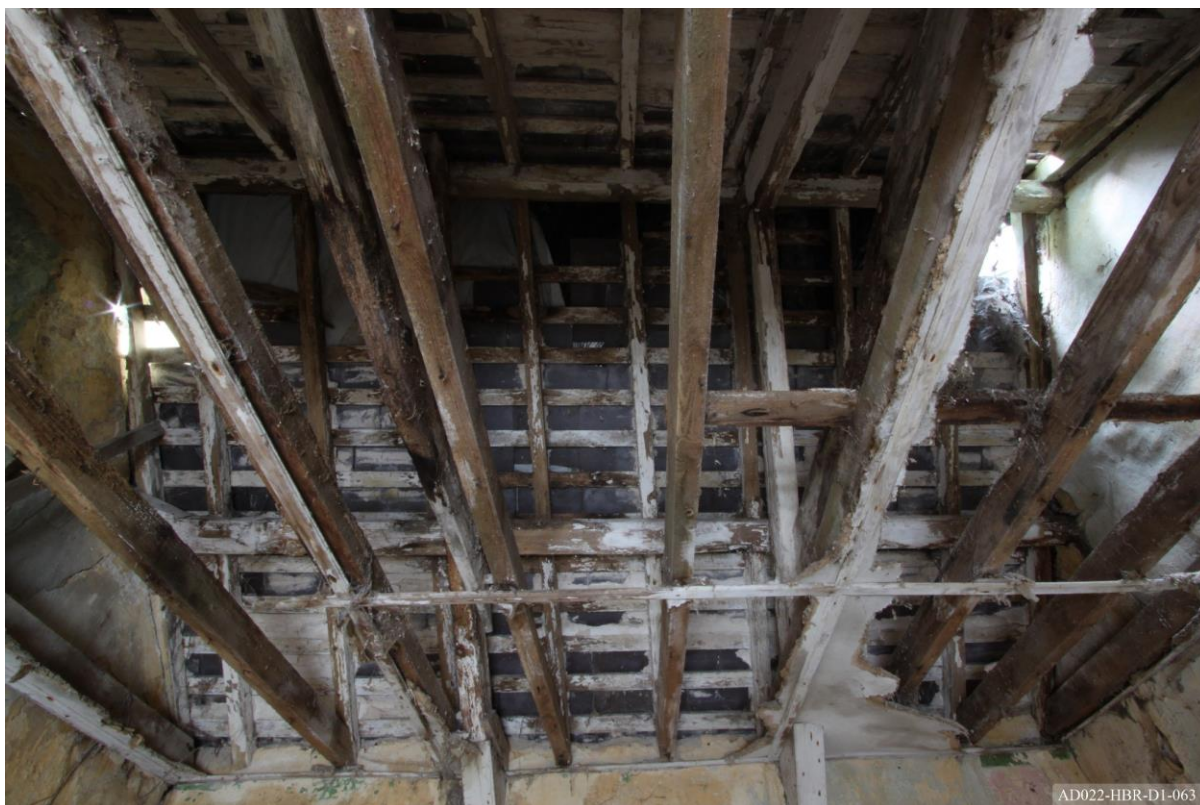
Plate 63 – View towards west of extension, showing roof trusses 9-10, purlin and rafters.
