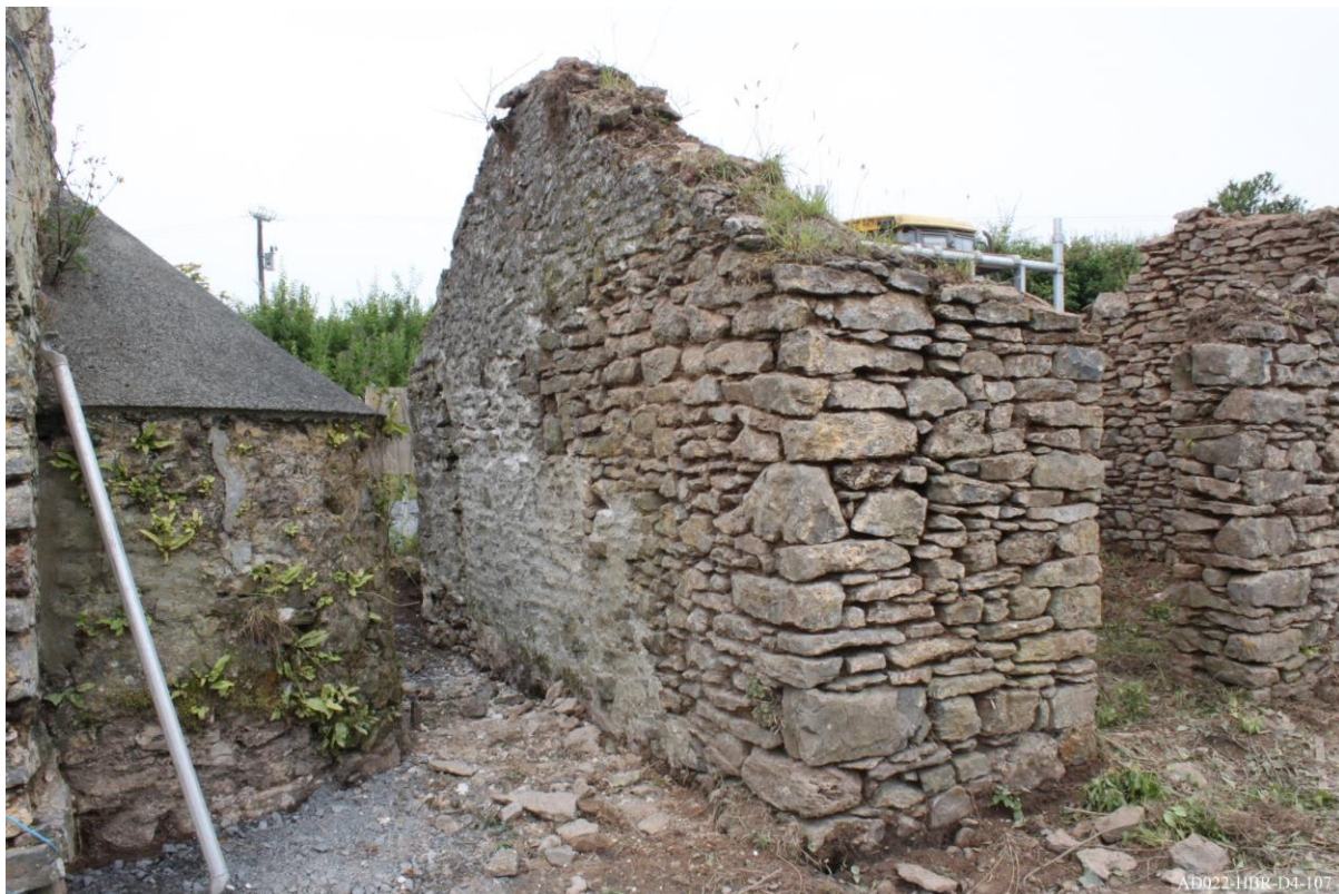
Plate 107 – View of south elevation of HB1.
