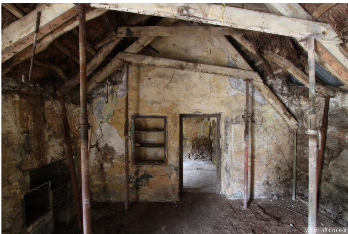
Plate 30 – View towards south of cottage, showing cupboard and doorway to extension.
