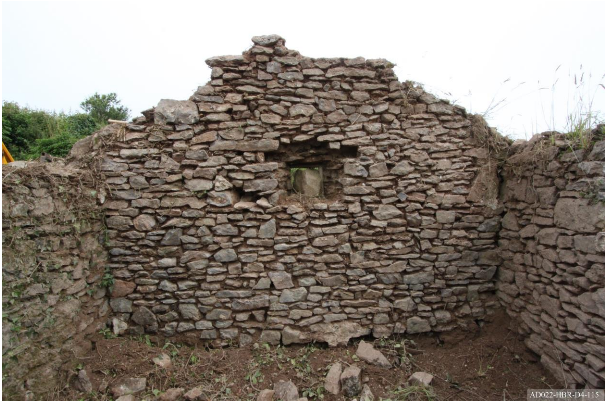
Plate 115 – View towards north of HB1, showing blocked window.
