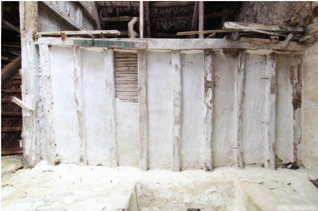
Plate 43 – View of underside of pantry ceiling, of cottage.
