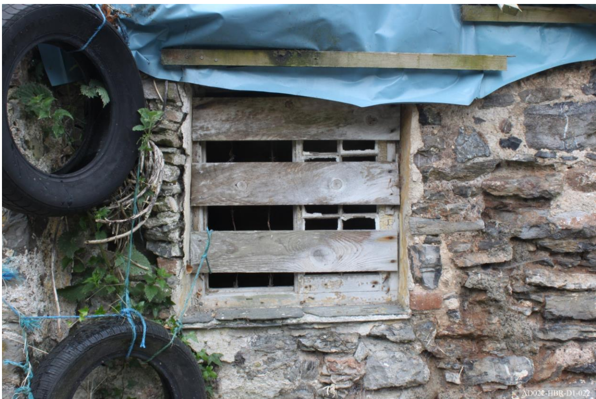
Plate 22 – View of east elevation, showing southern window of cottage.
