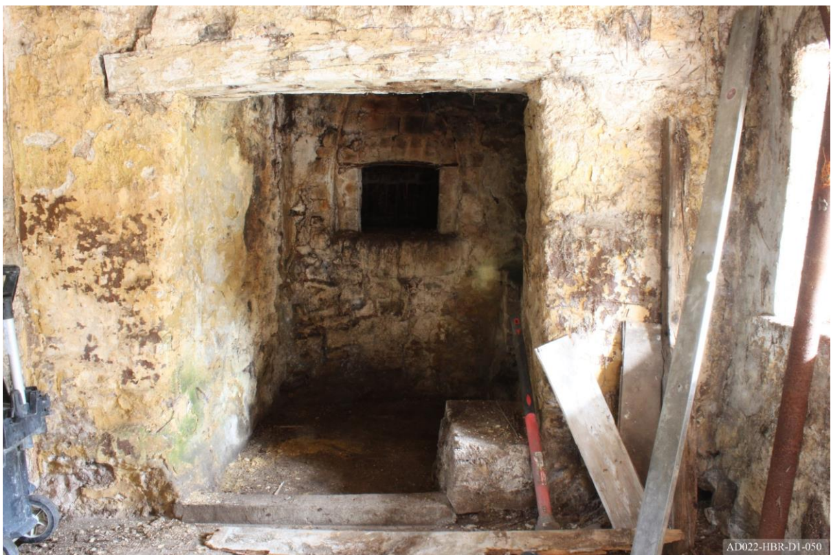
Plate 50 – View towards north of cottage, showing fireplace.
