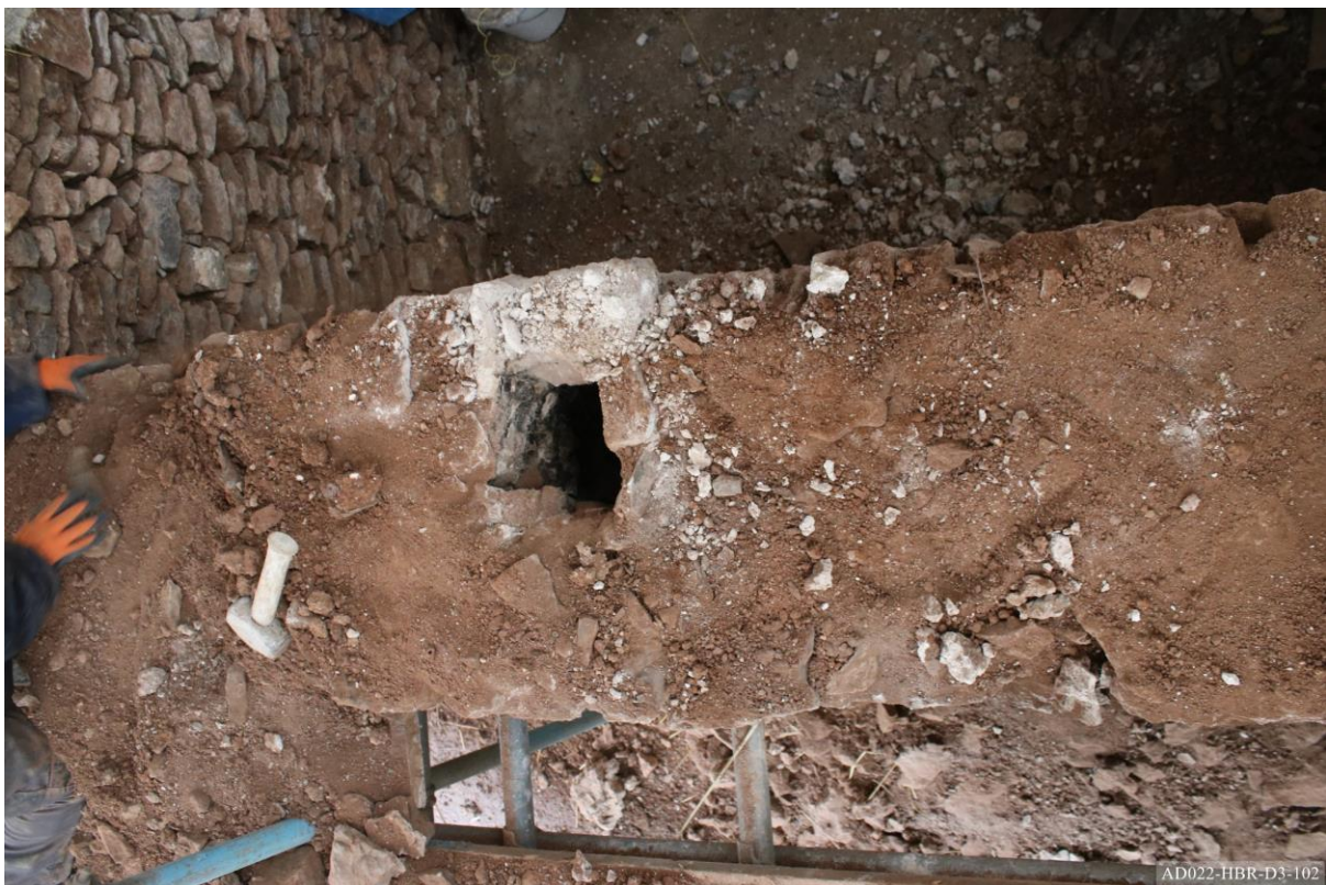
Plate 102 – View showing chimney flue, and earth mortar and rubble fill to south gable wall.
