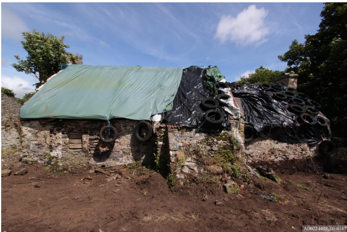
Plate 14 – View of west elevation, showing cottage (left) and extension (right).
