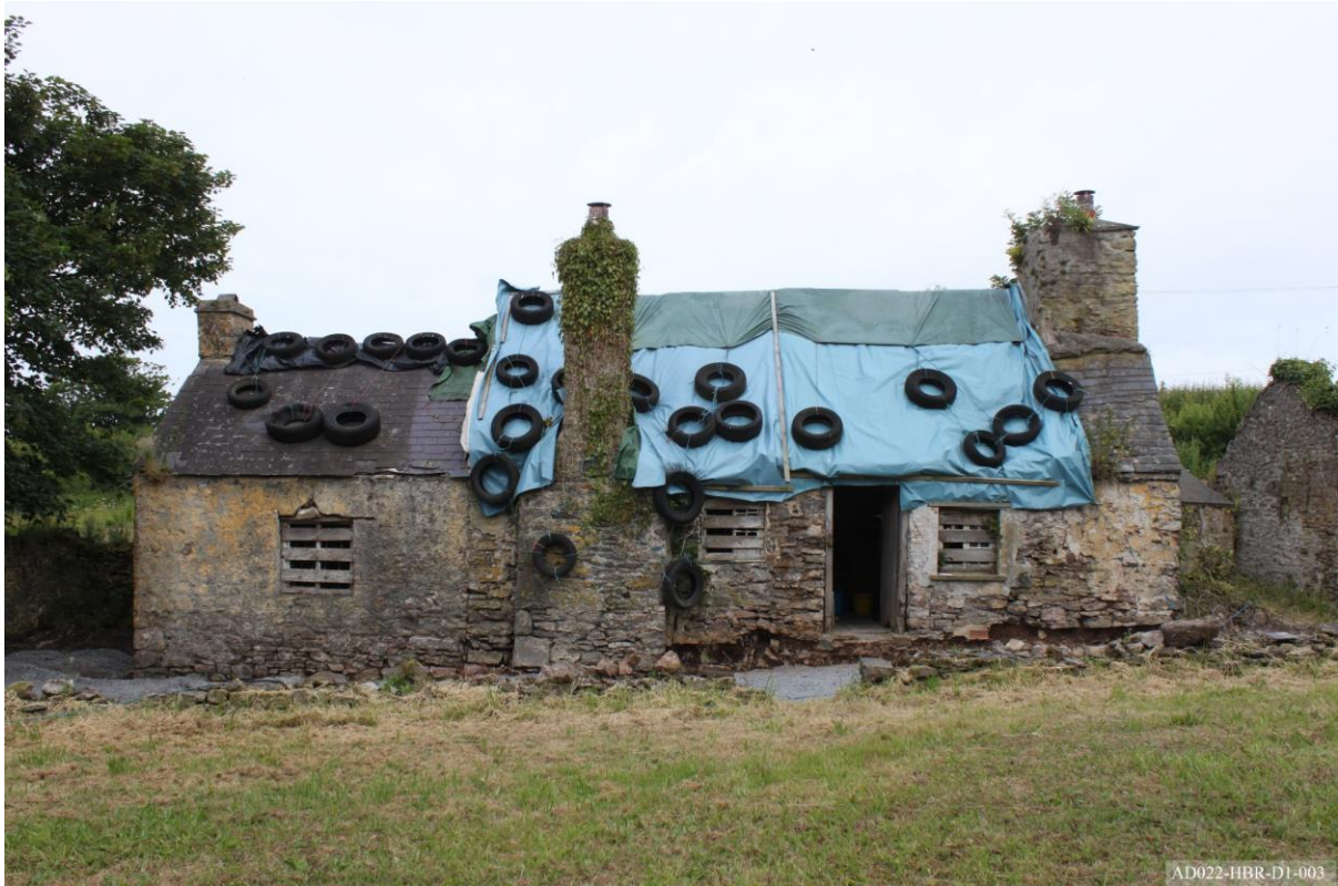
Plate 3 – East Elevation, showing cottage (right) and extension (left).
