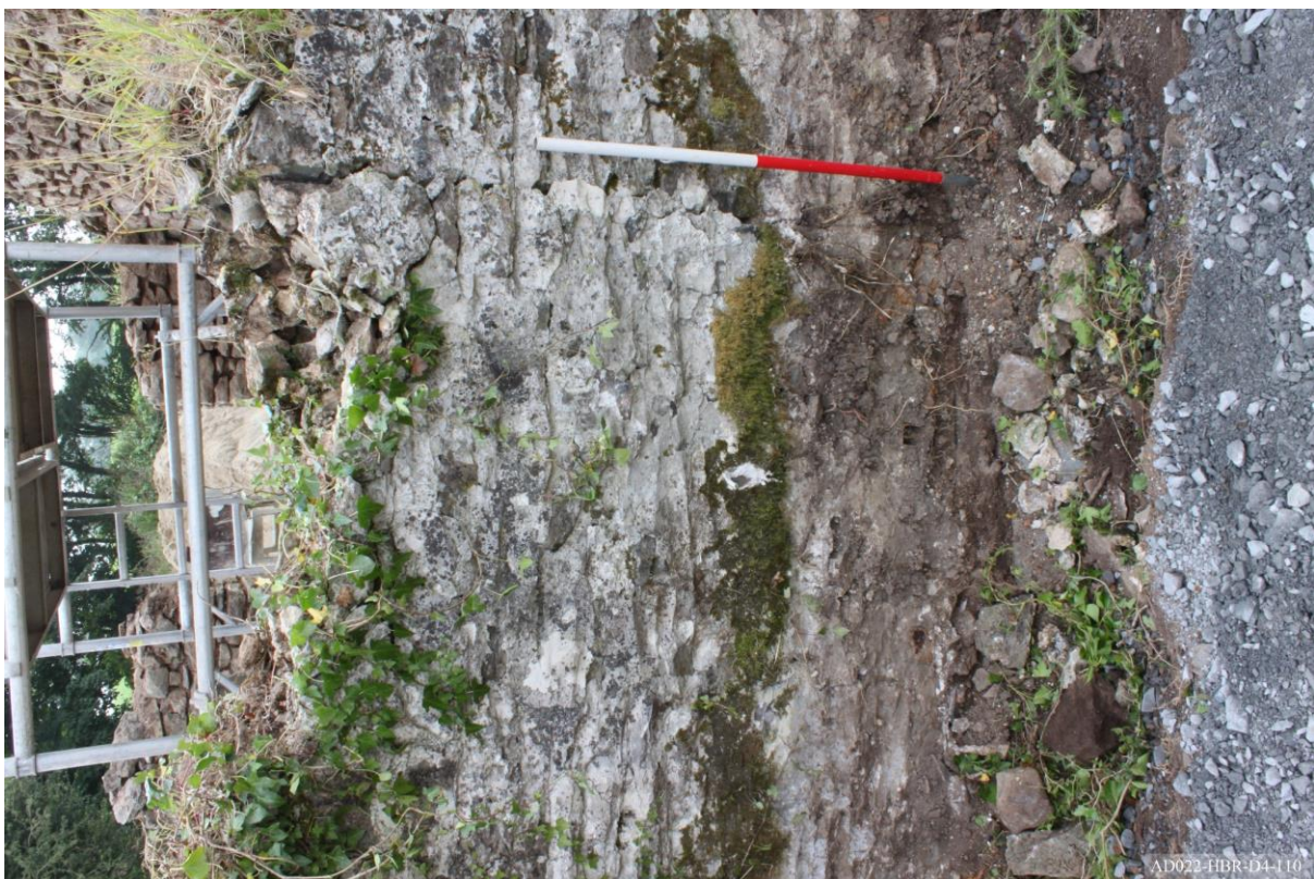
Plate 110 – View of west elevation of HB1, showing masonry joint to blocked doorway.
