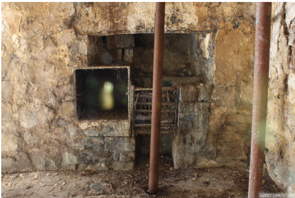
Plate 53 – View towards east of cottage, showing range to lateral chimney.
