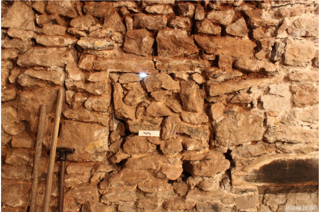
Plate 81 – View towards south of extension, showing blocked window.
