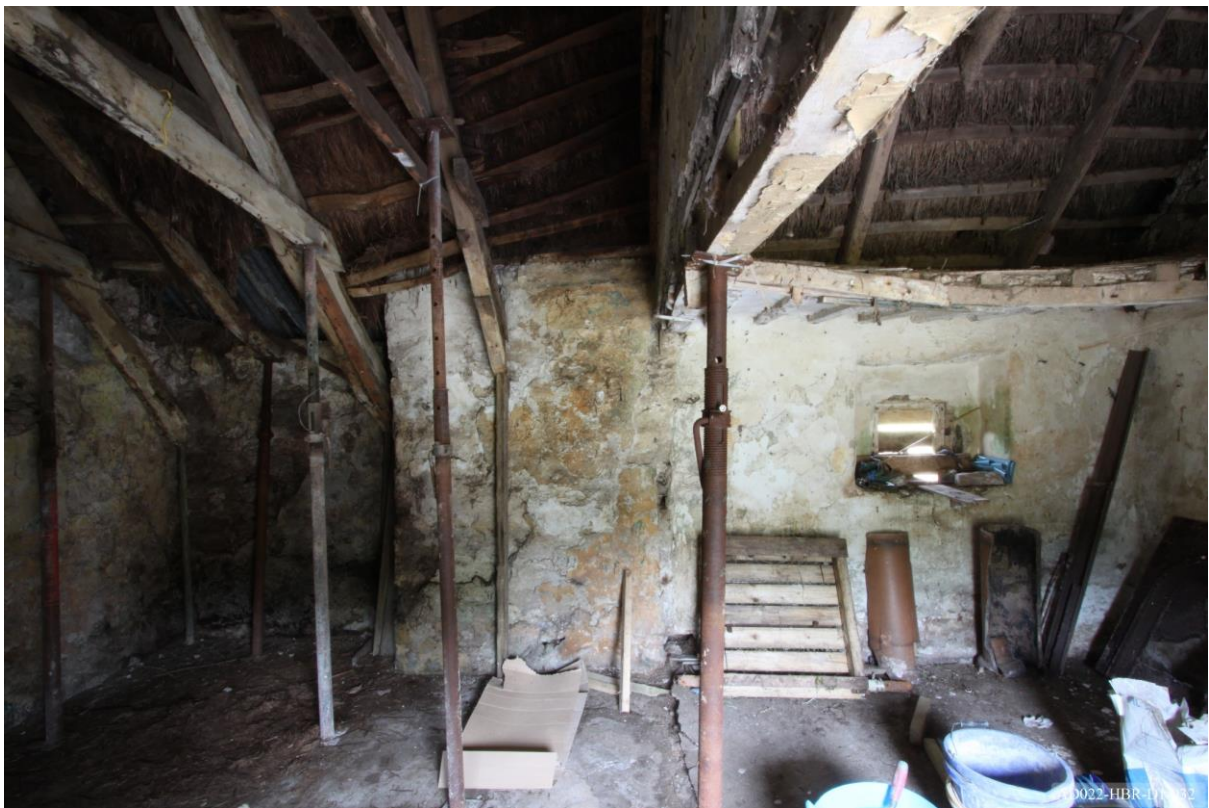
Plate 32 – View towards west of cottage, showing outshut and pantry window.
