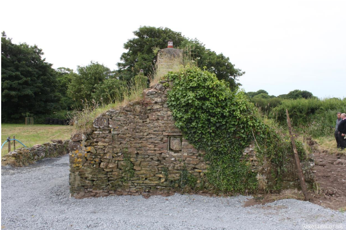
Plate 6 – North elevation of homestead building.
