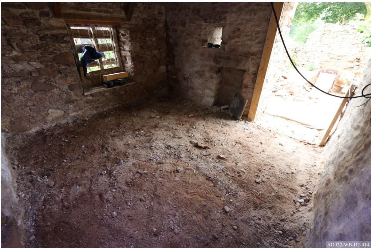
Plate 150 – Internal excavation, showing extension after removal of cement floor (201).
