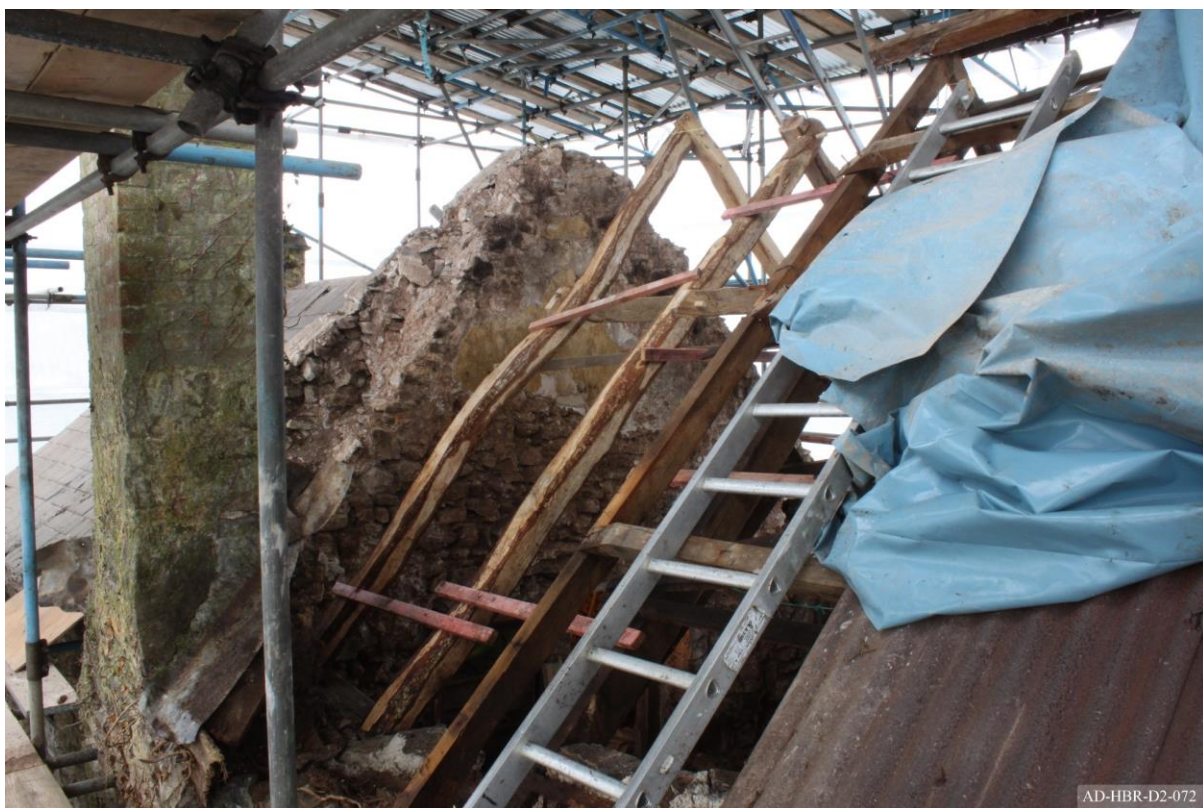
Plate 72 – View towards south-west of cottage, showing new trusses to south end.
