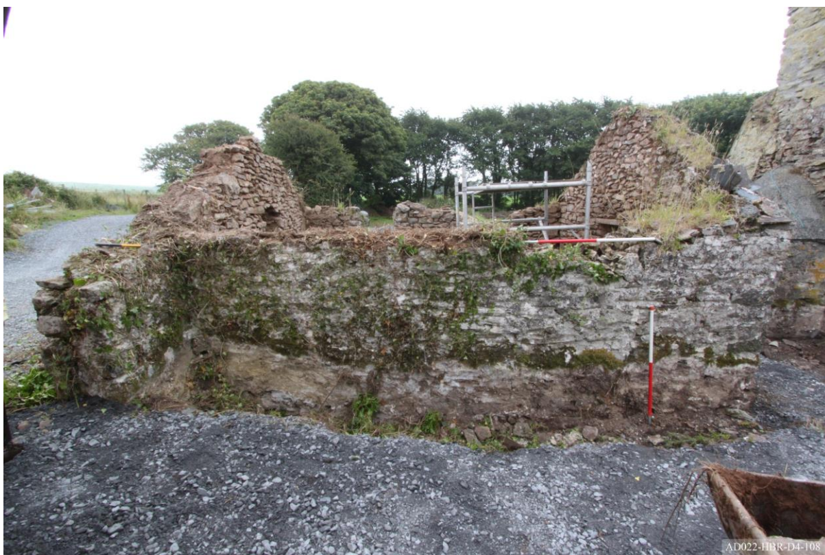
Plate 108 – View of west elevation of HB1.
