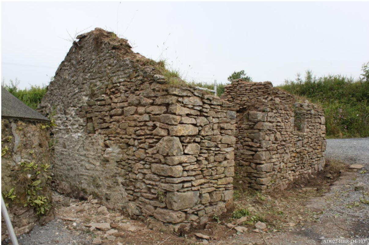
Plate 103 – View of east and south elevation of HB1.
