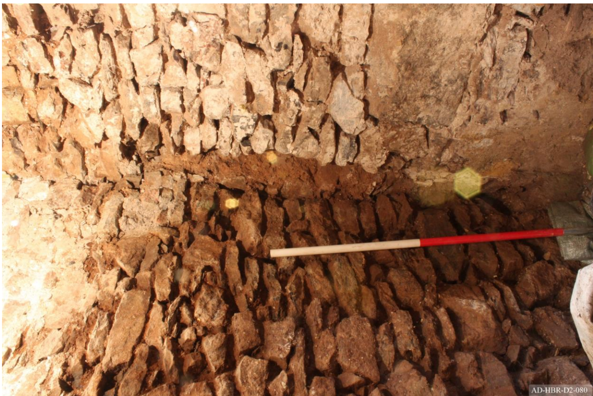
Plate 80 – View towards north-east of extension, showing small remaining element of earlier building.
