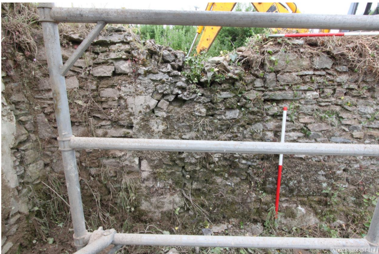
Plate 114 – View west of HB1, showing blocked doorway.
