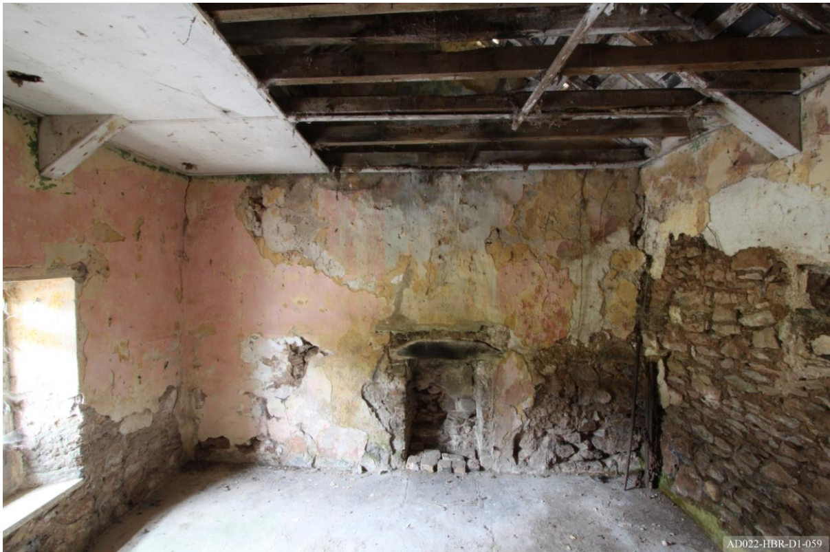
Plate 59 – View towards south of extension, showing fireplace.
