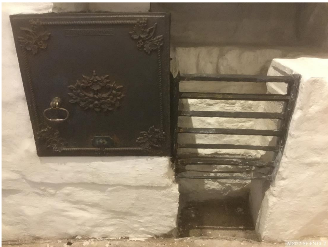
Plate 163 – Cast iron oven door refurnished and back in situ . FN10.
