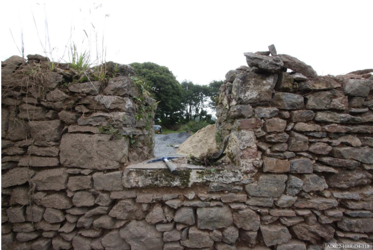
Plate 118 – View towards east of HB1, showing window reveals.
