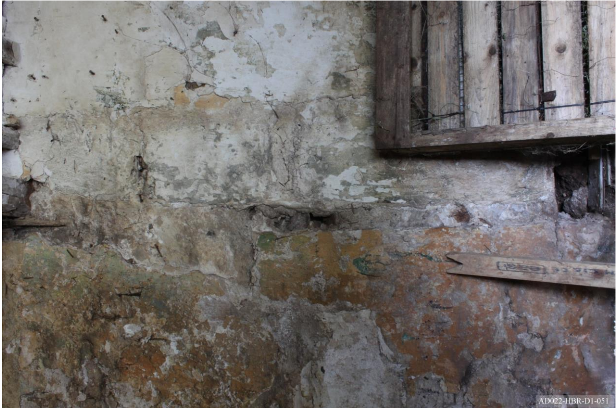
Plate 51 – View towards west of cottage, showing plaster of former partition.
