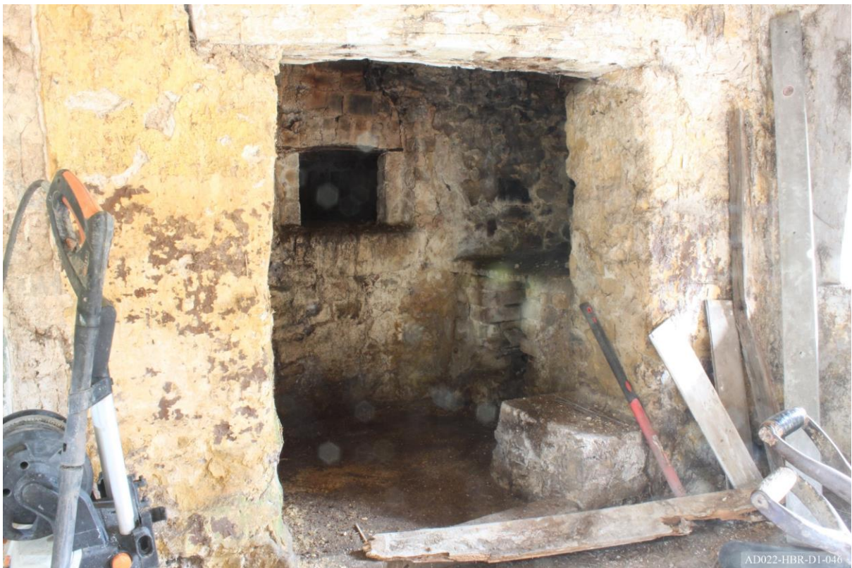
Plate 46 – View towards north of cottage, showing fireplace and bread oven.
