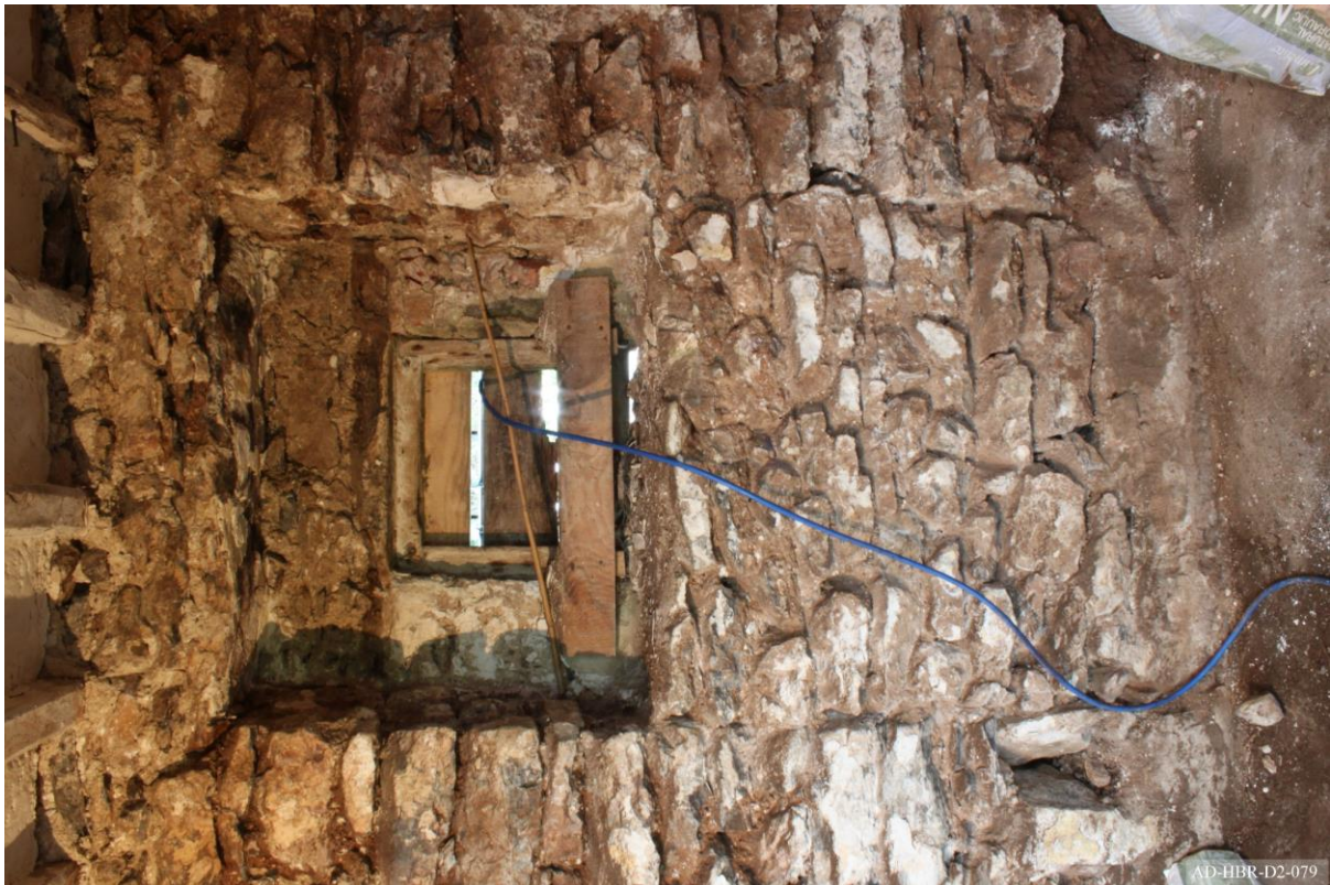
Plate 79 – View towards west of cottage, showing clear blocking of earlier doorway.
