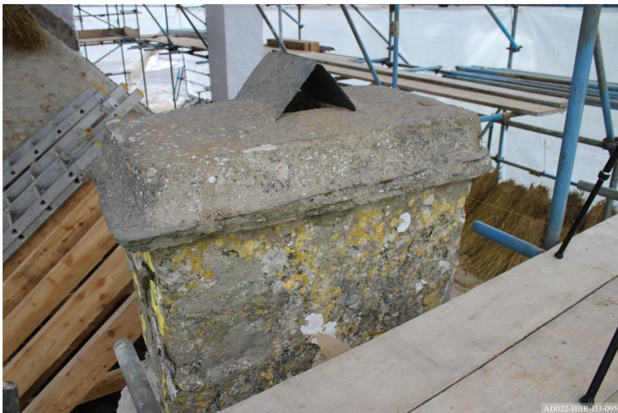
Plate 95 – View towards north-east, showing south elevation of chimney prior to dismantling.
