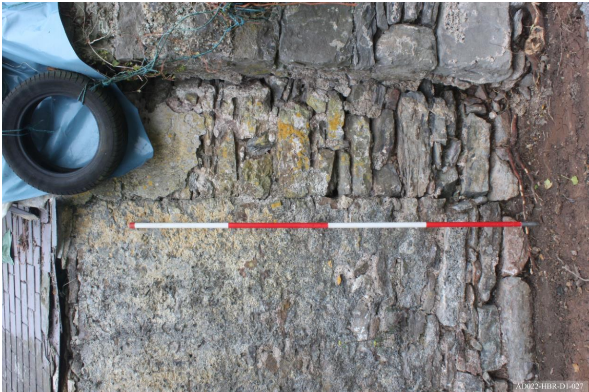
Plate 27 – View of east elevation, showing joint between cottage and extension.
