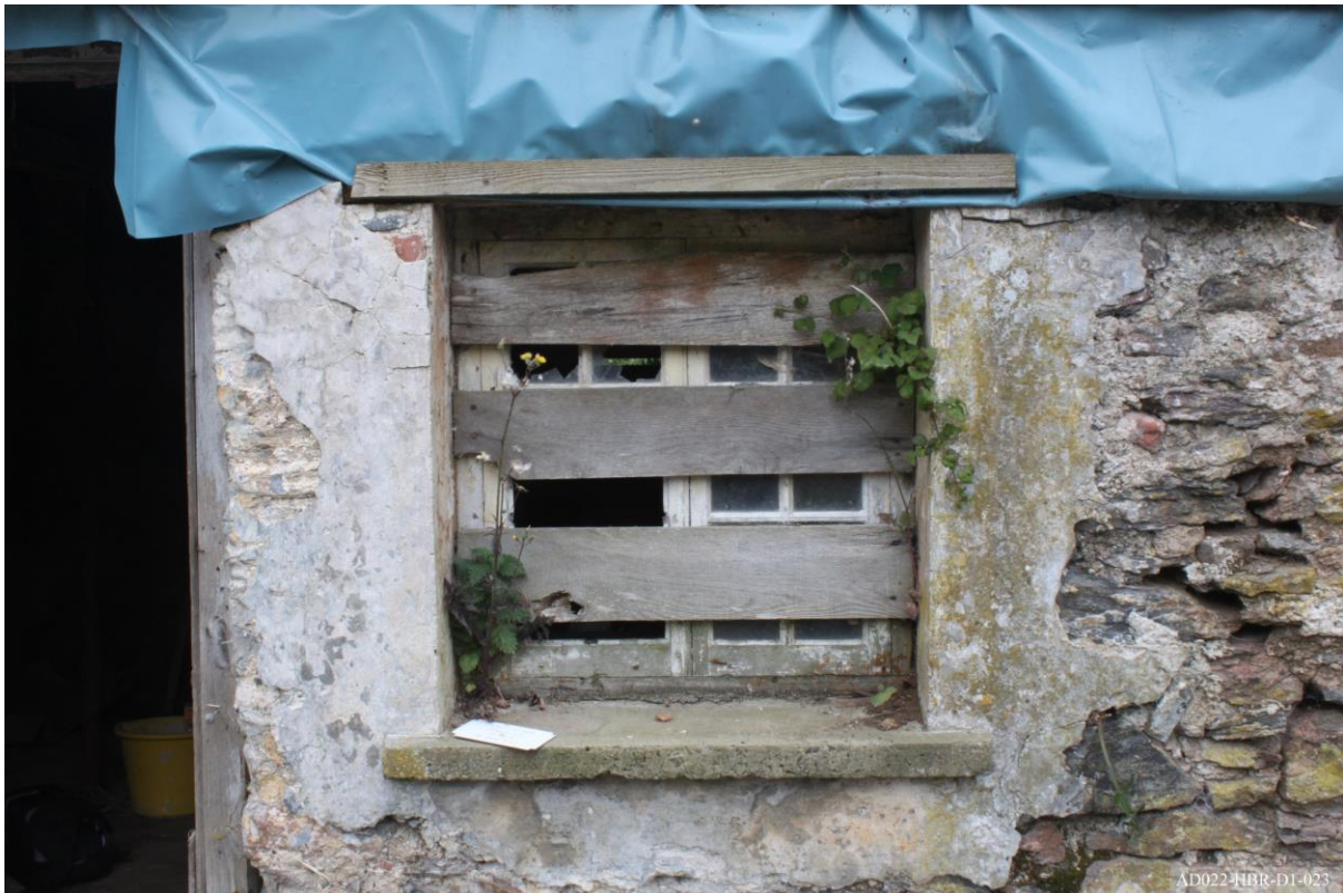
Plate 23 – View of east elevation, showing north window of cottage.
