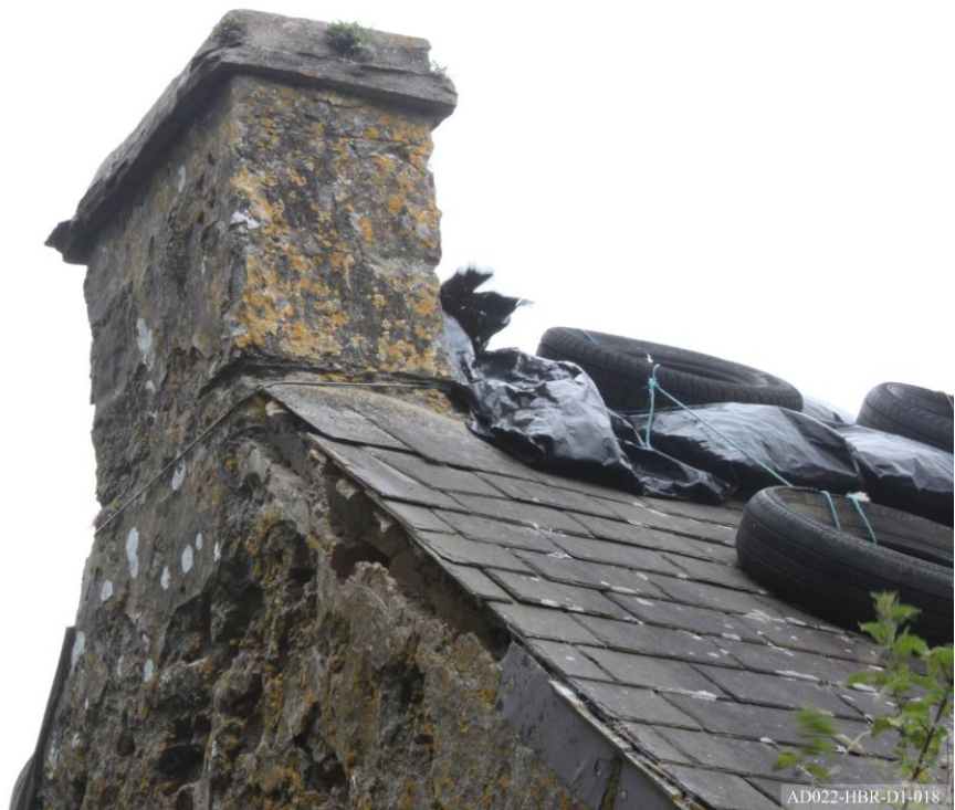
Plate 18 – View towards west, showing chimney stack to south elevation of extension.
