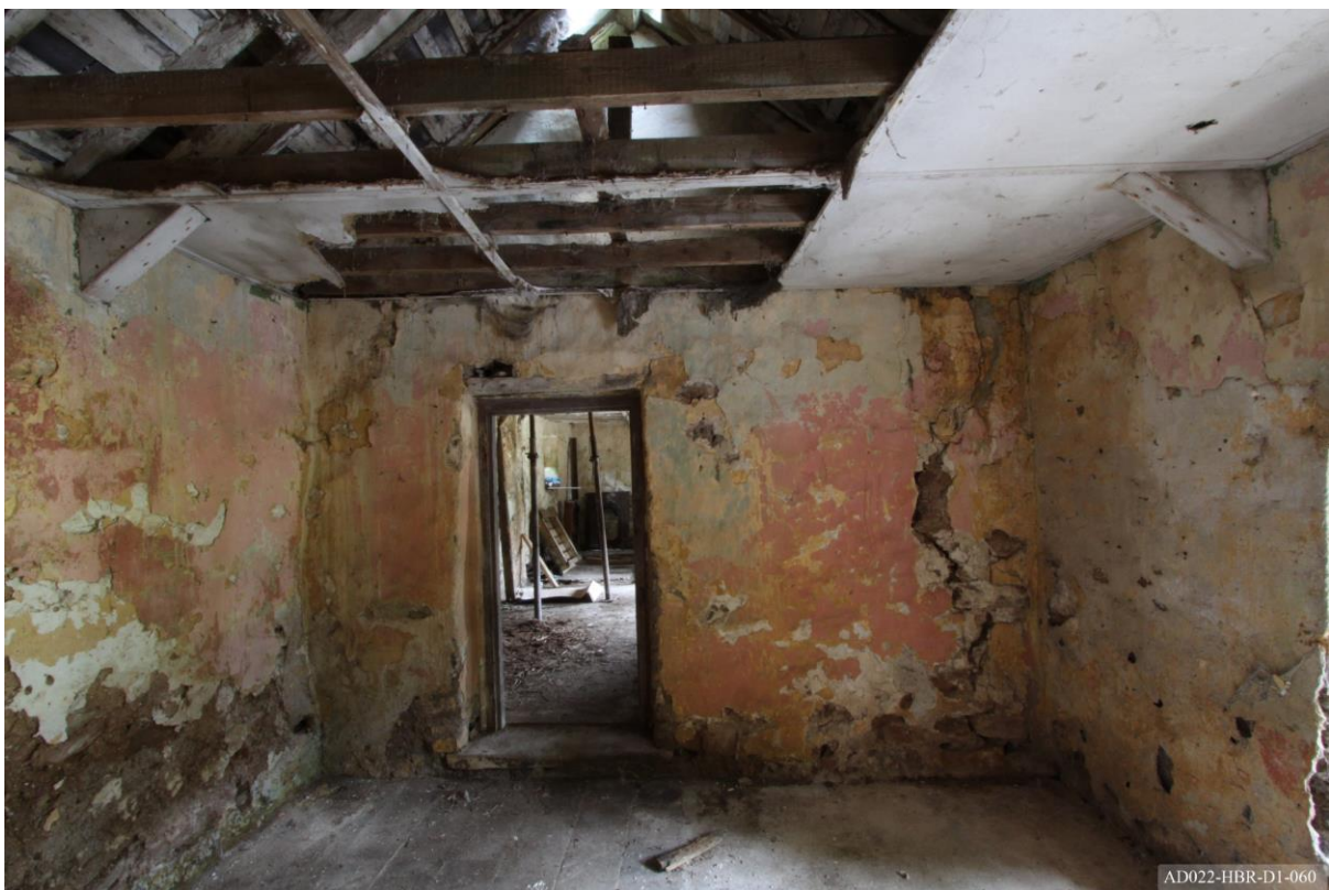
Plate 60 – View towards north of extension, showing doorway to cottage.
