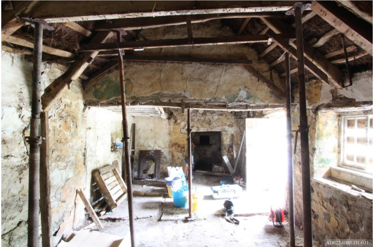
Plate 31 – View towards north of cottage, showing partition truss.
