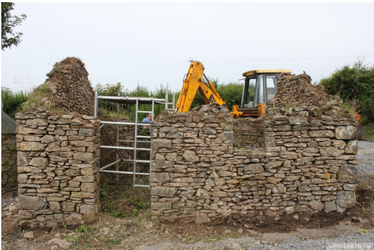
Plate 104 – View of east elevation of HB1.
