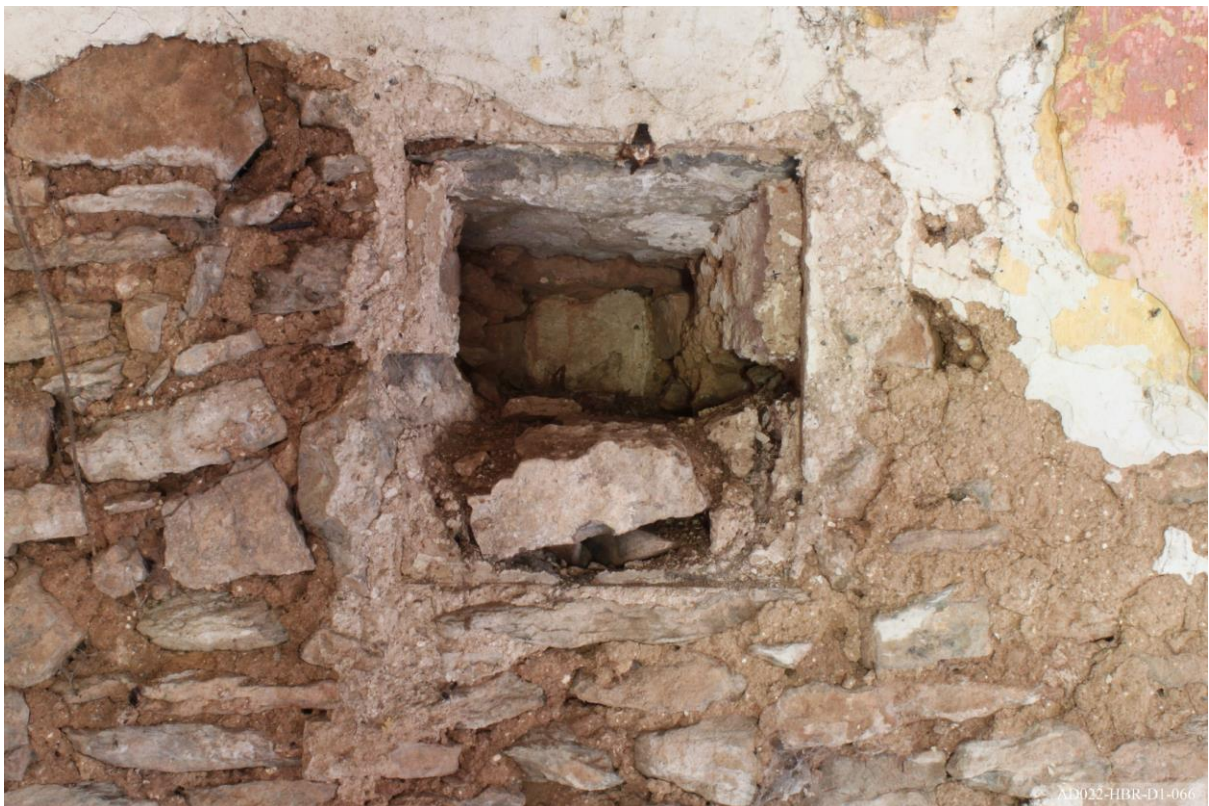
Plate 66 – View towards west of extension, showing detail of ventilation slit.
