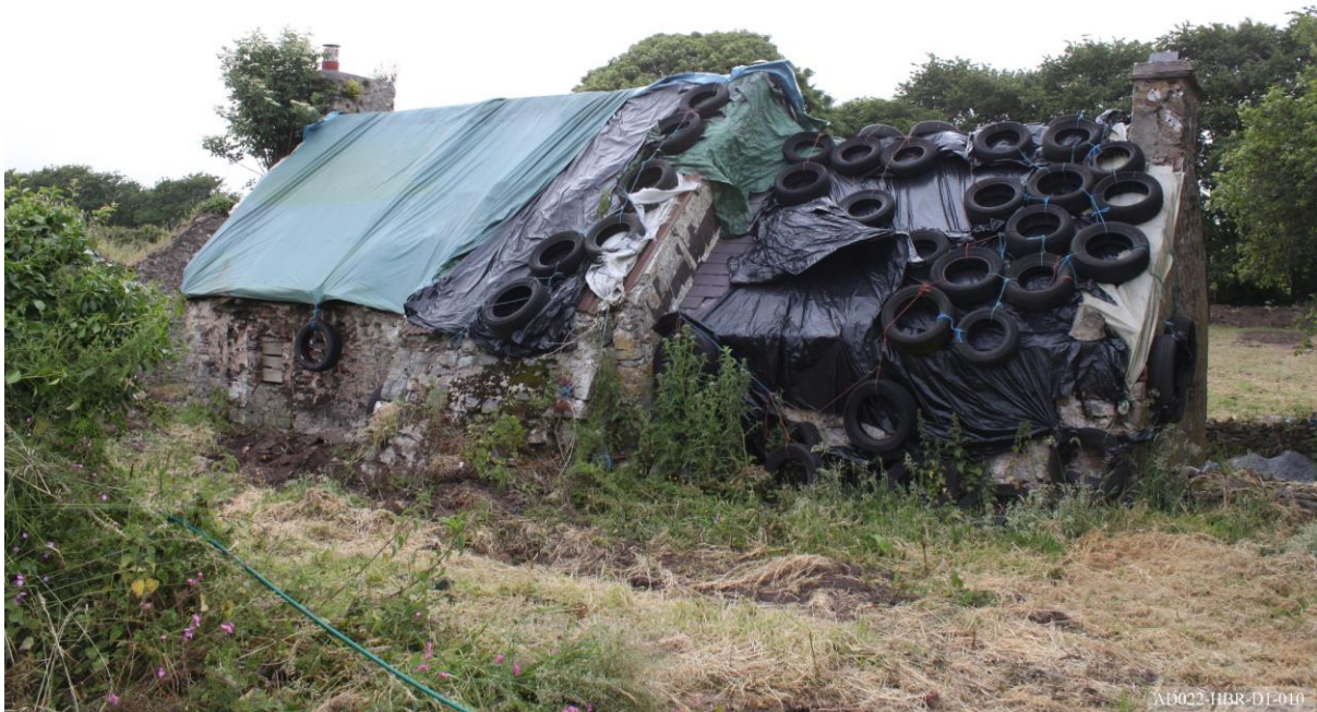
Plate 10 – View towards the north-east, showing the cottage (left) and extension (right).
