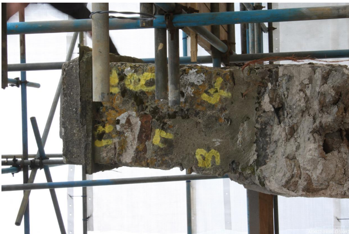
Plate 92 – View towards east, showing west elevation of chimney prior to dismantling.
