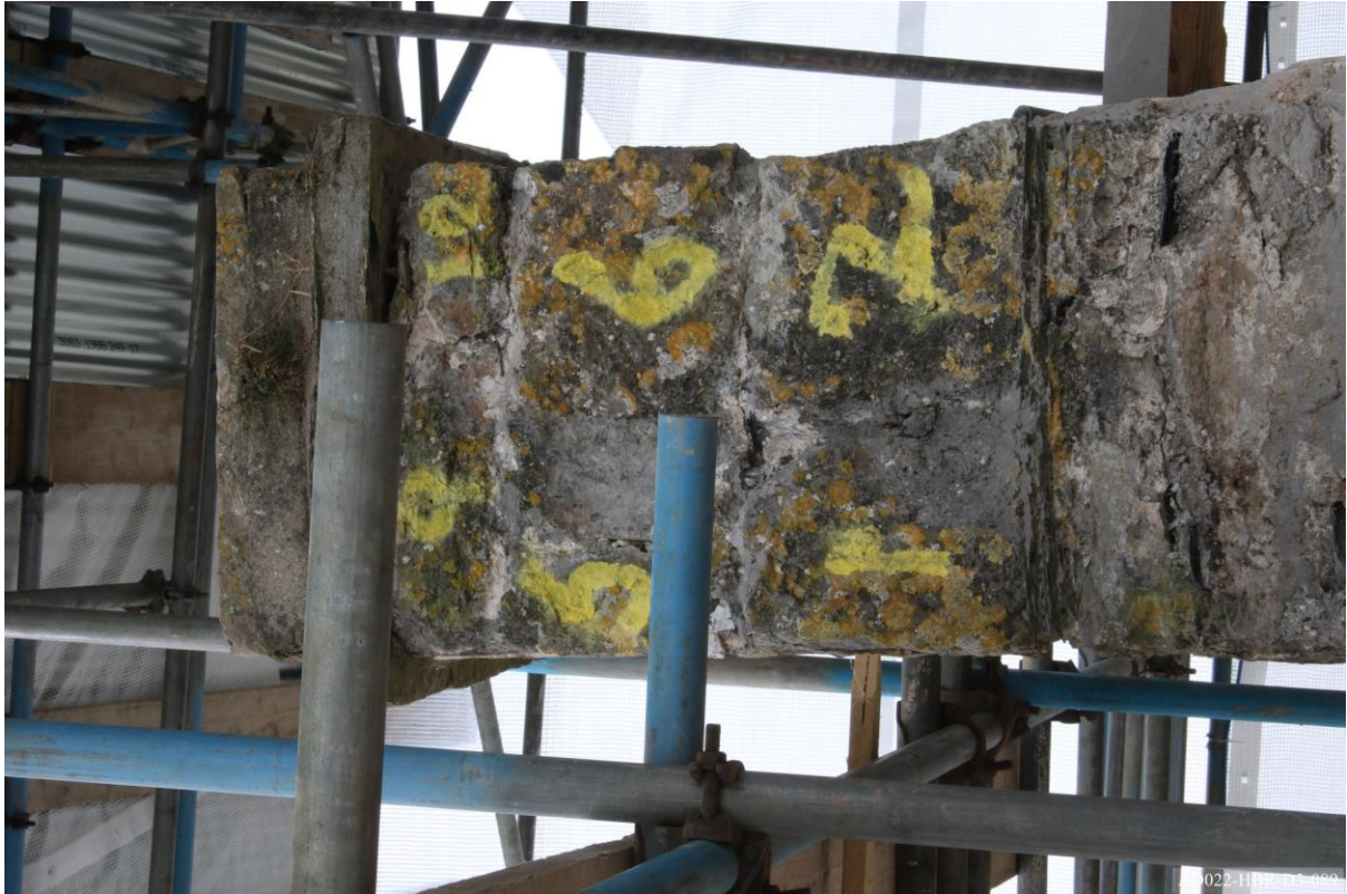
Plate 89 – View towards west, showing east elevation of chimney prior to dismantling.
