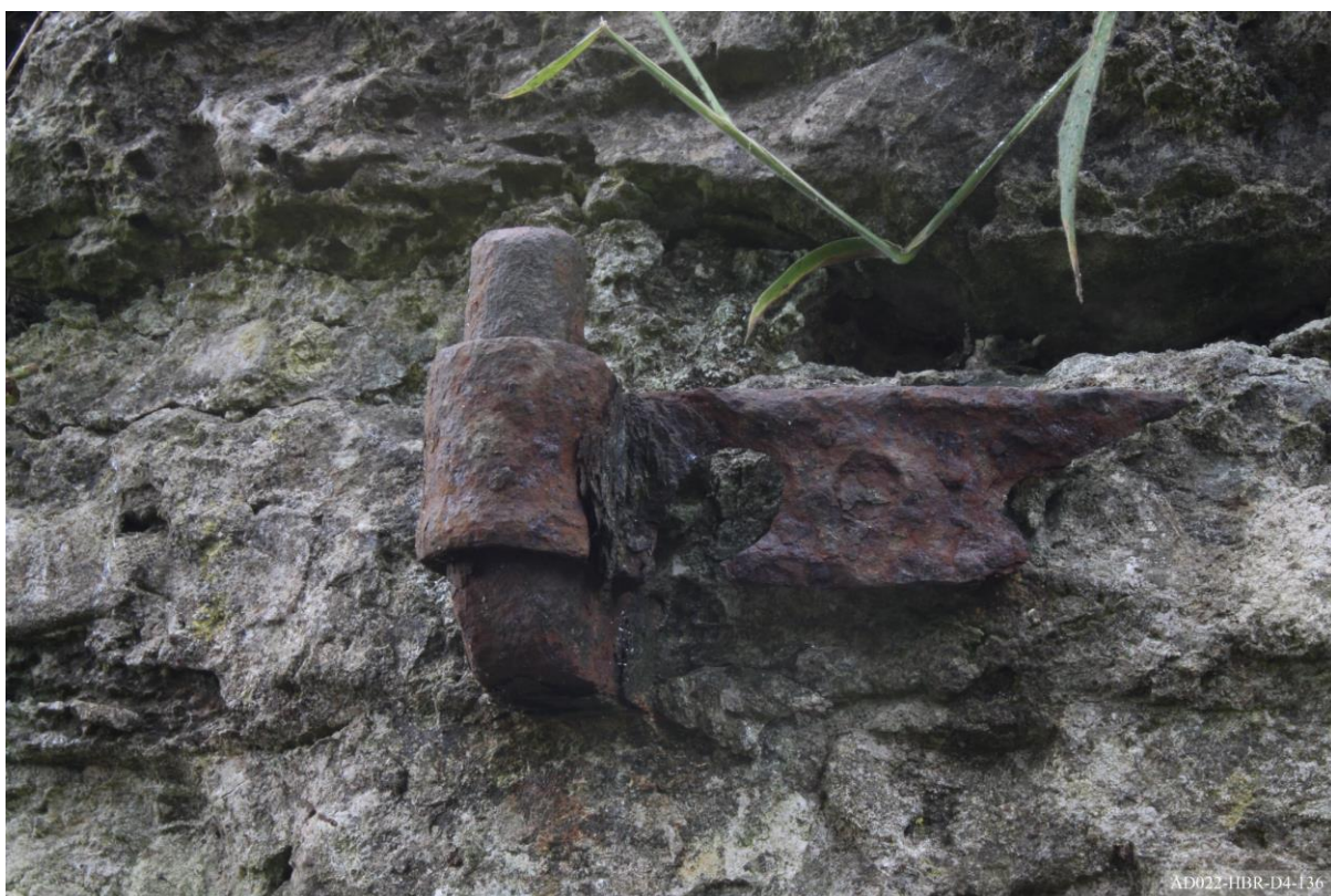
Plate 136 – Iron pintle with remaining strap hinge to pigsty entrance.
