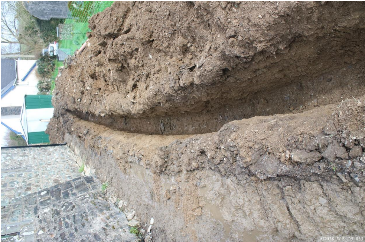
Plate 33 – Service trench to south of church.
