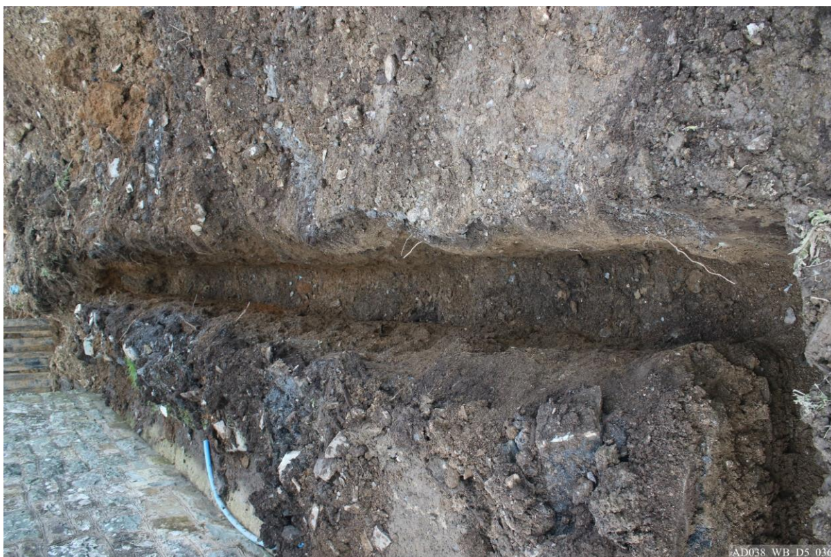
Plate 36 – Service trench to north east of church.
