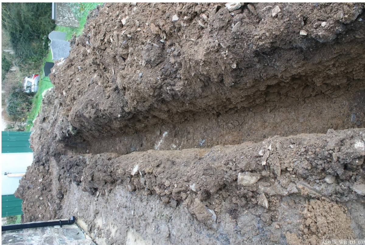
Plate 35 – Service trench to south of church.
