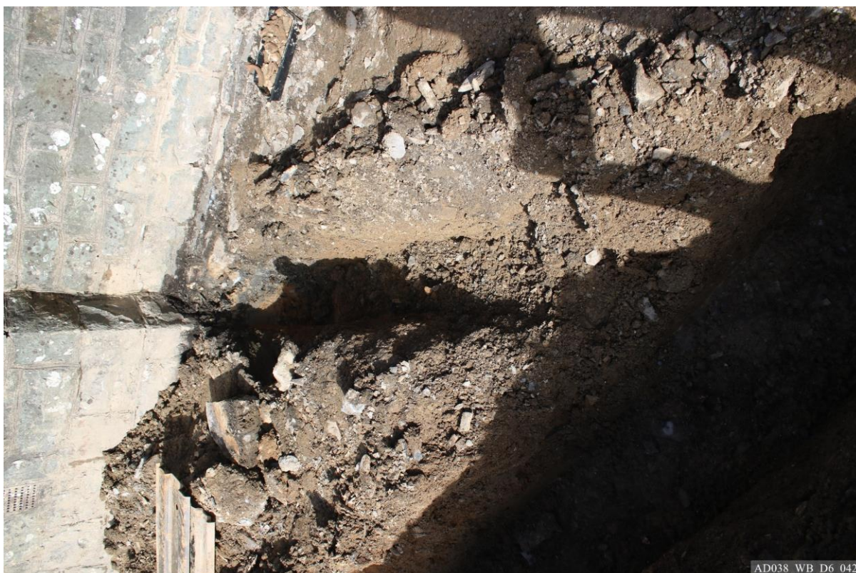
Plate 42 – Service trench to west of church.
