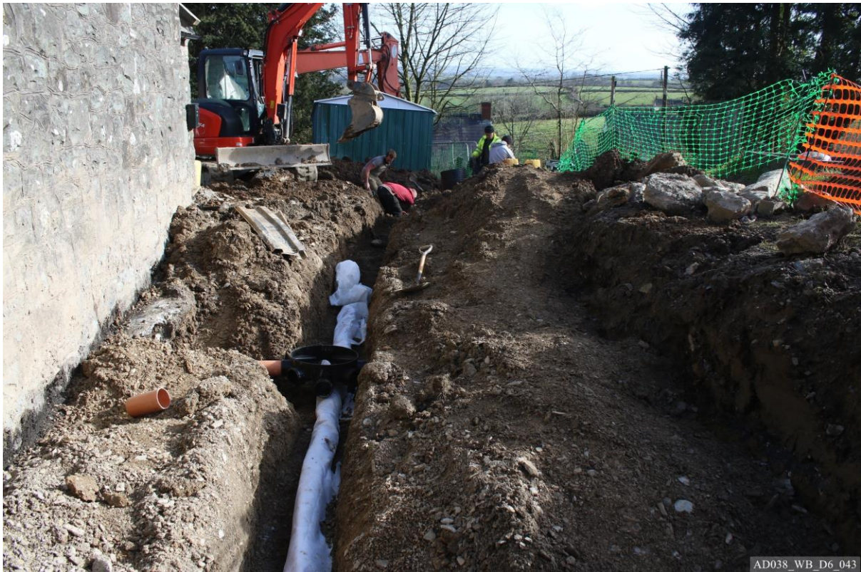
Plate 43 – Service trench to west of church.
