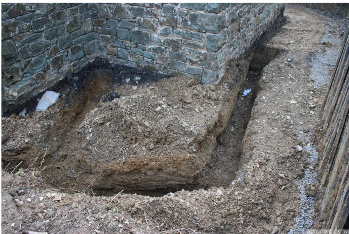
Plate 38 – Service trench to north-east of church.
