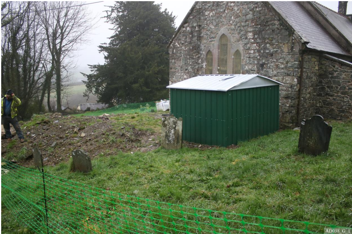
Plate 50 – View south-west, showing gravestones to be removed (G1-4).
