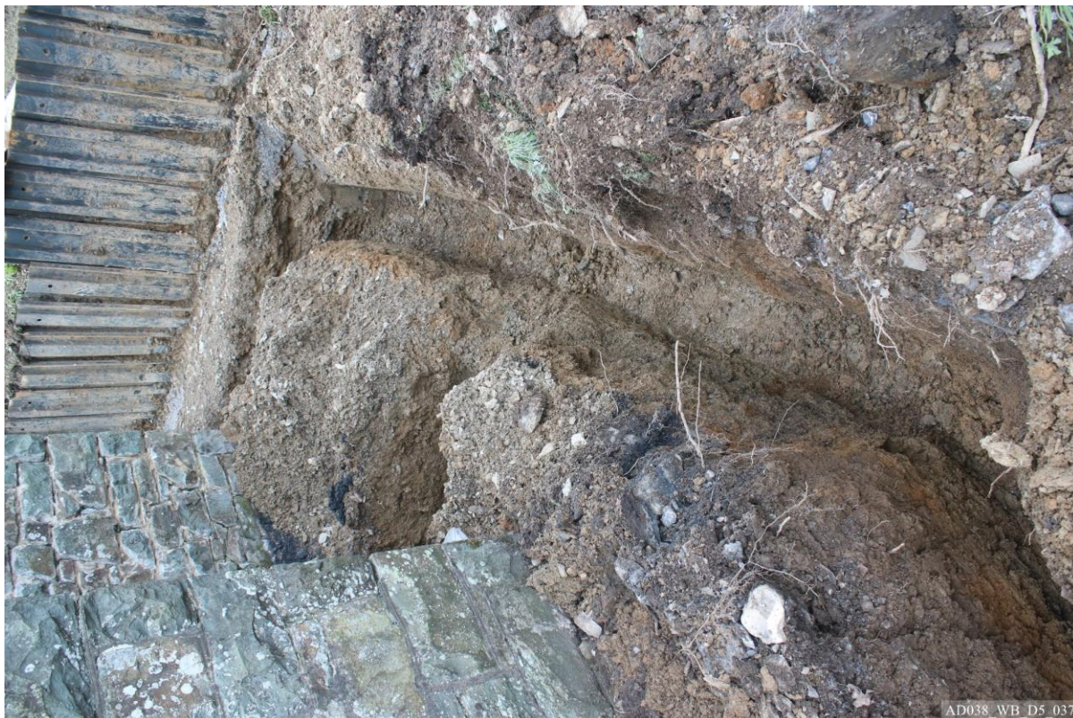
Plate 37 – Service trench to north-east of church.
