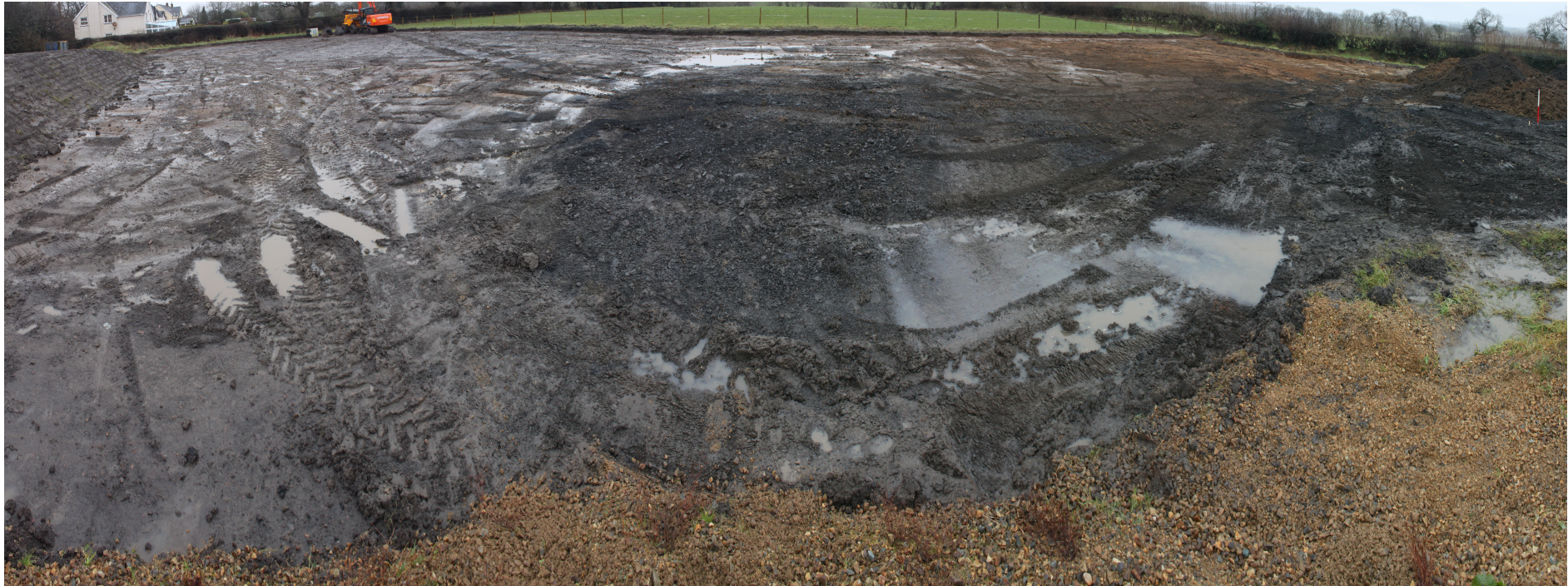
Plate 1 - Overview of stripped area.
