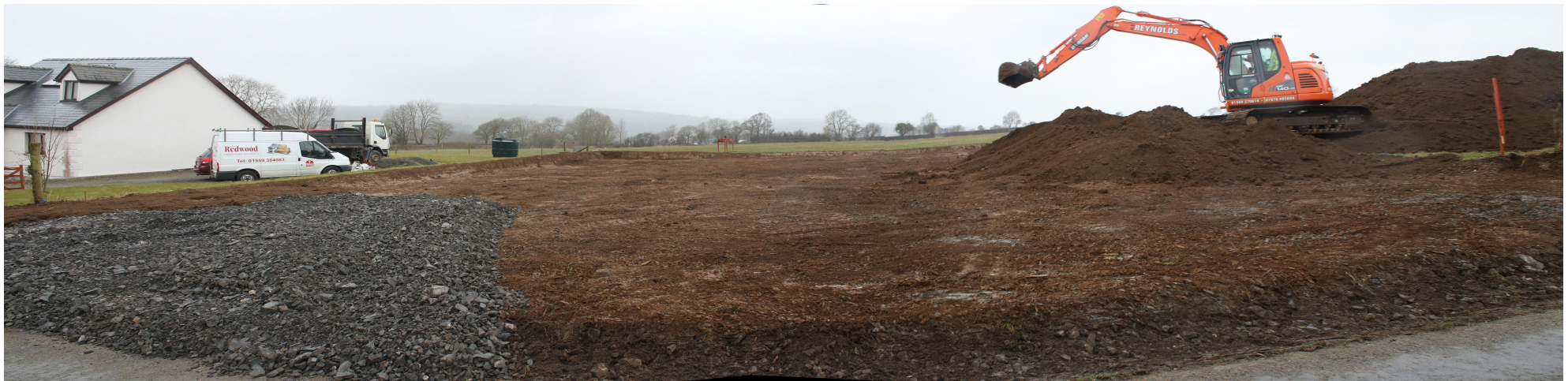
Plate 1 - ADo47_001 - Site Panorama, viewed north.
