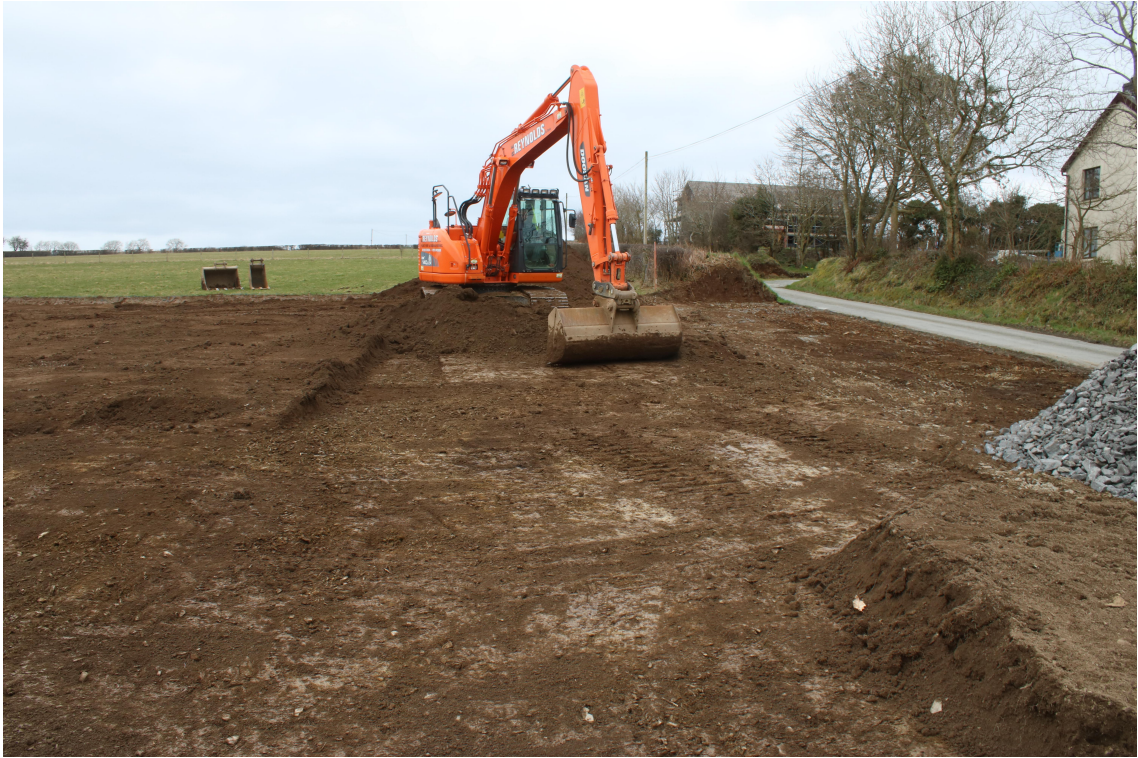
Plate 2 - ADo47_002 - Site stripping and bunt deposit 103 , viewed north-east.
