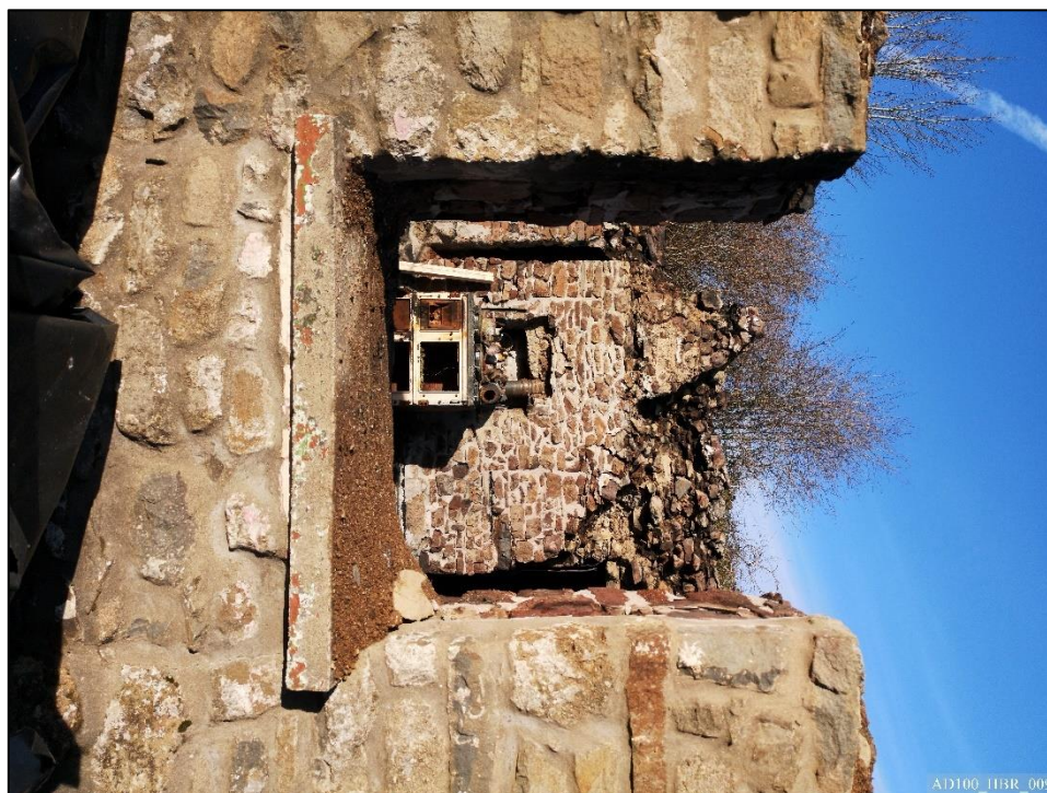
Plate 9 East elevation, showing window formed from 18 th century doorway.
