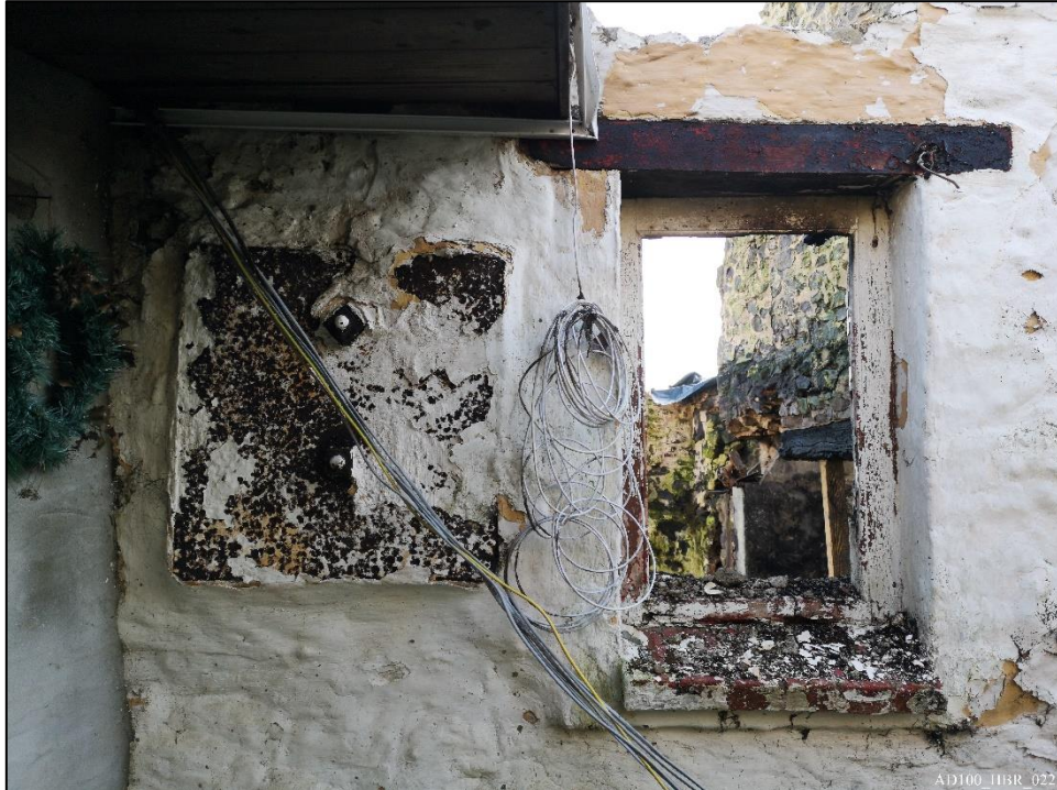
Plate 22 – West elevation, showing wall tie plate.
