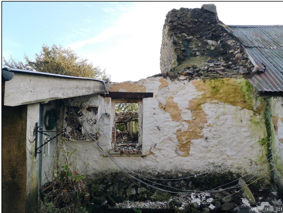
Plate 21 – West Elevation, showing window and wall tie plate.
