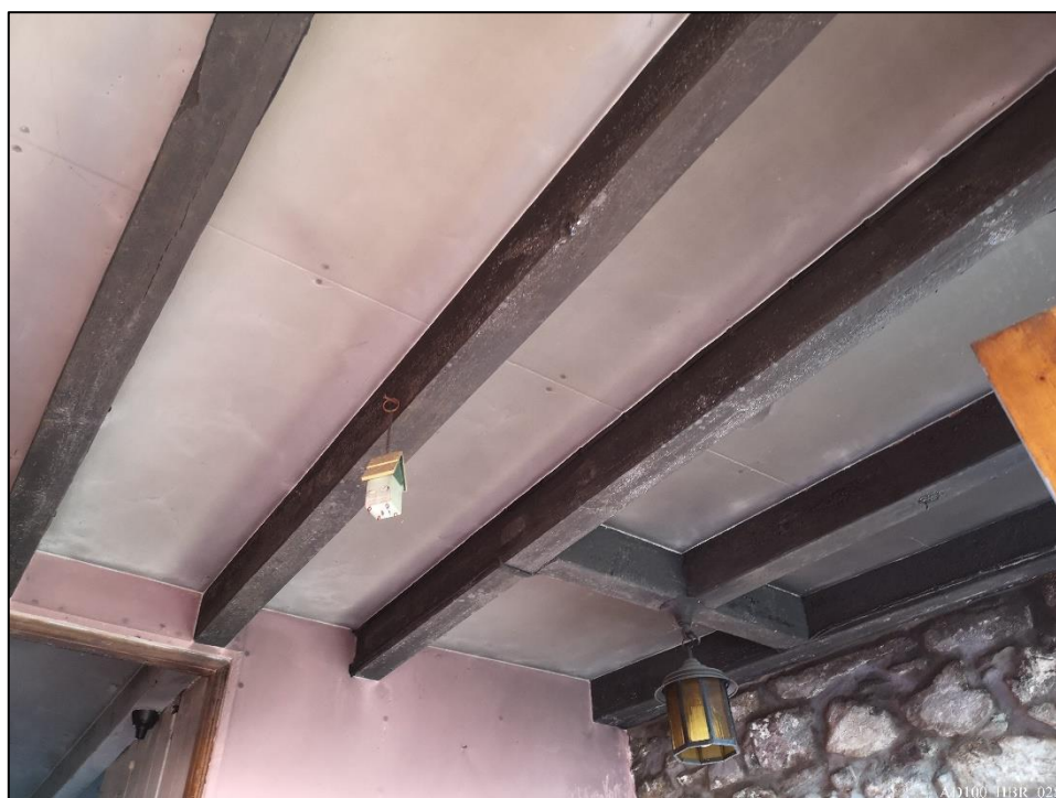
Plate 28 – Lobby, showing ceiling with trimmer for a former stair.
