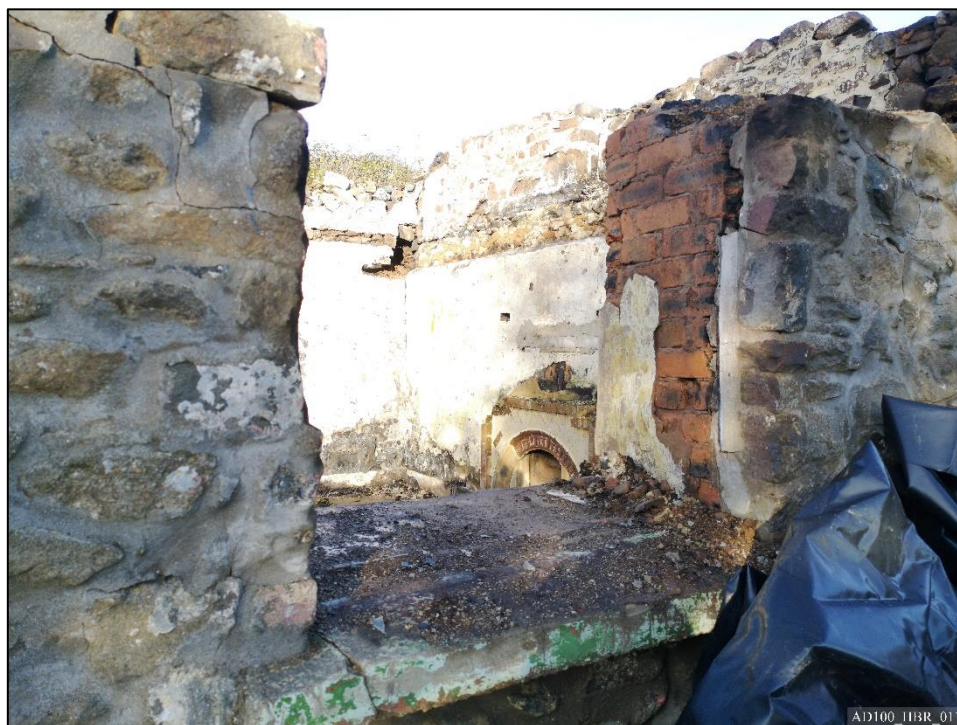
Plate 11 – East elevation showing enlarged window to parlour.
