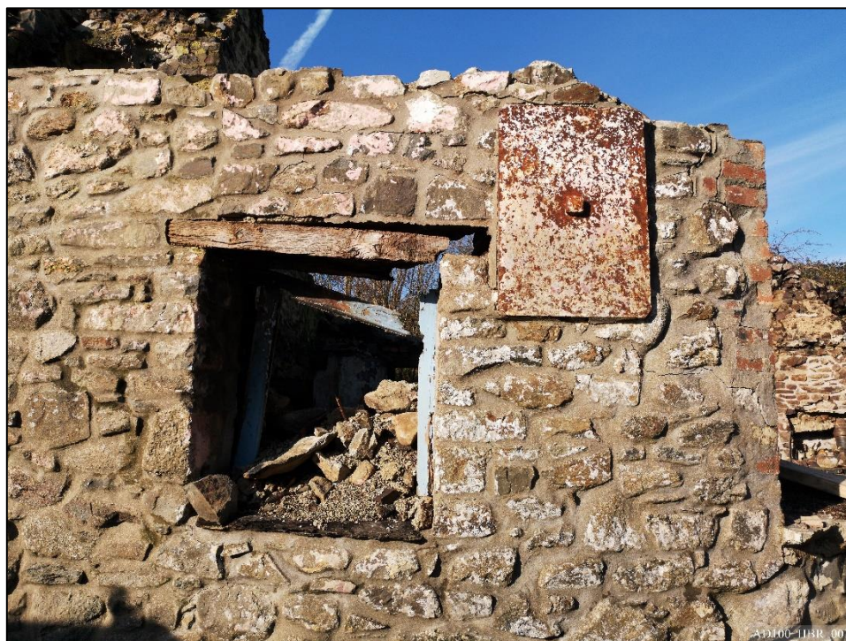
Plate 7 – East elevation, showing tie plate to stair projection.
