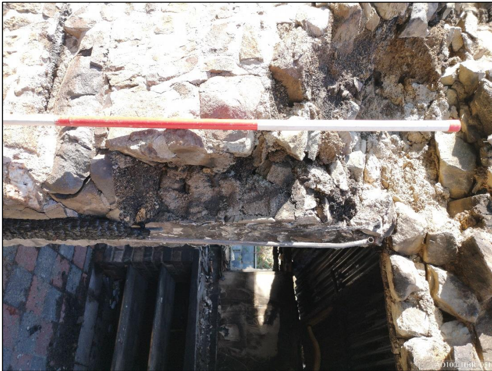
Plate 51 – Cruck pocket for T4 to west lateral wall.
