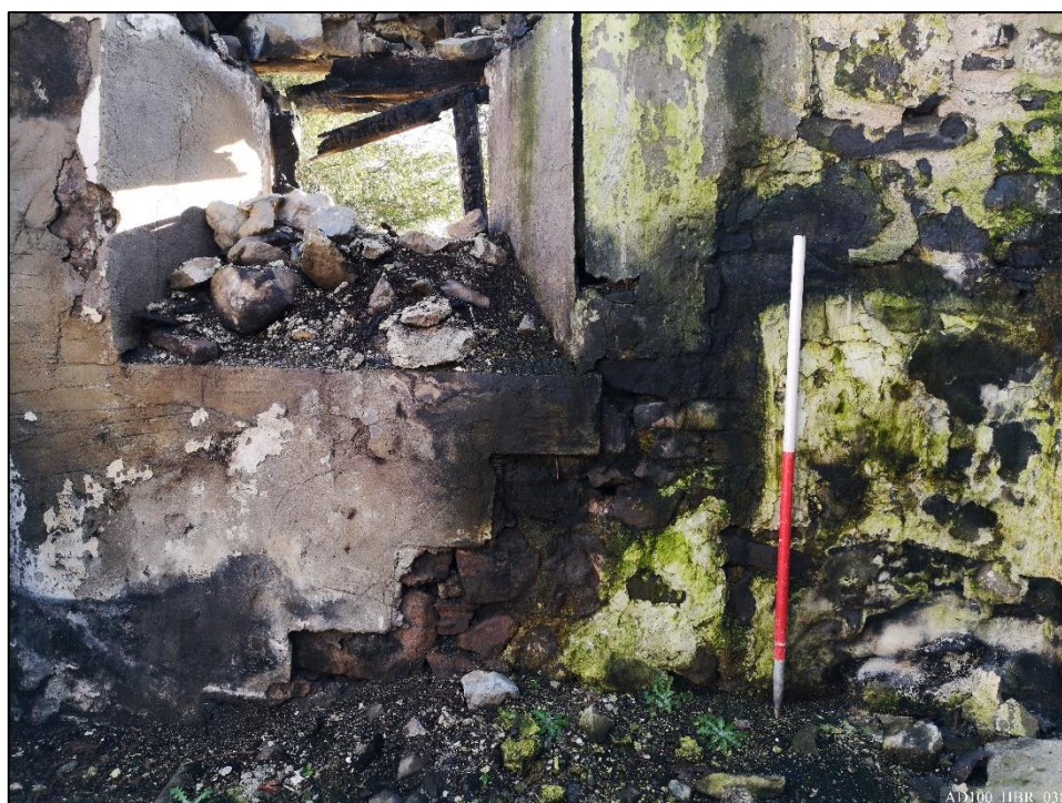
Plate 38 – Plaster marks to stair projection, showing treads and risers.
