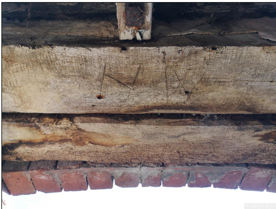
Plate 75 – Inscribed initials to reused timber to north window in east elevation of byre.
