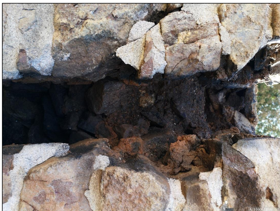
Plate 54 – View inside cruck pocket, showing clay-earth mortar.
