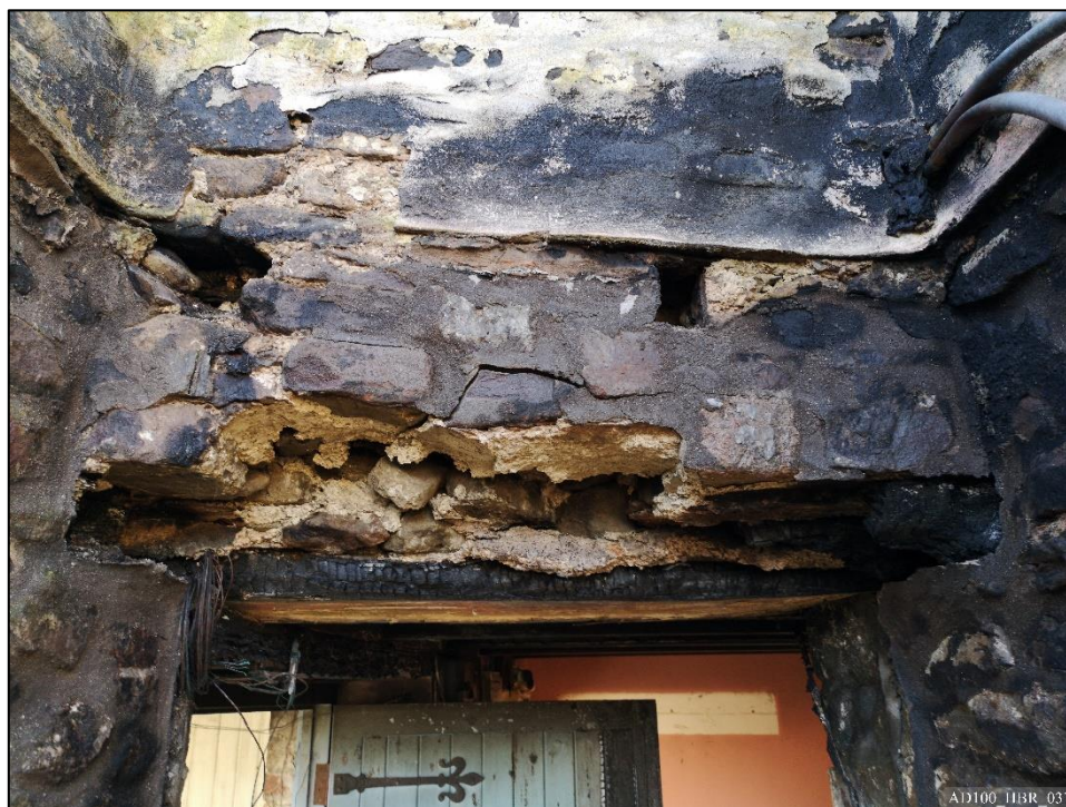
Plate 37 – Joist pockets, showing level of first floor over doorway from byre.
