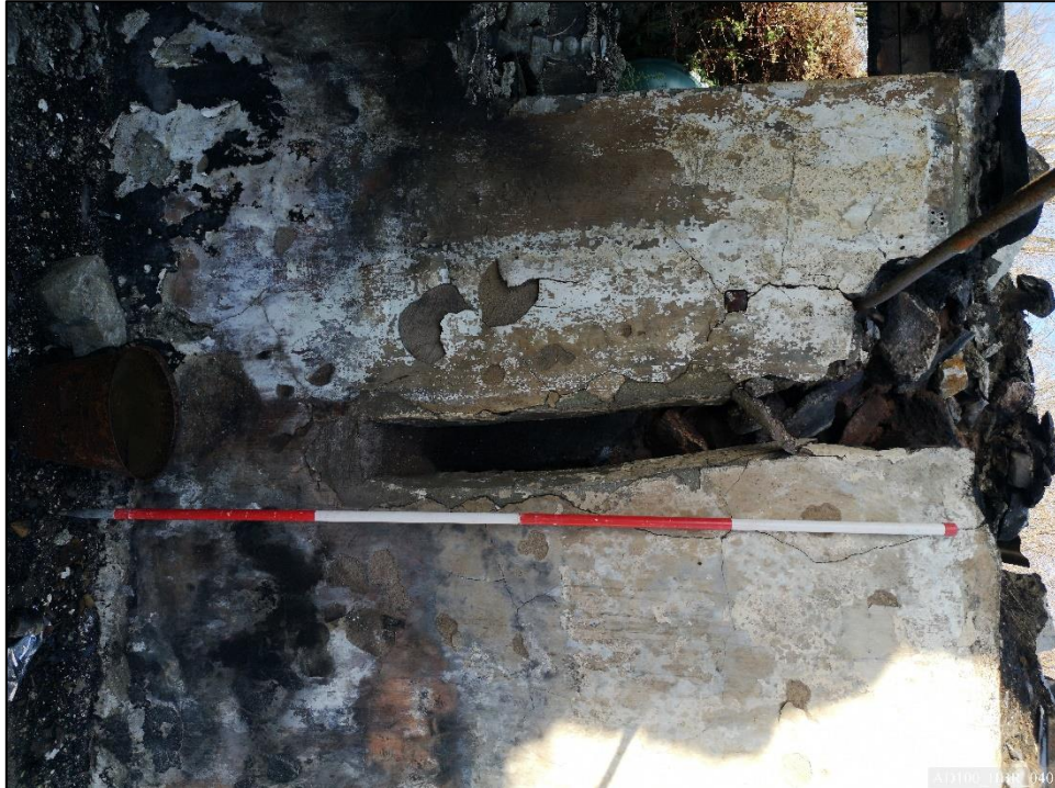
Plate 40 – Cruck pocket for T2 to west lateral wall.
