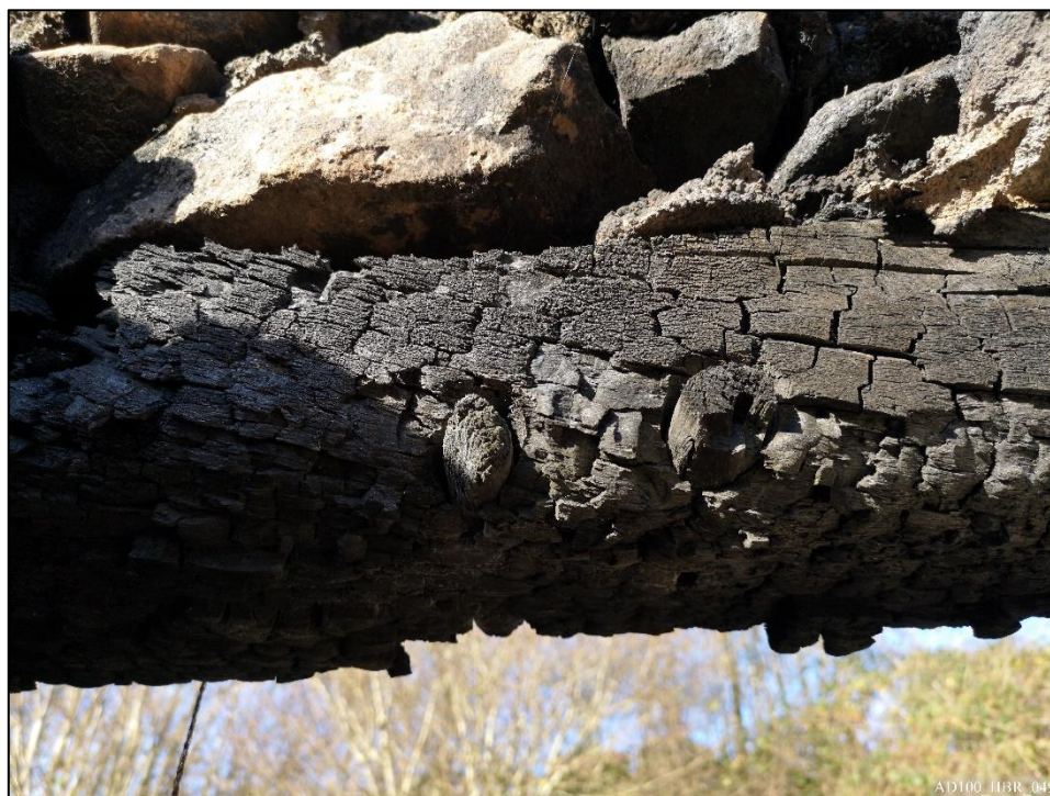
Plate 49 – Reused timber lintel, showing pegs in situ.
