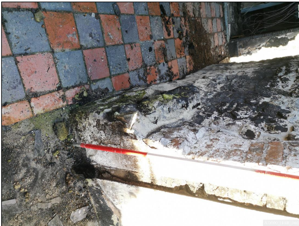
Plate 66 – Detail showing plinth to west lateral wall, demonstrating original thickness of Phase I.
