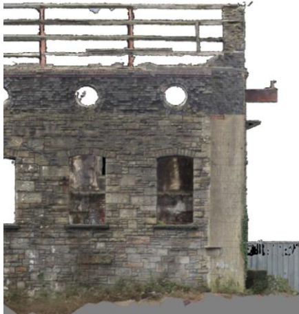
North West external elevation
