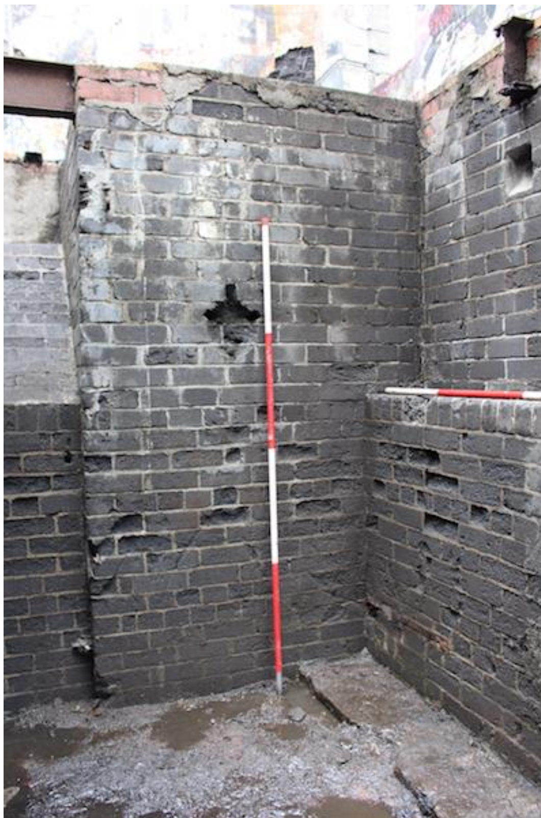
Plate 36. West-facing photo showing west wall of inspection platform [207].
