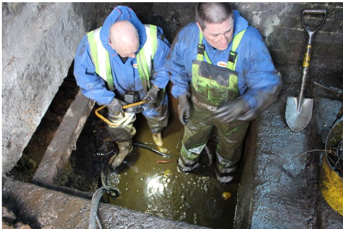
Plate 13. Working shot during the excavation of sump [103] showing water ingress.
