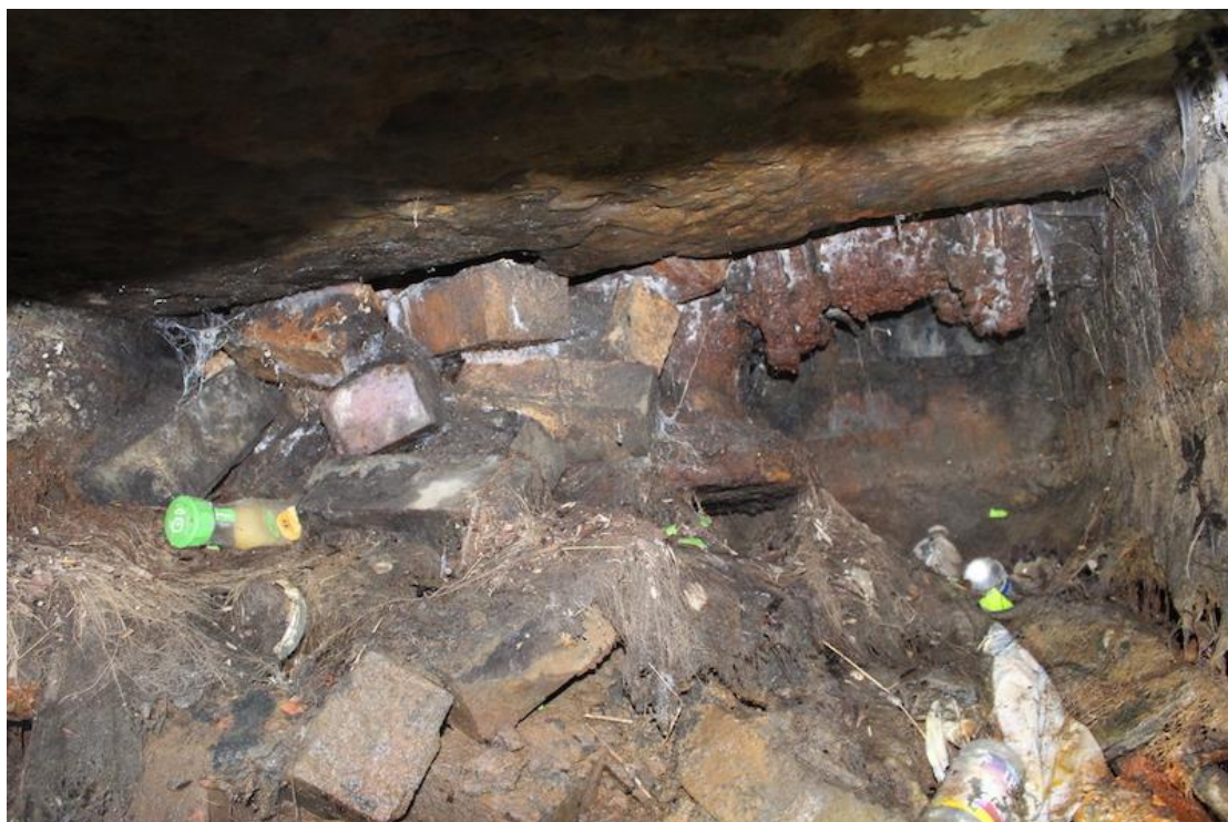
Plate 14. Working shot during the excavation of sump [103] showing the back wall and in situ pipe work. It also shows brick backfill (102).
