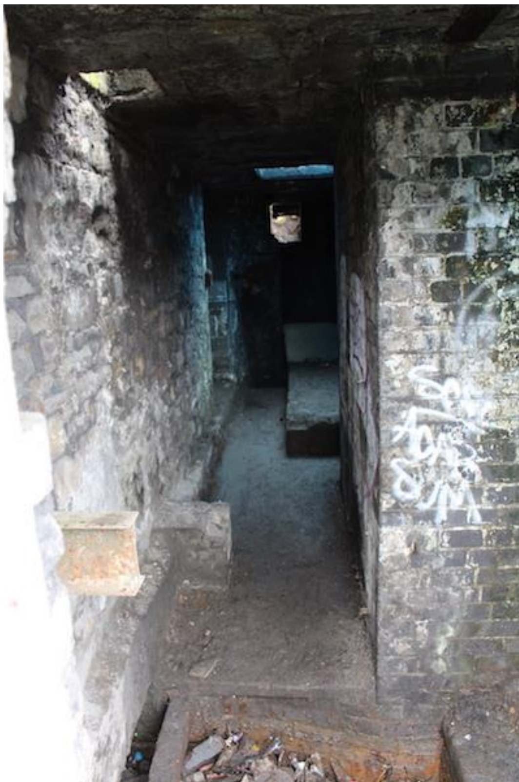
Plate 11. West facing post-excavation photo of main basement [105] showing sump [103] in foreground.
