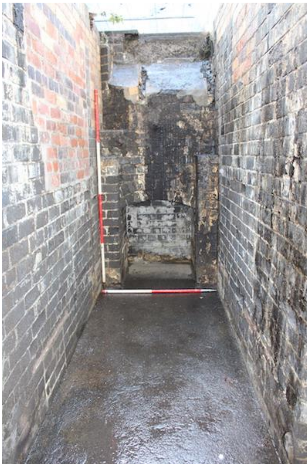
Plate 42. West-facing photo of stairwell [106] showing brick arched recess at base of stairwell and later inserted slots to carry stairs. Later red/ yellow brick infill in the north and south walls of the stairwell is also visible.
