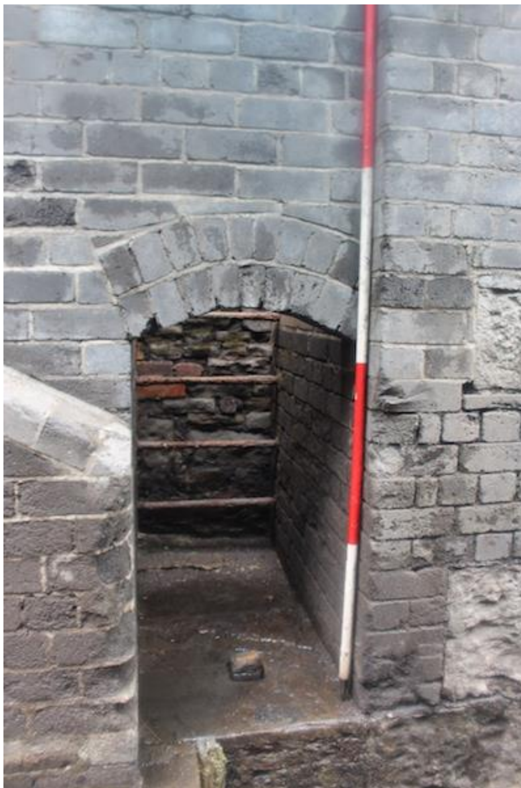
Plate 33. North-facing photo from inspection platform [207] showing access to manhole tunnel.
