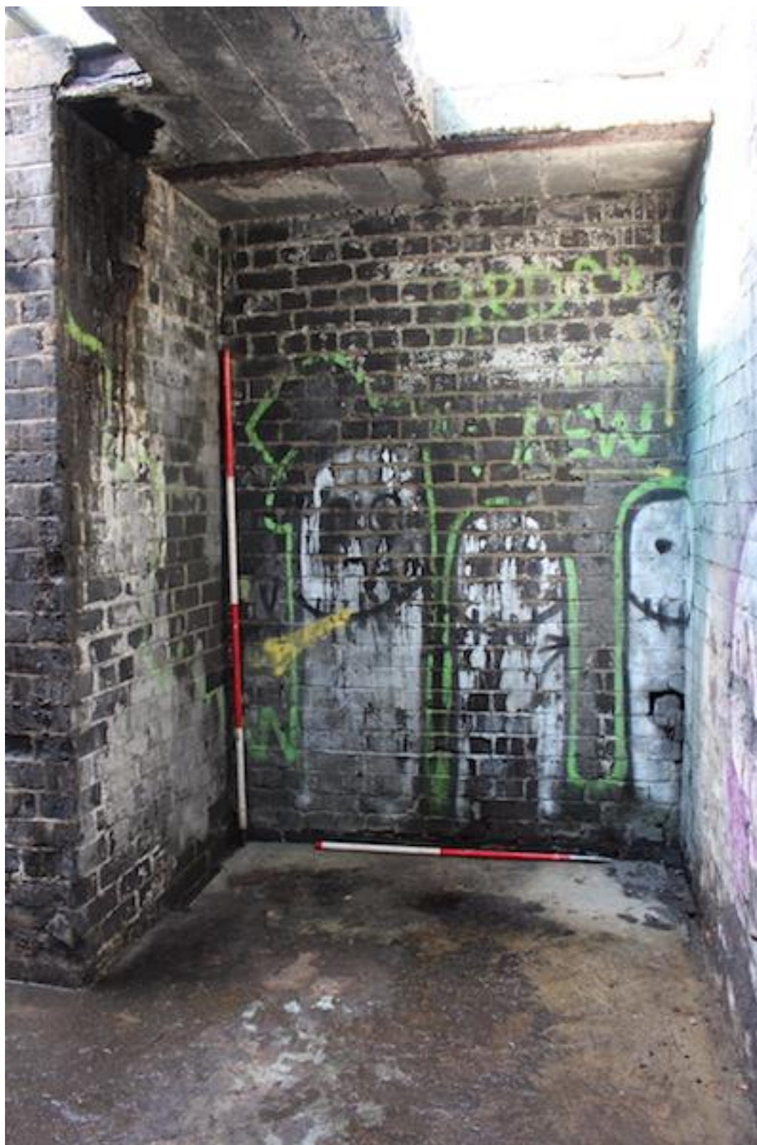
Plate 43. North-facing photo showing recessed north wall of stairwell [106].
