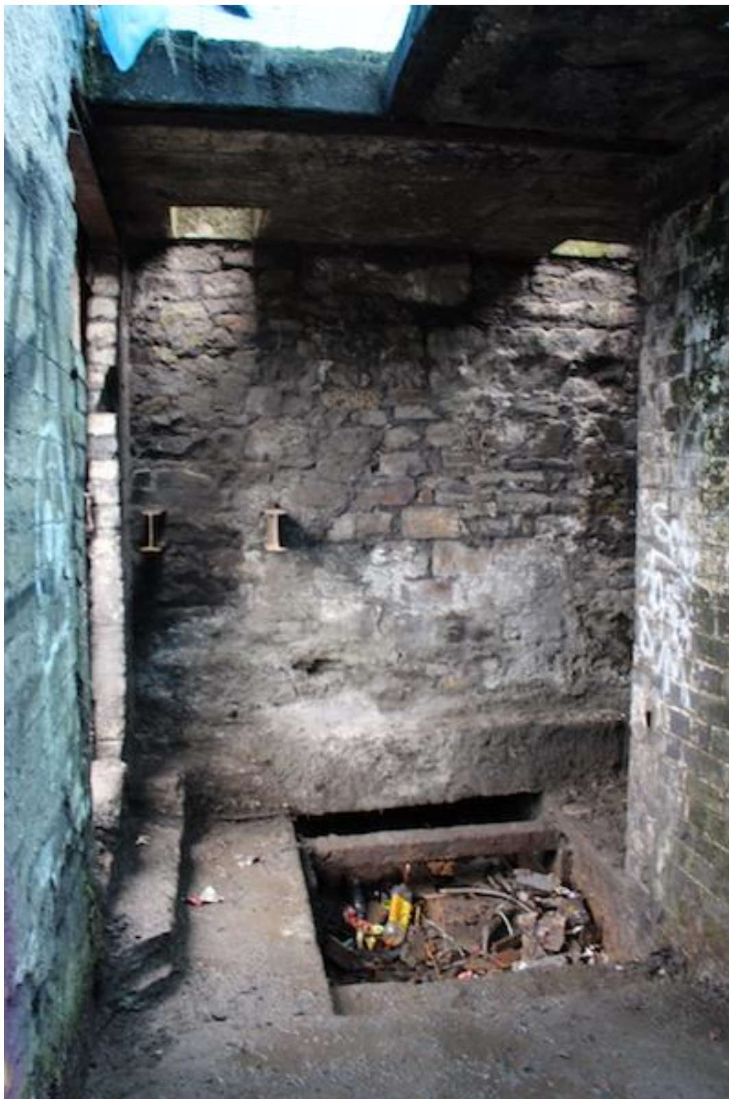
Plate 12. South facing post excavation photo of basement [105] showing sump [103].
