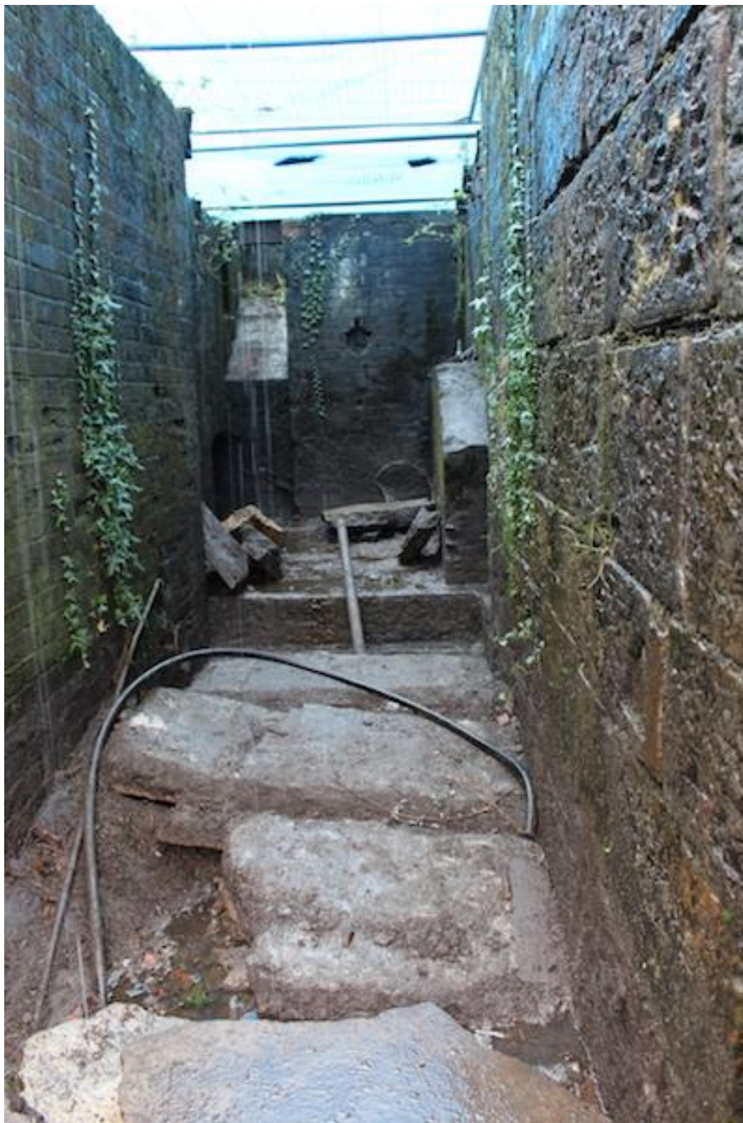
Plate 19. West facing photo showing re-deposited concrete slabs (202) within wheel pit [206].
