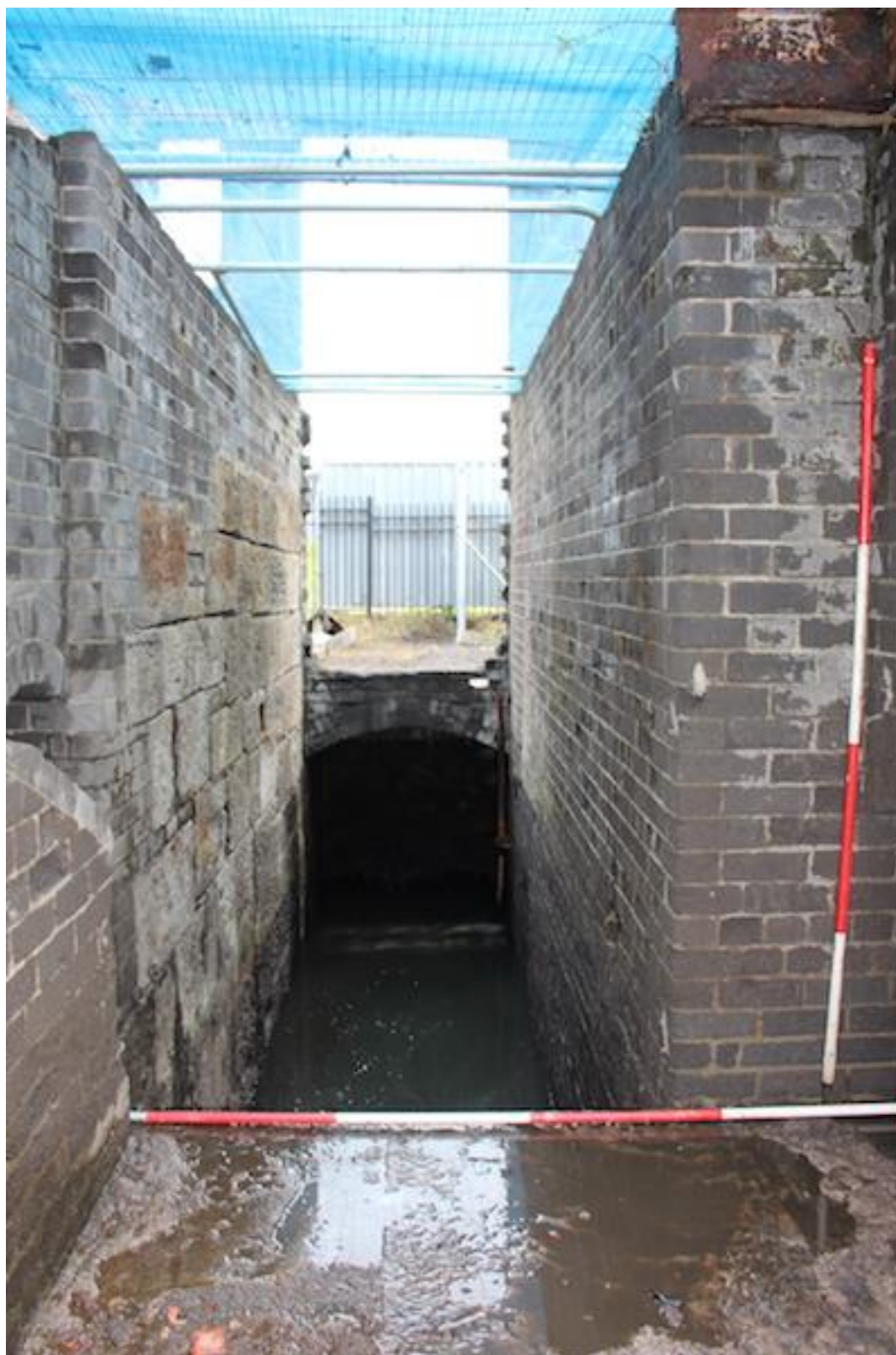
Plate 32. East-facing photo from inspection platform [207] showing wheel pit [206] and rope chamber [205].
