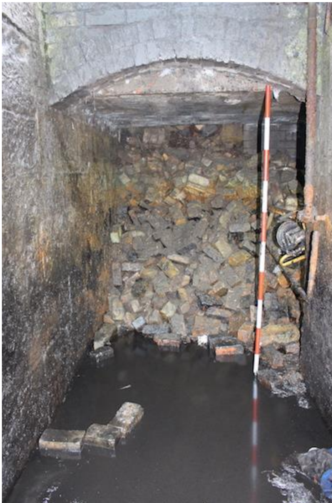
Plate 27. East-facing post –excavation photo showing rope chamber [205] extending east from the base of wheel pit [206]. Brick backfill (204) was not fully removed due to concerns about subsidence.
