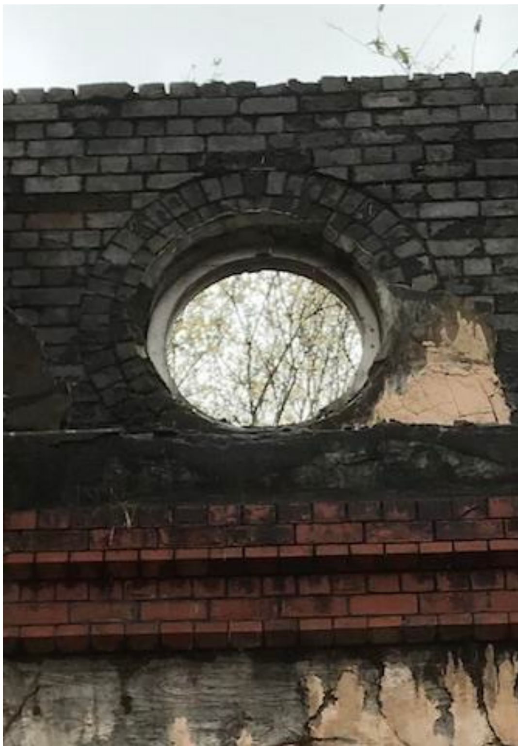
Plate 53. North-facing photo showing in-situ ocular window frame.
