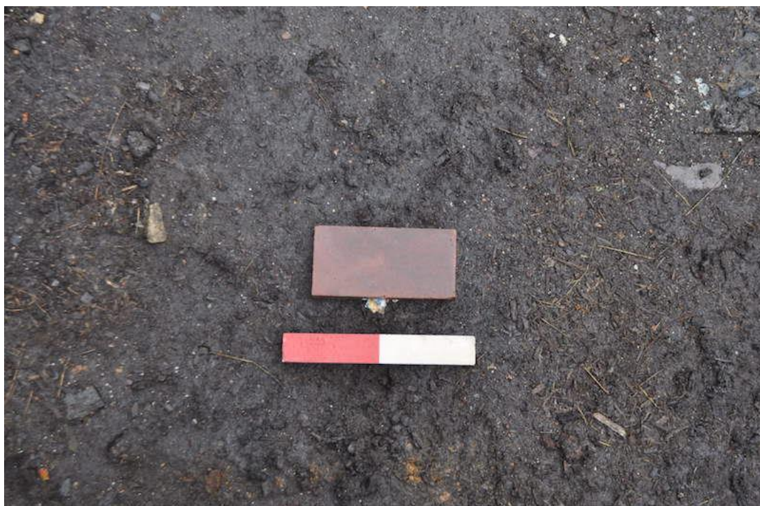
Plate 69. Quarry tile. These remain in situ in the machine floor of the Vivian Engine House.
