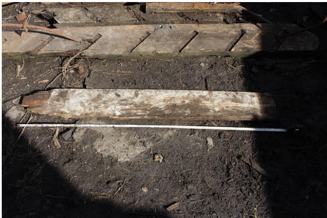
Plate 47. One of a number of white-painted timber tongue & groove timber boards that were recovered from both main basement [105] and wheel pit [206].
