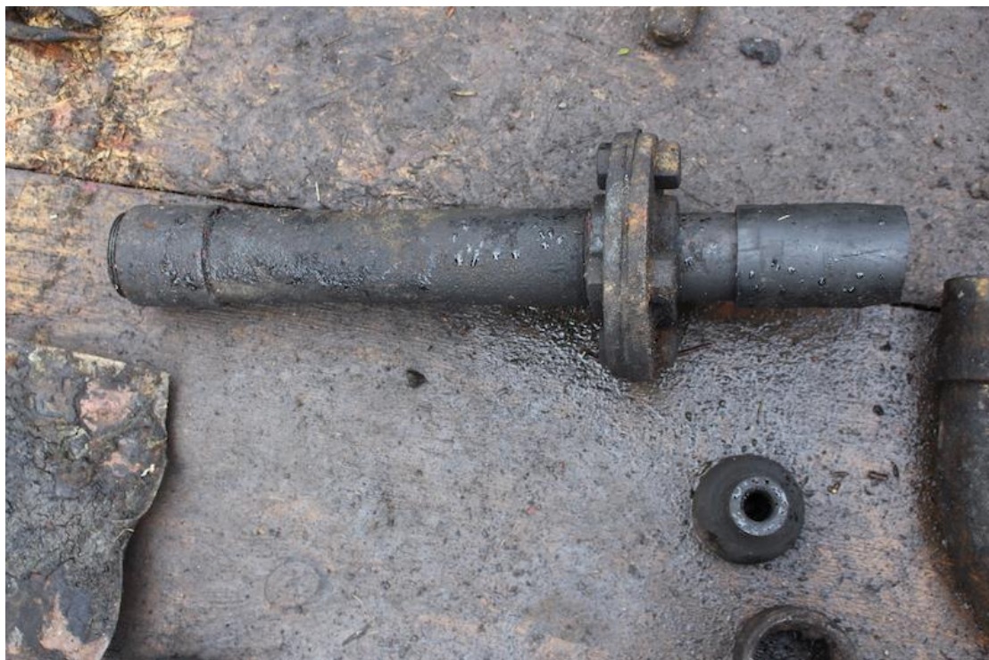
Plate 92. Example of section of pipe recovered from wheel pit [206].
