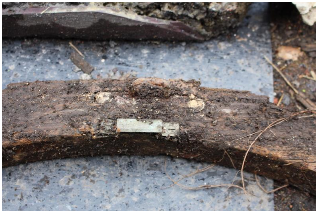
Plate 51. Detail photo of window catch attached to section of ocular window frame. A further example remains in situ in the Vivian building.
