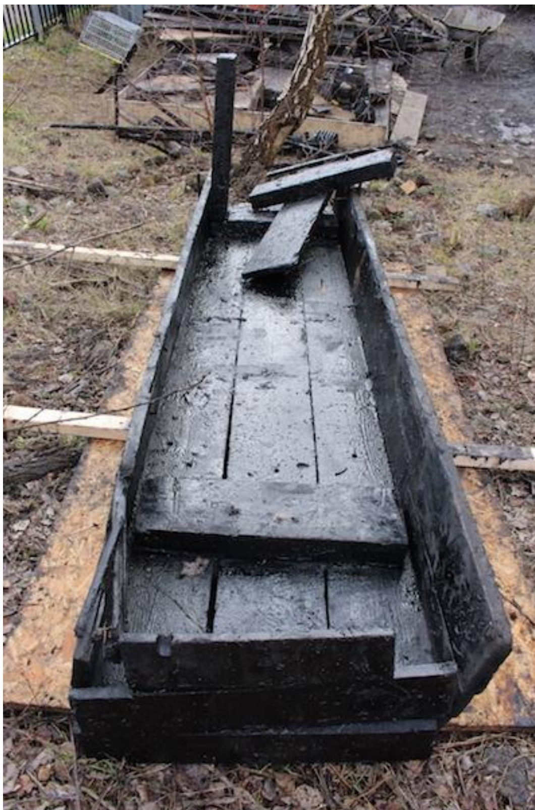
Plate 74. End view of the large section of timber leat recovered from wheel pit [206].
