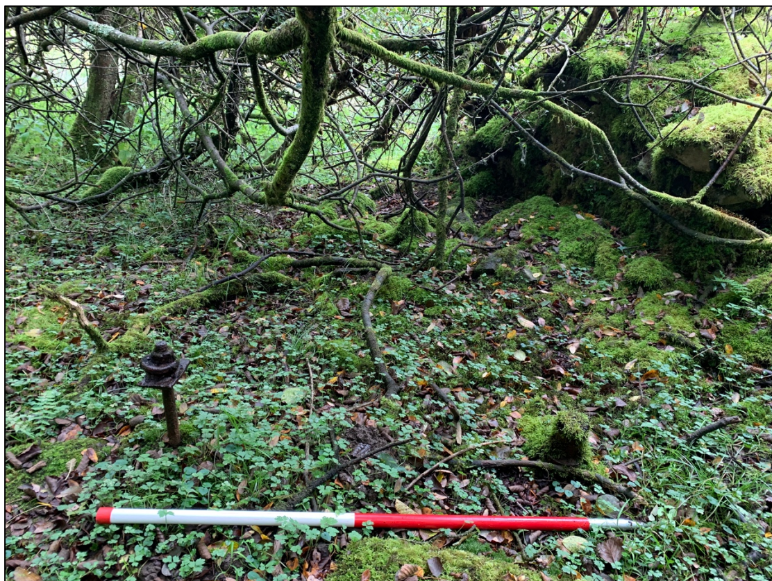
Plate 24. South facing detail of metalwork within structural remains of 'Structure' (GGAT06430m) at western terminus of 'Old Tramway' within Waunwyllt Colliery.
