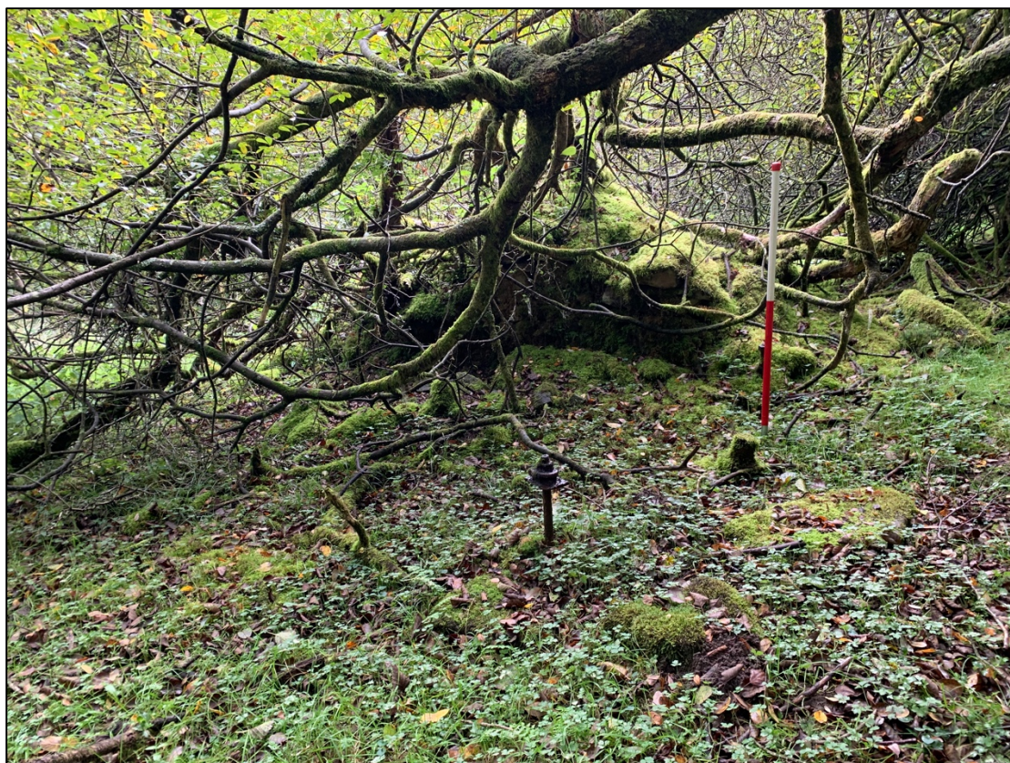
Plate 22. South east facing view of structural remains of 'Structure' (GGAT06430m) at western terminus of 'Old Tramway' within Waunwyllt Colliery.
