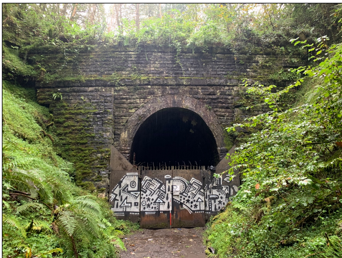
Plate 42. South west facing detail of the Neath Valley Railway Tunnel.
