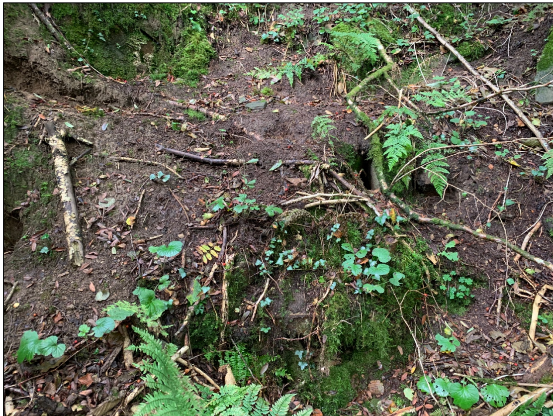
Plate 29. South east facing detail of Old Level (BPW02) close to Pen-y-lan Farm (GGAT03746m) showing structural masonry.
