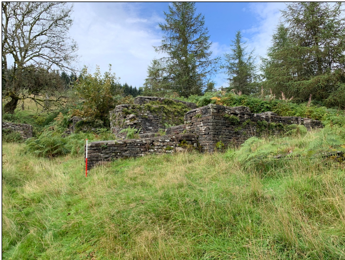
Plate 33. North west facing view of Pen-y-lan Farm.
