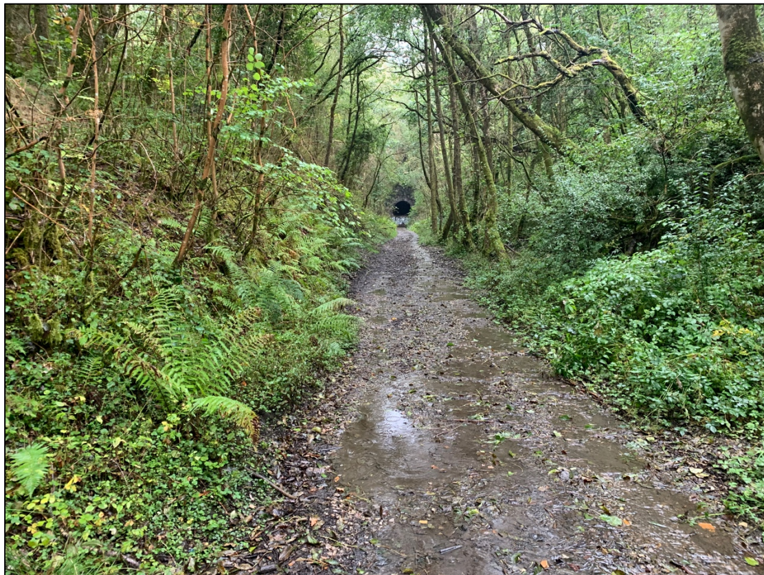
Plate 41. South west facing view of Neath Valley Railway Tunnel and Cutting.
