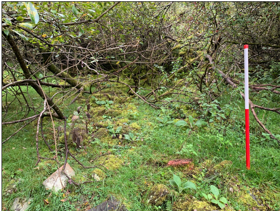
Plate 25. North east facing view of demolition rubble associated with structural remains of 'Structure' (GGAT06430m) at western terminus of 'Old Tramway' within Waunwyllt Colliery.
