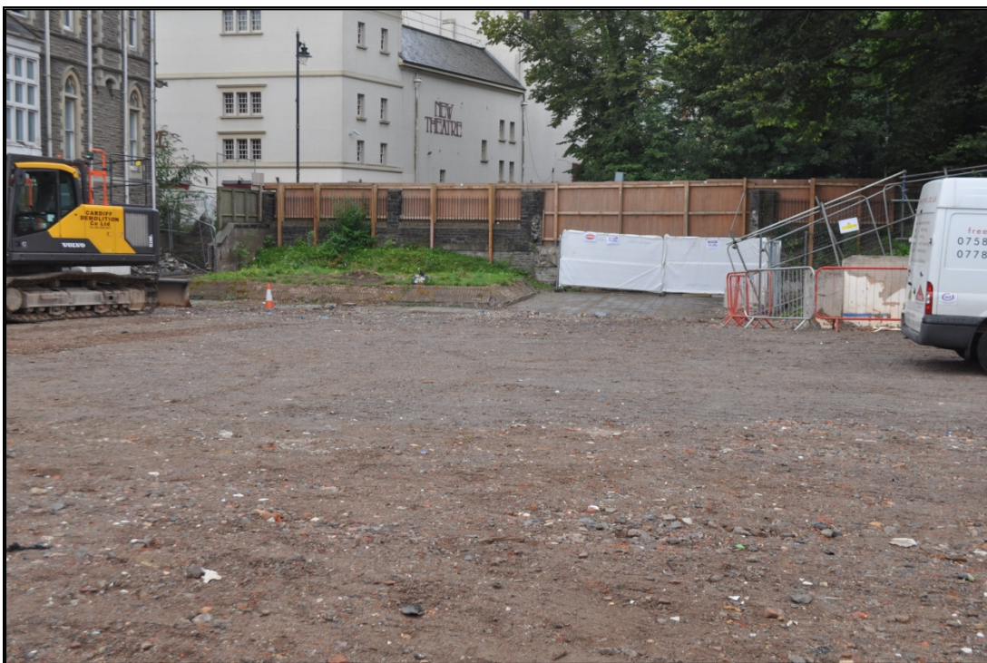
Plate 8 – General view across excavation area (looking west).
