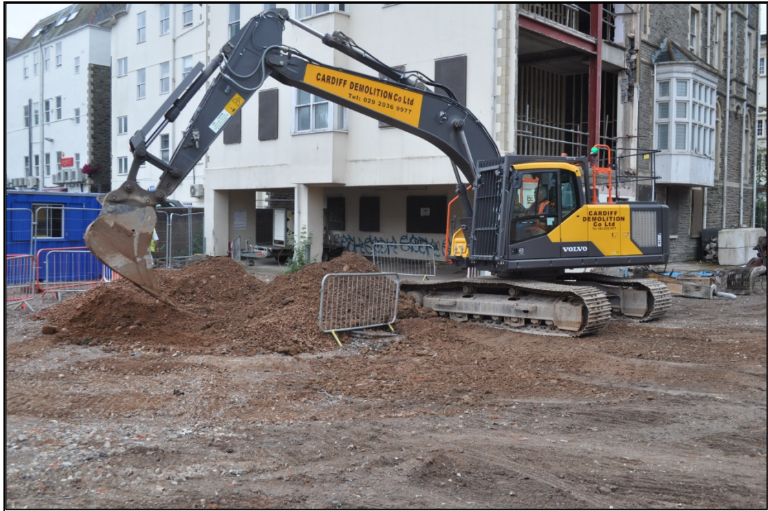
Plate 9 - General view across excavation area (looking southwest).
