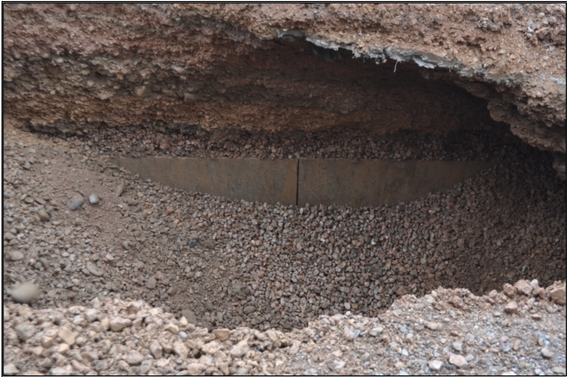
Plate 1 - Trench 1 revealing the southern wall of the encased Bute Feeder Canal [105] (looking north).
