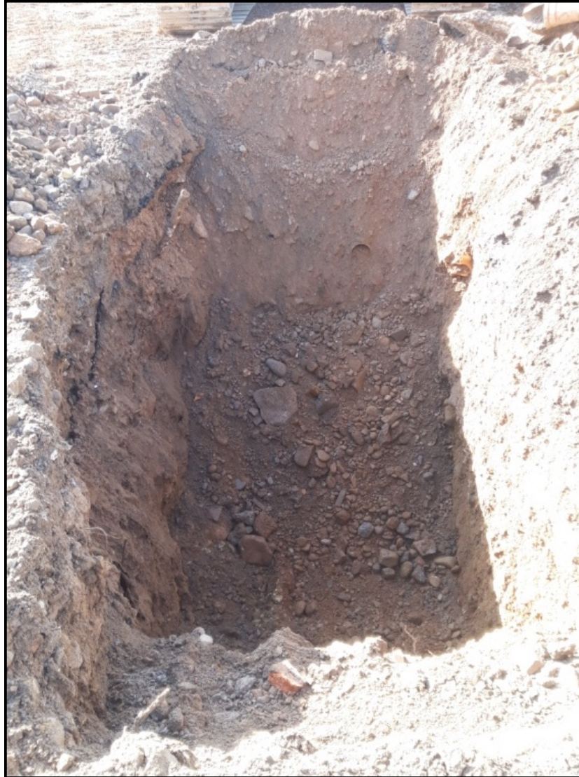
Plate 6 –Trench 5 showing made ground 502. (looking south)
