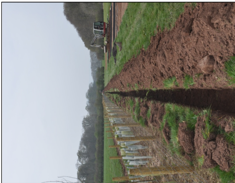
Plate 19. Excavation of service trench and caravan platforms (view W)
