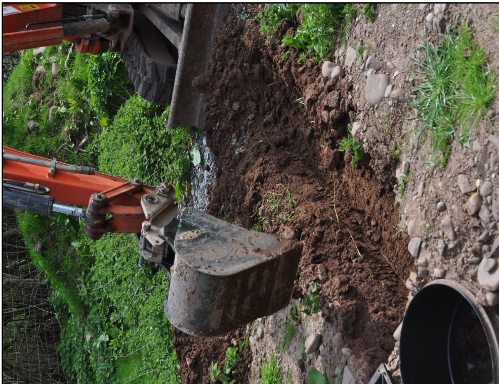
Plate 26. Final element of groundwork linking the service trenches T1 and T2 to the manhole (view SE)
