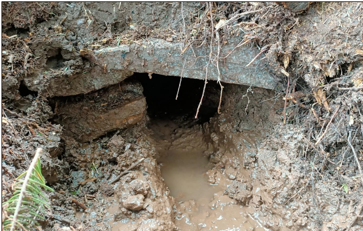
Plate 6. Outfall head [026] of Historic Culvert IV (ID28 in Appendix IV)
