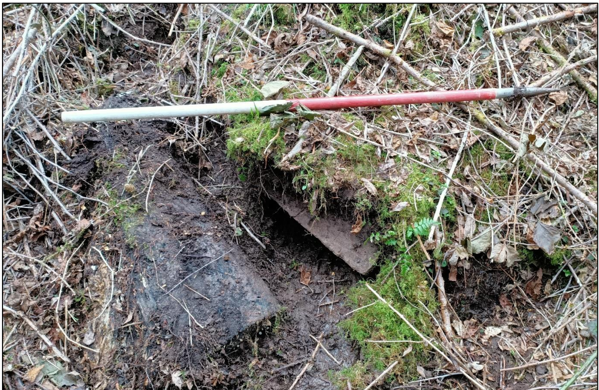
Plate 10. Outfall head [042] of Bryn Melyn Culvert I (ID30 in Appendix IV)
