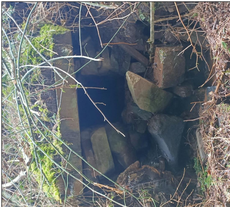
Plate 4. Outfall head [018] of Historic Culvert III (ID27 in Appendix IV)
