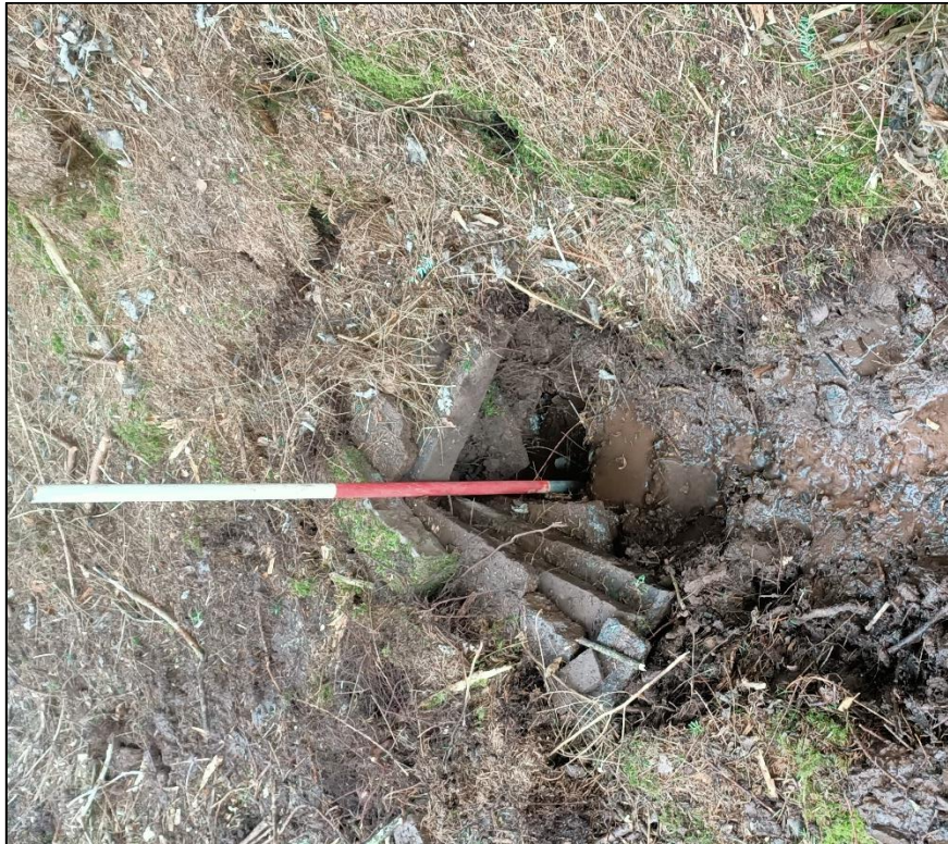
Plate 11. Inflow head [047] of Historic Culvert VI (ID33 in Appendix IV)
