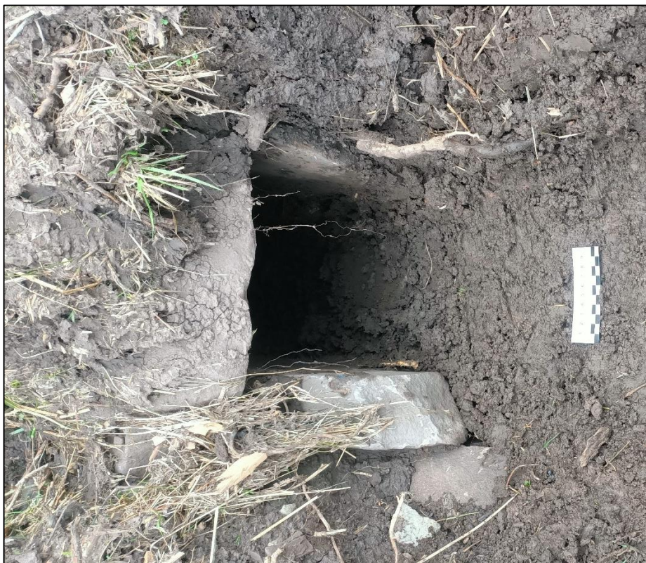
Plate 18. Outfall head [075] of Historic Culvert X (ID43 in Appendix IV)
