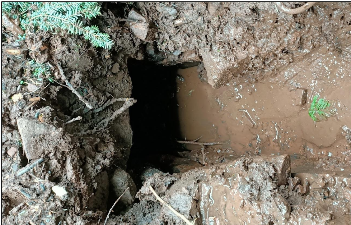
Plate 5. Inflow head [024] of Historic Culvert IV (ID28 in Appendix IV)
