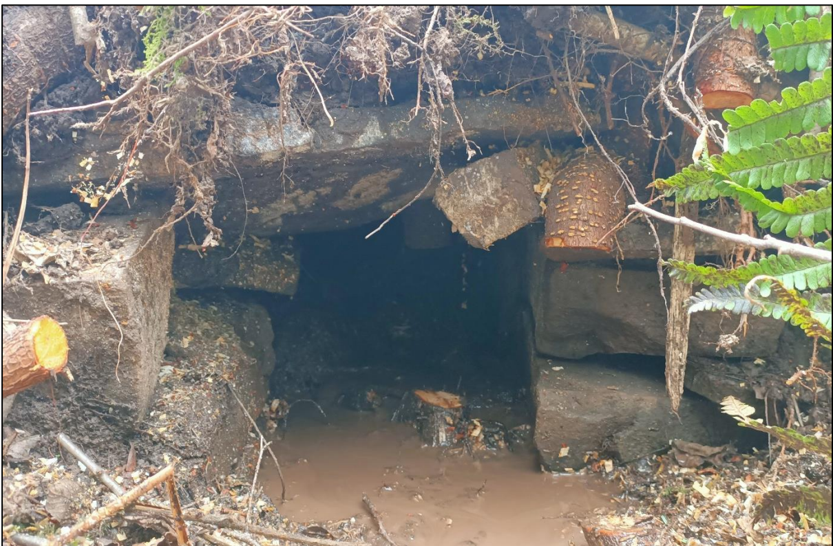
Plate 8. Outfall head [036] of Historic Culvert V (ID29 in Appendix IV)
