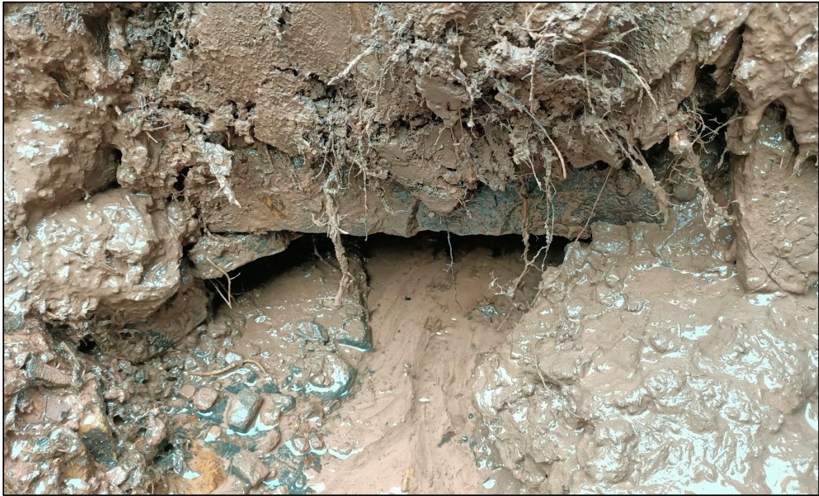
Plate 7. Inflow head [032] of Historic Culvert V (ID29 in Appendix IV)
