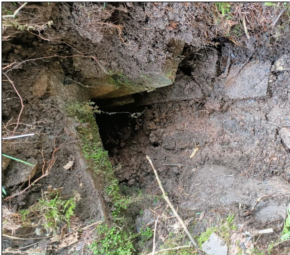
Plate 14. Outfall head [057] of Historic Culvert VII (ID34 in Appendix IV)
