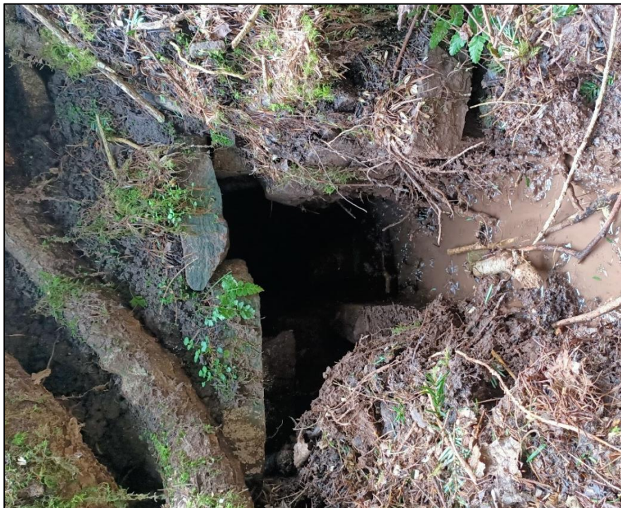
Plate 12. Outfall head [050] of Historic Culvert VI (ID33 in Appendix IV)
