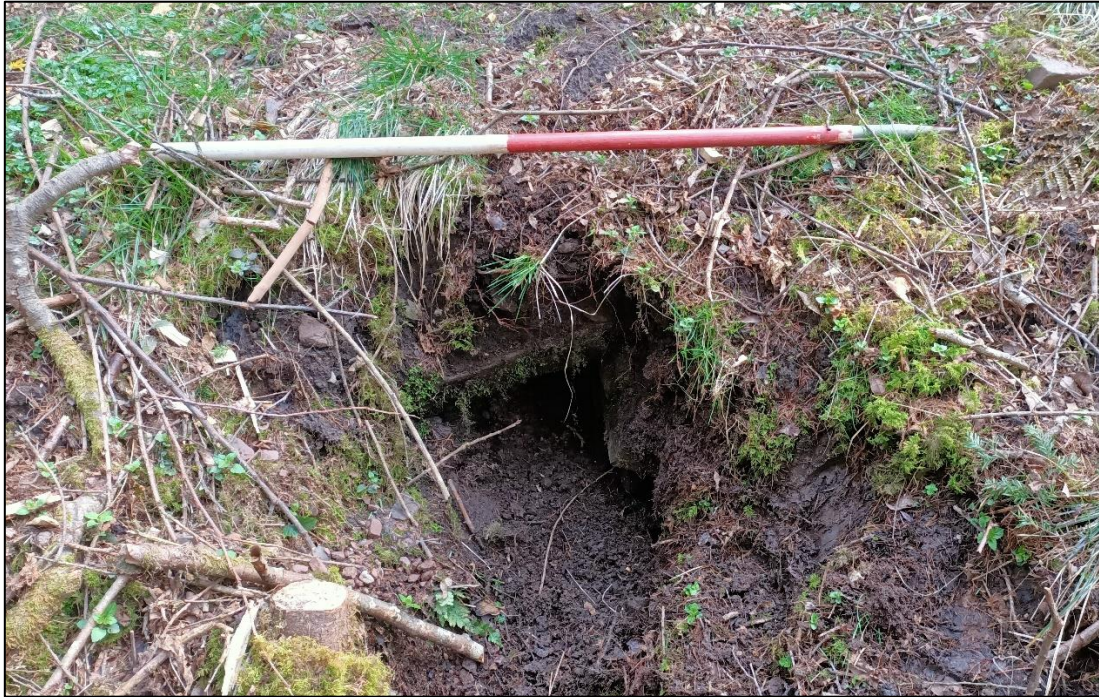
Plate 13. Inflow head [054] of Historic Culvert VII (ID34 in Appendix IV)
