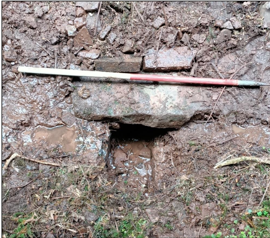
Plate 3. Inflow head [014] of Historic Culvert III (ID27 in Appendix IV)
