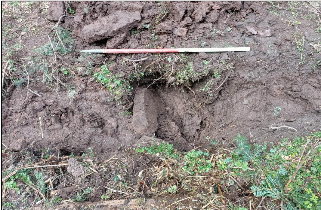
Plate 1. Outfall head [008] of Historic Culvert II (ID26 in Appendix IV)
