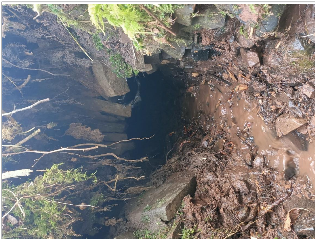
Plate 16. Outfall head [066] of Historic Culvert IX (ID36 in Appendix IV)
