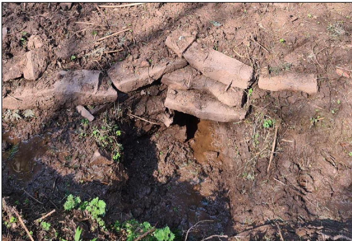
Plate 2. Inflow head [004] of Historic Culvert II (ID26 in Appendix IV)
