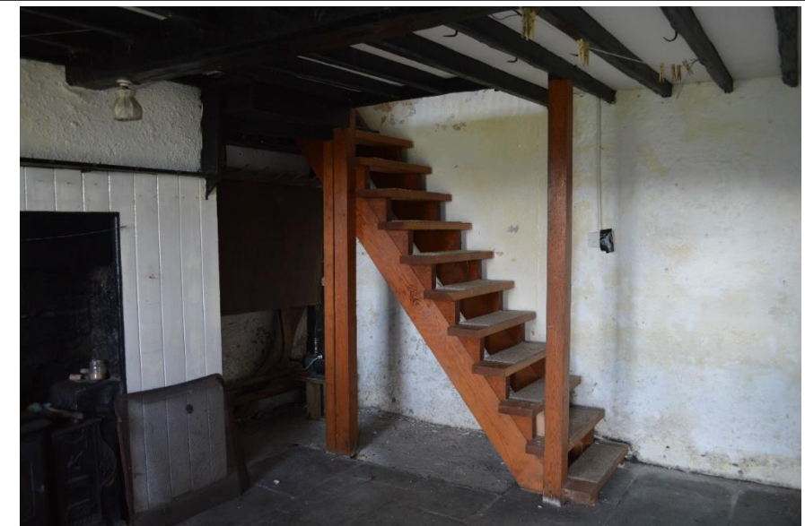
Fig. 13 The hall showing new stairs
