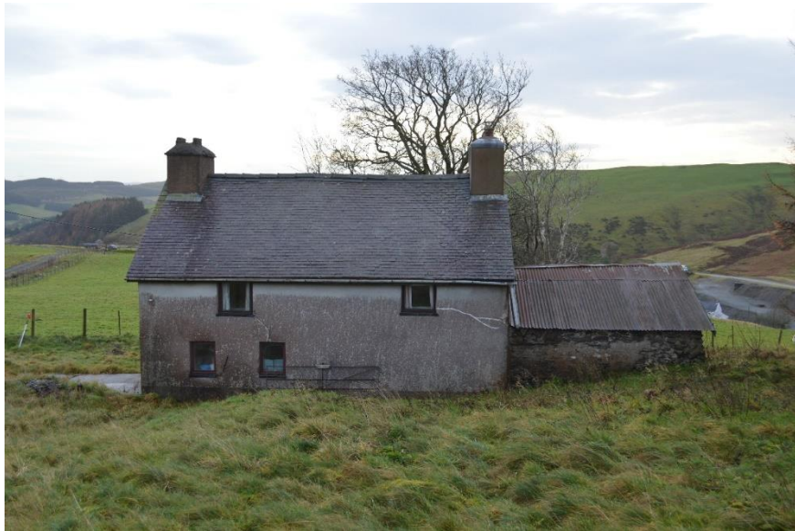
Fig. 8 The north-western elevation
