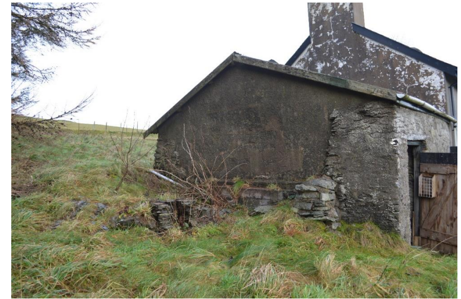
Fig. 7 The south-western end of the byre and site of outbuilding
