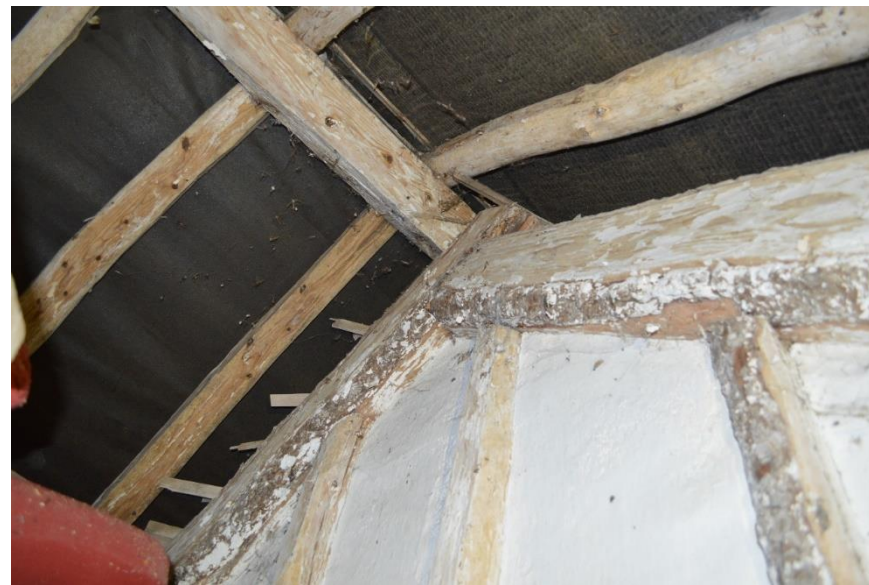
Fig. 21 Apex of roof
