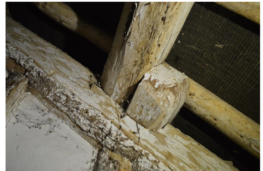
Fig. 22 Roof truss showing purlins
