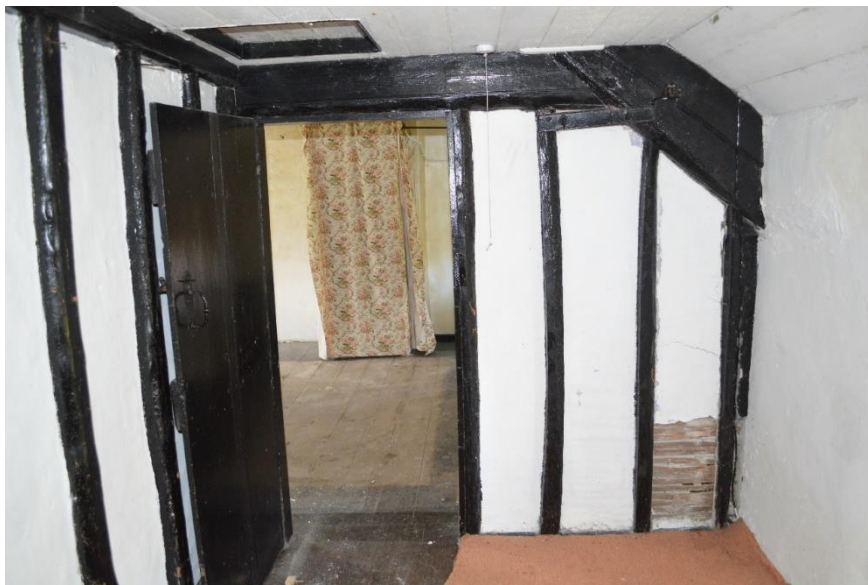
Fig. 20 Bedroom three showing timber and lath and plaster partition
