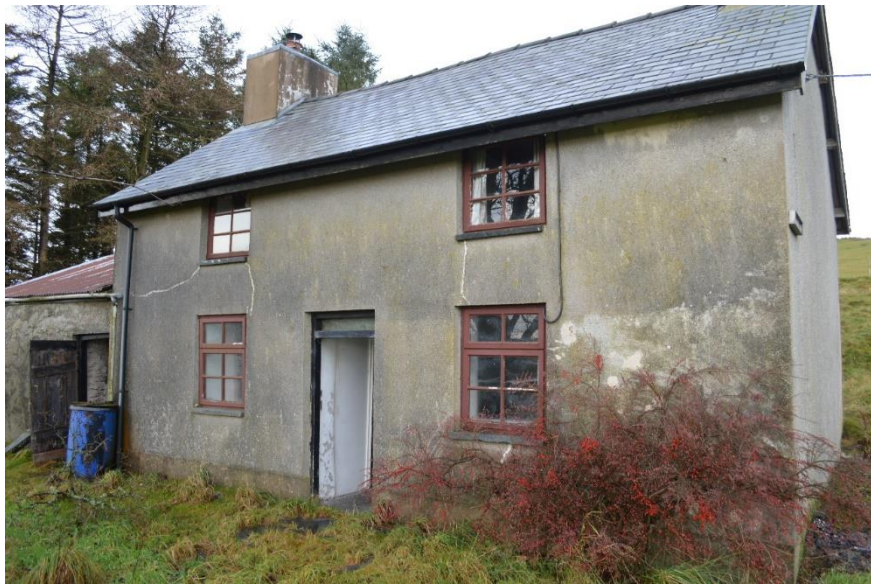
Fig. 5 The south-eastern elevation
