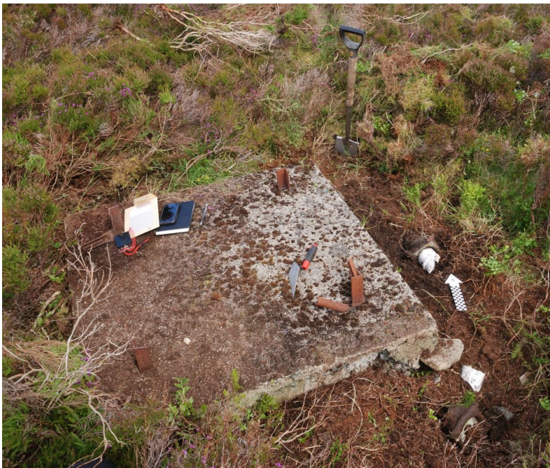
49. A counterpoise base (concrete of 4' x 4') for the 1923 extension, showing remnant lattice ironwork (32" x 32") and two large tubular insulator fixings, now known from detail visible in MS.Photogr.c.243 image 718 (inset, right) to be used to strain the wires at the tower; a 'jumper' wire interconnected both sides of the counterpoise wire over the tower. Concrete = 4' x 4'. 53.121962°, -4.169796°
