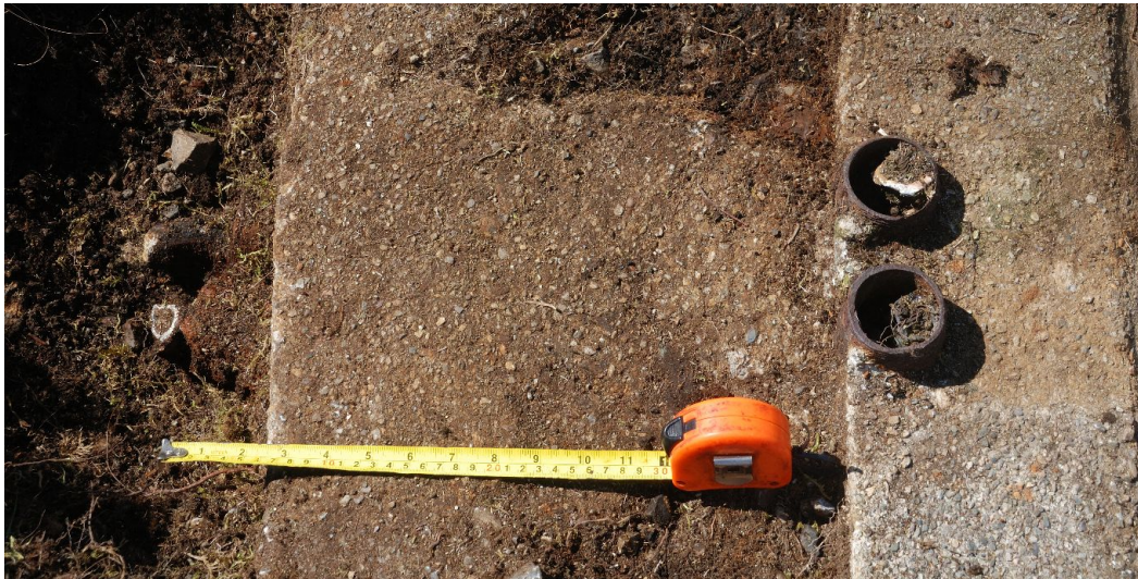
82. Twin feedline entering the double ATI base, left, emerging within the building through iron tubes, right and 83, below:
