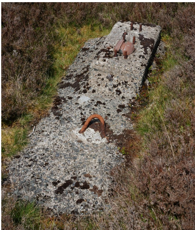
22. Winch base and wire-guiding loop (erosion of the underside of the loop apex is evident by touch). The lighter fine concrete at the base of the loop, evident at all winder sites, suggests it was added at a later point to the base. Protruding block 25\frac{1}{2} " x 7\frac{1}{2} " (with variations); bolt centres 10" and 11"; bolts \frac{3}{4} " dia, protruding 2\frac{1}{2} ". Lower base typically 85\frac{1}{4} " x 37". Lower and upper base apparently cast as one unit. A broken brown stay insulator rests to the rear.
