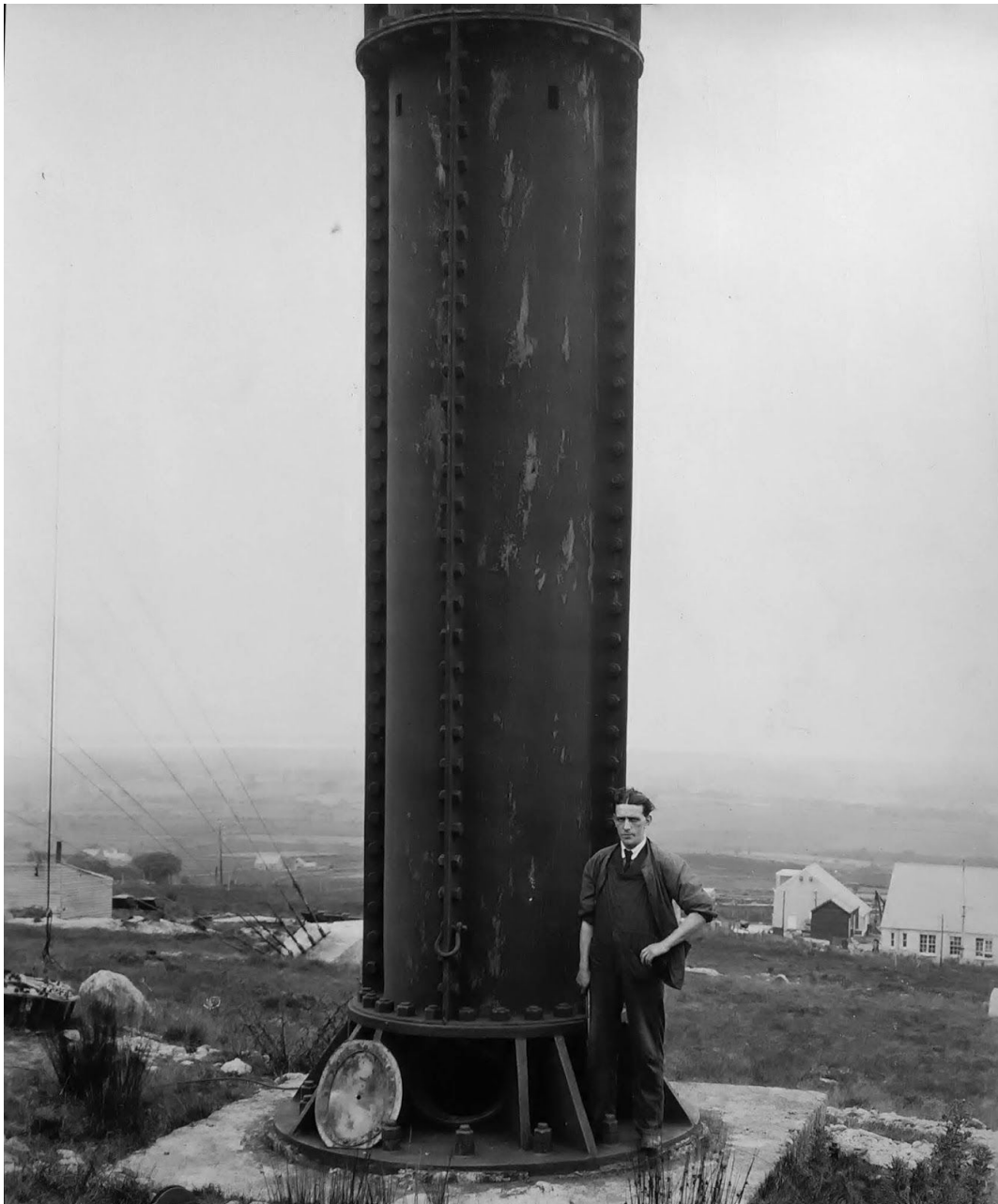
12. Central mast (Mast 2) of the first three masts at the transmitter (western) end of the antenna. A hatch is laid open, giving access to the ladder running to the top gallery, within (The Wireless World, July 1914, p.218). The baseplate at the concrete (6' diameter bolt outer to bolt outer) is of 16 bolts of 2" OD, with two nuts of 2½" OD securing each. The ¼ section mast elements, each 15 feet long, are of fairly thin steel (see 129), perhaps ¼" or less thick, with 29 bolts joining each vertically. Rectangular holes, of unknown purpose but possibly to facilitate erection, are seen in the upper centre of each section – also seen in images of Marion (USA) and Ullandhaug (Norway) masts. The lower part of the mast was 3'6" in diameter (presumably internal, but not known – both referenced accounts fail to indicate), the upper part 2'6" (The Wireless World, July 1914, p.217 and Marconi station pamphlet in MS.Marconi.198). Note the 7-stay anchor at rear left of mast and what is probably a triatic halyard, at far left. The item on the floor at left is difficult to identify. The lanyard is behind, rather than connected to it. There are no small steel masts either side of the transmitter house at this time. Bodleian Special Collections MS. Photogr. c.243, document P.2092. Date unknown, but pre-elevated counterpoise, and therefore pre-1921, probably around 1918.
