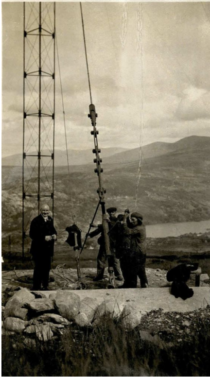
138. Tensioning of one of the stay cables using rods to adjust the large threaded turnbuckles. Probably Mast 15, anchor A. Grounding connections and straps are not installed as yet in this photograph of January, 1924. Bodleian Special Collections MS.Photogr.c.243, photo 715/x.
