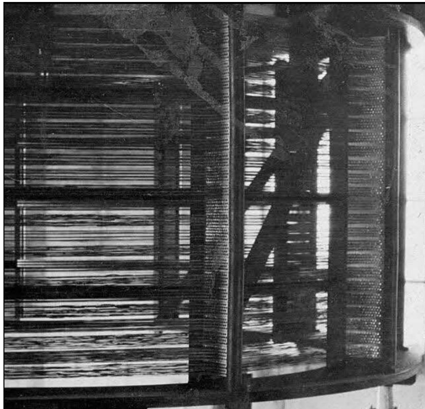
C6. Detail of '9176' insulators seen in their role as inductor wire spacers at the upper inductor house.
