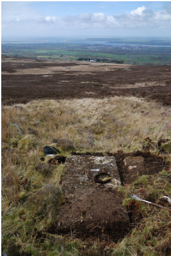
D28. Concrete platform and lesser platform to its right, separated by a 1ft sloping gap. The second platform seems, from the sequence of concrete at the foundation level, to have been built after the first, main platform. The platforms are at the head and aligned with the centre of an inclined trackway running at least as low down as Mast 9, the centre mast of the rearmost three masts of the original, 1914 antenna. The recovered oval band is seen, placed for documentation, with the tape open to 1ft. The transmitter hall lies in front of the trees in the distance (upper centre).
