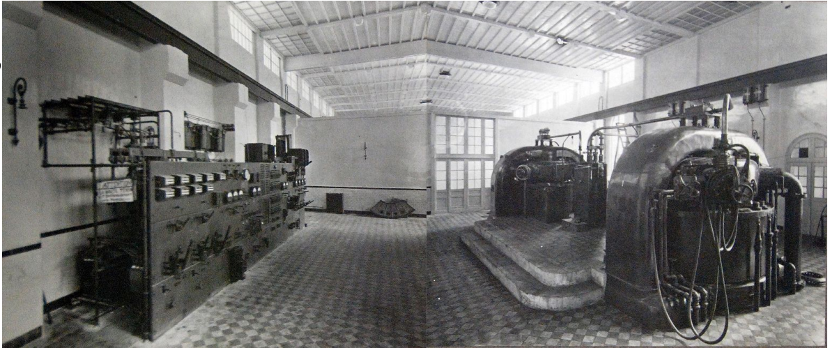
Poulsen arc transmitters, of 500kW each, seen in a panoramic, two-photograph image of the transmitter room at Lafayette station, Croix d'Hins, France. The installation at Carnarvon would have looked much the same. Image © Bibliothèque nationale de France, under academic licence.
