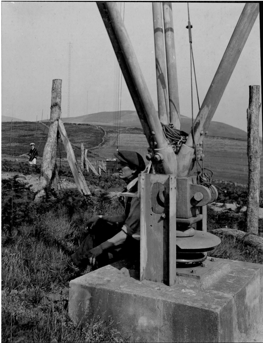
R8. A worker takes a break at the base of a receiving antenna support mast in this contemplative scene. Note the halyard, which is seen to run inside standoff brackets in other images. Four other lattice masts of the original, ‘inverted-L’ receiving antenna are seen to run up the hill in the distance. The top of the nearest mast seen in its entirety clearly has a horizontal arm. This supported a single wire either side; contemporary accounts describe it as a “two wire” antenna (Bodleian Special Collections, MS.Marconi.198), though electrically, it was one, connected at a common anchor point and then to the receiving sets. A man in naval uniform bearing the sleeve insignia of Lieutenant looks on, centre right, hinting at a WW1-era date. The mast converges on a tilting bearing. The steel uprights, with roughly-cut oval openings either side of the base mount would almost certainly have been a temporary pivot or securing point for erecting the mast at installation. Guy wires kept the mast vertical. The base remains in-situ, but the steelwork is now rapidly dissolving in the salt-laden gales. Bodleian Special Collections, MS.Photogr.c.243, photo P.2097, date unknown, probably ca. 1918. The distinctive curved field boundary, which is unchanged today, permitted the location to be confirmed as 52.581847°, -4.066318°
