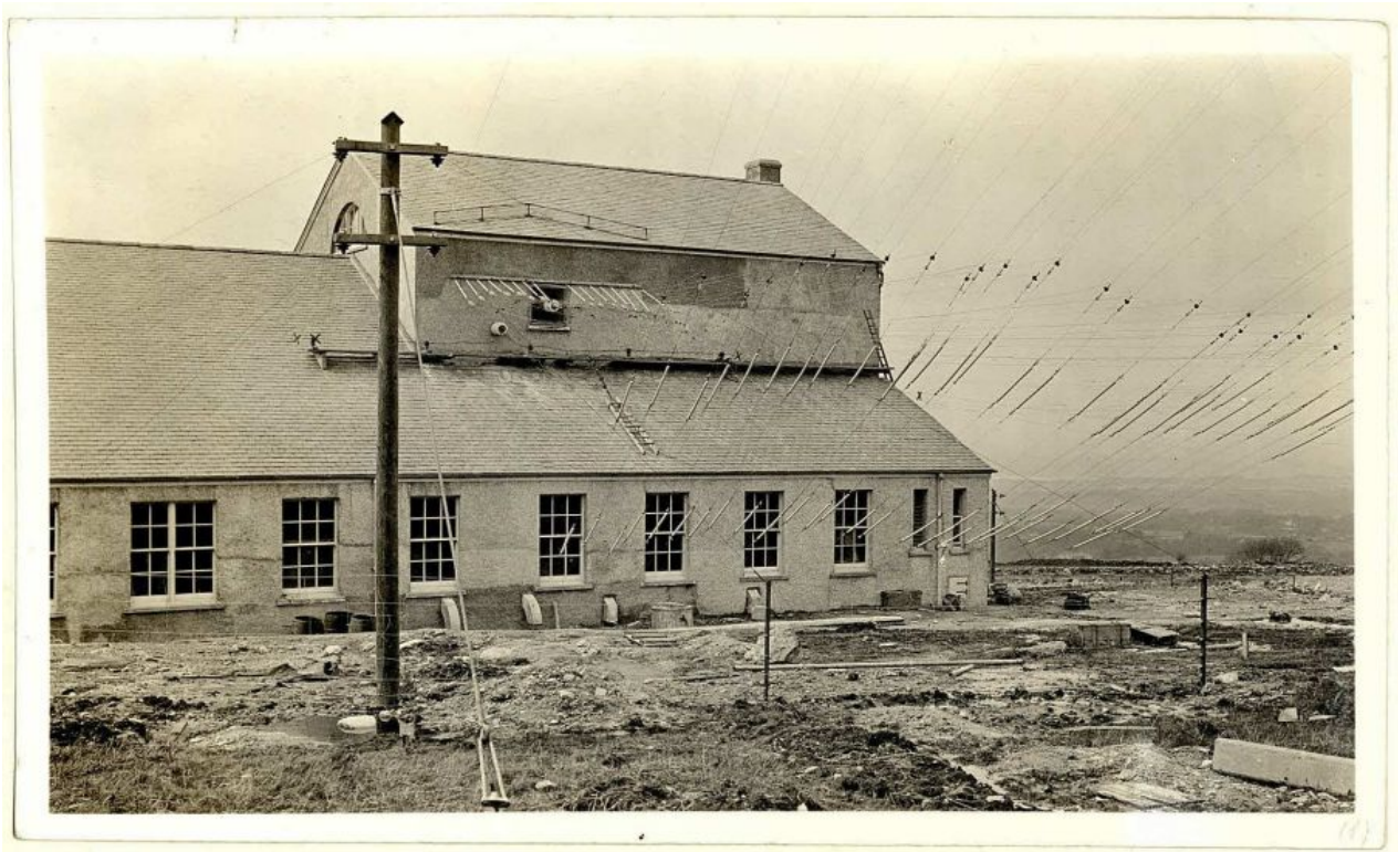
26. Carnarvon transmitter house, antenna and ground feedlines, date unknown, but from the debris and ground disturbance, early-on and certainly not later than 1917, as the same image appears in Bucher (op.cit. p.294). The 'telegraph' pole at left seems to feed the two dark fence posts in the right foreground, which have multiple wires, almost certainly the start of the buried earth screen, running into the ground (cf.45).
