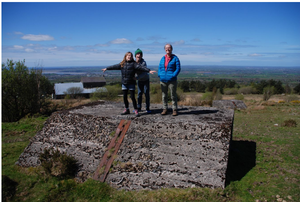
9. A wider, April 2017 view of concrete anchor 3B, with family members for scale! Transmitter buildings seen in background, centre left. The blocks present a 35.5-37 degree (varies slightly between blocks) sloping face, within which stay attachment points are inserted between and bolted to a concreted-in, \frac{1}{4} "-thick, pair of 4"x4" 'L'-section steel retainers, 7' long (slot between is 1.5" wide). Anchors 143" x 124", height variable according to surrounding ground, typically about 45". Anchor fixings 4.25" long. Their mass, some 98 tons ('Trans-Ocean Wireless Telegraphy, New Transatlantic Service, The English [sic] Station Described'; The Wireless World, July 1914, p. 218) has led to at least two of the anchor bases tipping in the peaty ground; 10D by 3 degrees and 4C by 5 degrees. Anchor 4B is in poor condition, but because of this, allows the internal anchor steelwork to be understood (see 123, 124 ).
