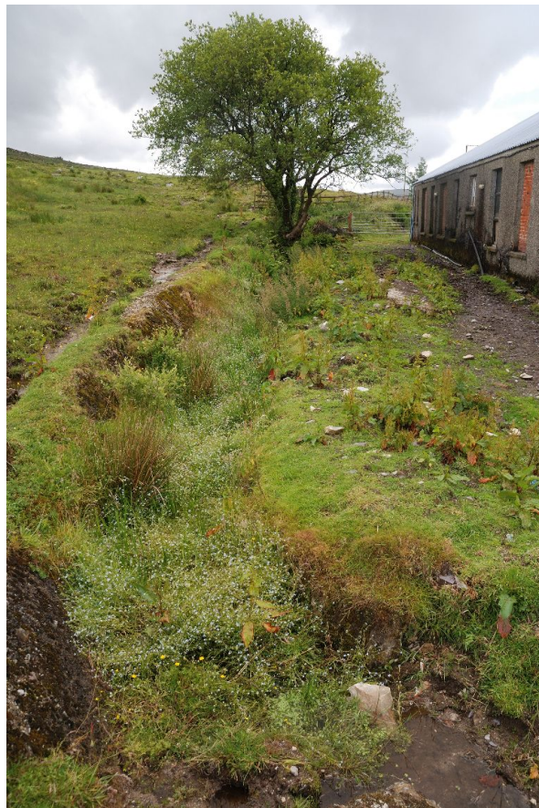
40. A low but substantial concrete retaining wall/dam (centre left) and deep drainage ditch (centre) in front of the station transmitter buildings. The site is extremely boggy and wet in all seasons, and is susceptible to soil movement.
