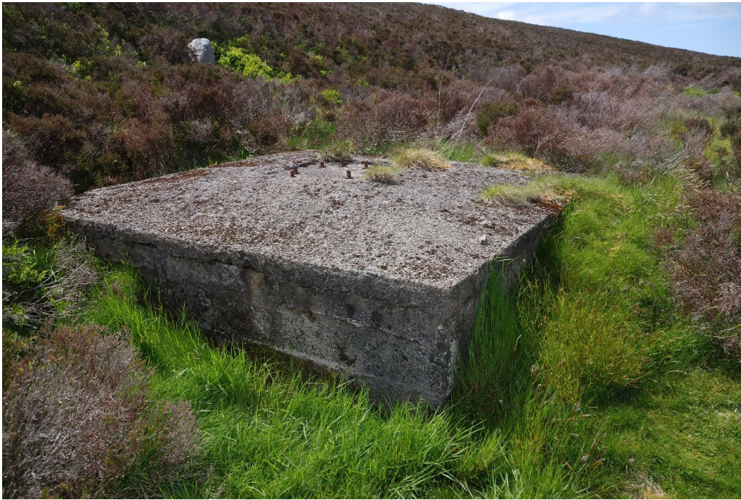
99. Profile of a 1923 lattice mast base block (one of three per 3-sided mast). As is the case for most of the concrete structures, the raised top surface, for drainage away from the metalwork, was evidently laid separately to the main block, and appears to be fairly weak in comparison. The bolts, however, ran deep into the main block. Note horizontal shuttering impressions. Tower 14, 53.123037°, -4.169589°.
