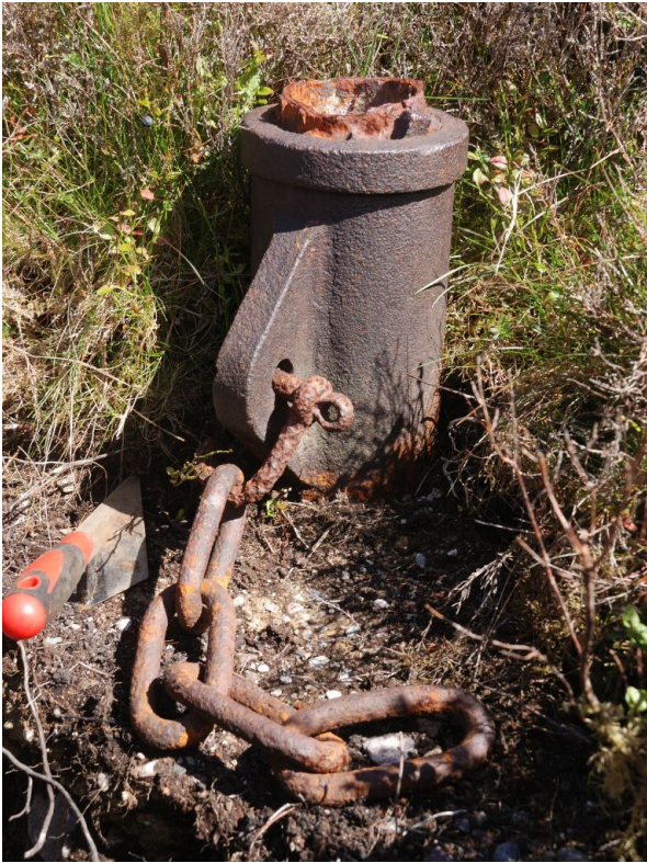
32. Iron tube base at Carnarvon, showing attachment point, shackle and chain, which is also seen at Marion (see 33). Chain appears more substantial at Carnarvon, and no trace of an attachment on the base block was found on any such base. 53.122130°, -4.176786°. Trowel blade = 6"/150mm.
