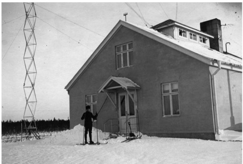
R6. A helical, 'Rendahl' mast, which were standard-issue, high strength-to-weight ratio designs for early Swedish wireless stations, here seen at Härnösand radiotelegraph station, callsign 'SAH', opened in 1916.
