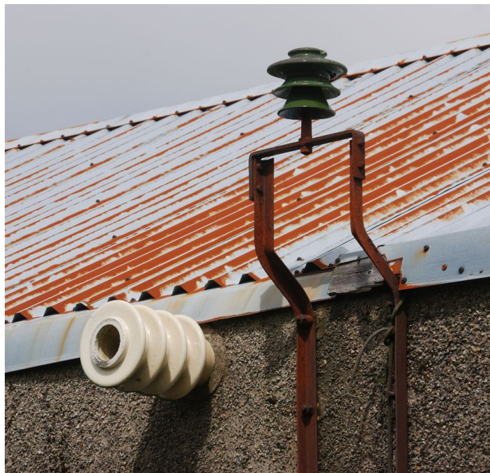
C38. At the southern end of the transmitter buildings, a large through-wall white insulator, of the same kind still seen at the eastern, antenna-facing elevation and at both, now demolished ATI buildings, remains in perfect condition. It may have been the connection to a later common earth point to the rear of the building. Alongside, a multi-part green insulator, of currently uncertain purpose. A brown multi-part insulator also remains in perfect condition, mounted slightly to the east on the same wall (C39, below).
