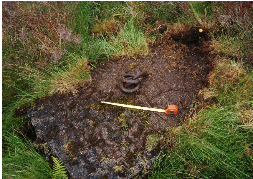
128. Small concrete base with central loop and two iron rings affixed, located 15 yards NE of Mast 16's base. It may have been related to triatic raising/lowering.
