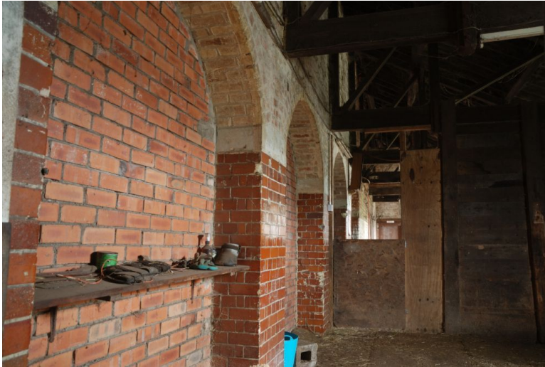
D20 , left: Interior vitreous glazed brick arches at the eastern, antenna-facing side of the transmitter hall. The arch infills are modern and now form part of a horse stable. The roof truss timbers are original and currently in excellent condition, though roof damage now threatens the long-term integrity of the building in general.
