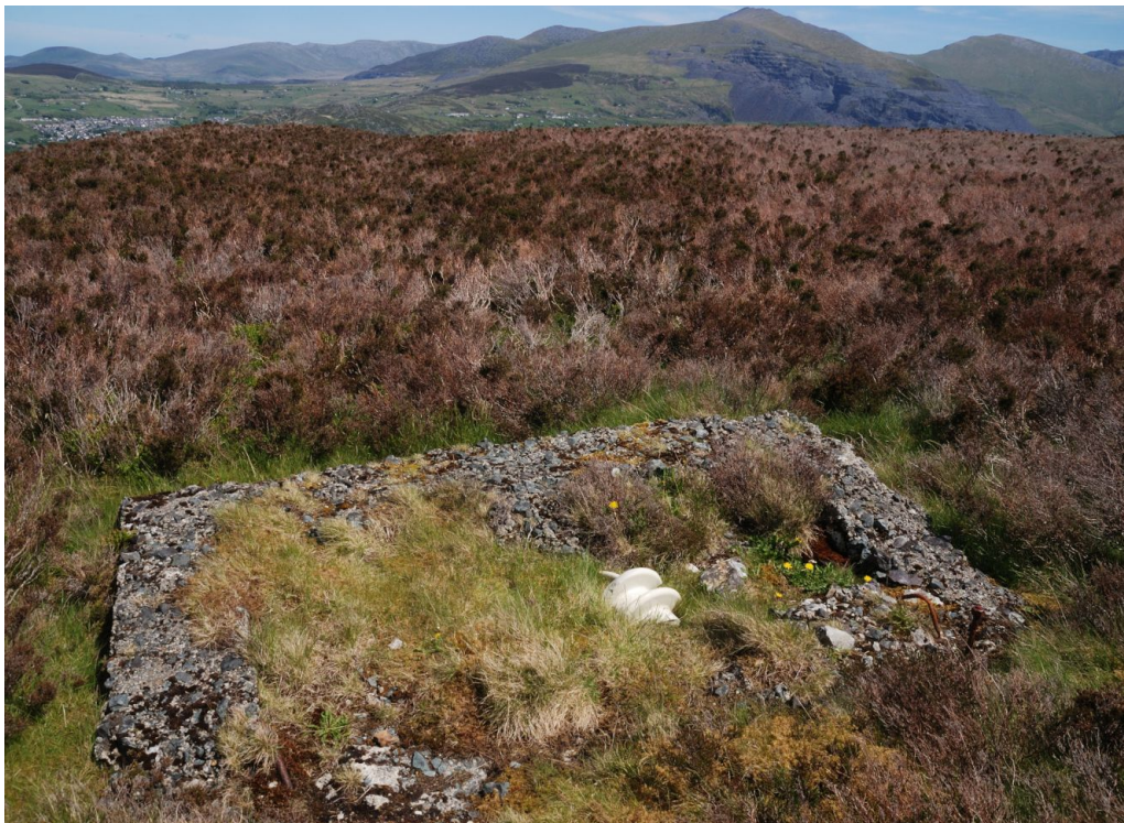
126. Rough concrete base lying near top of incline to lower 1923 extension site. Surface cleaning revealed that it incorporates substantial \frac{3}{4} " bolts and impression of a machine base. It is thought to be the base of the incline brake pulleys. Note the remains of a ATI through-wall insulator, probably brought up from the single ATI at the foot of the incline during salvage operations in 1939. 53.123140°, -4.171421°
