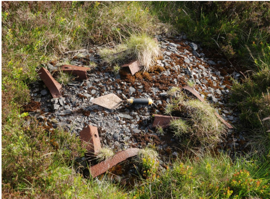
48. A typical concrete base for an elevated counterpoise lattice mast of the 1914 antenna, with remains of the mast legs ( 1\frac{3}{4} " x 1\frac{3}{4} " L-section steel). Many of the bases can only now be found when the pattern of installation is worked out from those few that are more readily found, and the pattern of shallow trenches for ground wires that are still seen to run between them. The bases in many parts of the lower end of the 1914 antenna are now fully buried by deep bog growth, whilst the bases for the 1923 extension are typically overgrown by dense, tall heather and, at the lower end, by bog growth. Trowel blade = 6"/15cm, bases typically 35"x35", lattice sides 20\frac{1}{2} " x 20\frac{1}{2} ".
