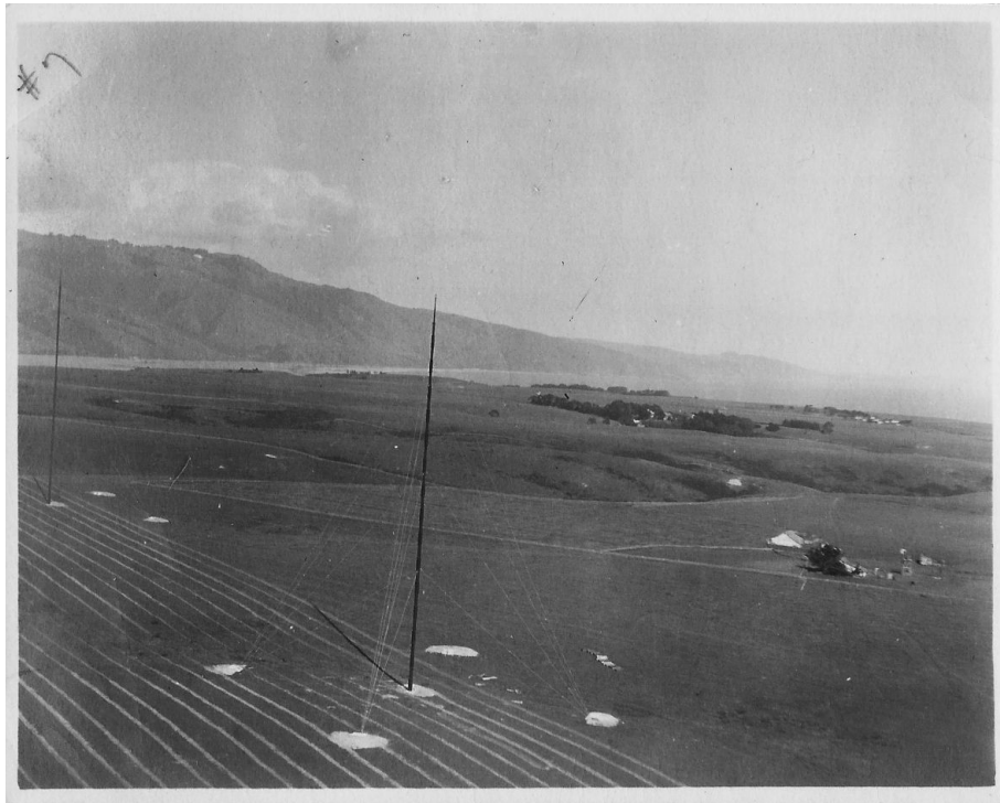
42. The pattern of the earth screen at Bolinas is seen very clearly, running lower centre to centre left, in an aerial photograph of 1913/14 (based on date of construction and opening given by Bolinas Museum, CA), taken shortly after installation where the bright cut ground for the wires contrasts strongly with the surrounding grassy cover. Survey at Carnarvon shows the extent of its buried screen was the same – to just inside the outer anchor blocks of each mast. Image courtesy California Historical Radio society
