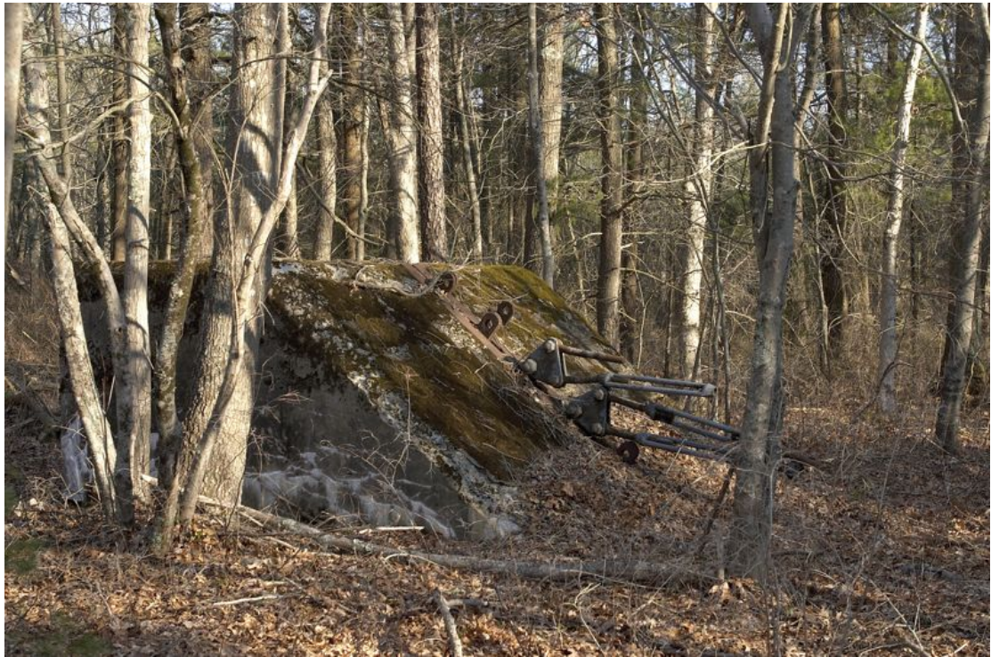
10. The familiar form, together with trapezoid, two-anchor attachment plates, now blending into the forest taking over the site of Marconi's Marion site, Massachusetts, USA. Image by kind permission of Marian Howell via Sippican Lands Trust.
