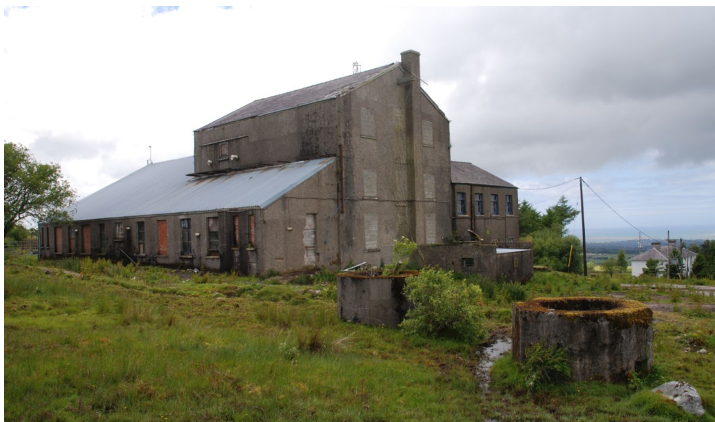
114. Octagonal inductor bases to the north of the transmitter house (on domestic land, access by kind consent of the occupiers). The nearest base, far right, is seen in a poor photo to support an inductor (see 116), and thus predates the 1925, GLJ 'third' antenna.
