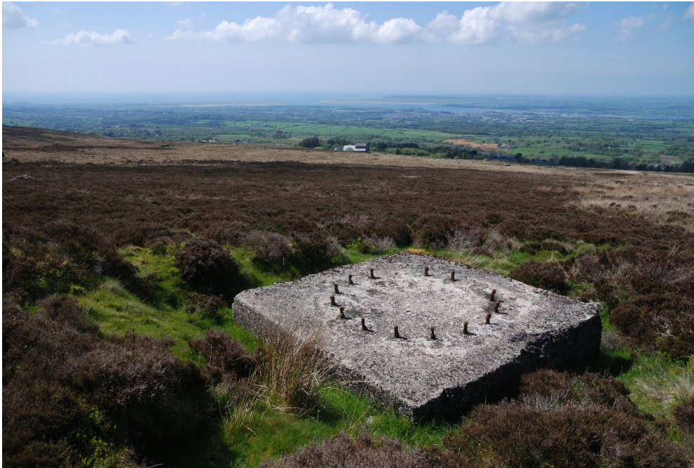
95. Concrete baseplate mounting block (Mast 6), with 16 bolts of 2" diameter at 14.5" centres protruding 4.25" in a ring 6 feet in diameter. 53.123082°, -4.182320°.
