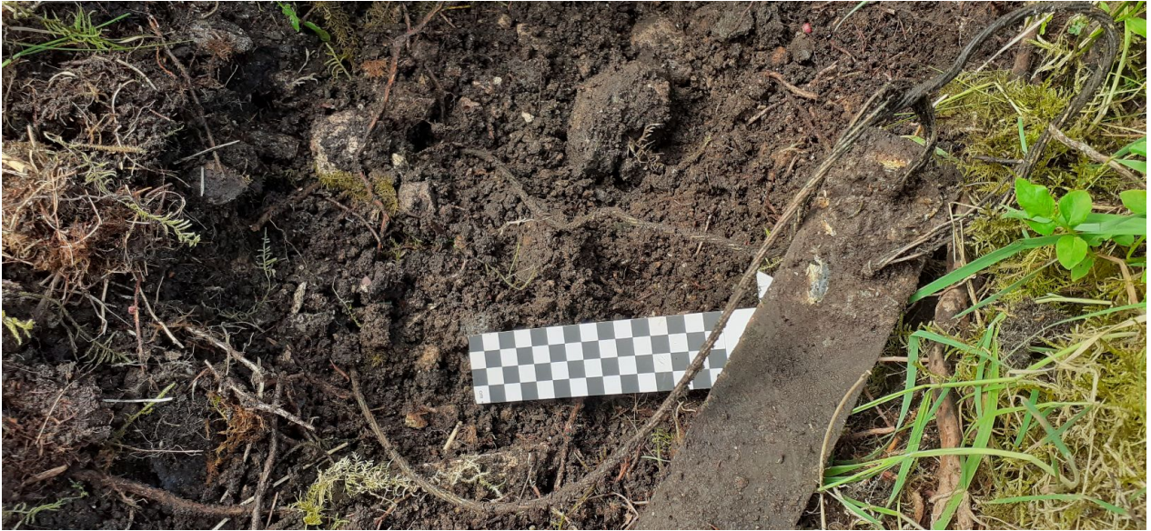
Excavated grounding strap (right) for the stay cable of Mast 13/17 at anchor block 13/17A, with two bonded, 7-strand copper wires running into the earth. The wires and band were covered with ballast-type stone. Scale squares = 1cm ( not arranged to show north).
