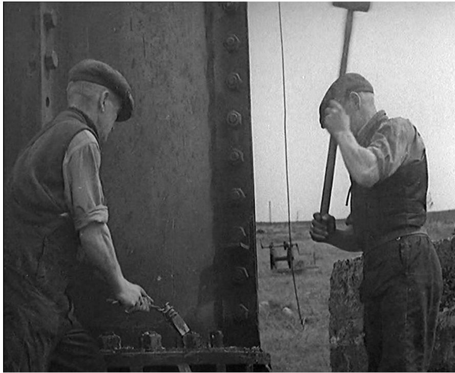
21. Hand-operated, empty, possibly triatic winch uphill of a mast, almost certainly Mast 1, given the concrete anchor to the immediate right of the hammer-wielding gentleman, during demolition in 1939. The scene shows the men splitting mast base to tube-securing nuts with a sharp chisel mounted on a thick twisted-wire handle to eliminate impact shock to the user's hand. This usefully explains the numerous split nuts still to be found across the site. Source: © Reuters via British Pathé, Film ID: 1013.05, issue date: 1/06/1939, under licence.
