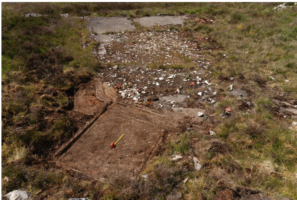
77. Light surface excavation revealed the porch base. Note drainage channels in concrete, which appear to have run on the inside of the building's skin. The drain for the whole building emptied at the lower far left corner of the porch. Porch is 5' wide (outer edges) by 69½" (to outer edge of drain channel). Tape open to 2'.
