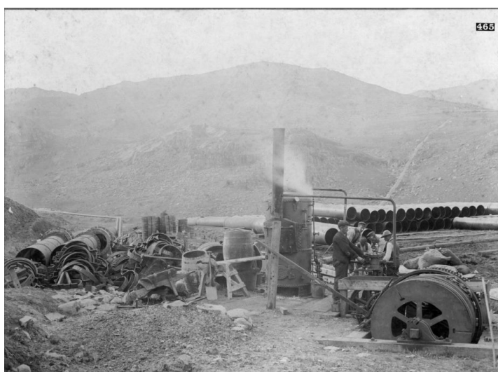
D34 : The steam haulage engines used for constructing the Marconi site were similar, if not identical to the ones used in 1905/6 for the construction of Cwm Dyli's supply pipes and power lines. Graham Isherwood considers that no permanent mounting was required for the haulage loads likely at Carnarvon, with temporary 'pegging' being sufficient to stabilise the system. Note the long brake lever. The engine is of a type widely advertised by Appleby Brothers of Southwark, London as being 'semi-portable', of which this may have been an example. Gwynedd Archives XS1245.6, under academic licence.
