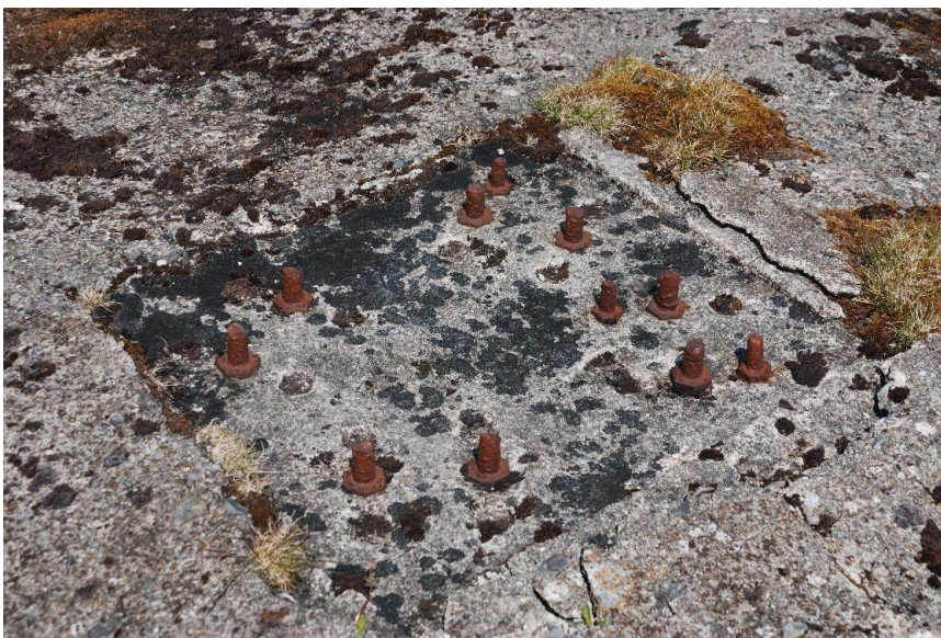
98. Bolts for attaching one of the three feet (Mast 12, foot A) of the 1923 extension masts. Central depression in base 26" x 24". This specific foot has the normal eight securing bolts set into the concrete, but also two, slightly smaller bolts at the inner side. All other pads show impressions of such bolts, which were presumably fixtures on the bottom metalwork of the mast that became fast in what must have been somewhat unset concrete at that point.
