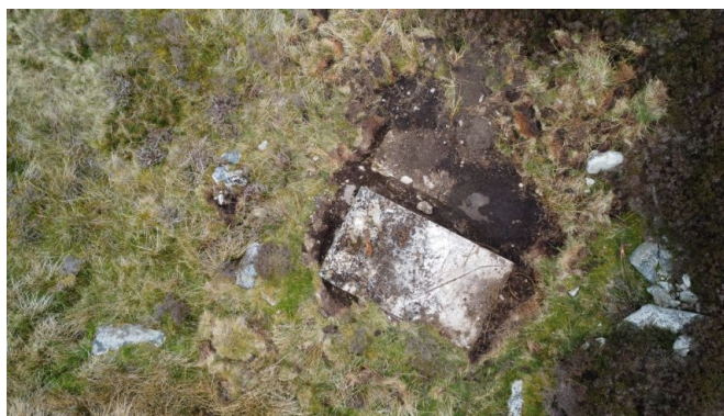
D32 , left: Main platform base after brush cleaning, showing narrow channel, draining to the rear and light impressions in the concrete surface, potentially those of double-bend pipework. The lime-rich concrete surface appears to be somewhat heat-modified at this point. Orientation as per arrow, 1ft gap between bases at far right, incline direction is to top centre (W-NW). D33 , below: aerial view of winder site.
