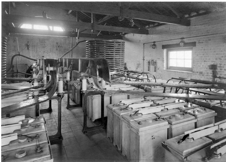
C20. The 'bridging' insulators seen at work, bridging glass-and-oil capacitor tanks of porcelain, in this case, in the transmitter building in 1918. The capacitors were a fundamental part of a resonating, so-called 'tank' circuit, acting in concert with the large inductor coils at background. Strips of copper conductor run inside the insulator channel. Image: Bodleian Special Collections, MS. Photogr.c.243, photograph number P.2072.
