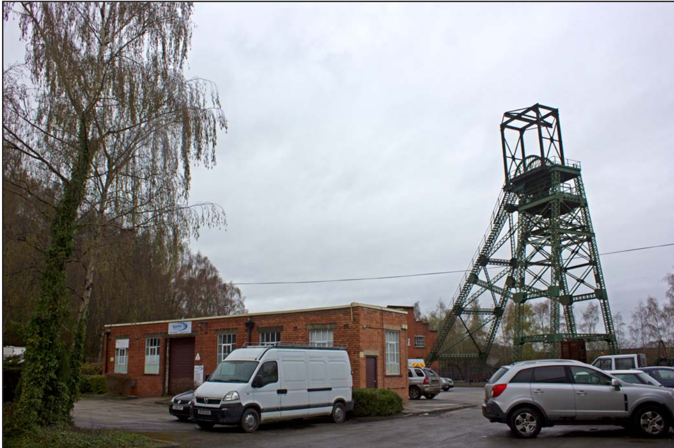
Plate 28: Bersham Bank Colliery, Offices & No.2 Winding Gear with Colliery Tip in Background, Plas Grono Road, Rhostyllen, Wrexham LL14 4EG - from the south
