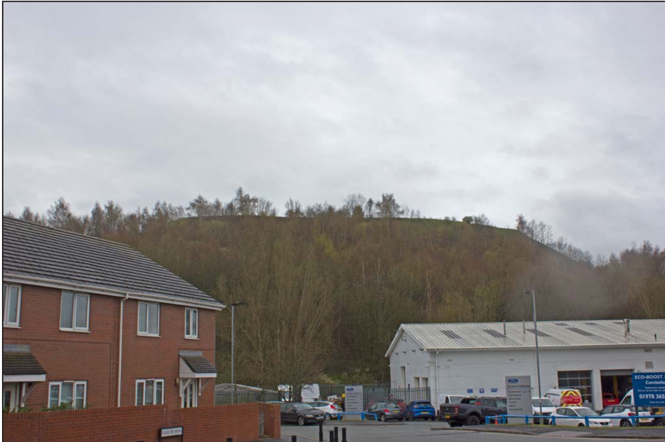
Plate 19: From ramp to Tudor Court/ Glan Yr Afon, shot of Bersham Bank Colliery Tip, Plas Grono Road, Rhostyllen, Wrexham LL14 4EG - from the north
