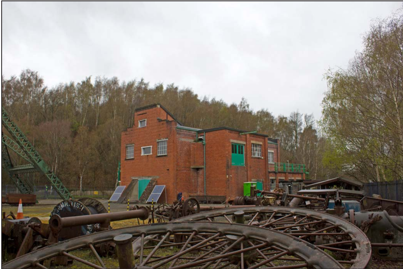
Plate 27: No.2 Winding Engine House with Colliery Tip in Background, Plas Grono Road, Rhostyllen, Wrexham LL14 4EG - from the east
