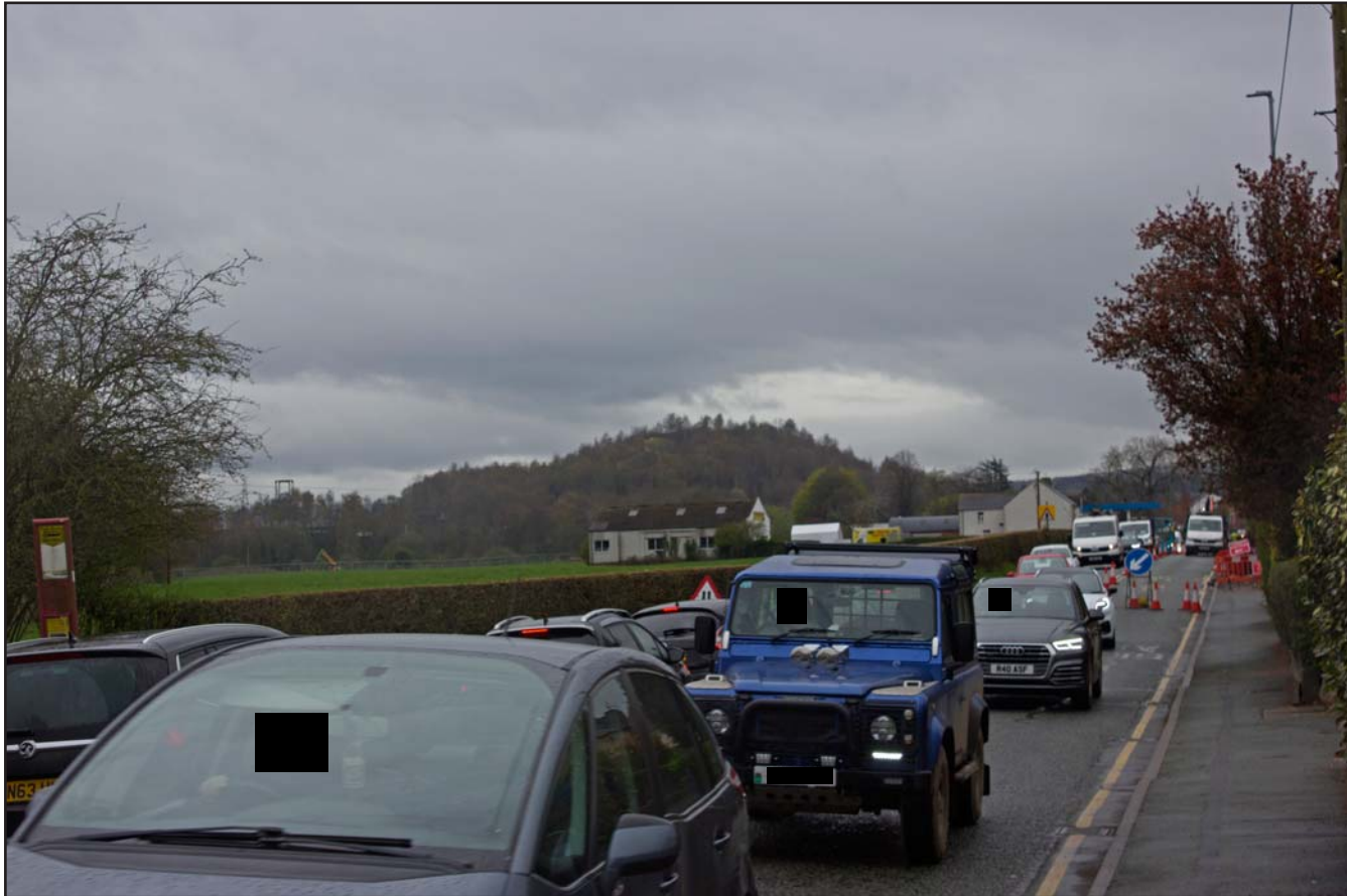
Plate 23: From Wrexham Road (A5152) near Old Farm Road, context shot of Bersham Bank Colliery Tip, Plas Grono Road, Rhostyllen, Wrexham LL14 4EG - from the northeast
