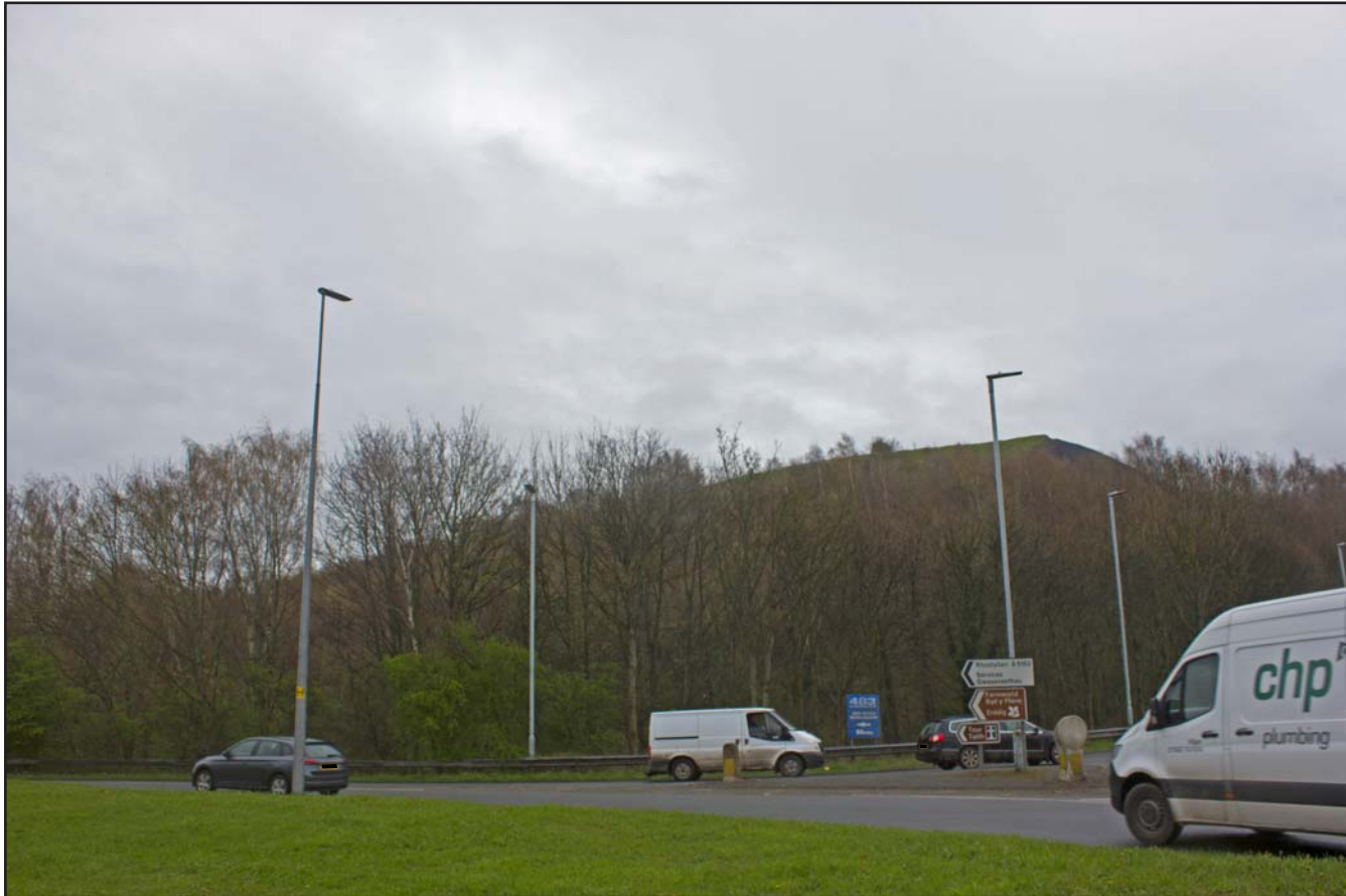
Plate 22: From Croesfoel Interchange, shot of Bersham Bank Colliery Tip, Plas Grono Road, Rhostyllen, Wrexham LL14 4EG - from the northwest
