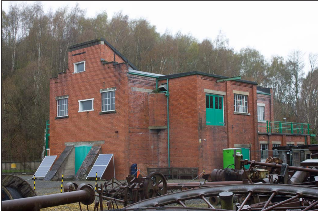
Plate 35: Engine Winding House with Colliery Tip in Background, Plas Grono Road, Rhostyllen, Wrexham LL14 4EG - from the east
