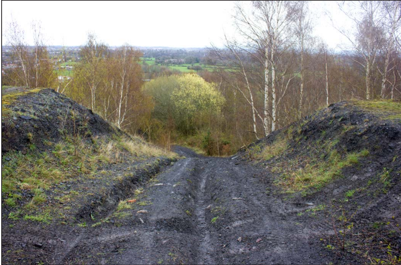
Plate 54: View of northeast access track on Bersham Bank Colliery Tip, Plas Grono Road, Rhostyllen, Wrexham LL14 4EG - from the southwest
