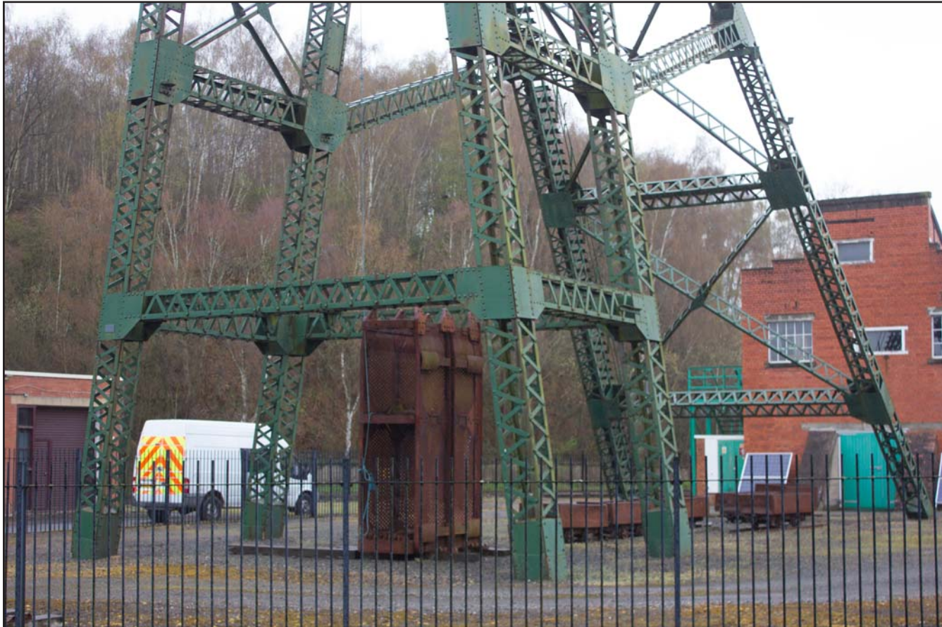
Plate 33: Base of No.2 Winding Gear & left side of Engine Winding House with Colliery Tip in Background, Plas Grono Road, Rhostyllen, Wrexham LL14 4EG - from the east
