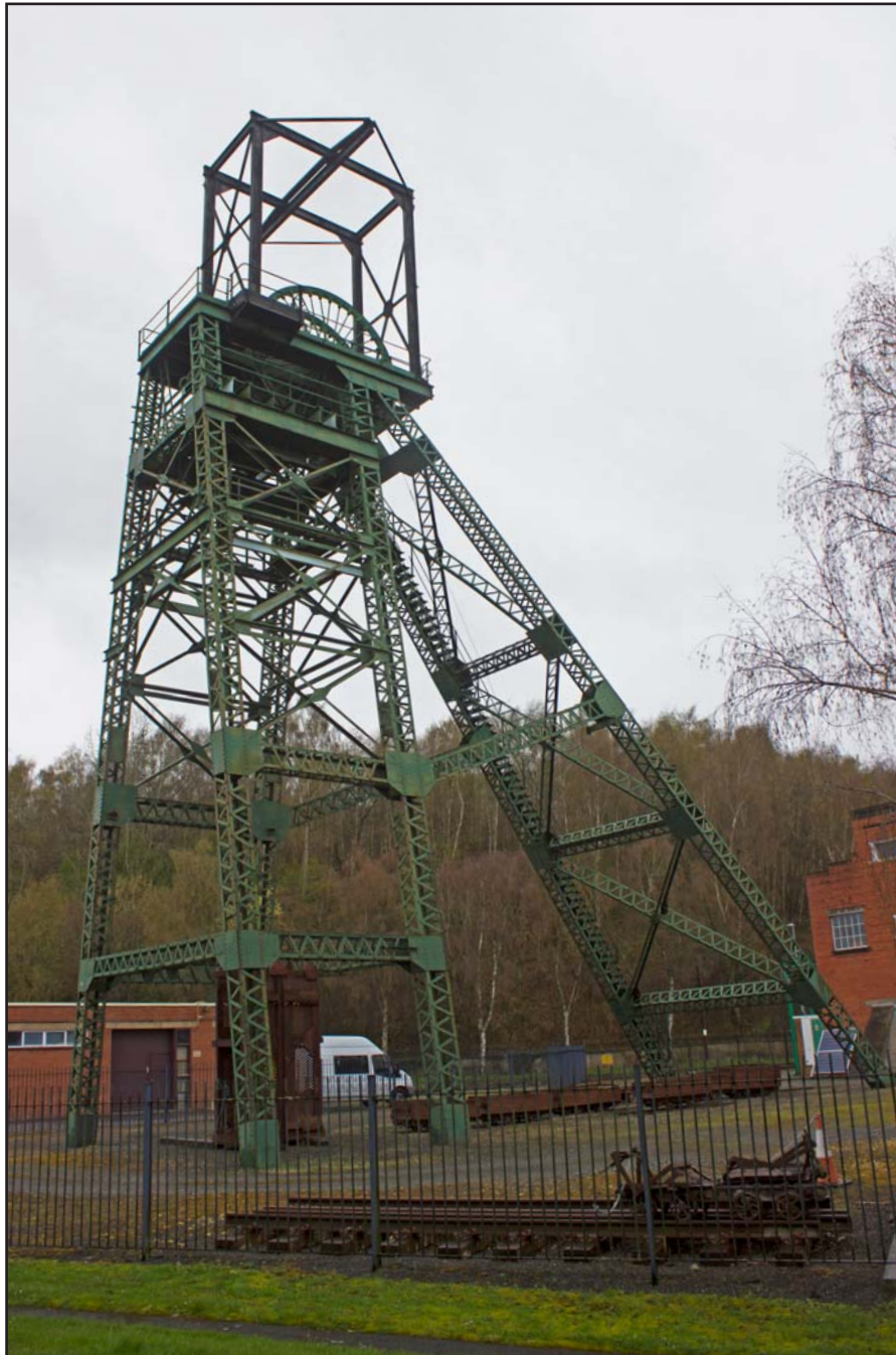
Plate 26: No.2 Winding Gear with Colliery Tip in Background, Plas Grono Road, Rhostyllen, Wrexham LL14 4EG - from the east
