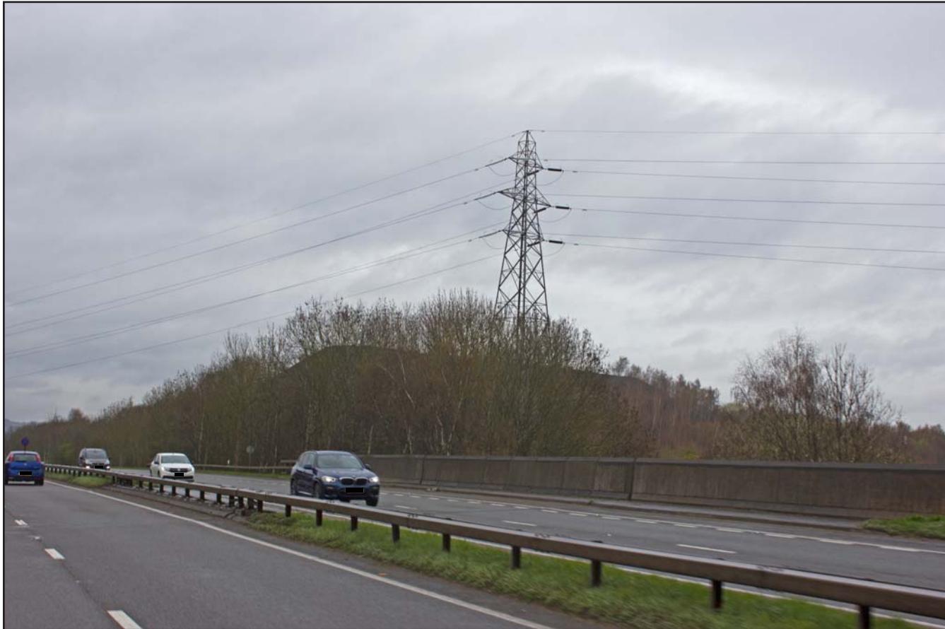
Plate 15: From A483 northbound approach, Context shot of Bersham Bank Colliery Tip, Plas Grono Road, Rhostyllen, Wrexham LL14 4EG - from the southwest
