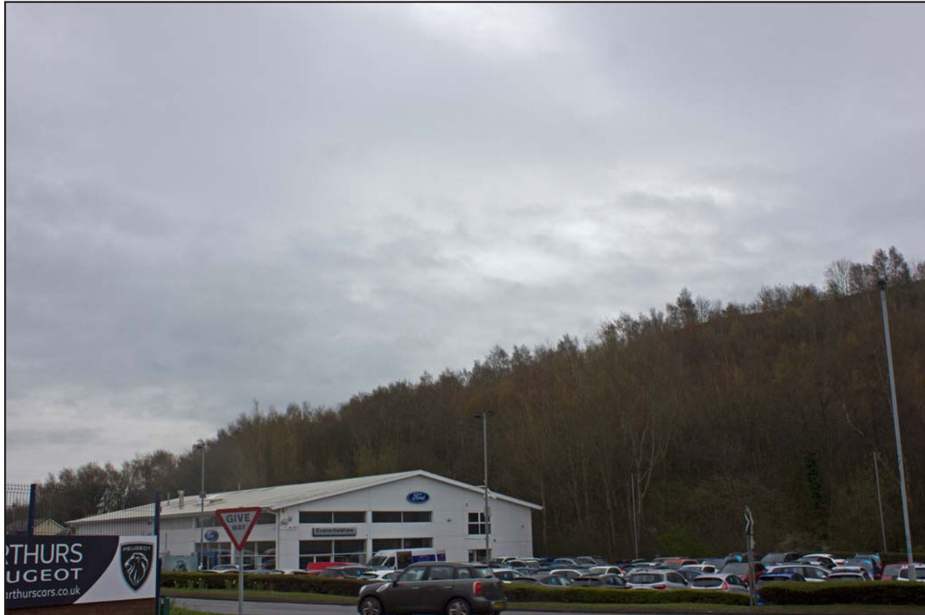
Plate 21: From Esso Garage, shot of Bersham Bank Colliery Tip (east half) , Plas Grono Road, Rhostyllen, Wrexham LL14 4EG - from the west
