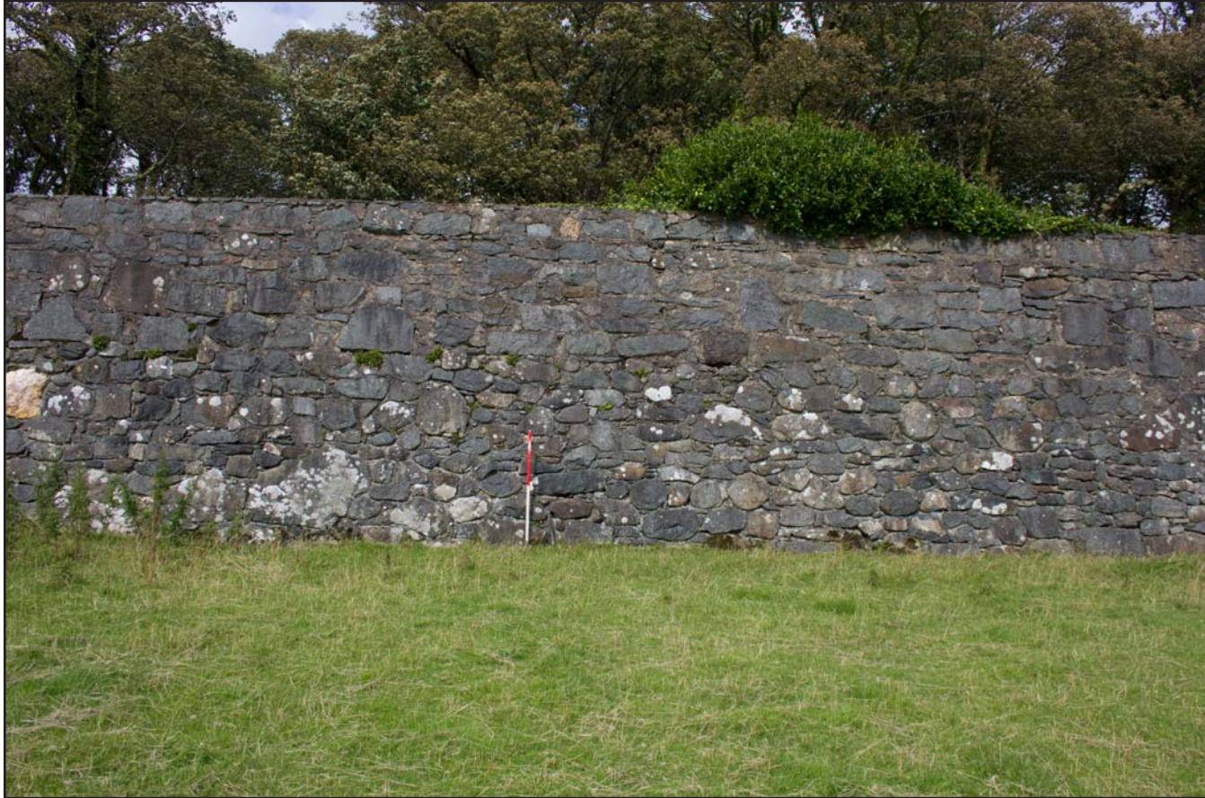
Plate 13: Field boundary wall (GAT PRN: 81361; feature 8) , from the south. Scale 1.0m.
