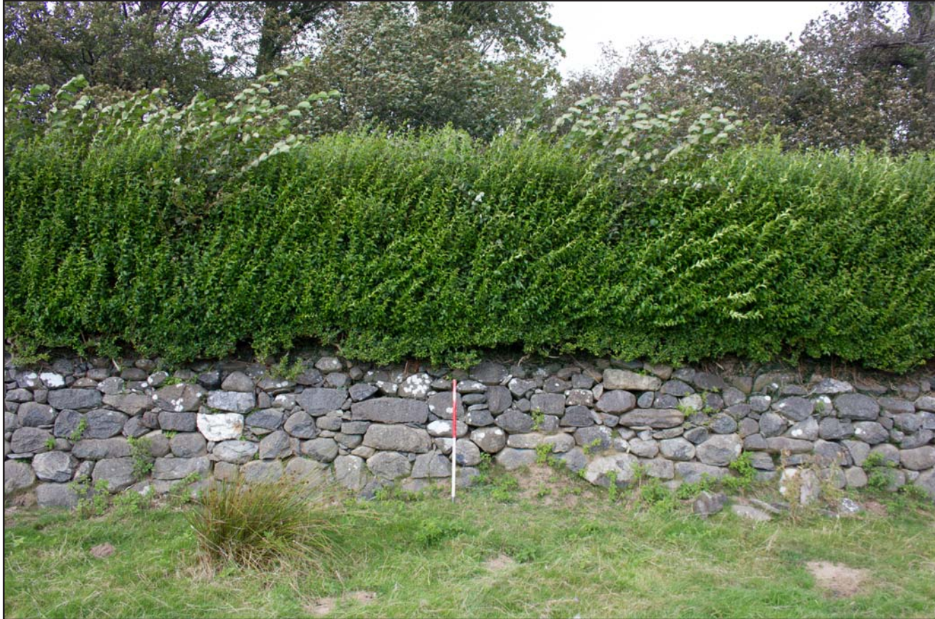
Plate 05: Field boundary wall (GAT PRN: 81354; feature 1) , from the south. Scale 1.0m.
