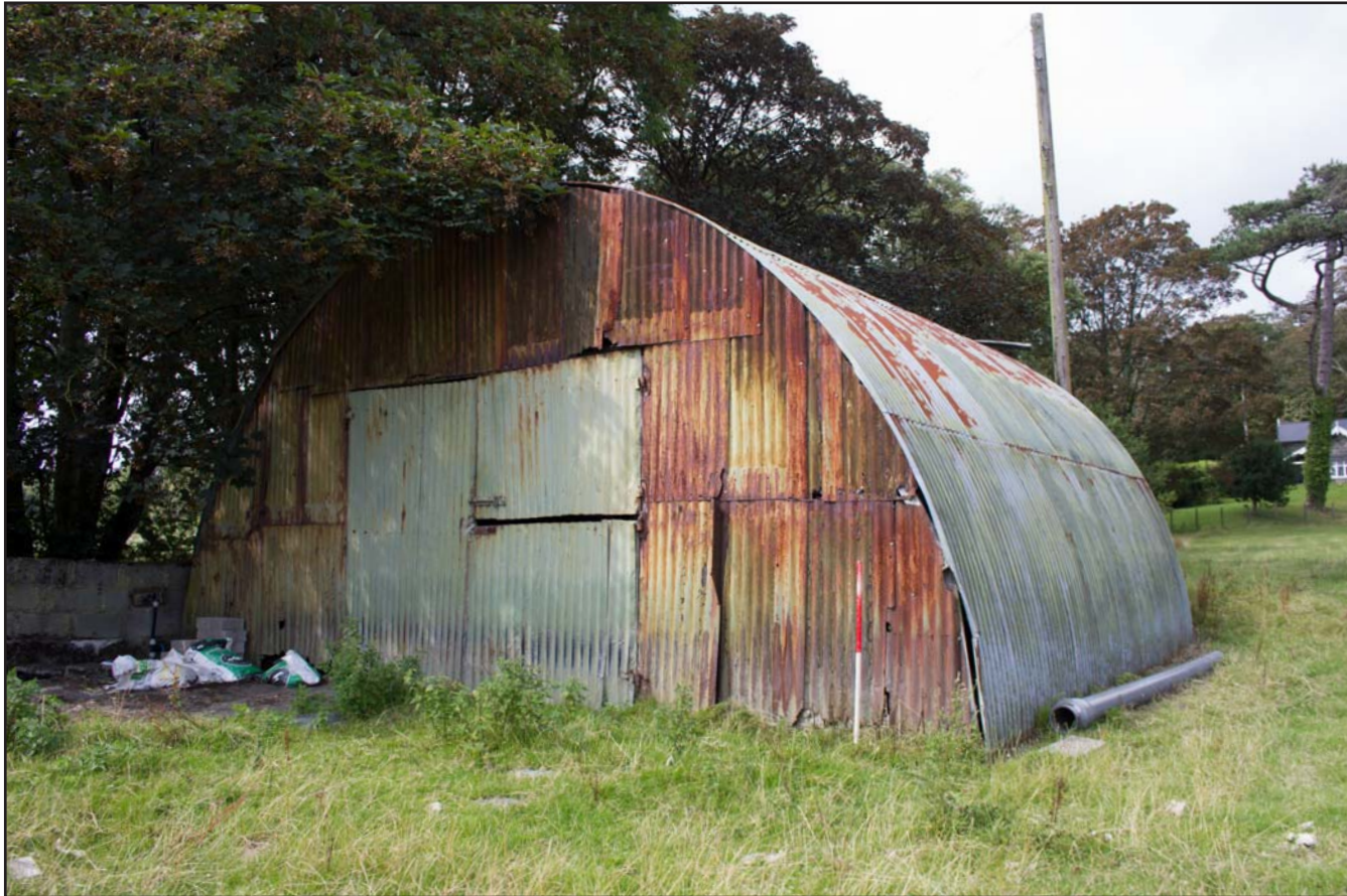
Plate 06: Corrugated iron barn (GAT PRN: 81355; feature 2) , from the southeast. Scale 1.0m.
