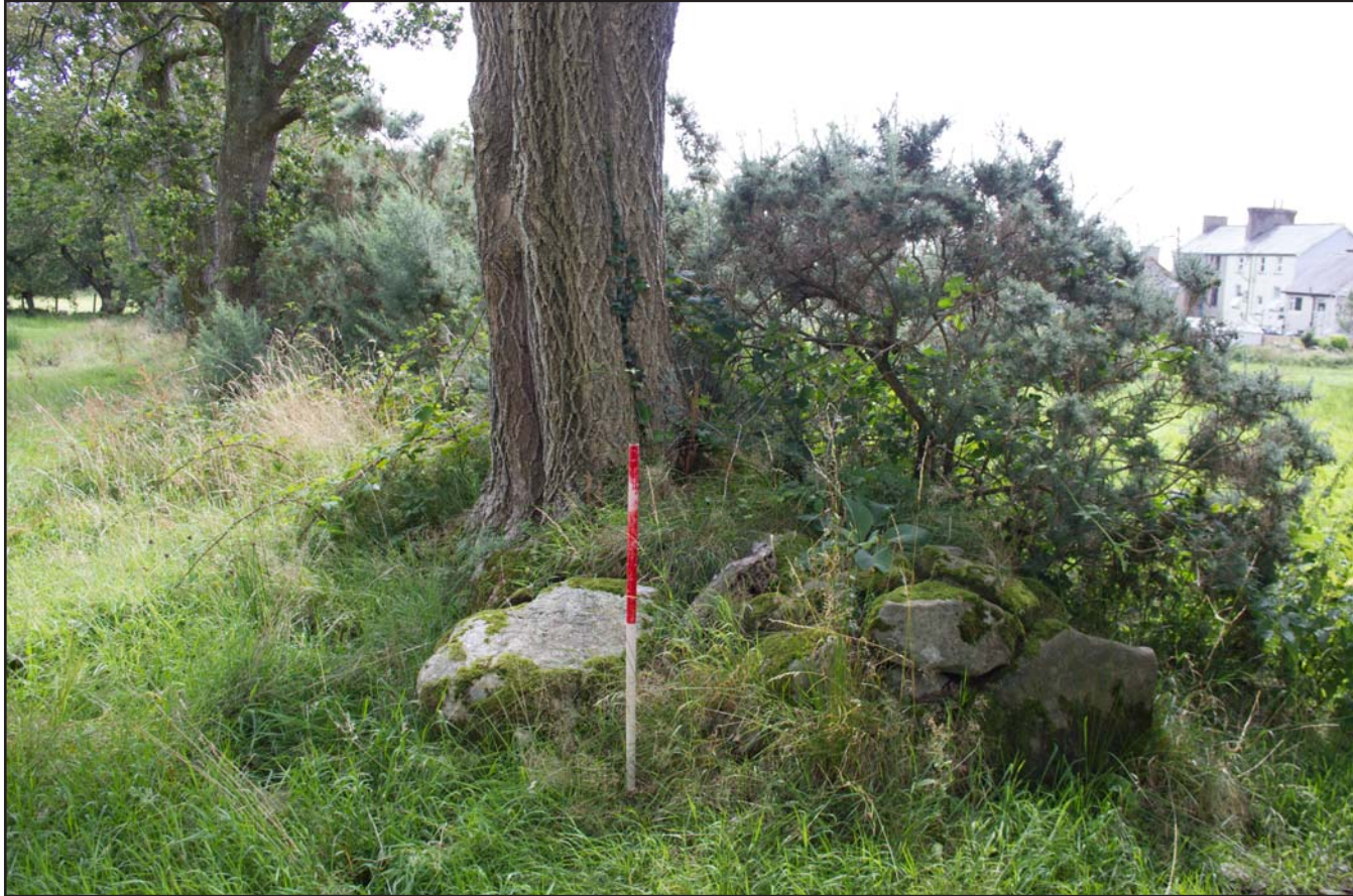
Plate 15: Field boundary wall- fields 5 and 6 (feature 3 / GAT PRN 81350), from the north. Scale 1.0m.
