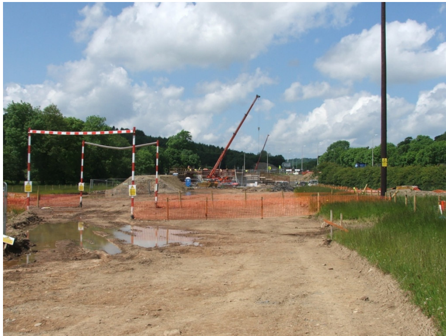
Plate 2: Road strip for '2+1 Road' looking west from Canaston Bridge Roundabout
