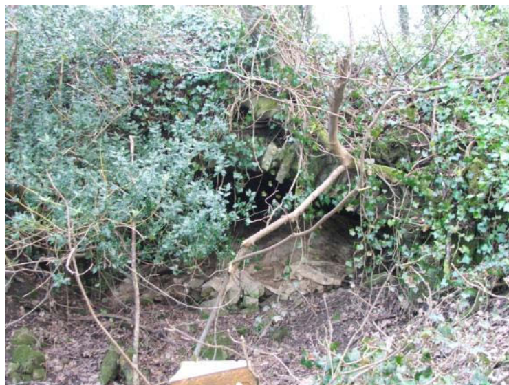
Plate 7: former Canaston Bridge prior to vegetation clearance and removal.
