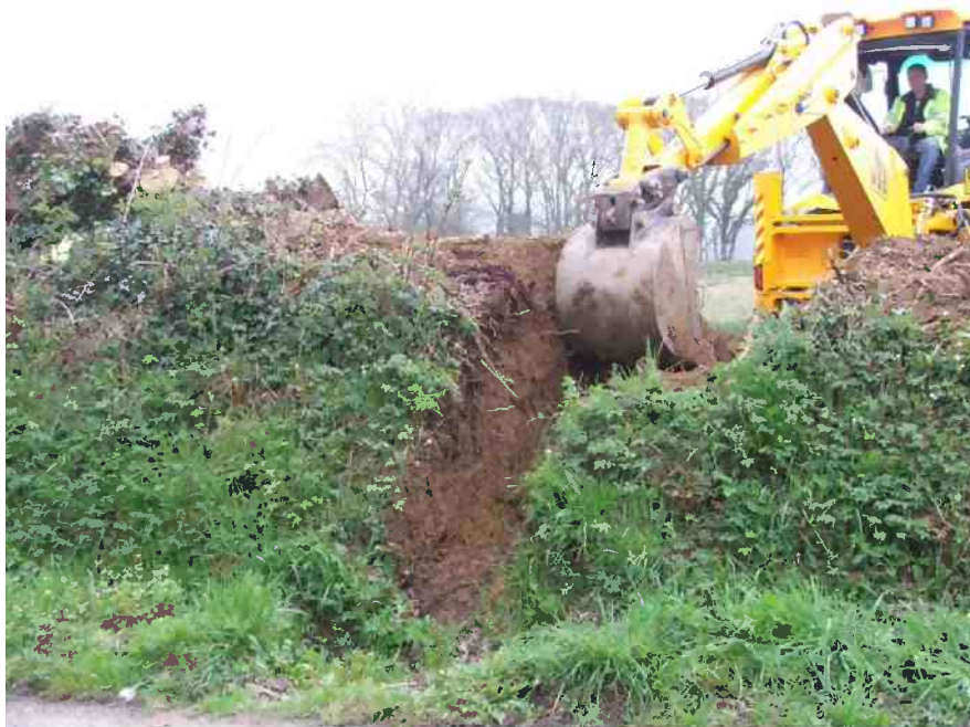
Plate 1: Removal of hedge bank to the north of the A40 at Toch Lane
