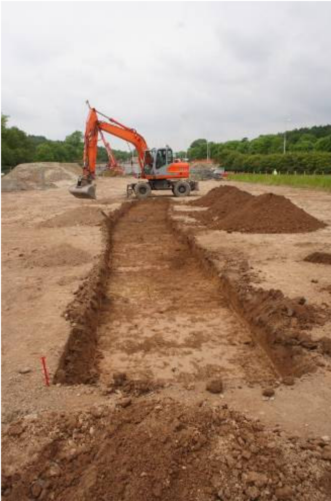
Photo 21: Trench 1 looking west
