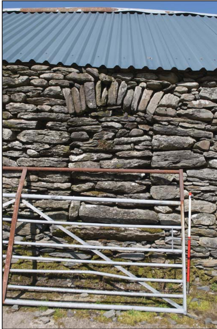
Plate 13: Exterior - Close-up of window infilled with stone in SE wall of barn; scale 1x1m; view from SE (archive reference: G2778_013).
