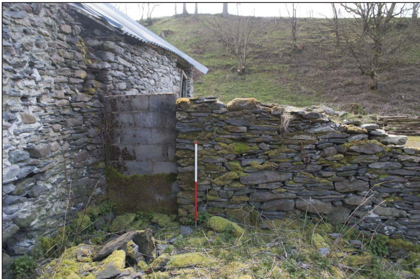
Plate 43: Interior Cottage - View of blocked up doorway into cottage; scale 1x1 m; view from NE (archive reference: G2778_043).
