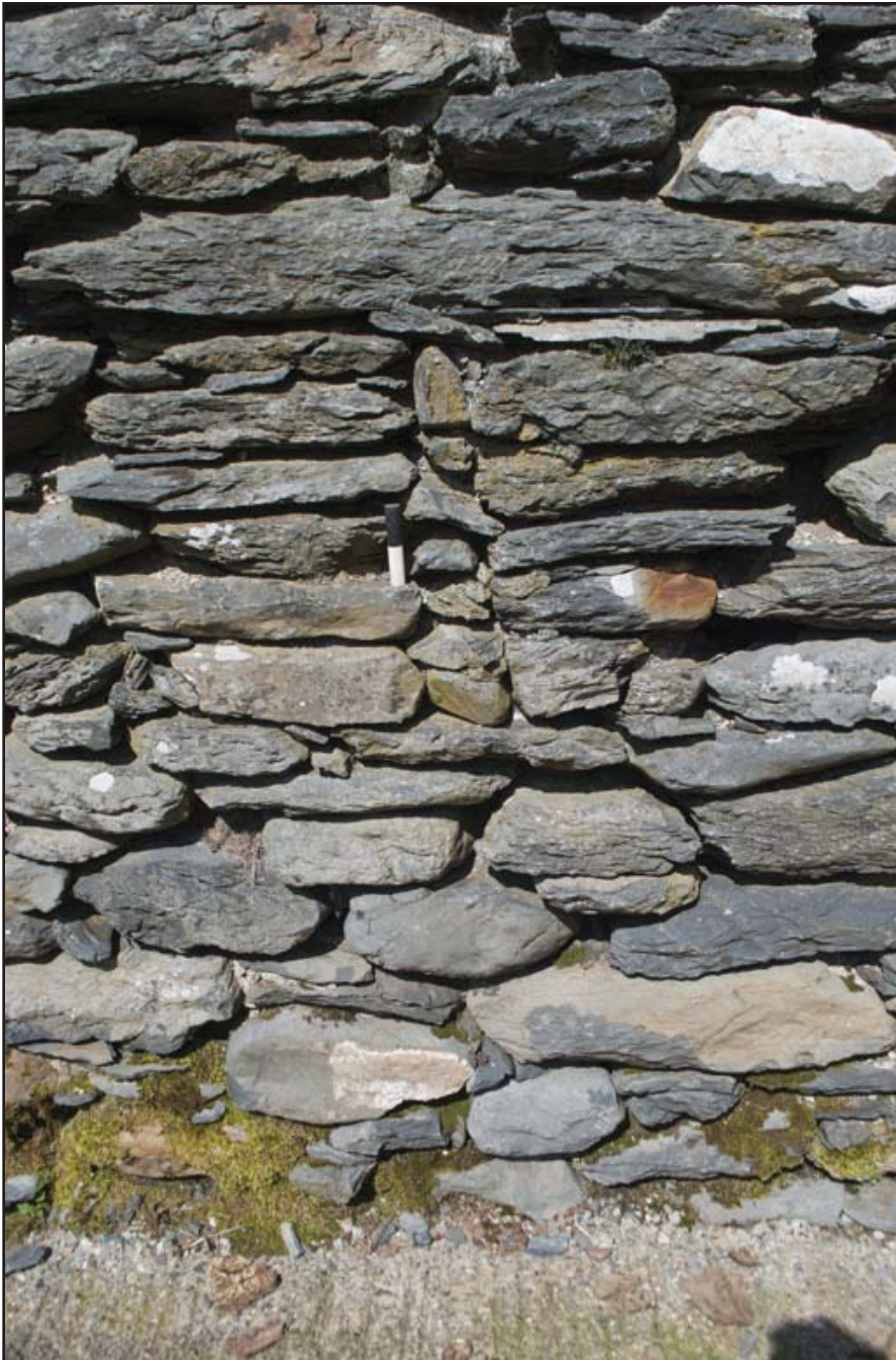
Plate 11: Exterior - Infilled ventilation slit in SE wall of barn; scale 0.10 m; view from SE (archive reference: G2778_011).
