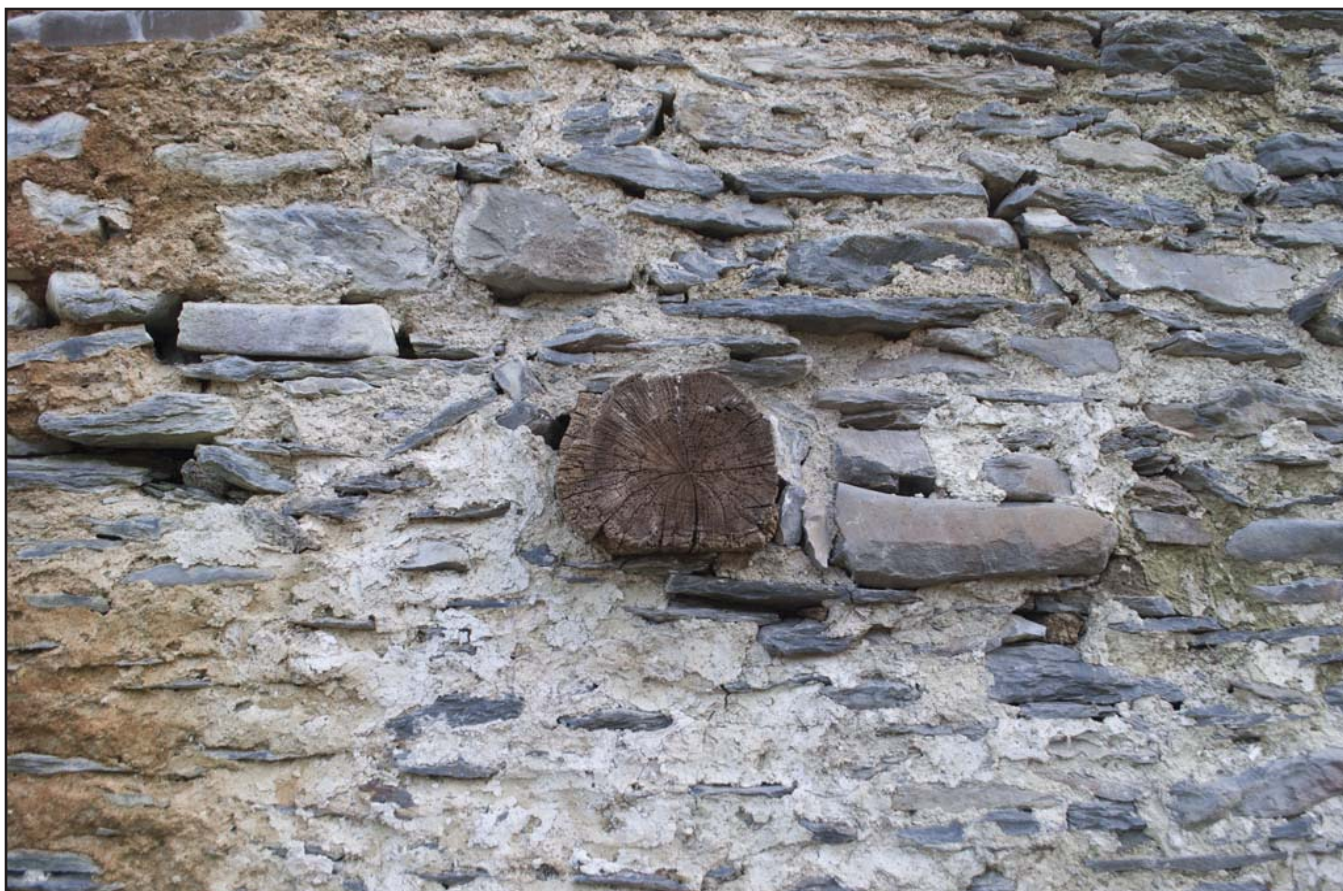
Plate 44: Interior Cottage - Close-up view of wooden beam protruding from SE gable end of the cottage; scale not used; view from N (archive reference: G2778_044).
