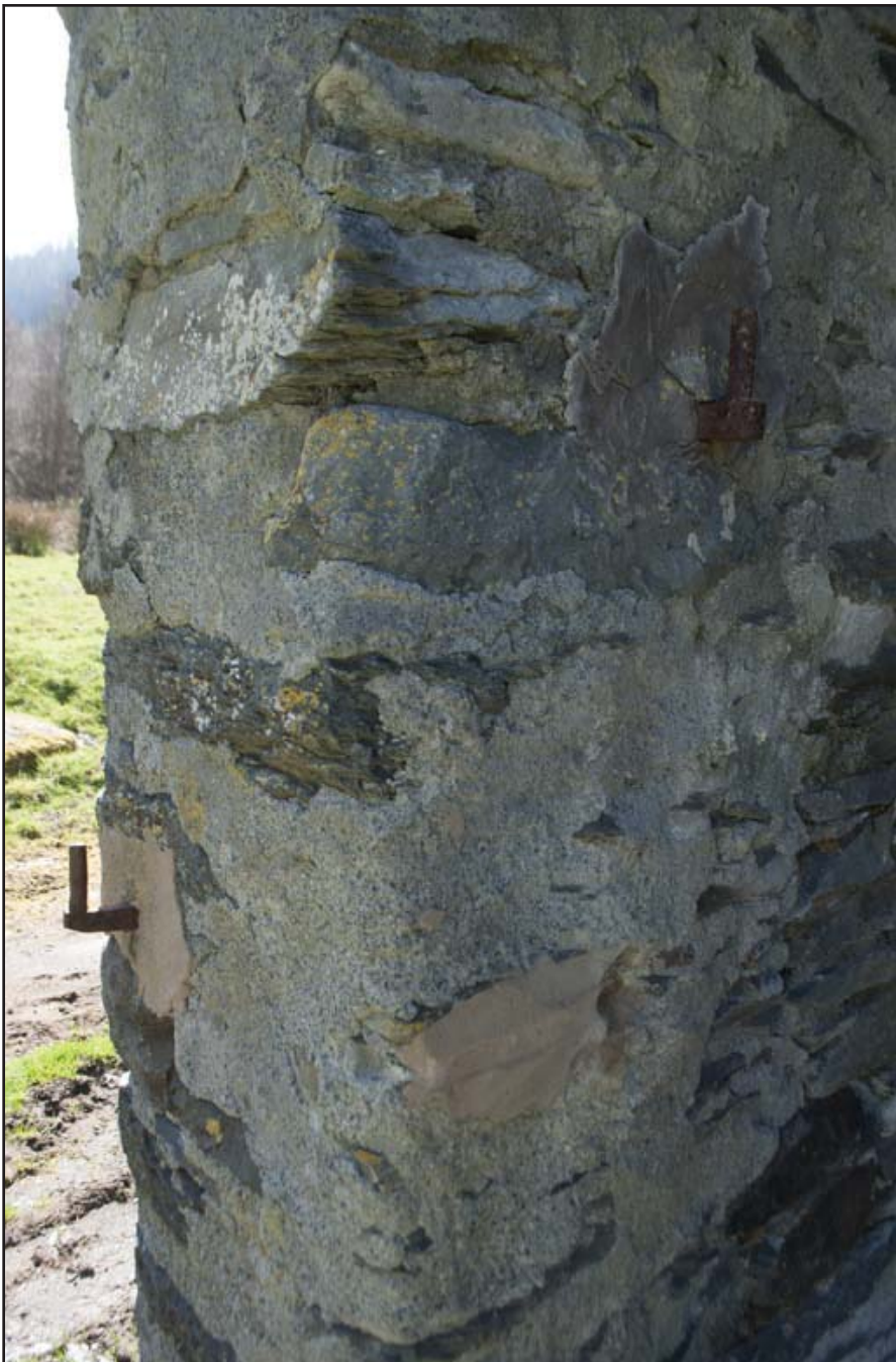
Plate 21: Exterior - Close-up of metal pins for gate in large entrance to barn; scale not used; view from N (archive reference: G2778_021).
