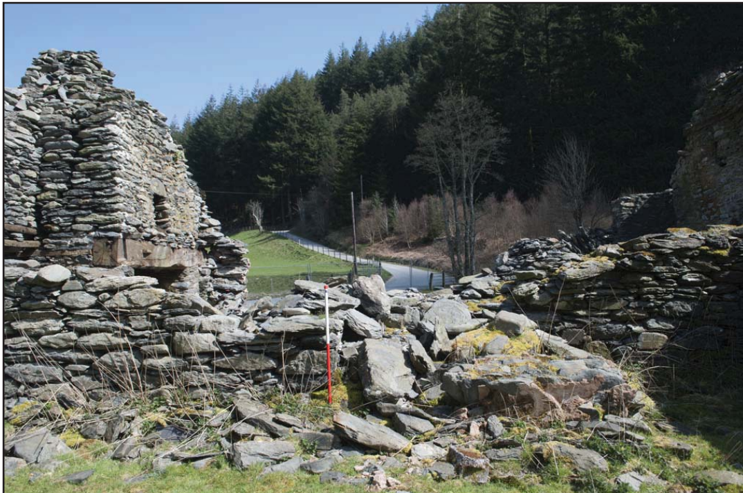
Plate 17: Exterior - View of collapsed SW wall of cottage and fireplace within; scale 1x1m; view from SW (archive reference: G2778_017).
