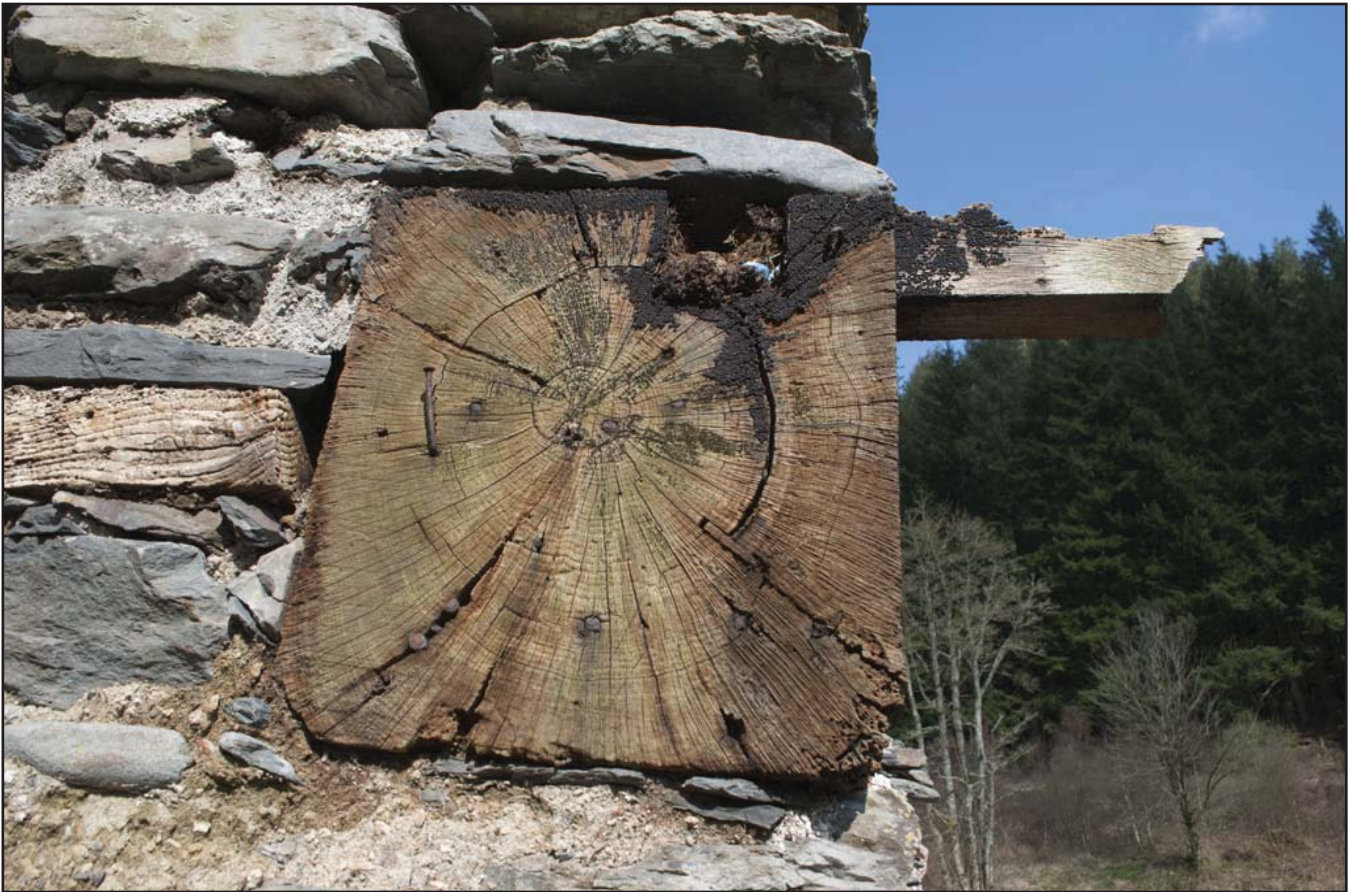
Plate 55: Interior Cottage - Close-up of wooden fireplace lintel; scale not used; view from SW (archive reference: G2778_055).
