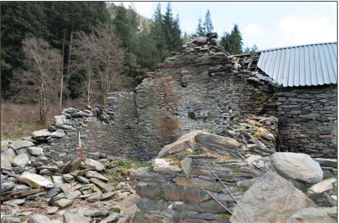
Plate 50: Interior Cottage - View of the NE wall of the cottage showing collapse, large concrete block; scale 1x1m; view from W (archive reference: G2778_050).
