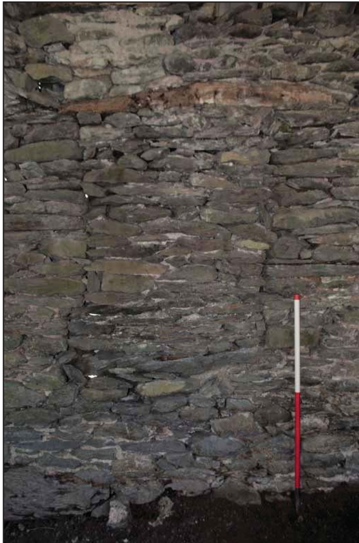
Plate 27: Interior Barn - View of window infilled with stone; scale 1x1m; view from N (archive reference: G2778_027).
