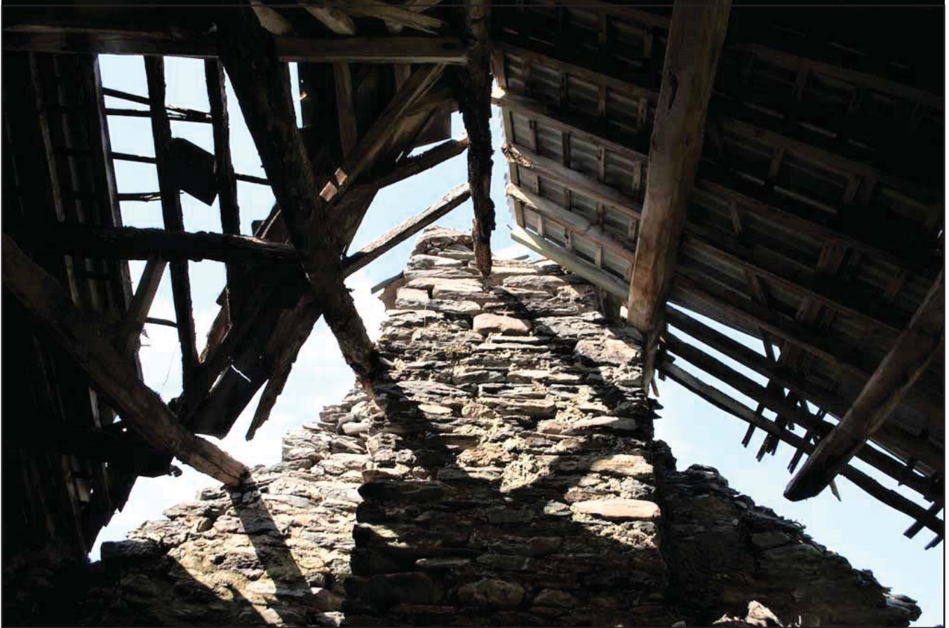
Plate 33: Interior Barn - View of collapsed roof above fireplace in barn; scale not used; view from S (archive reference: G2778_033).
