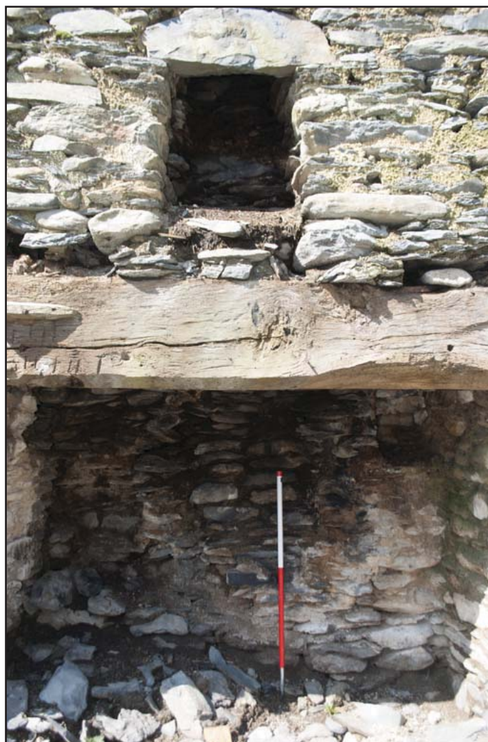
Plate 40: Interior Cottage - Close-up view of fireplace showing first floor fireplace above and small alcove in the right hand corner; scale 1x1m; view from SE (archive reference: G2778_040).
