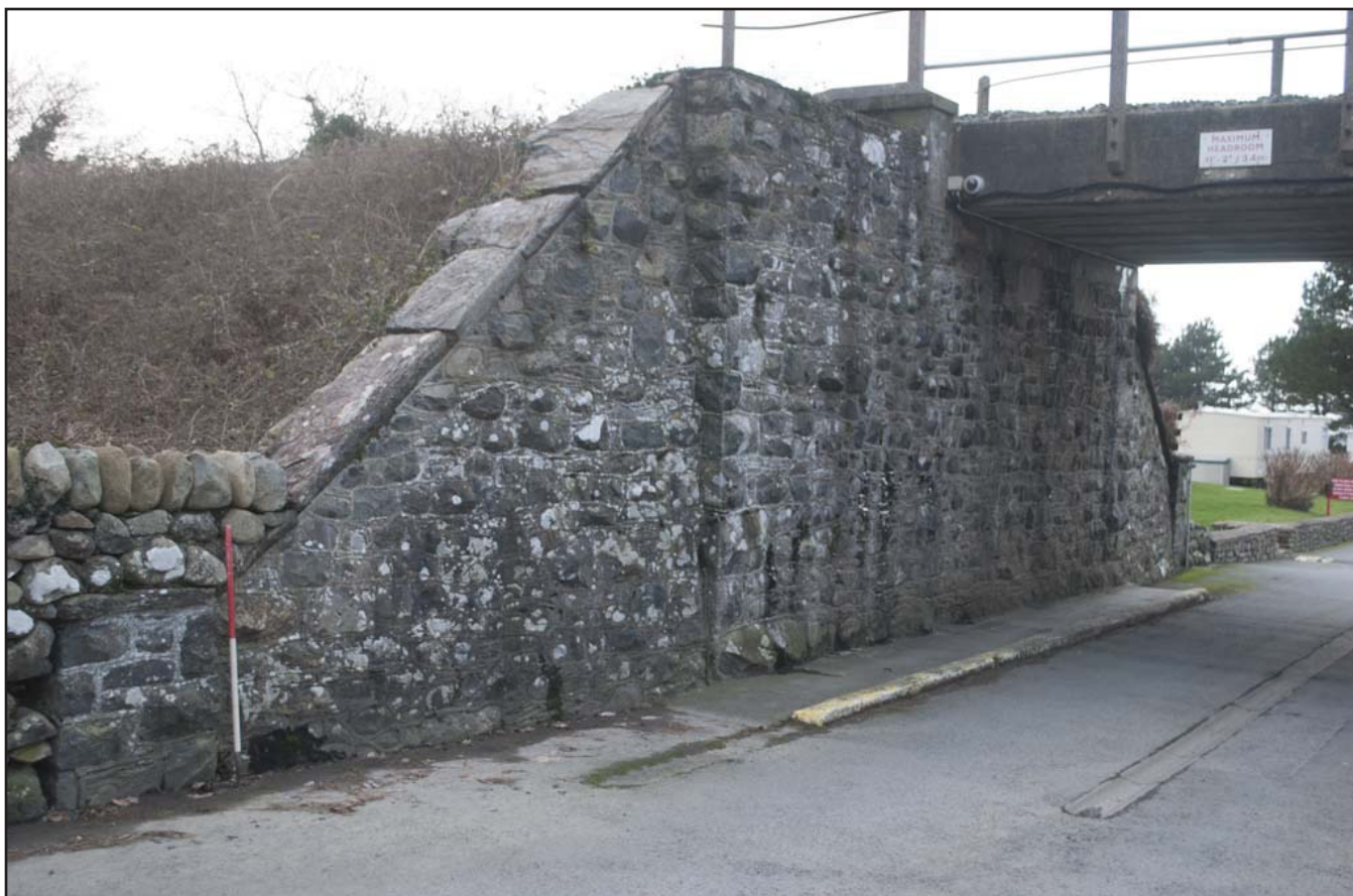
Plate 2: Angled view showing 19th century snecked granite railway bridge abutment on SE side; scale 1m; view from E (archive reference: G2760_02).
