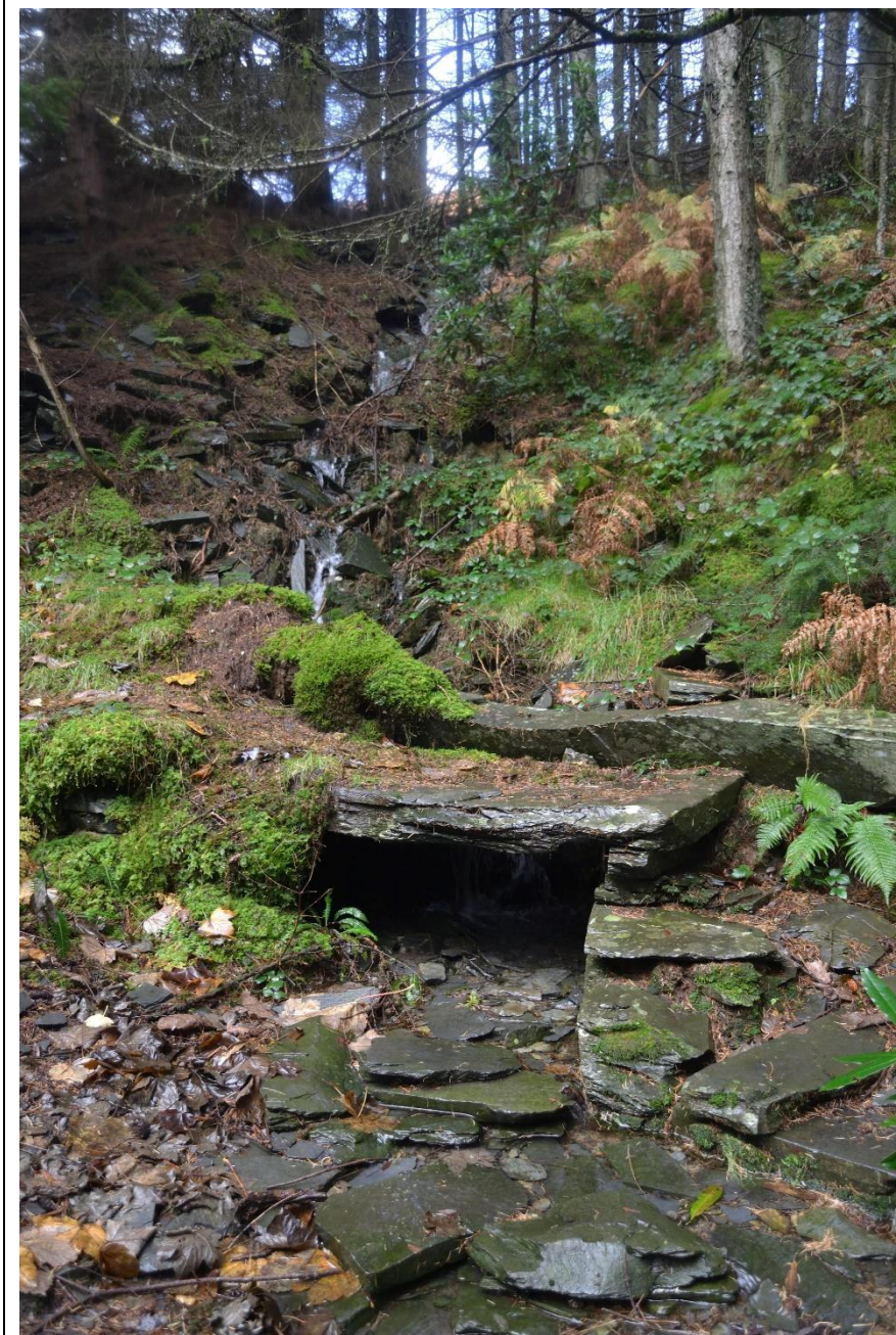
Bridge on the Quarry Path, from SE (archive reference: G2754_0028)
