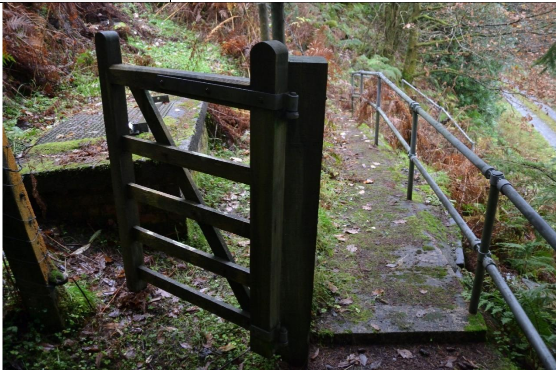
Structure over water intake and concrete access steps from E (archive reference: G2754_0063)
