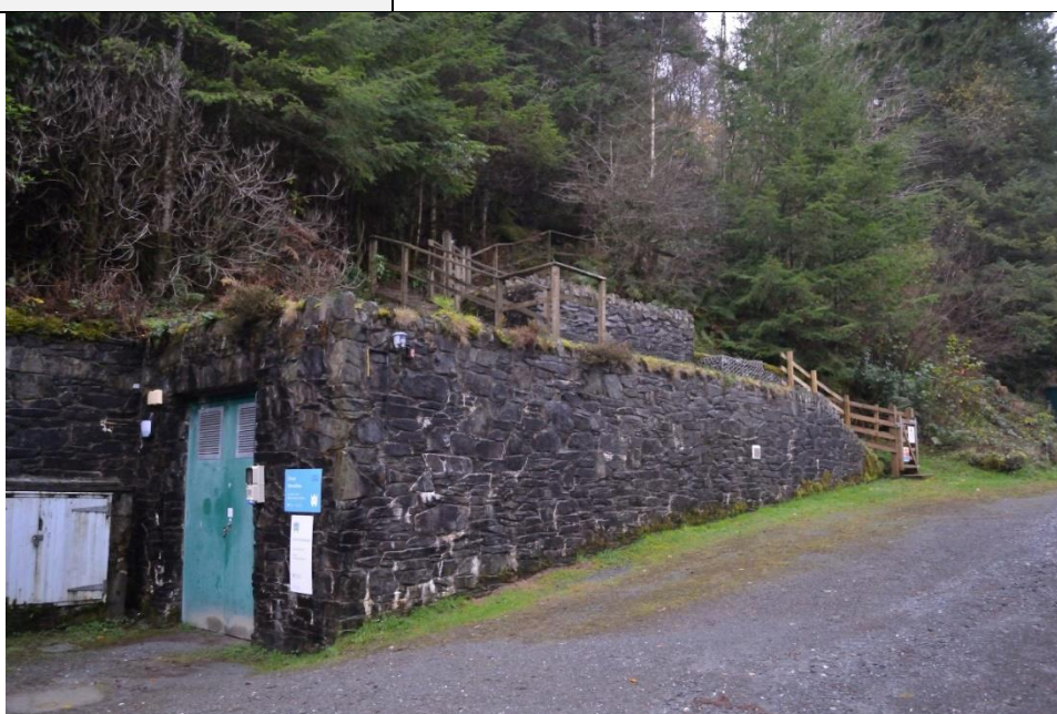
Water works building with steps up to the reservoir from SE (archive reference: G2754_0082)
