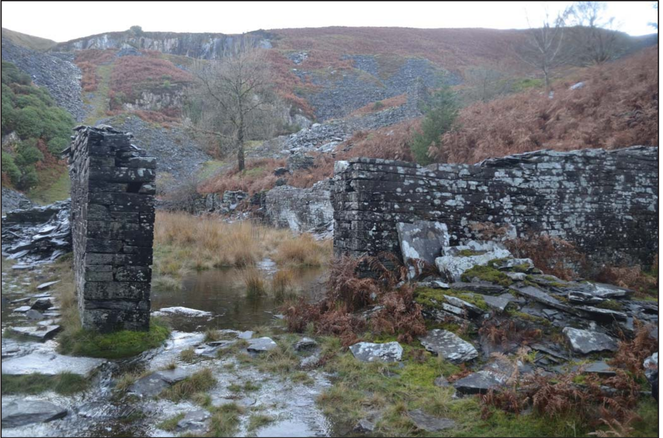
Plate 4. Slate processing mill PRN 99016 from east-north-east (archive reference: G2754_0030)
