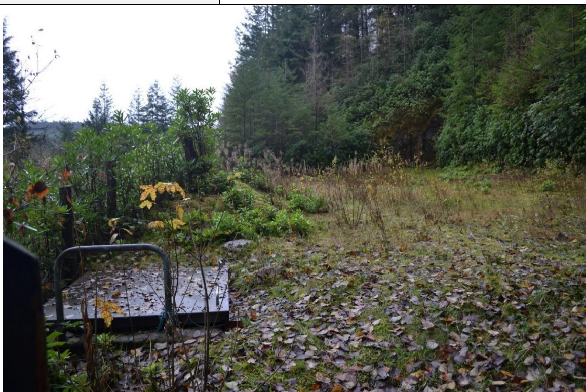
Covered reservoir inside the old quarry from NW (archive reference: G2754_0076)
