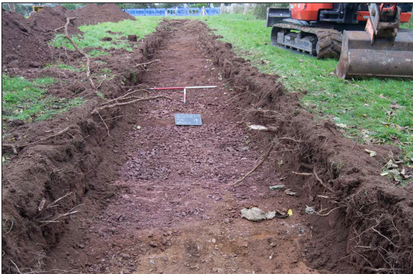
Plate 02: Pipe trench after topsoil and subsoil removed at the southern end of the field; scale: 2x1m (archive reference: G2557_009).
