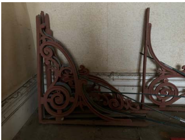
Figure 3, 4 and 5 above and right- salvaged cast iron fretwork to the front supporting columns of the pedestrian walkway. These shall be cleaned down, fitted and repainted
