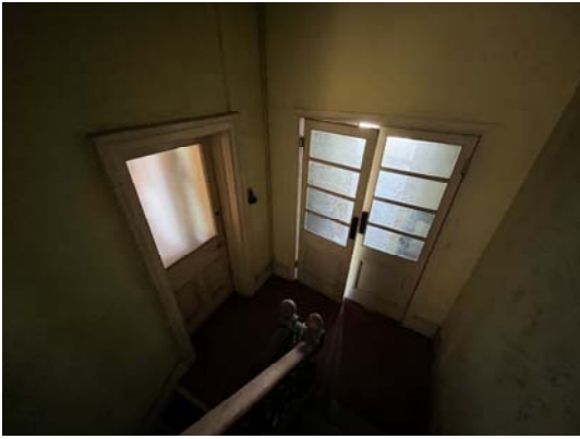
Figure 10 left – first floor landing- number 3 showing double door entry into accommodation
