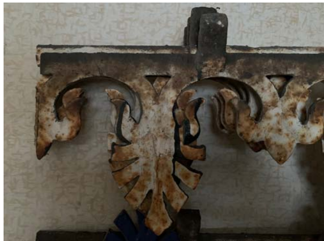
Figure 3, 4 and 5 above and right- salvaged cast iron fretwork to the front supporting columns of the pedestrian walkway. These shall be cleaned down, fitted and repainted
