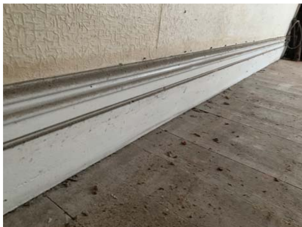
Figure 9 left – skirting section within the main property
