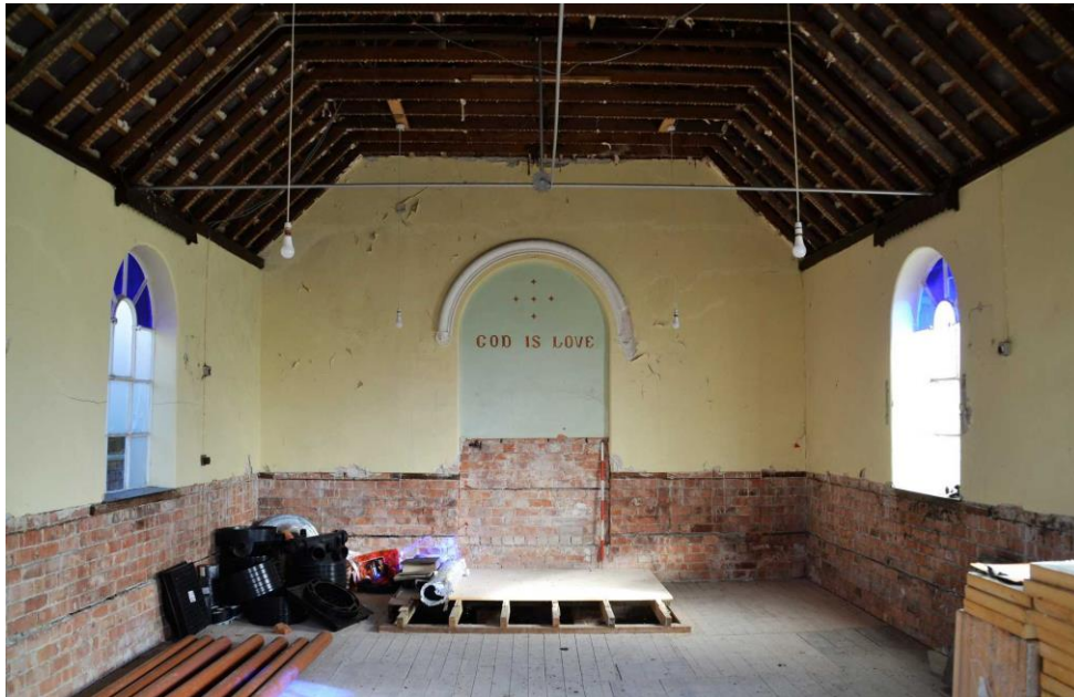
Fig. 6 South-facing interior elevation showing round-headed recess CPAT 4981_018
