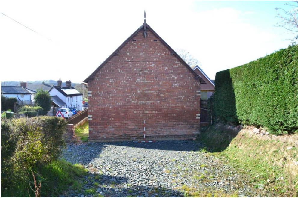
Fig. 4 North-facing elevation of the building Photo CPAT 4981_005
