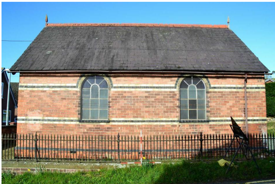
Fig. 5 East-facing elevation of the building Photo CPAT 4981_004
