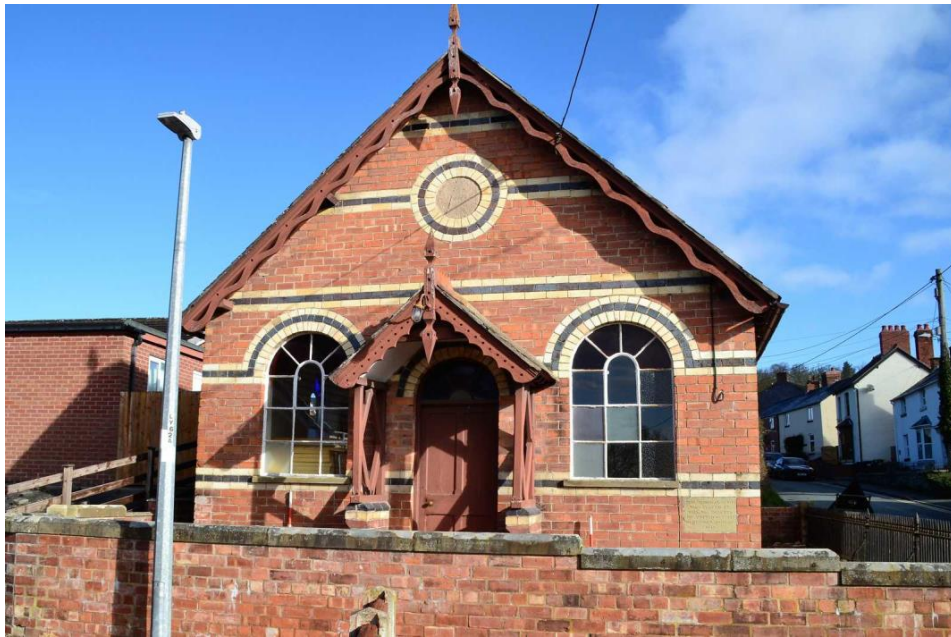
Fig. 3 Southern facing elevation of the building Photo CPAT 4981_001
