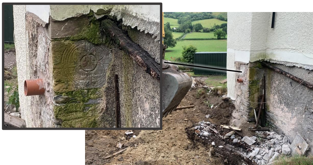
Fig. 3 Carved medieval stonework built into chimney stack CPAT photo 5018-9 and 28
