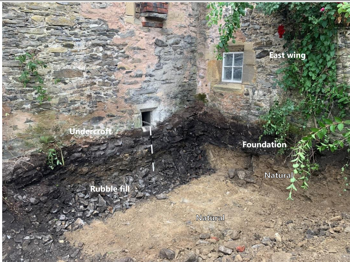
Fig. 7 Photo showing rubble-filled cut along undercroft wall CPAT photo 5018-20
