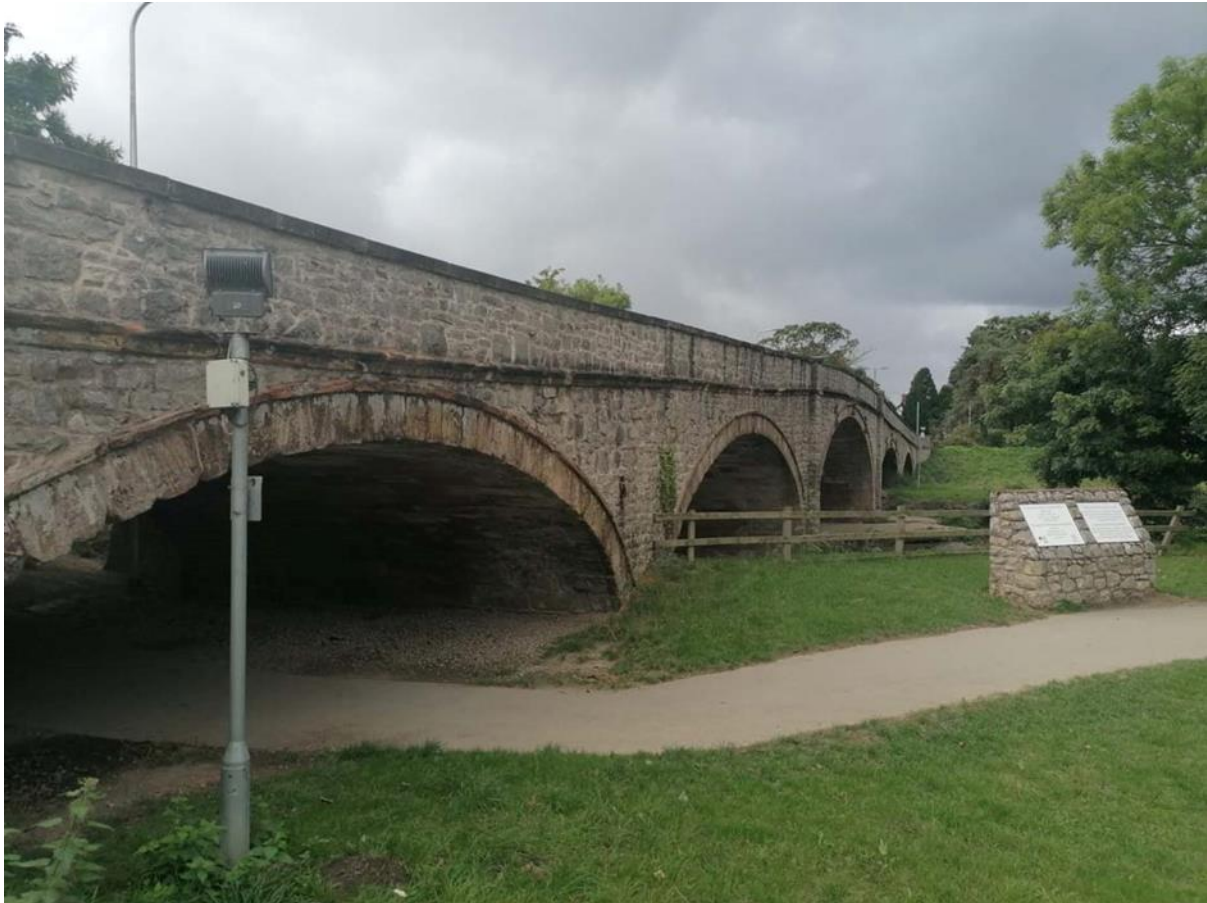
Figure 3 St Asaph bridge scheduled monument
