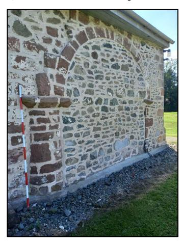
Figure 3. Bricked in aisle arch. Photo CPAT 2646-0013
