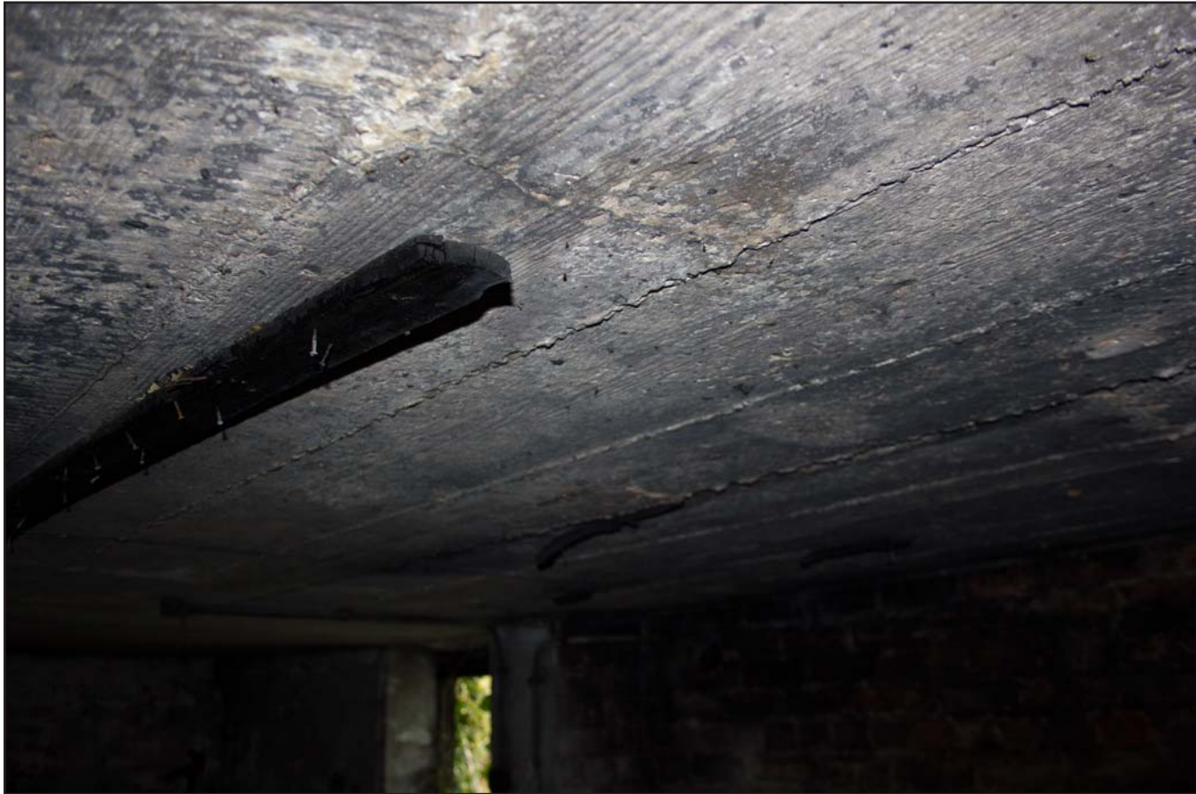
Plate 14: Air Raid Shelter 1 Main Room showing ceiling brackets, from the east.
