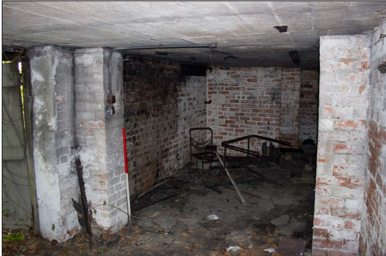
Plate 13: Air Raid Shelter 1 Main Room, from the south. Scale 1.0m.
