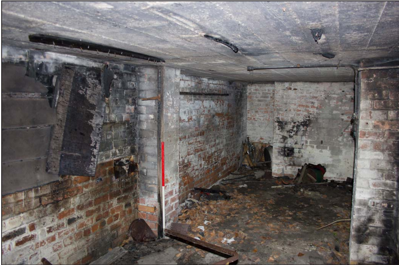
Plate 12: Air Raid Shelter 1 Main Room, from the north. Scale 1.0m.
