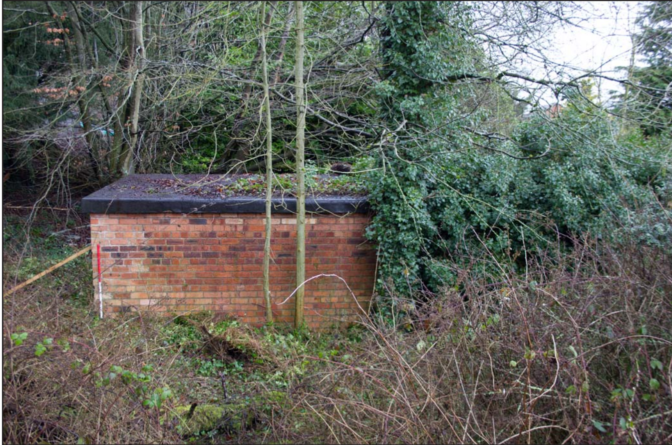
Plate 01: Air Raid Shelter 1 southeast facing external elevation, from the southeast. Scale 1.0m.
