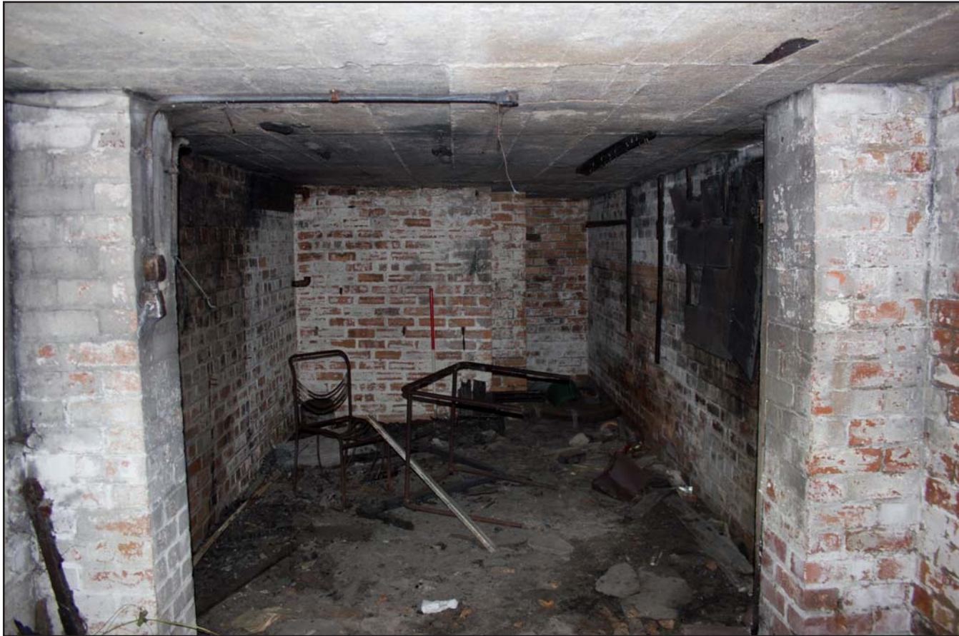
Plate 10: Air Raid Shelter 1 Main Room, from the southwest. Scale 1.0m.
