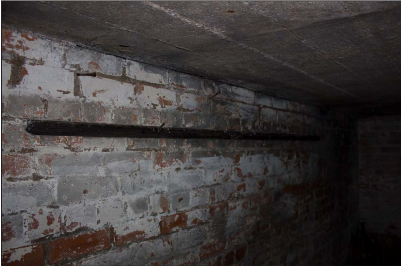
Plate 18: Air Raid Shelter 1 Main Room showing coat hook rail, from the north.
