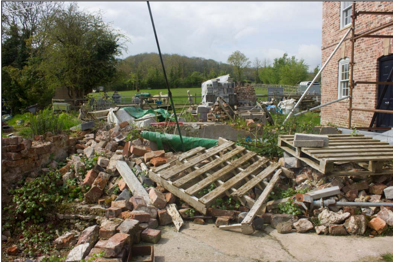
Plate 09: Interior of southwest elevation of the outbuilding at the Farmhouse, Panton Hall, Old Bagillt Rd, Bagillt, Flintshire - from the northeast - 1.00m scale
