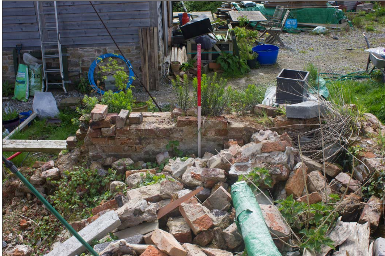
Plate 08: Interior of southeast elevation of the outbuilding at the Farmhouse, Panton Hall, Old Bagillt Rd, Bagillt, Flintshire - from the northwest - 1.00m scale
