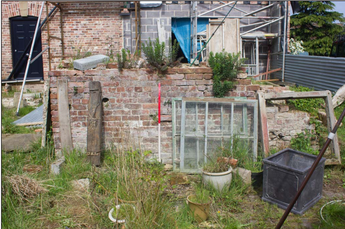
Plate 04: Southeast elevation of the outbuilding at the Farmhouse, Panton Hall, Old Bagillt Rd, Bagillt, Flintshire - from the southeast - 1.00m scale
