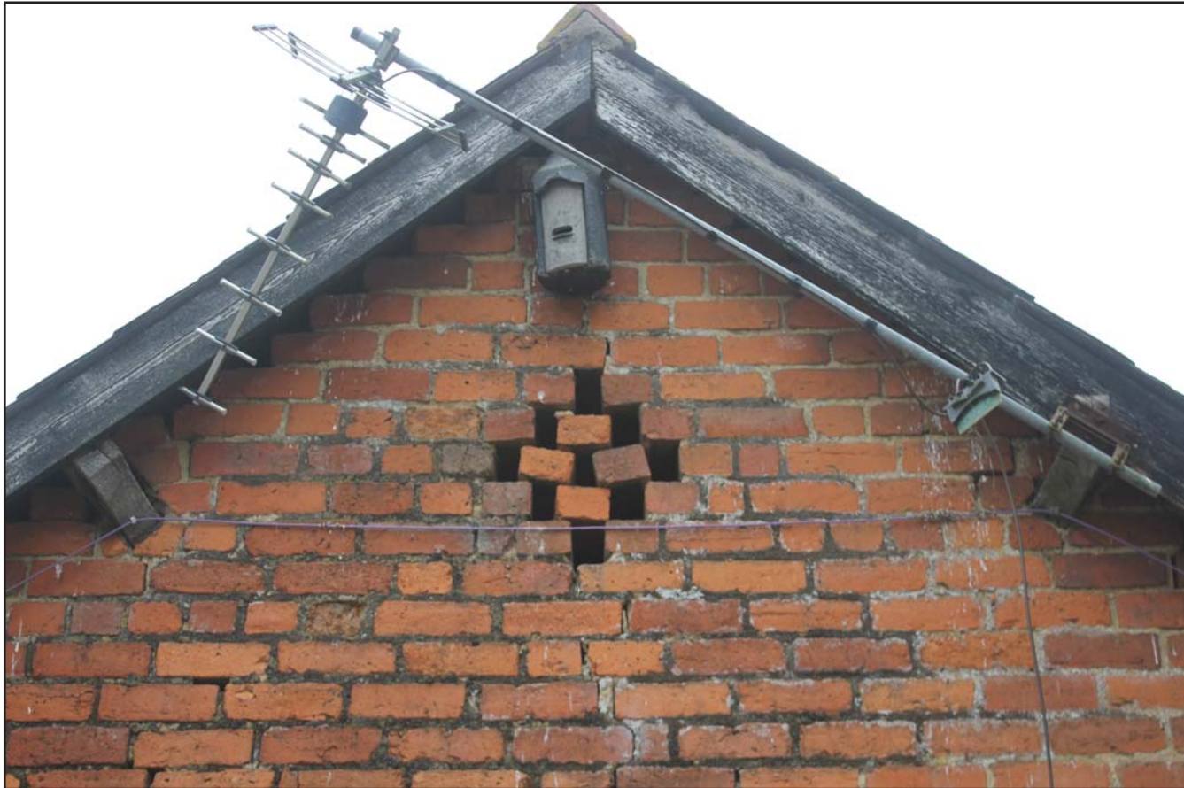
Plate 19: Western elevation, diaper/diamond shaped ventilation embrasure on the outbuilding at The Birches, Rhos-Y-Meirch, Knighton, Powys - from the west - no scale
