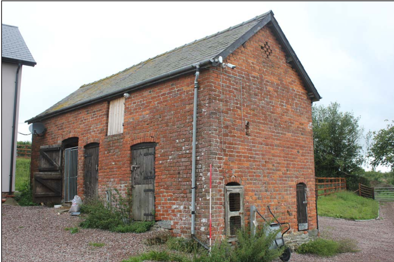
Plate 04: Oblique shot of southern and eastern elevations of the outbuilding at The Birches, Rhos-Y-Meirch, Knighton, Powys - from the southeast - 2.00m scale
