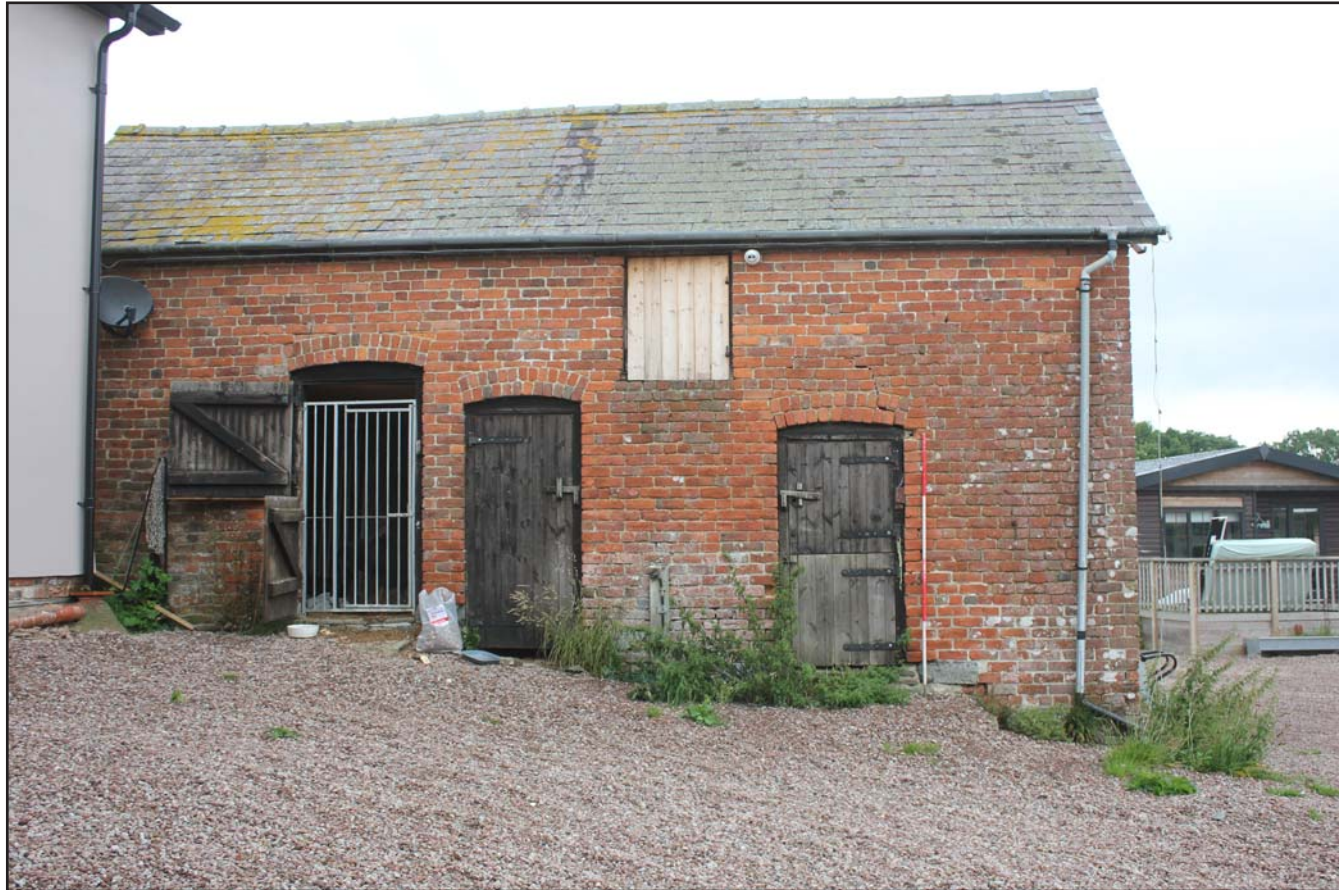
Plate 03: Southern elevation of the outbuilding at The Birches, Rhos-Y-Meirch, Knighton, Powys - from the south - 2.00m scale
