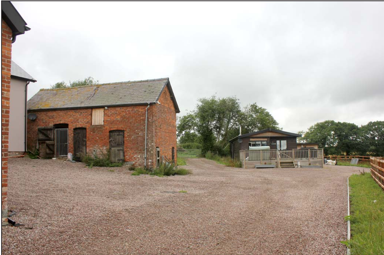
Plate 01: Context shot of outbuilding at The Birches, Rhos-Y-Meirch, Knighton, Powys - from the south - 2.00m scale
