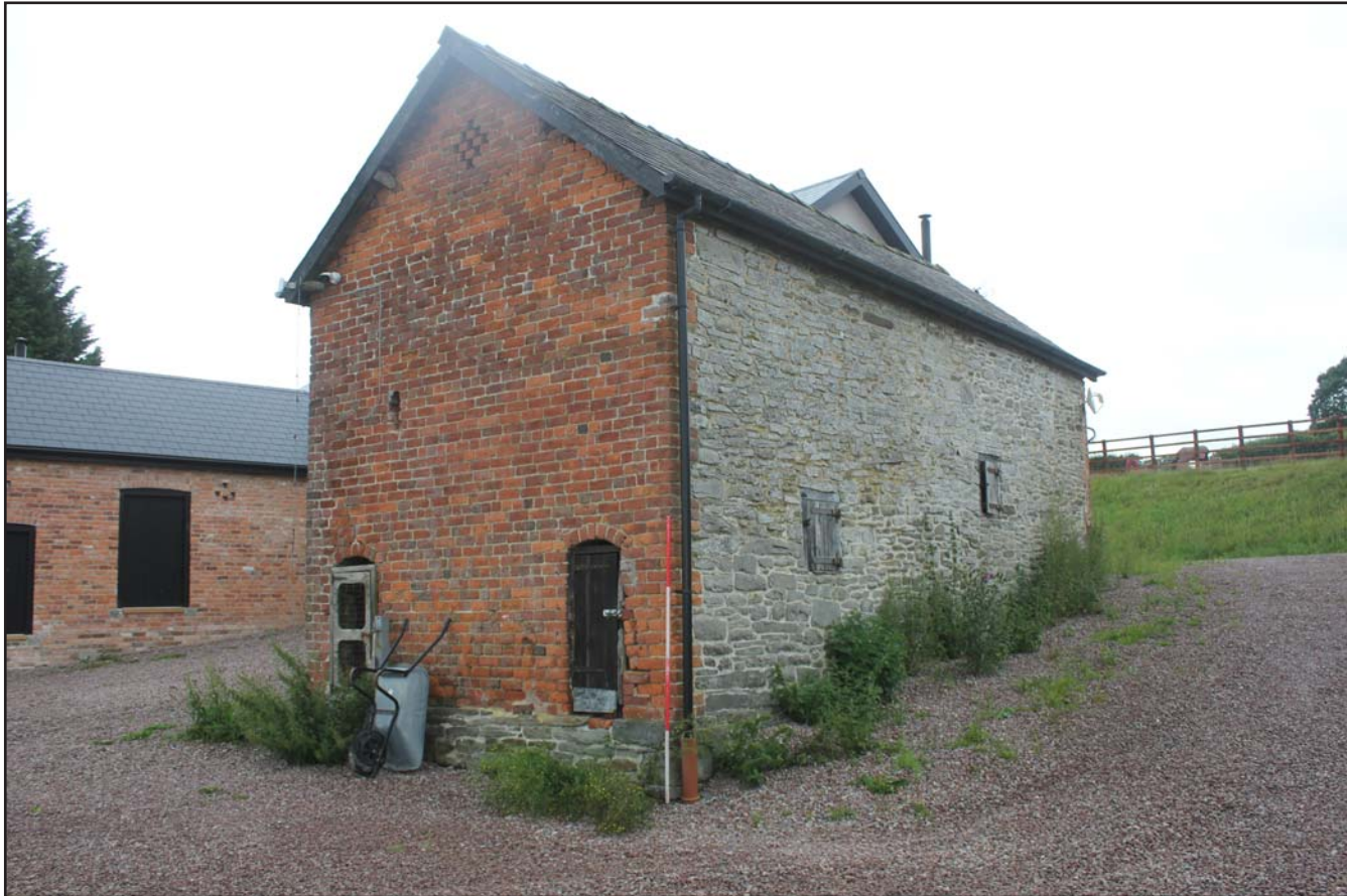
Plate 06: Oblique shot of northern and eastern elevations of the outbuilding at The Birches, Rhos-Y-Meirch, Knighton, Powys - from the northeast - 2.00m scale
