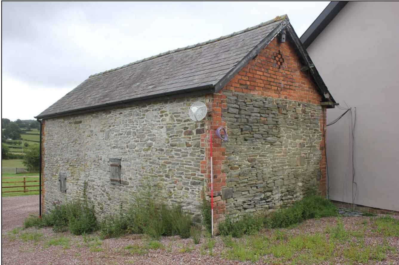
Plate 08: Oblique shot of northern and western elevations of the outbuilding at The Birches, Rhos-Y-Meirch, Knighton, Powys - from the northwest - 2.00m scale
