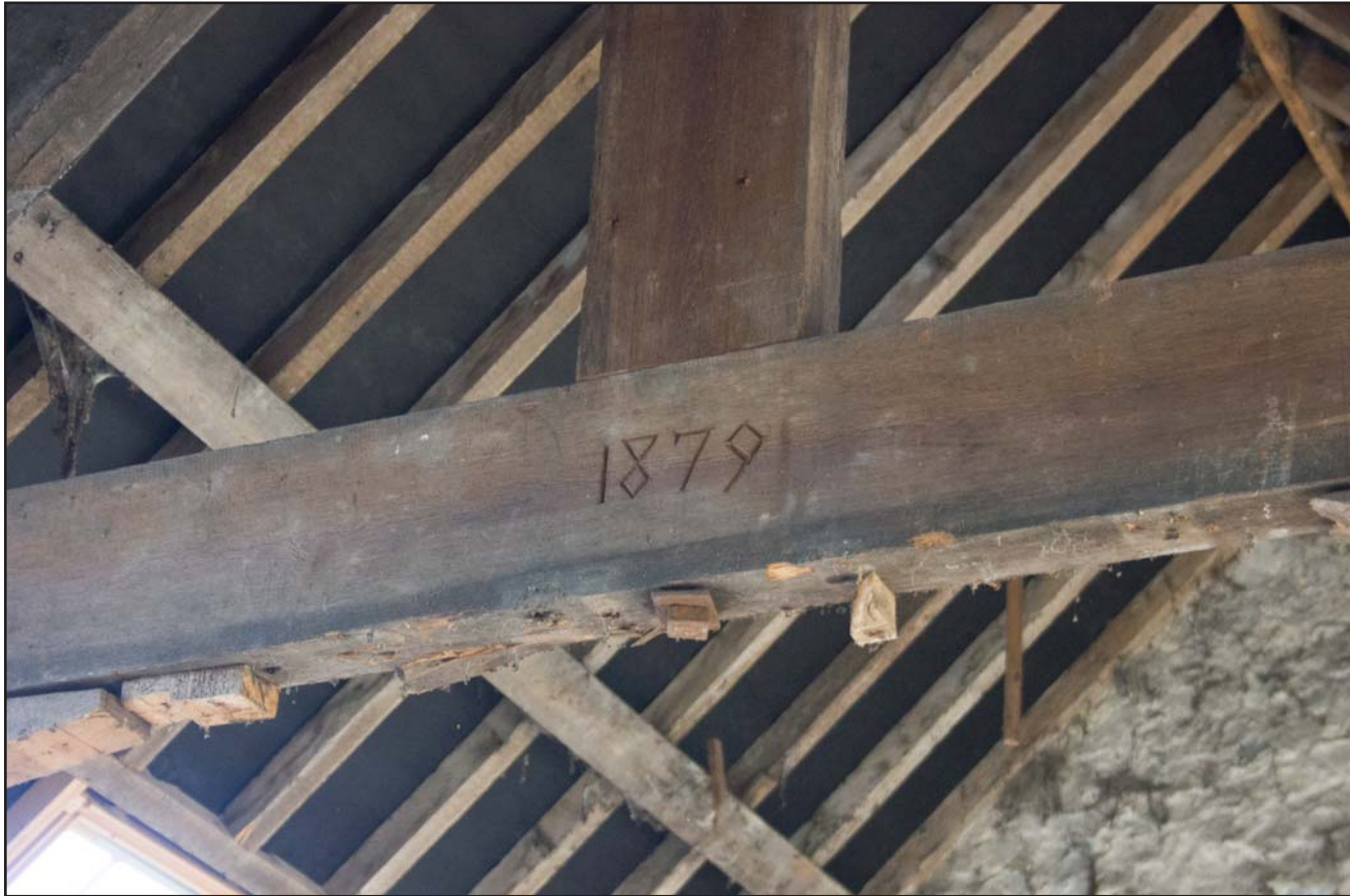
Plate 20: Carved date “1879” on roof truss within Capel Sion, Pontfadog, Llangollen - from the north - no scale
