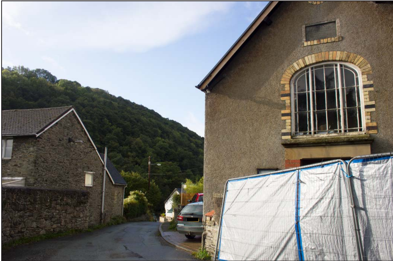
Plate 02: Context shot of Capel Sion, Pontfadog, Llangollen - from the northeast - no scale
