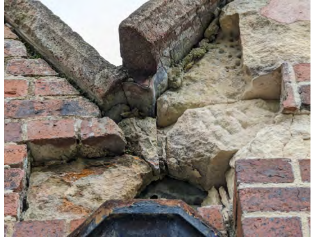
Figure 8 Weathering to the point at which the two gables join
