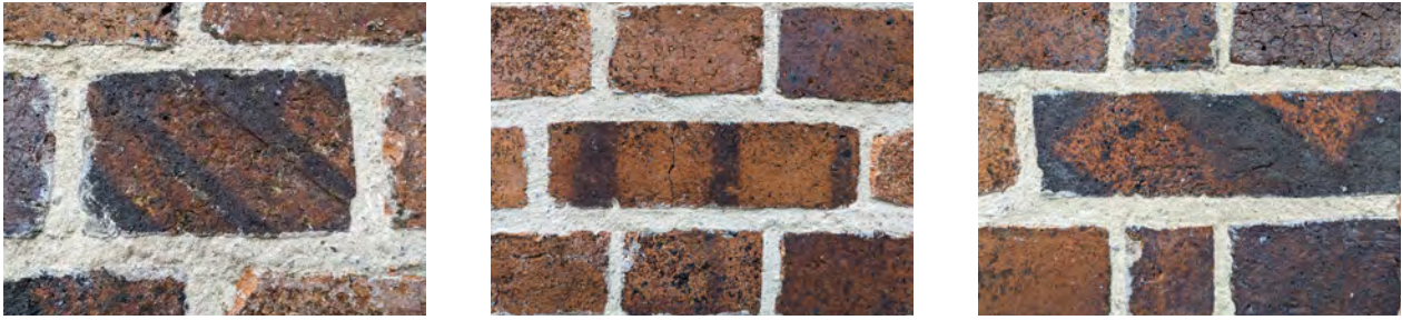
Figure 26 Brickwork patterns
