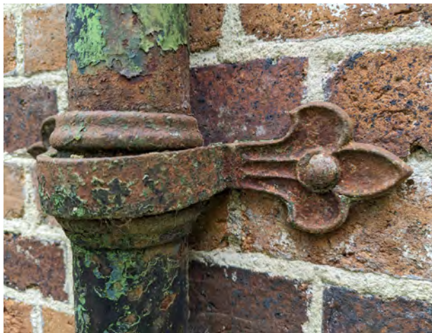
Figure 32 Iron drainage pipes with decorative features
