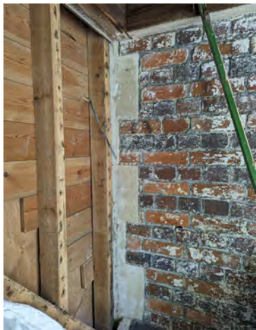
Figure 29 Sandstone door surround of former external doorway
