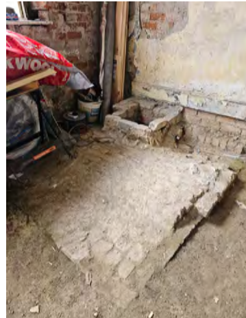
Figure 55 Curved brick ramp atop stone slabs
