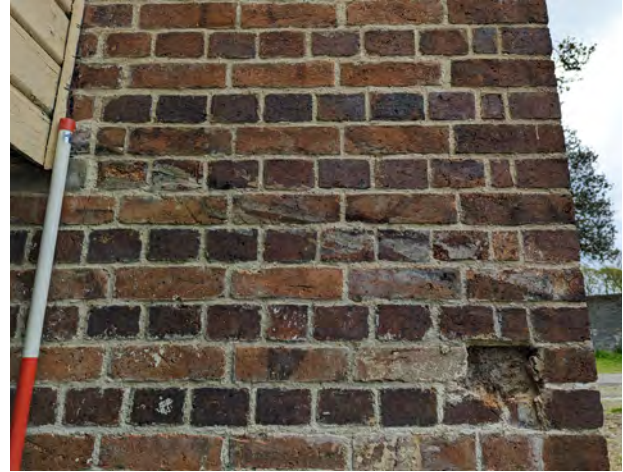
Figure 28 Raggle of former lean-to extension
