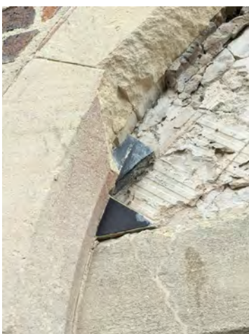
Figure 11 Tympanum with only two dark-blue tiles remaining
