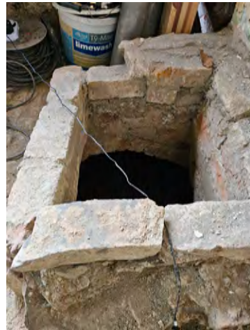
Figure 53 Curved brick inside shaft feature
