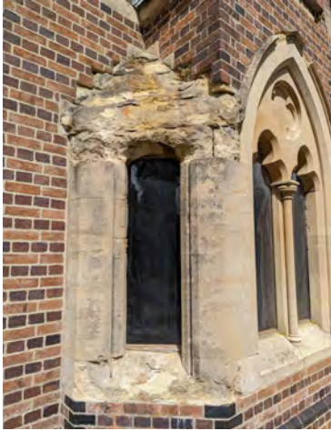
Figure 16 Poor condition of the window bay
