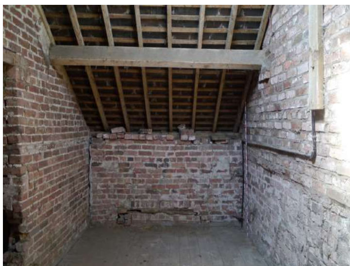
Plate 36 - South-west wall room F1
