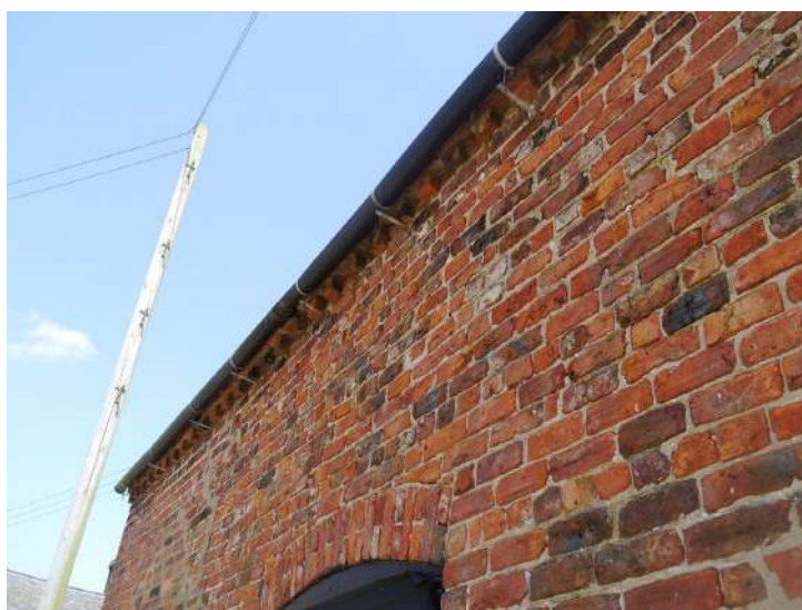
Plate 4 - Dentil top course south- west elevation
