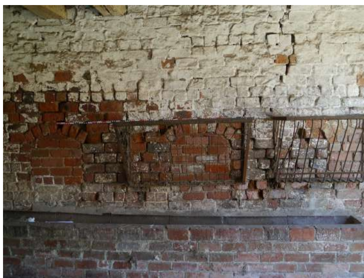
Plate 30 - Three sealed air ventilation features on the south-west wall in room B8
