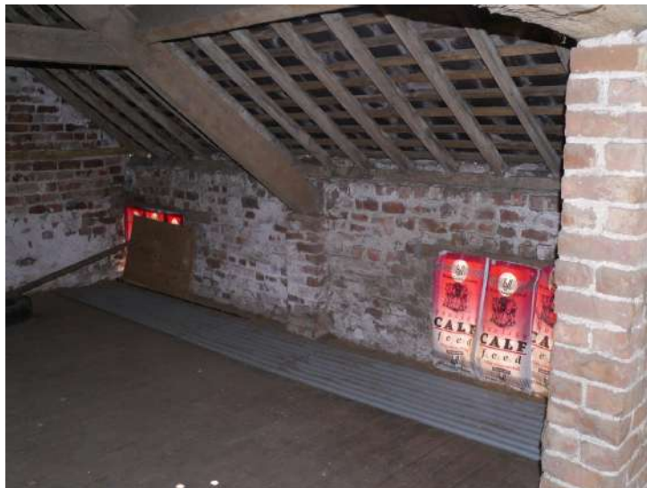
Plate 38 - Two window features and brick wall post
