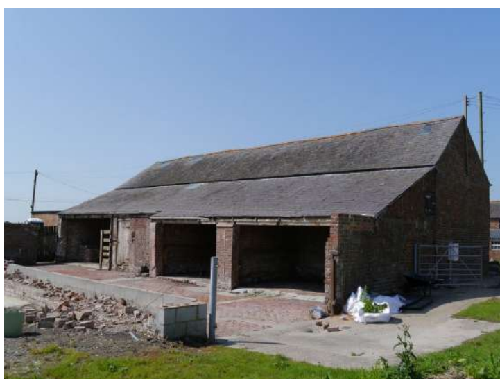
Plate 2 - North-east elevation of rooftop
