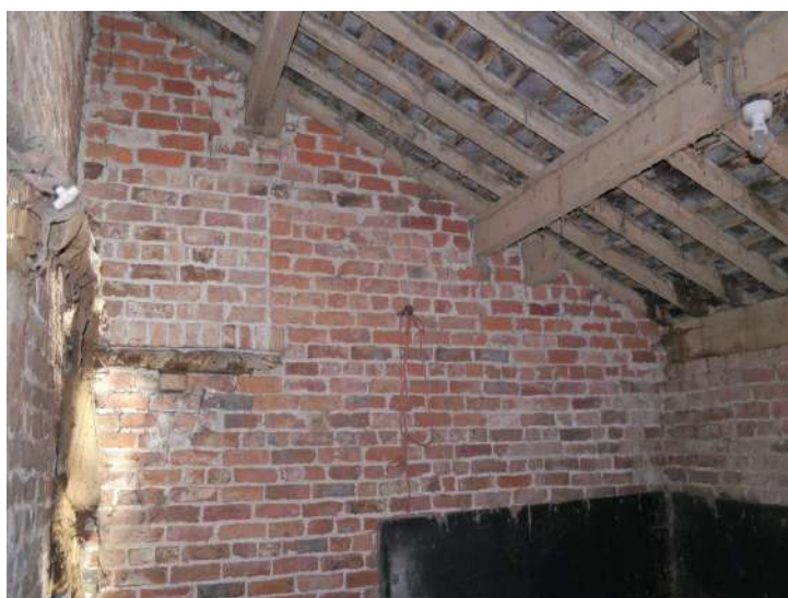
Plate 19 - Sealed air ventilation window north-west elevation room B3
