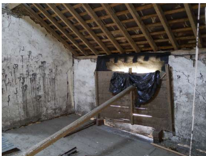
Plate 42 - Window feature room F4
