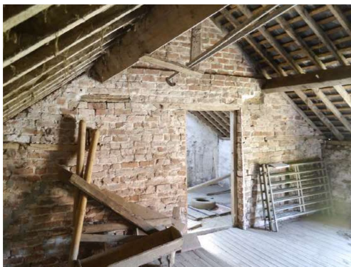
Plate 40 - South-east elevation room F3
