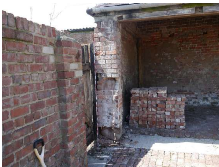
Plate 12 - Sandstone with imbedded iron hinges room B4
