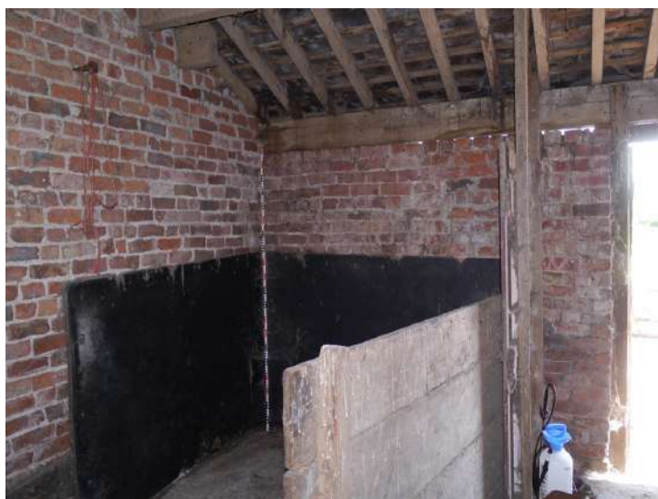
Plate 18 - Internal features room B3
