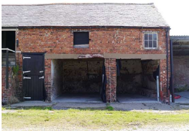
Plate 6 - Threshold of room B8 (left) and B9 (right)
