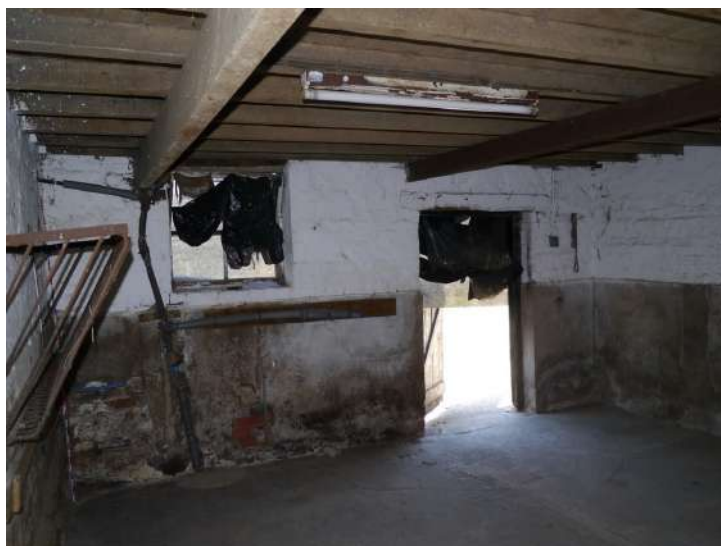
Plate 25 - Threshold and Window on south-west elevation in room B6
