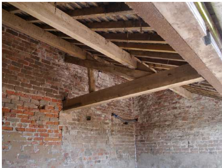
Plate 21 - Open roof with steel joist room B4
