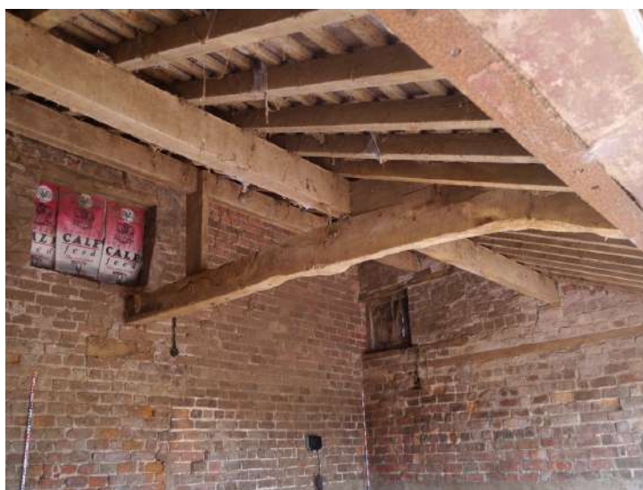
Plate 15 - Air ventilation window north-west wall room B1
