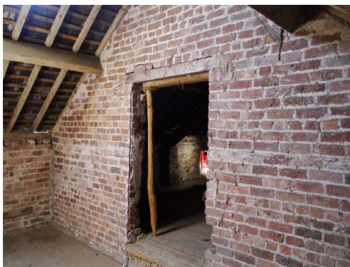
Plate 34 - Threshold south-east wall room F1
