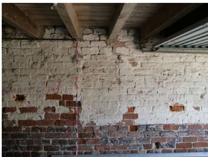
Plate 24 - Sealed air ventilation feature north-west elevation room B5
