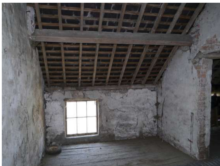
Plate 45 - Window feature south-west elevation room F5
