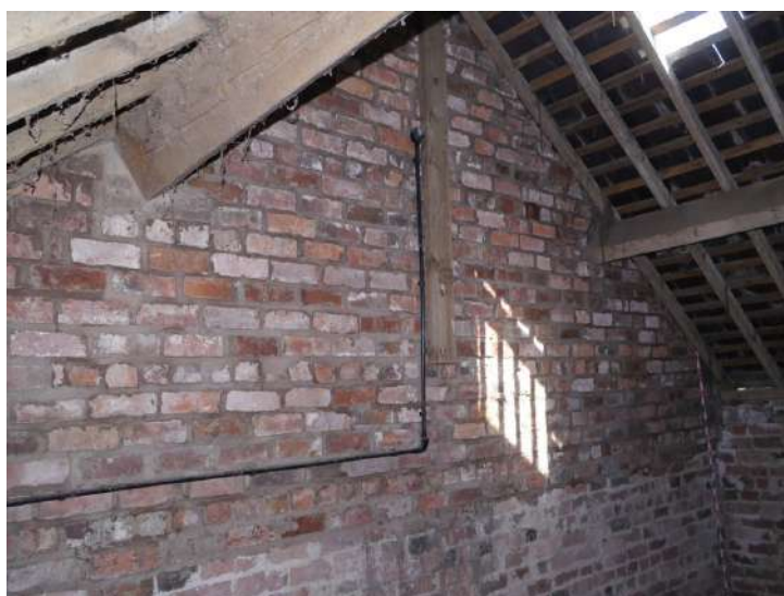
Plate 35 - North-west wall room F1
