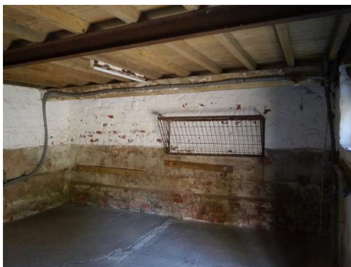
Plate 26 - An iron cast hey rack and concreted stall foundation
