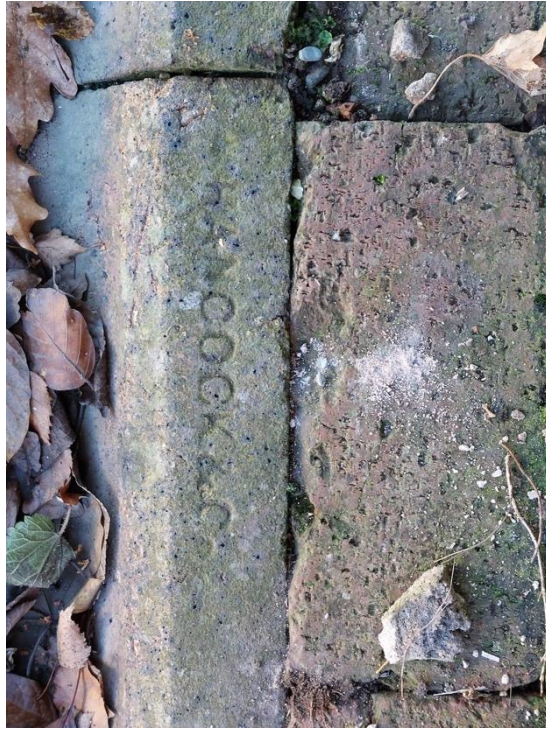
Plate 64 - Detail Shot Showing Frogged Drain
