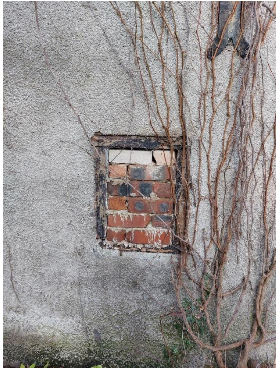
Plate 25 - Bricked up window, South East Facing Elevation
