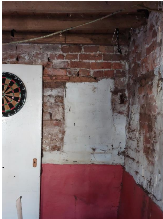
Plate 61 - Detail Shot of Bricked up Window on North West Facing Elevation of Room G5
