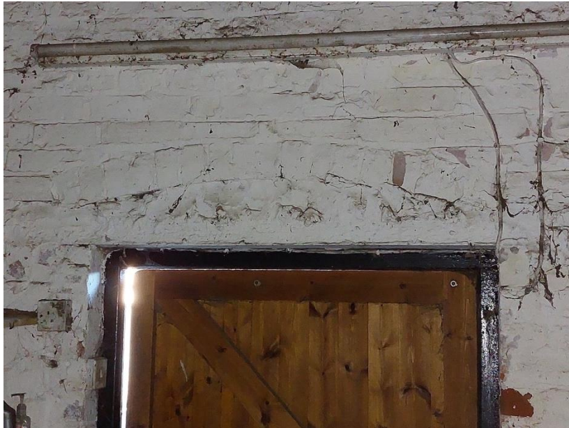
Plate 54 - Detail Shot Showing Brick Flat Arch Above Doorway on South East Facing Elevation of Room G4
