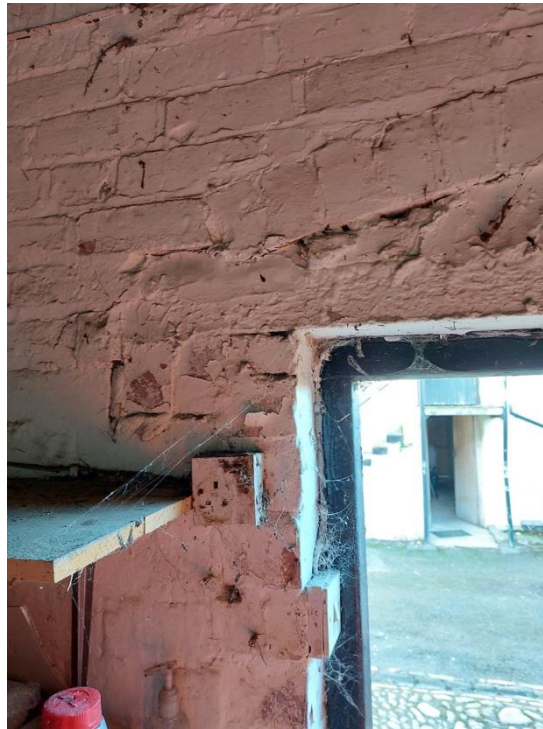
Plate 55 - Detail Shot Showing Modern Brick Used to Narrow the Doorway in G4
