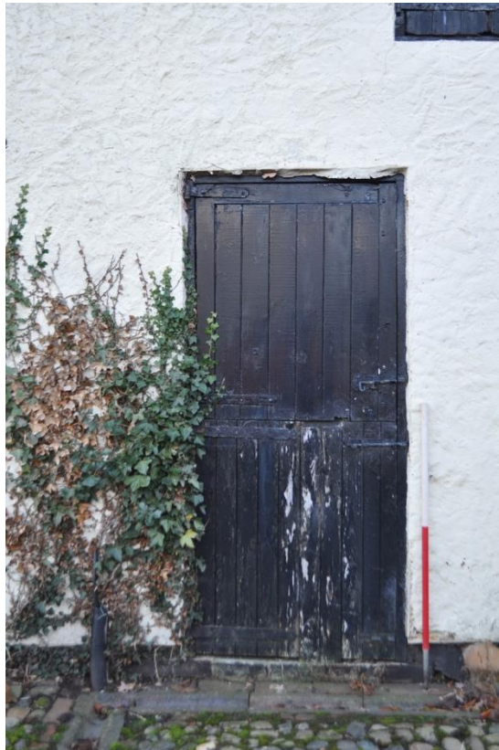
Plate 11 - Dutch Split Door, North West Facing Elevation
