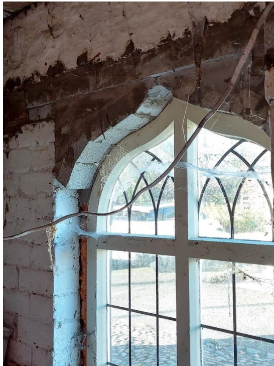
Plate 65 - Detail Shot Showing Modern Materials Used to Fit Ogee Window
