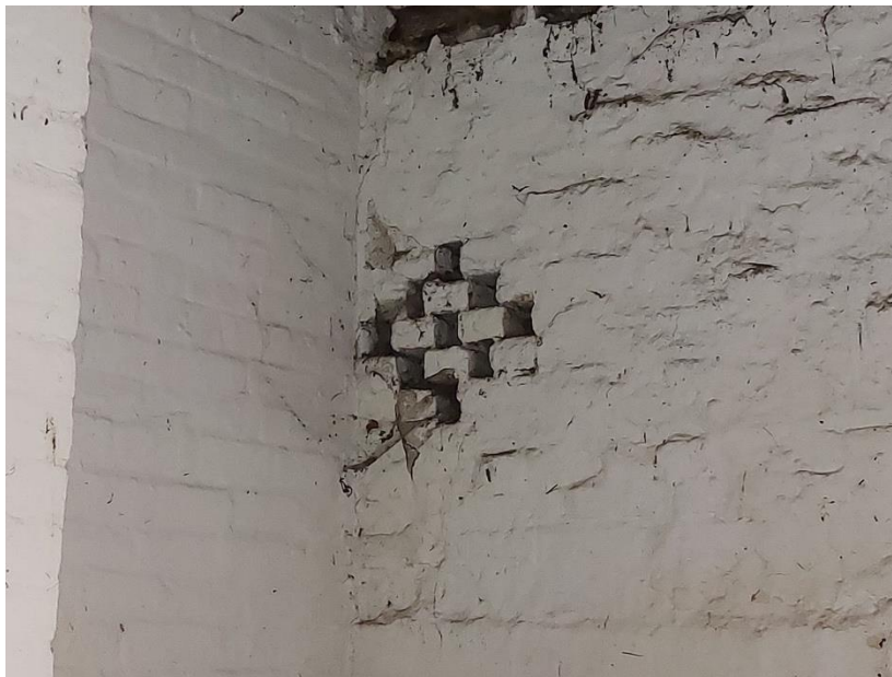
Plate 49 - Detail Shot of Air Vent on North East Facing Elevation of Room G3
