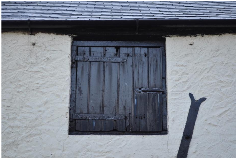
Plate 7 - Upper Window with Wooden Shutter on North West Elevation
