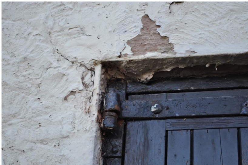
Plate 10 - Iron Fittings on Batten Door, Detail Shot, North West Facing Elevation
