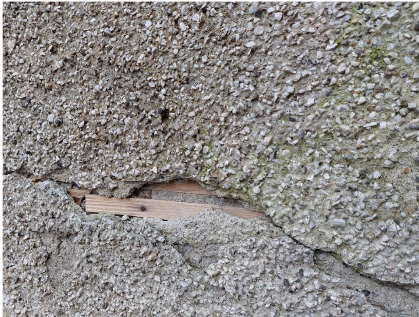
Plate 20 - Detail Shot Showing Lath and Plaster Render on South West Facing Elevation
