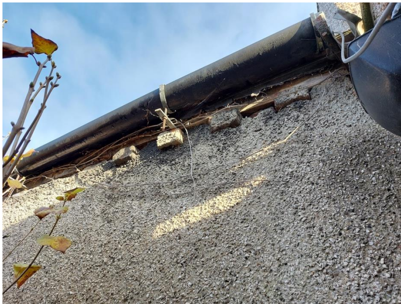
Plate 23 – Dental course brickwork on South West Facing Elevation
