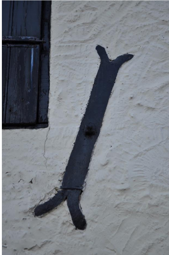
Plate 15 - Detail Shot, Patress Plate, North West Facing Elevation
