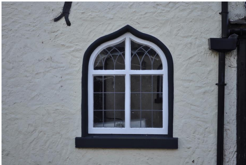
Plate 8 - Ogee Window, Ground Floor, North West Facing Elevation
