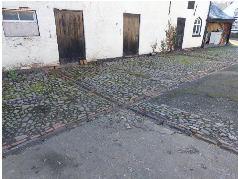
Plate 30 - Exposed Cobbled Surface in Front of North West Facing Elevation
