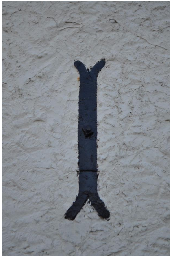
Plate 14 - Detail Shot, Patress Plate, North West Facing Elevation
