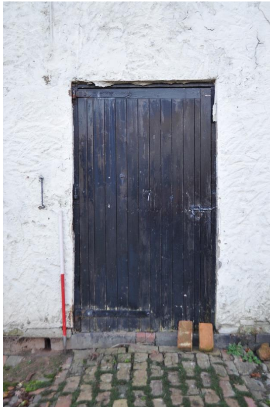
Plate 9 - Batten Door, North West Facing Elevation
