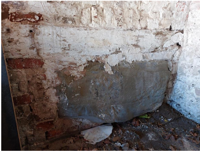
Plate 70 - Detail Shot of Stone Insert and Wooden Lintel on South West Elevation of G6
