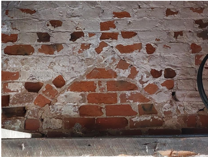
Plate 72 - Detail Shot of Bricked-Up Ogee Window on North East Facing Elevation of Room G6
