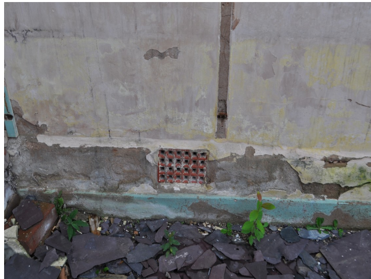
Plate 2- AirVent Brick on Northwest Facing Elevation
