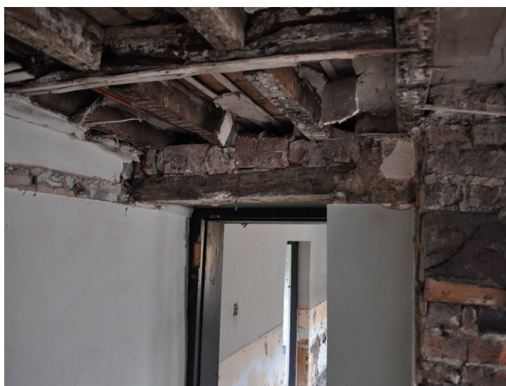
Plate 18-Wooden Lintel Above Doorway on Southwest Facing Elevation of Room G2
