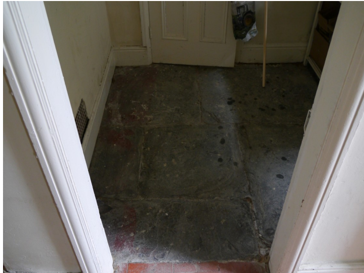
Plate 28 - Stone flag floor in L3 and L4
