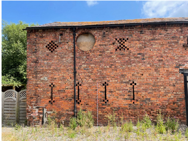
Plate 11 - Air ventilation holes and pitching eye south west elevation of Phase 5
