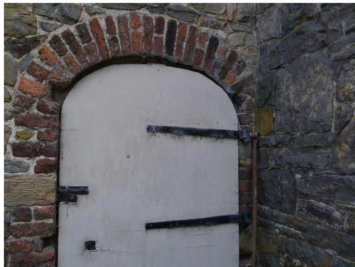
Plate 4 - Phase 2 truncating Phase 1 doorway
