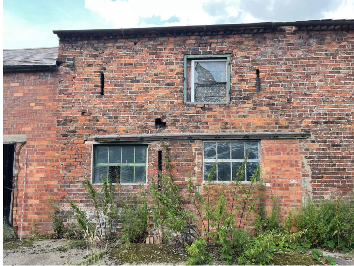
Plate 17 - Sealed doorway and two adjacent window features, north-east elevation of Phase 5
