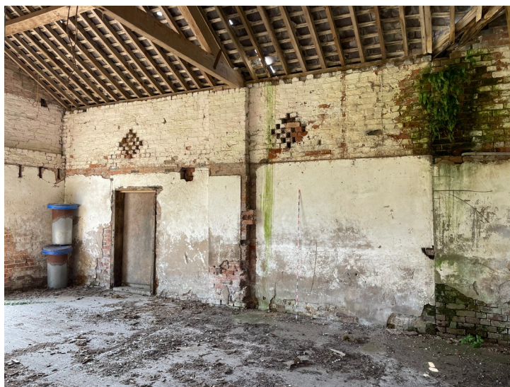
Plate 55 - Doorway and two air ventilation features along south-west elevation Room B9
