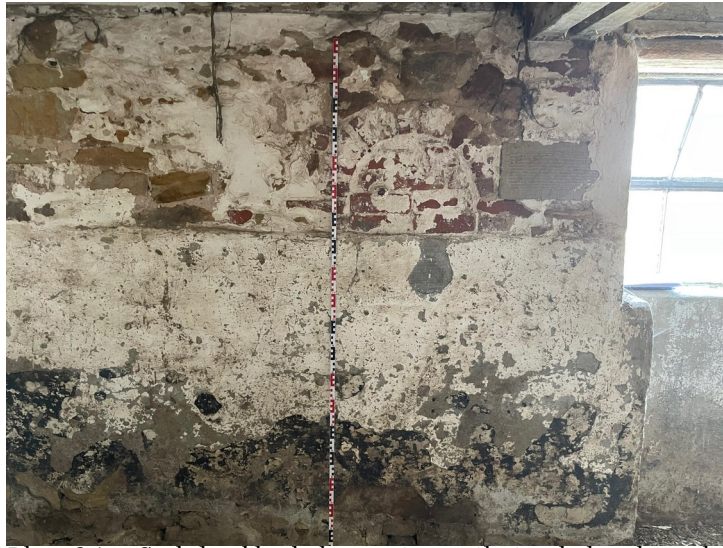
Plate 31 - Sealed cubby holes or air ventilation holes along the north-west elevation in Room B1
