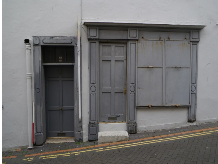
Plate 14 - Doorway to 1 College Street and shopfront for 2 College Street
