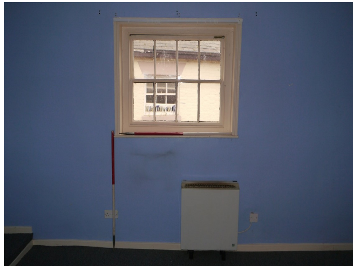
Plate 48 - Window on southern wall of S2
