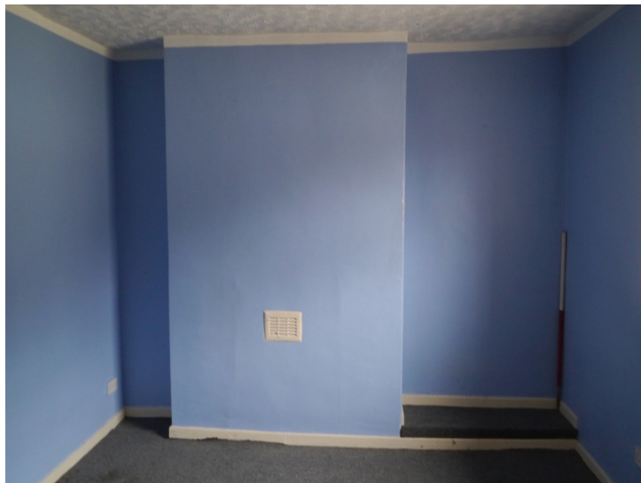
Plate 47 - East wall of S2
