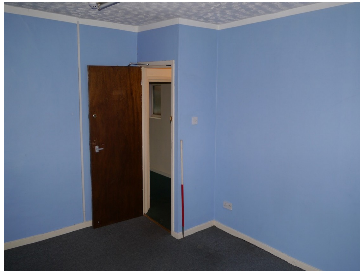
Plate 49 - North wall of S2
