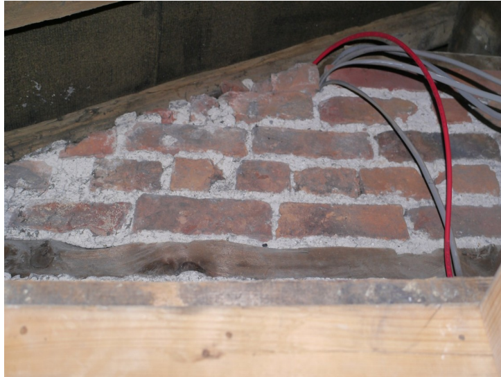
Plate 50 - Dividing wall between 2 and 3 College Street, looking east
