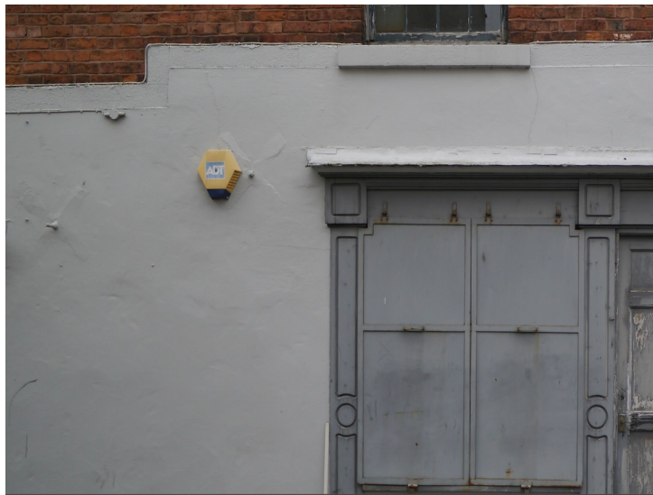
Plate 9 - Wall ties to the west of number 3 shopfront
