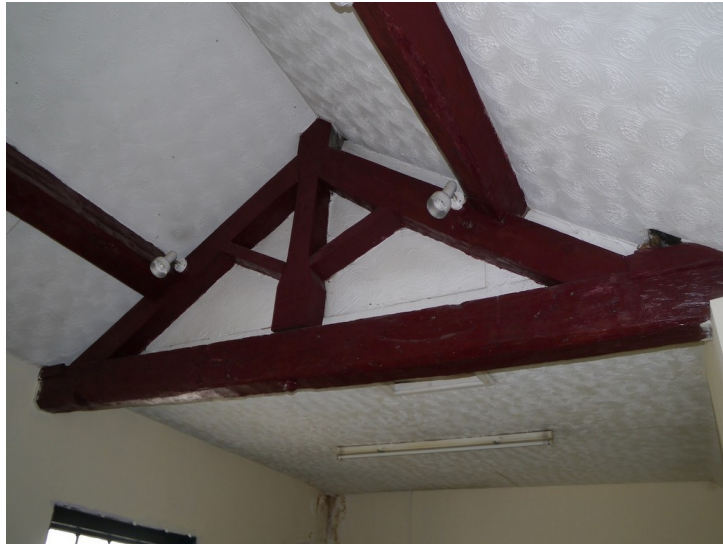
Plate 46 - Ceiling truss in S1, looking southwest
