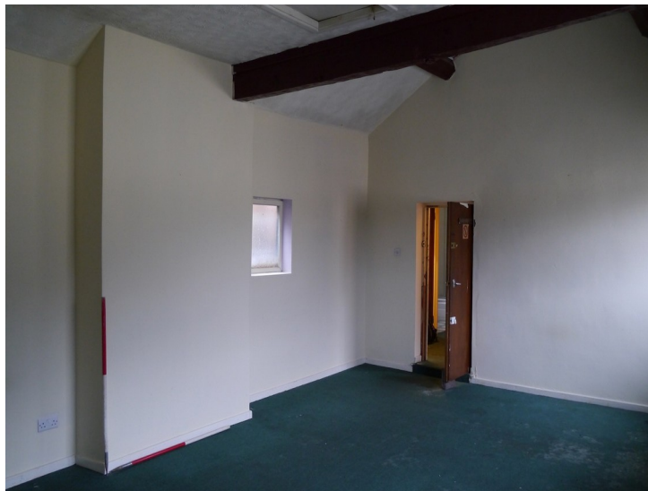
Plate 44 - East wall of S1
