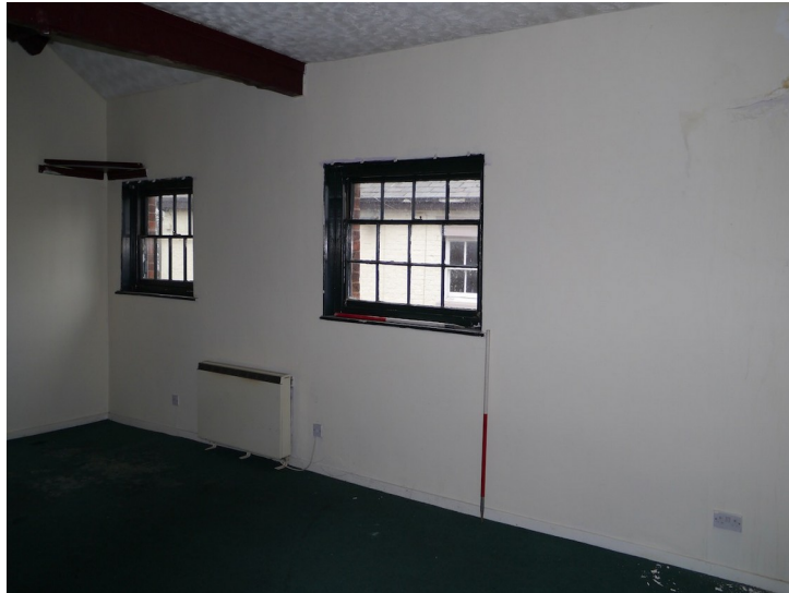
Plate 45 - Windows on south wall of S1
