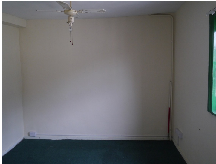
Plate 53 - East wall of S3
