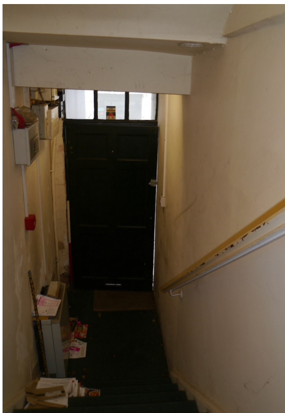
Plate 30 - Room G7, looking south
