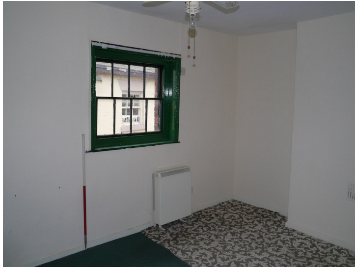
Plate 52 - South wall of S3
