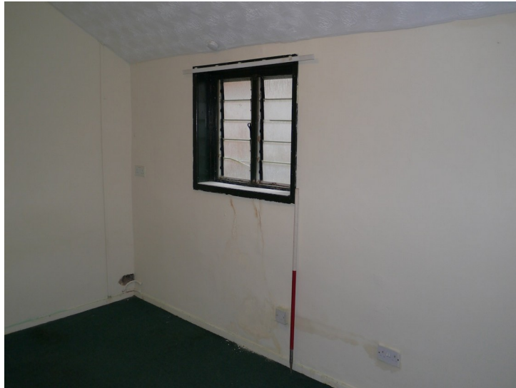
Plate 54 - North wall of S4
