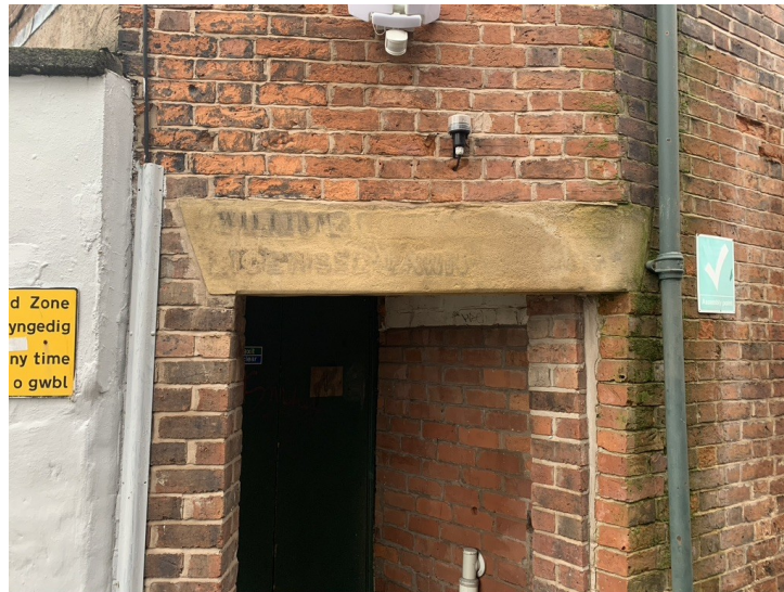
Plate 2 - Pawnbroker lintel to northeast of the study structure
