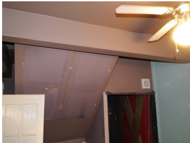
Plate 28 - Ceiling line of G6 showing inserted staircase and boxed in beam
