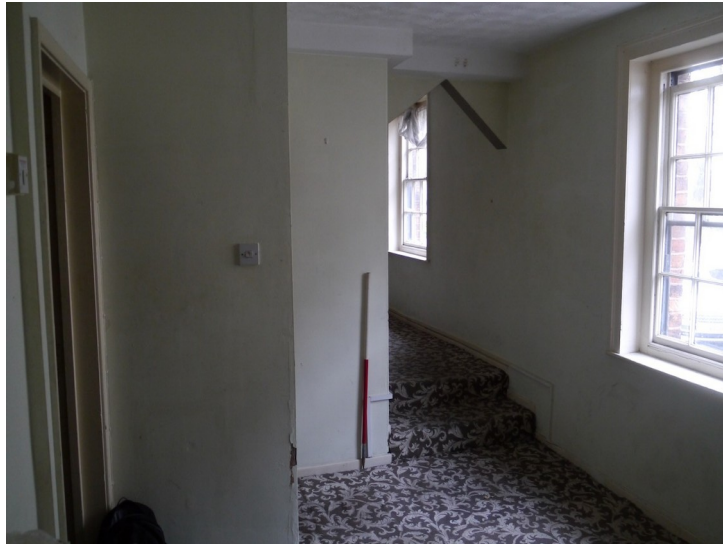
Plate 39 - Room F2, looking southeast
