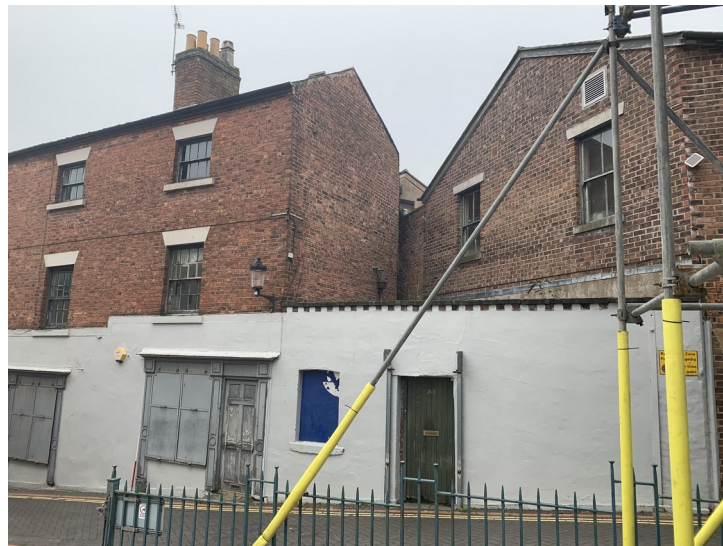
Plate 16 - Eastern extent of southern elevation
