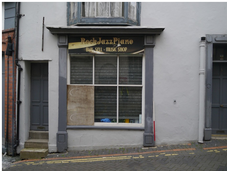
Plate 15 - Shopfront of 1 College Street
