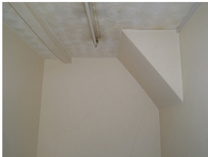
Plate 33 - Ceiling of F5, looking west
