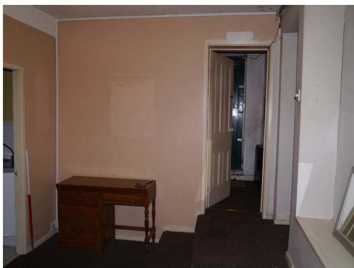
Plate 31 - Access to E2 on east wall of G3
