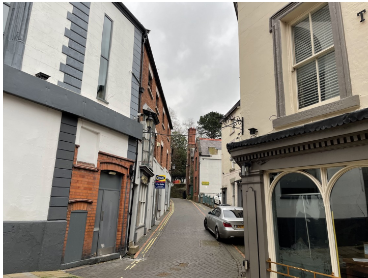
Plate 7 - Junction of 1 College Street with the neighbouring property to the west.
