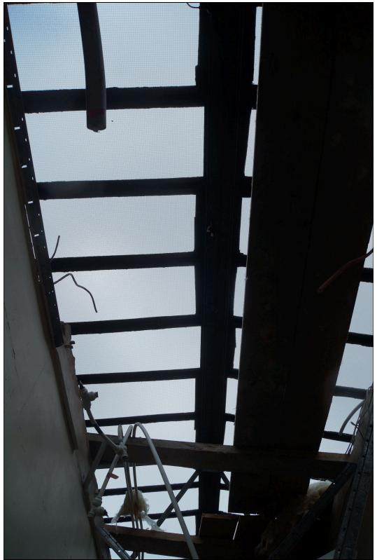
Plate 48: A view of the large skylight taken from inside the lamp room. The glass roof increased the light entering the lamp room, where the important work of preparing safety lamps for miners to take on their underground shift was carried out. Looking southwest.
