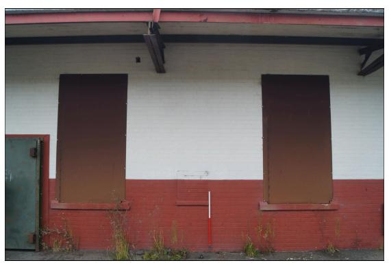
Plate 45: A view of shuttered windows and a bricked-up hatch in the northwest elevation of the lamp room. Looking southeast.
