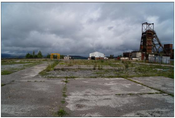
Plate 33: A view of the open area to the southwest of the headframe and engine house at Tower Colliery. The ground here is all built up with deposits of waste dating from the early history of the colliery. Looking north.
