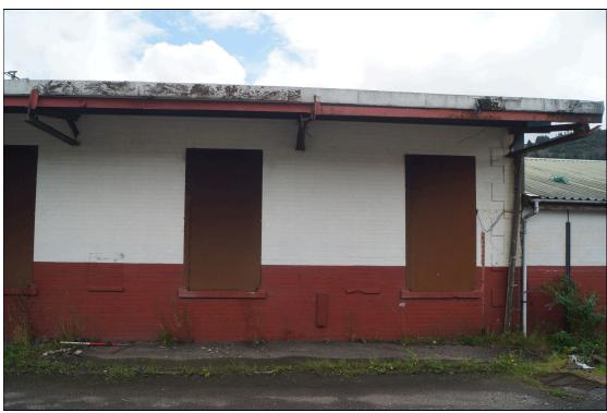
Plate 44: A view of the southern end of the northwest elevation of the lamp room. The large windows of the lamp room are shuttered and the small hatches where safety lamps were passed out to miners walking to the pithead at the start of their shift can be seen as bricked-up features between the shuttered windows. Looking southeast.
