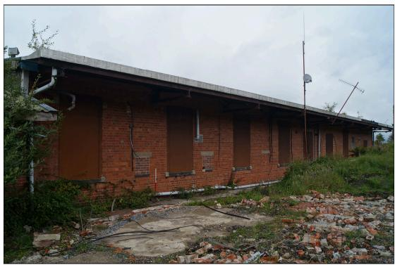
Plate 16: A view of the southeast elevation of the lamp room building (ID Number 13). The three blocked up hatches visible in the wall were the hatches through which miners returned their safety lamps at the end of a shift, protected by the broad overhang of the roof. The large windows, now shuttered, gave good light inside the building. Looking north.
