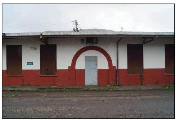
Plate 41: A view of A view of the brick archway in the northwest elevation of the lamp room. An open ended passage ran through the building here, dividing the lamp room to its right from the colliery offices to its right. It was blocked up during the later 20<sup>th</sup> century when the office space was extended. Looking southeast.
