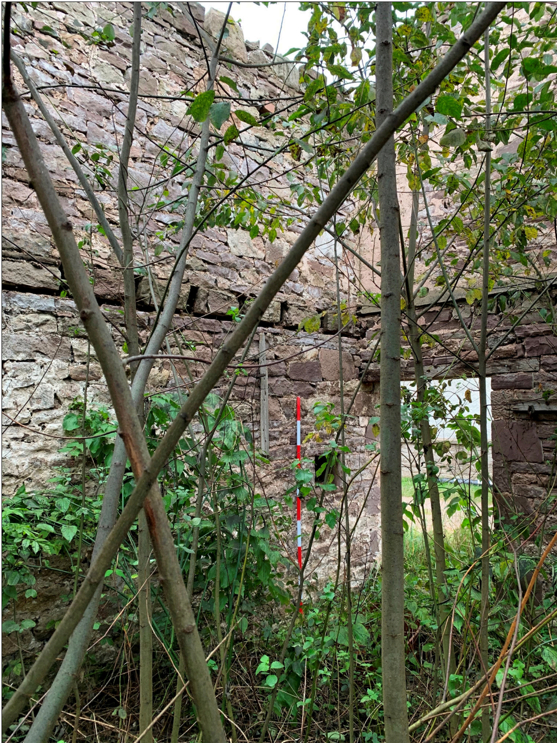
Plate 34: LLN2020_0034 - A view towards the door into the eastern annexe, viewed from inside the building. The joist holes in the northern wall are visible, as is the recess in the northern wall just inside the doorway. Looking northeast.
