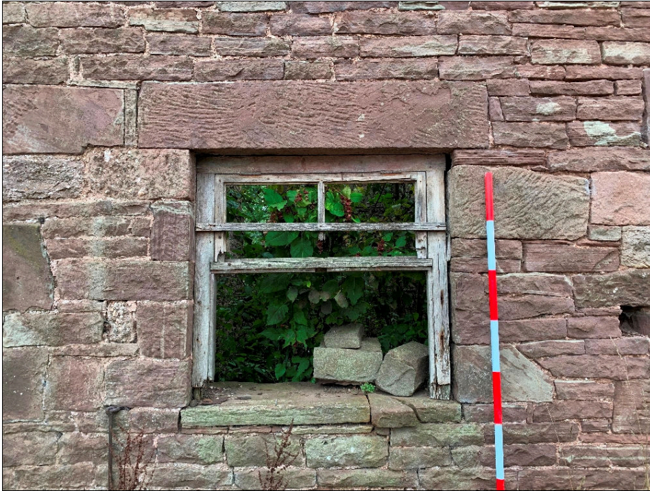
Plate 9: LLN2020_009 - A view of the ground-floor window in the eastern wall of the eastern annexe, showing the remains of the wooden window frame. Looking west.
