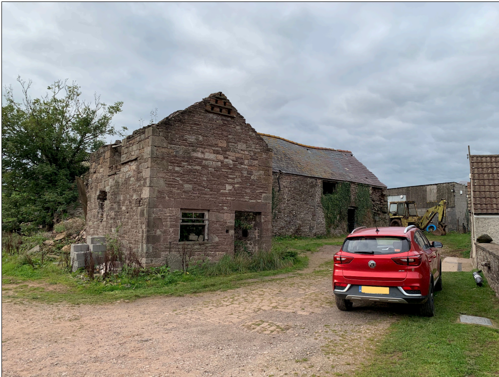
Plate 91: LLN2020_0091 - A view of the barn and cow house complex, with the eastern annexe in the foreground. Looking northwest.
