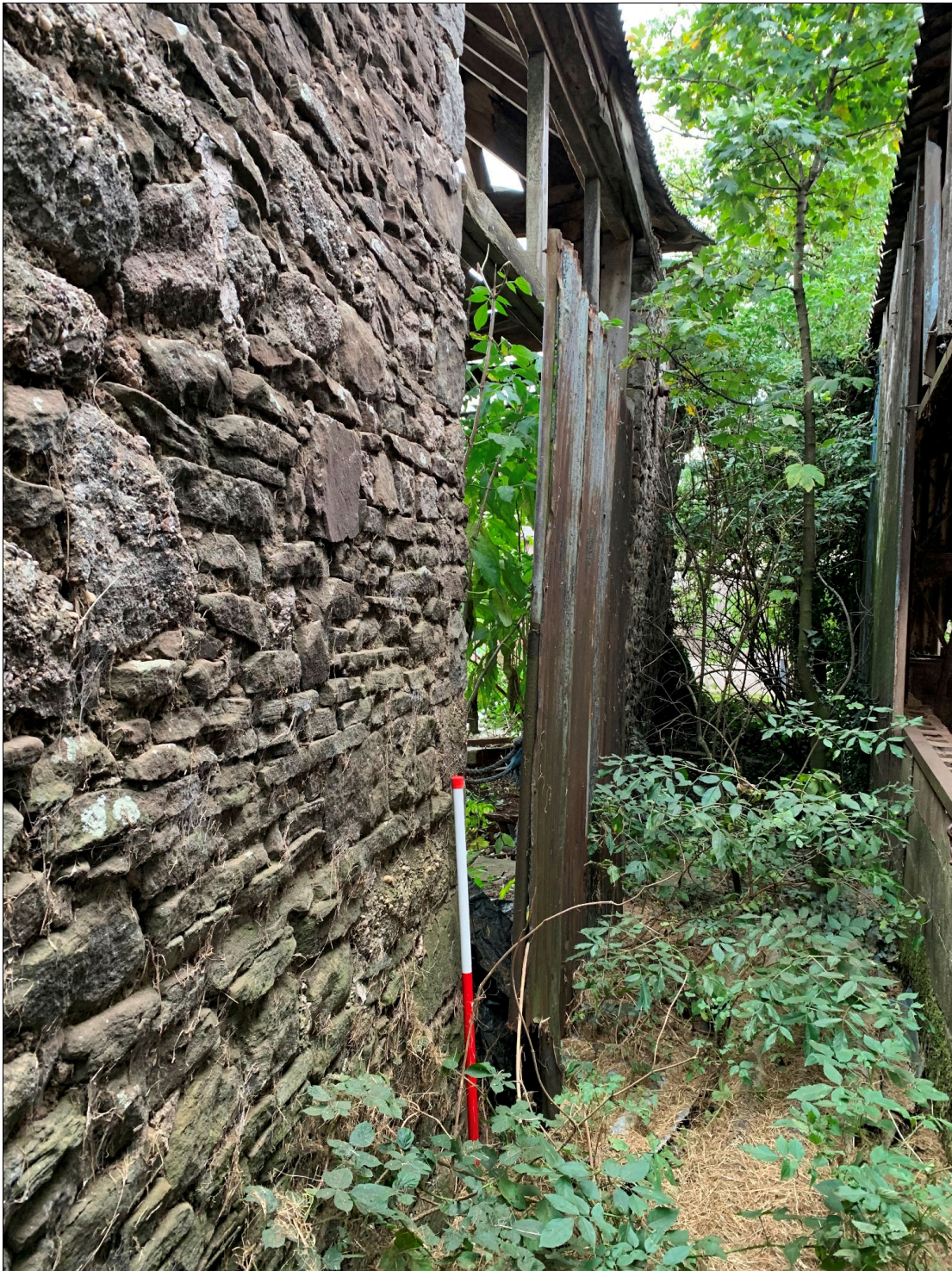
Plate 67: LLN2020_0067 - A view of the western wall of the barn, looking towards the doorway. The modern shed to the west is built close to the barn. Note the use of roughly-coursed sandstone here with some blocks of rough quartz conglomerate visible to the upper left. Looking south-southeast.
