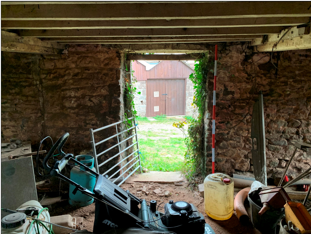
Plate 83: LLN2020_0083 - A view of the central doorway into the cow house. Looking east.
