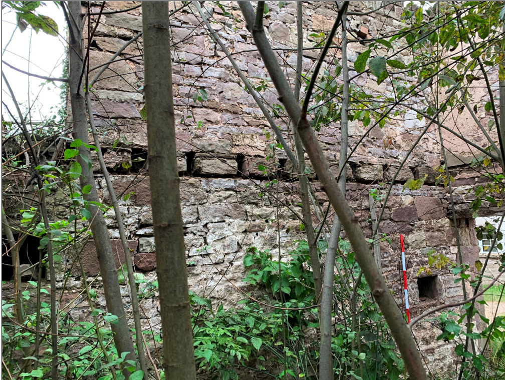
Plate 36: LLN2020_0036 - A view of the joist holes in the northern wall of the eastern annexe. Looking north-northeast.
