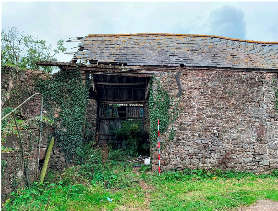
Plate 15: LLN2020_0015 - A view of the large doorway in the eastern side of the barn, with the western doorway visible through it. Note the straight joint to the right edge of the photograph where the cow house is attached to the barn. Also note the break in the slate roof where the southern part of the roof has collapsed. Looking west.
