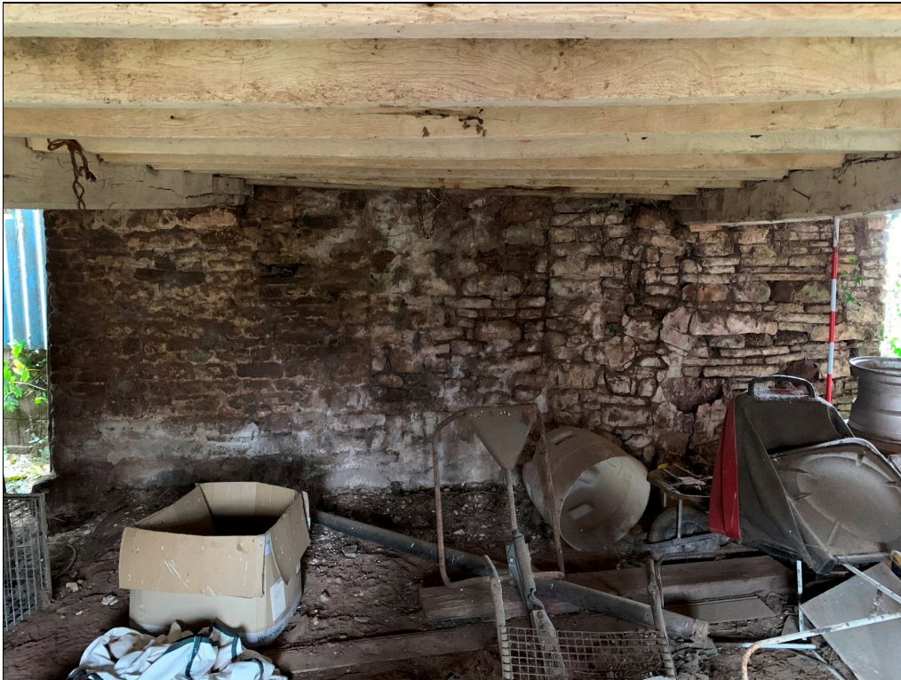
Plate 86: LLN2020_0086 - A view of the blocked-up central doorway in the western wall of the cow house. Looking west.
