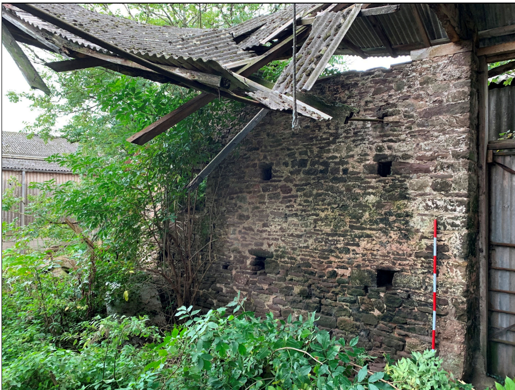
Plate 43: LLN2020_0043 - A view of the western wall inside the barn showing two of the three pairs of ventilation holes in the wall. Looking southwest.
