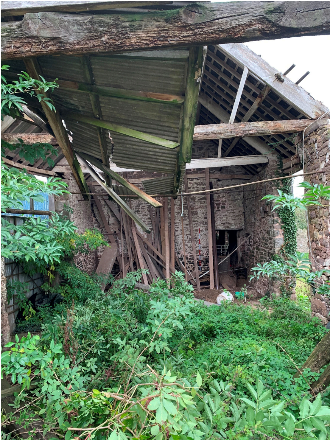
Plate 51: LLN2020_0051 - A view inside the barn. Looking north.
