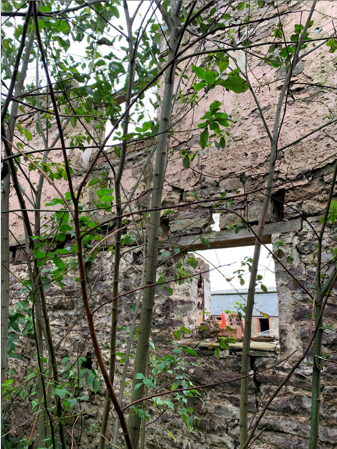
Plate 33: LLN2020_0033 - A view of the joist holes inside the southern wall of the eastern annexe. Looking southeast.
