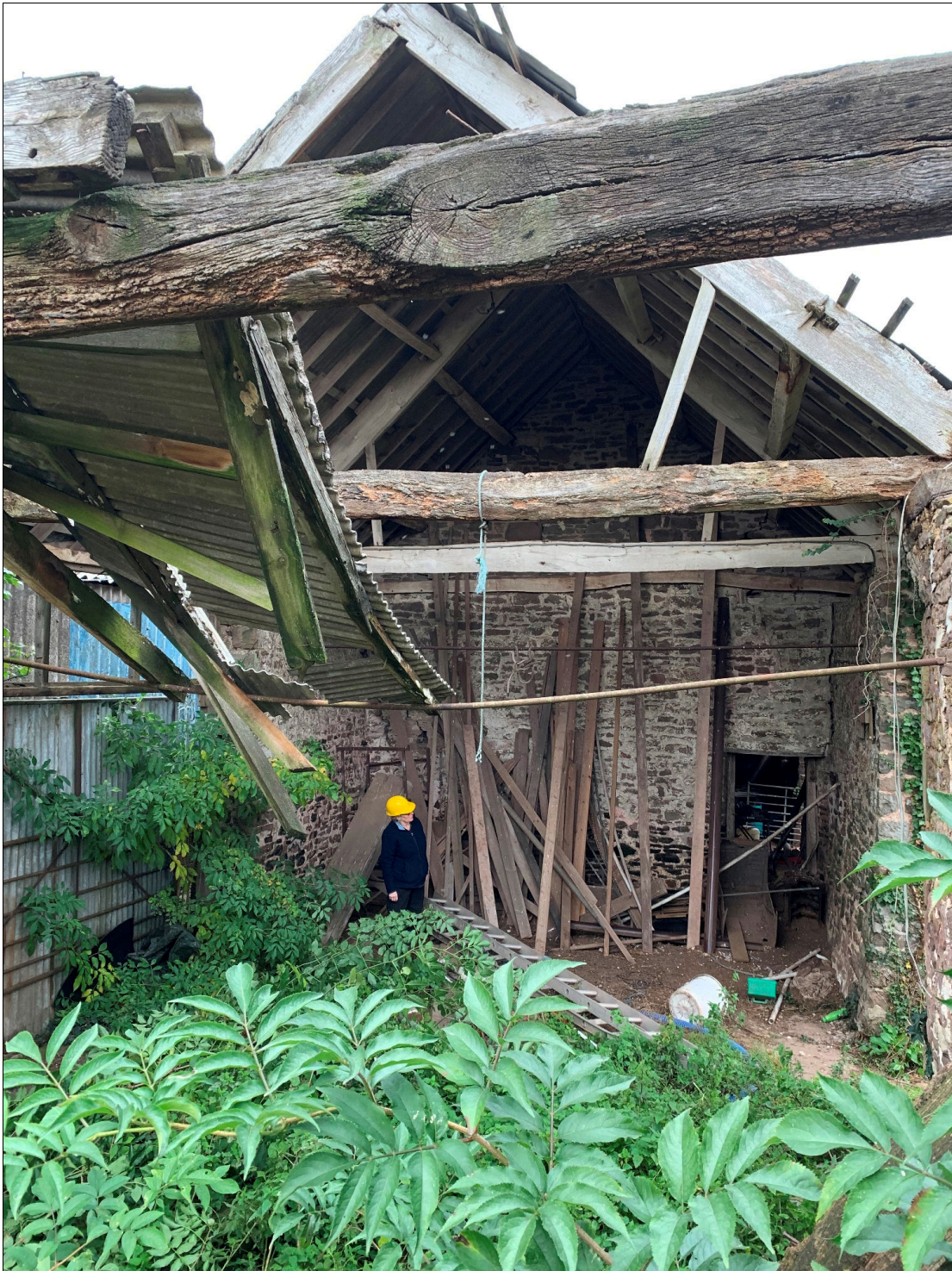
Plate 54: LLN2020_0054 - A view inside the barn. Note the surviving roof trusses towards the northern end of the barn. Looking north.
