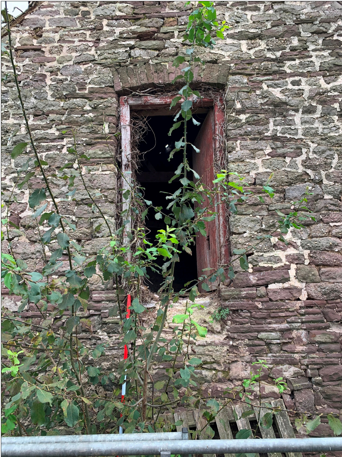
Plate 25: LLN2020_0025 - A view of the doorway into the upper floor of the cow house in the northern gable wall. This doorway also has a red sandstone arch above the doorframe. Looking south.
