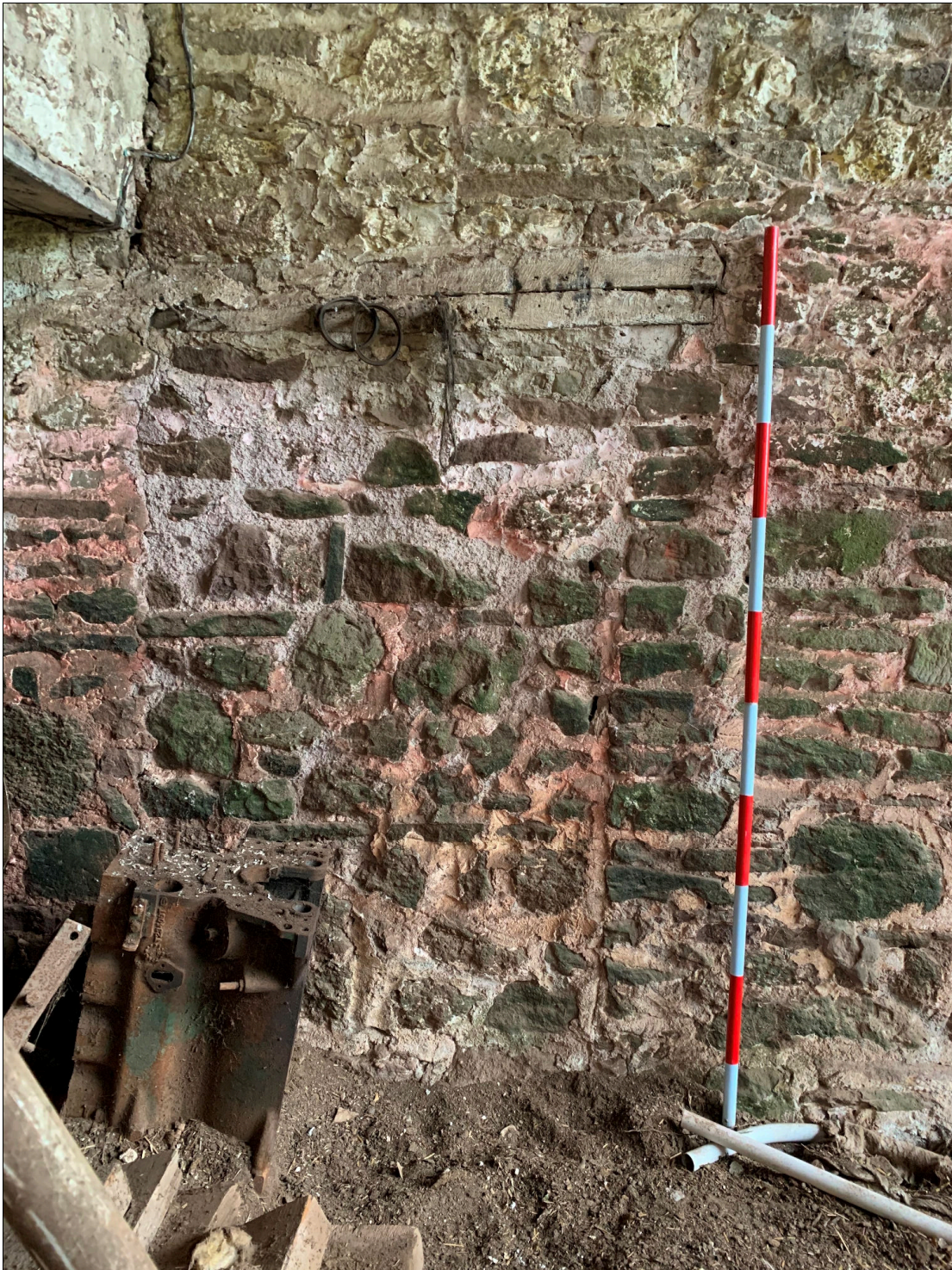
Plate 63: LLN2020_0063 - A view of the blocked-up doorway through the eastern wall at the northeastern corner of the barn. Looking east.
