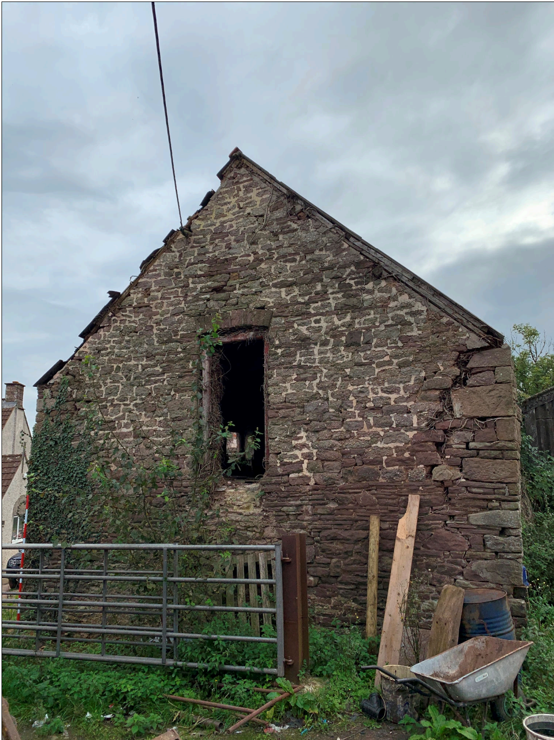
Plate 22: LLN2020_0022 - A view of the northern gable end of the cow house. Red sandstone slabs were used to construct the ground floor wall, with harder quartz conglomerate used for the upper floor. Looking south-southeast.
