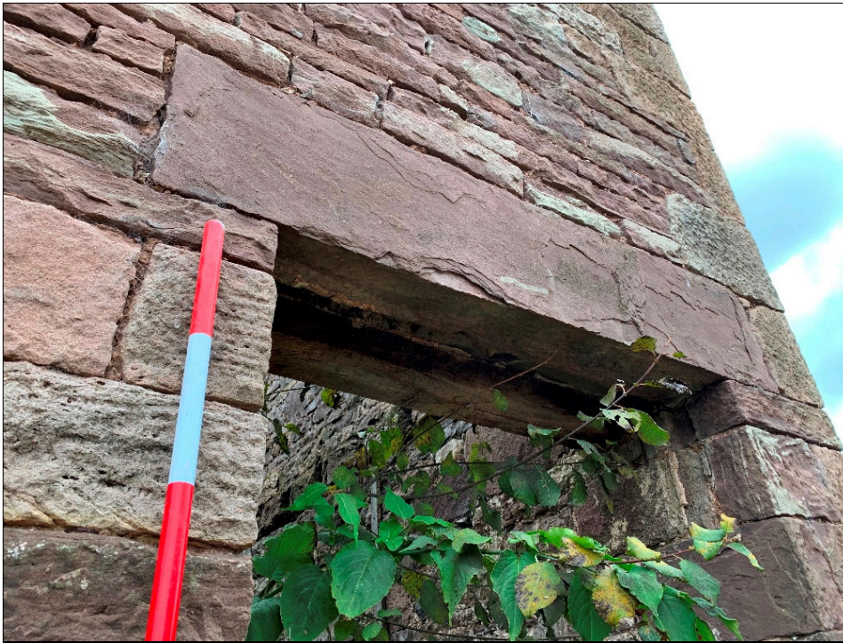
Plate 11: LLN2020_0011 - A view of the lintel above the doorway into the eastern annexe, showing the wooden lintel behind the stone slab. Looking northwest.
