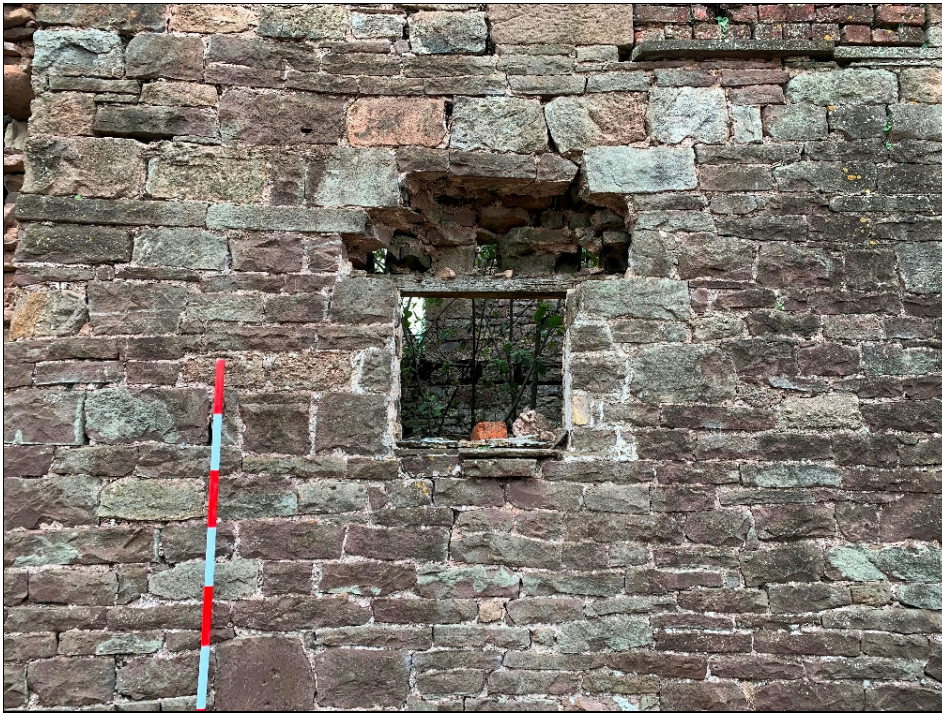
Plate 7: LLN2020_007 - A view of the small ground-floor window in the southern wall of the eastern annexe. The lintel has been removed. Looking north.
