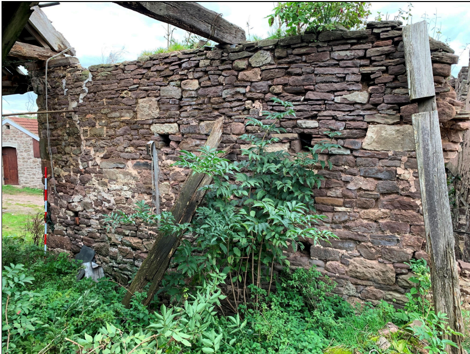
Plate 46: LLN2020_0046 - A view of the eastern wall inside the barn, showing the ventilation holes, some of which have been blocked in the past. Looking northeast.
