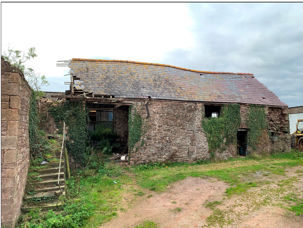
Plate 94: LLN2020_0094 - A view of the barn and cow house. Looking west-northwest.
