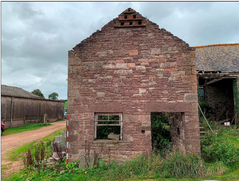
Plate 8: LLN2020_008 - A view of the eastern gable wall of the eastern annexe, showing the door and ground level window. Note the dove holes at the top of the wall. Looking west.
