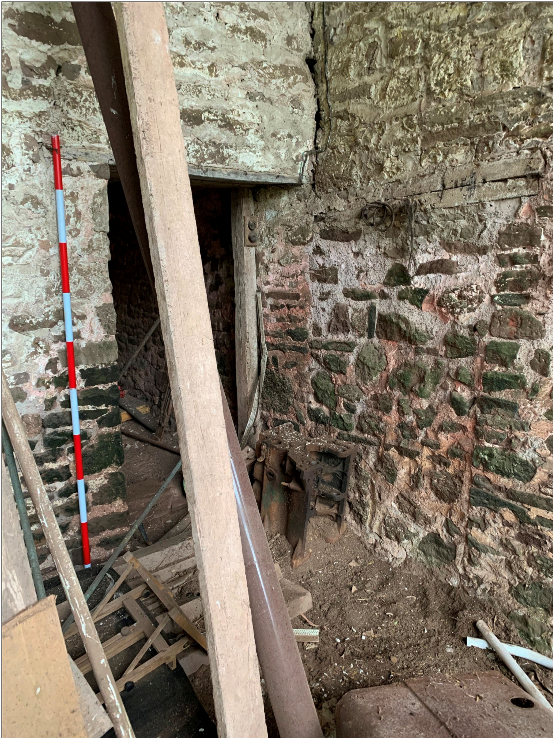
Plate 62: LLN2020_0062 - A view of the blocked-up doorway through the eastern wall at the northeastern corner of the barn. Looking northeast.
