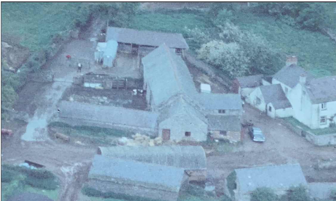
Figure 6: An aerial photograph of Llan y Nant taken c.1970.
