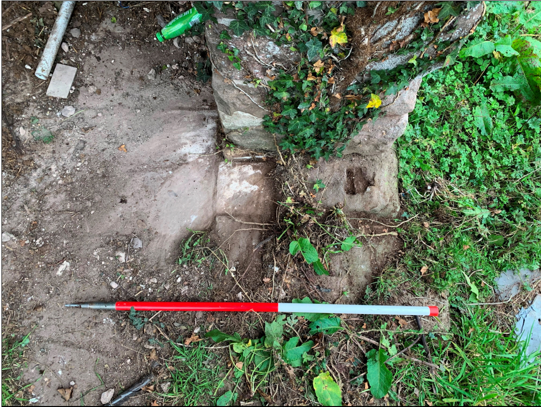
Plate 64: LLN2020_0064 - A view of a niche in a stone at the base of the wall at the north side of the eastern barn door. Note the stone slabs forming the floor to the left. Looking north.
