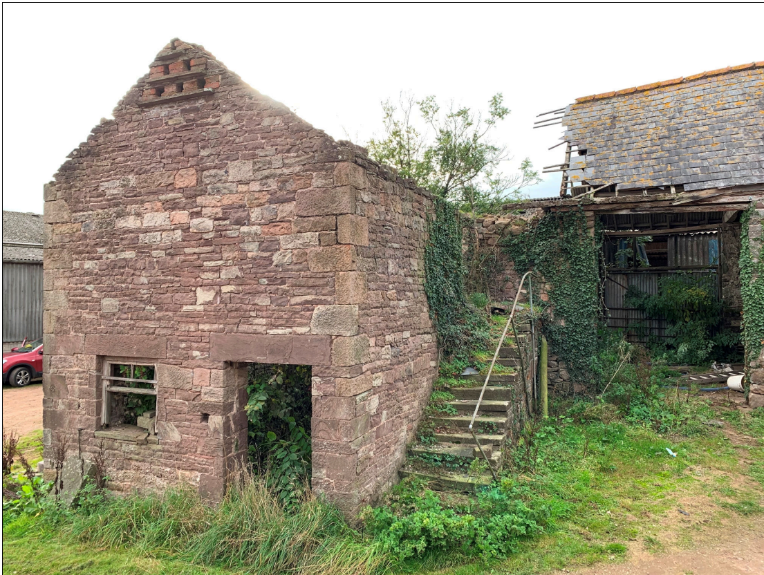
Plate 95: LLN2020_0095 - A view of the eastern annexe. Looking west-southwest.
