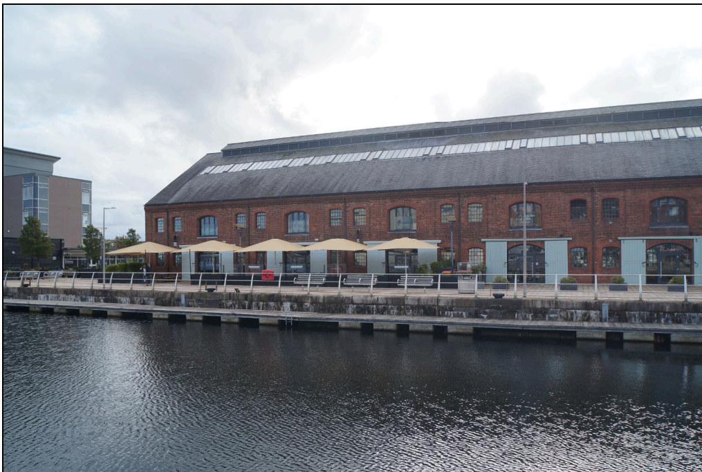
Plate 2: JSH2020_002. The southern end of the eastern side of the J Shed showing altered roofline and skylights, looking south-southwest. The pergola would not be visible in this view. The umbrellas provide a visual line along the building where the wooden gangway was attached originally.
