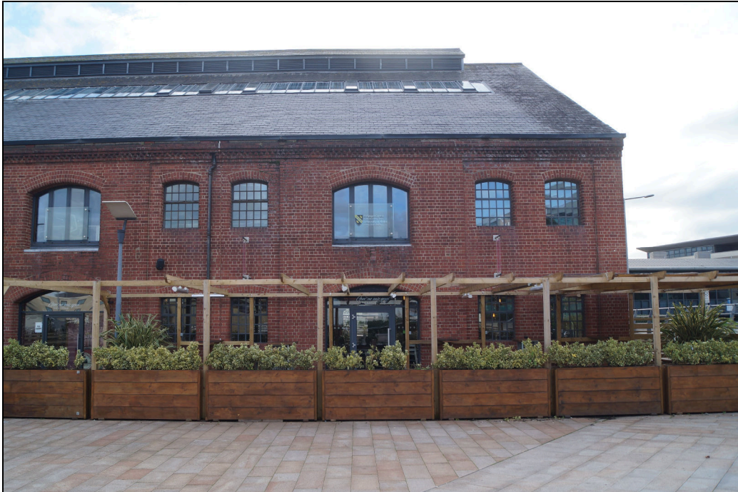
Plate 17: JSH2020_017. Looking west-southwest at the northern end of J Shed and the pergola. Almost all of this end of the building was rebuilt from foundations in the late 1950s.
