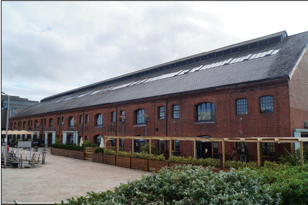
Plate 5: JSH2020_005. The eastern side of the J Shed, looking south. It can be seen here that the pergola in front of Unit 1 does not significantly screen views of the listed building. Note the modern roof. The original roof was a plain, slate roof with no vents or windows.
