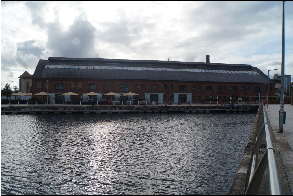
Plate 1: JSH2020_001. A view of the eastern side of the J Shed across the acute angle of Prince of Wales Dock, looking southwest. The chimney of the ice factory, also a Listed Building, can be seen above the roof. The building was converted in 2005 which included addition of the row of skylights and the ridgeline ventilation.
