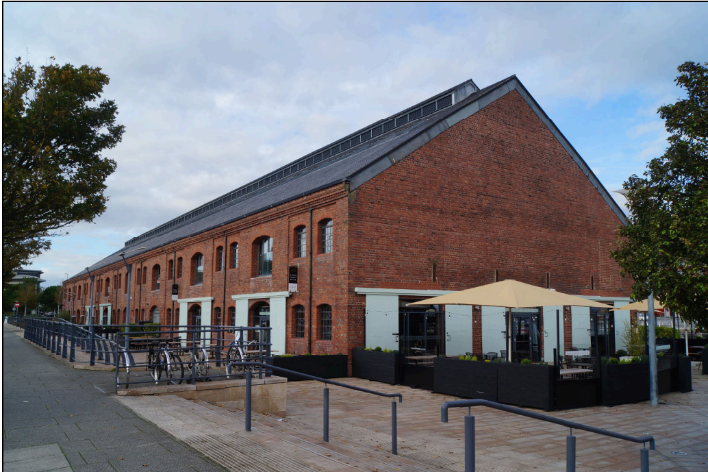
Plate 9: JSH2020_009. Looking northeast at the southern end of J Shed, showing modern street furniture and seating.
