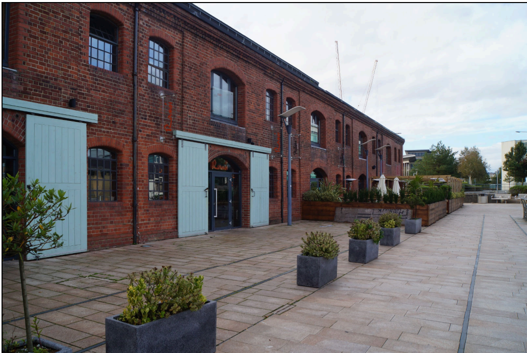
Plate 14: JSH2020_014. The central and northern part of eastern side of the J Shed, looking northwest. The pergola can be seen but does not obscure the view of the building.
