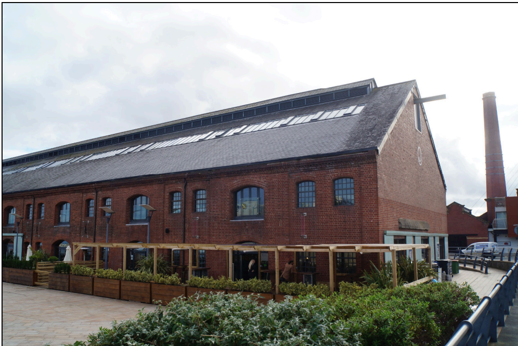
Plate 4: JSH2020_004. The northern end of the J Shed with the pergola in place, looking southwest. This end of the building, including the first set of doors, has been rebuilt after bomb damage during the war. The chimney of the early 20 th century ice factory is visible to the right – another of the very remaining original buildings in the dock area.
